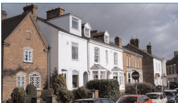
Inappropriate dormer windows by the War Memorial
