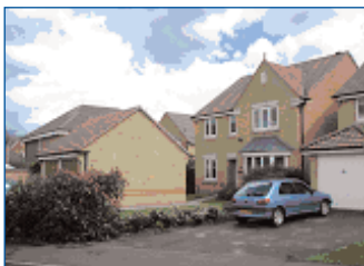
Poorly positioned detached garage
