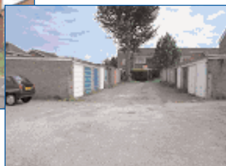
Communal garages Azalia Drive
