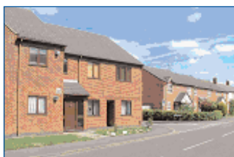
Inappropriate 1990s infill development
