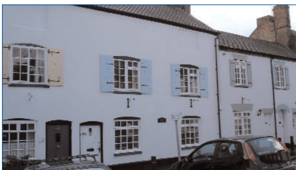
Cottages with inappropriate window shutters
