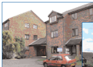
Flats in Willow Close off Pyeharps Road
