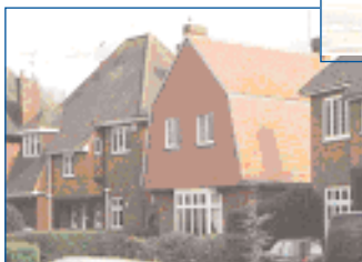
Older houses in Sapcote Road
