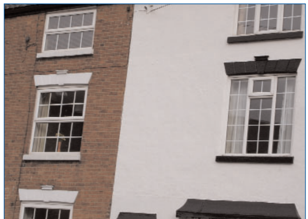
Windows with stone lintels and sills. Window lintels featured have raised keystones
