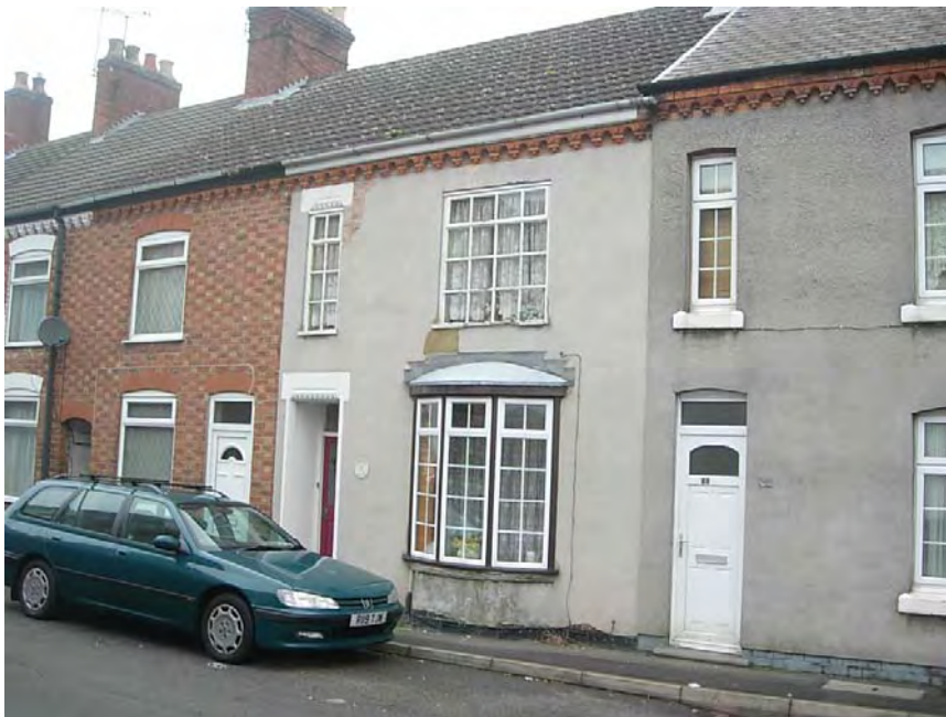
Number 21 New Street is a distinctive property due to the ground floor bay window and wooden window frames at first floor level. This property was originally the foreman's house for the former factory at 6 New Street, and therefore has a slightly widened front elevation.
