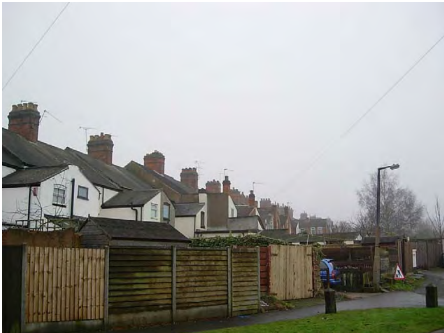
Viewing the rear of the residential terracing on Hinckley Road from Heath Lane South provides an excellent aspect of the roof ridge line as the dwellings were constructed up the road, and the many examples of original chimney stacks and pots can clearly be seen.
