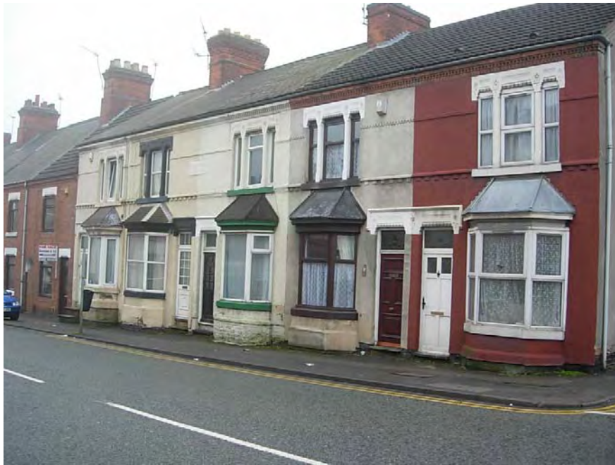
At numbers 31 to 39 Hinckley Road (known as West End Terrace) the conservation area would benefit from the painted render and brickwork being returned to its original state. These are the only properties on this row to have bay windows.
