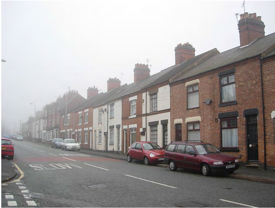
There is an excellent view south-westwards up Hinckley Road of the Victorian residential terracing. There have been some modern alterations, but many original features such as the red brick chimney stacks, for example, remain highly visible.
