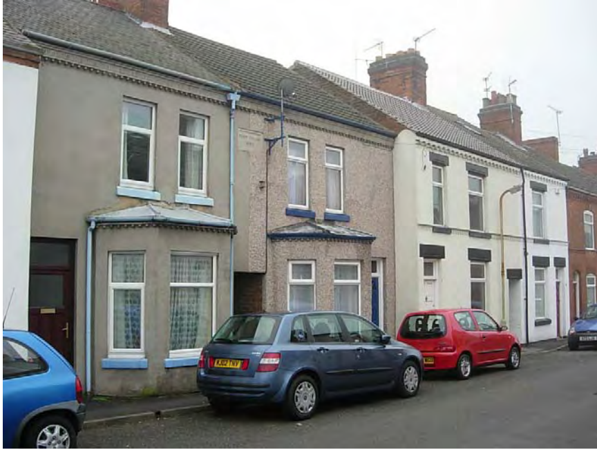
The two dwellings at 41 & 43 New Street, known as Fern Villas and built in 1894, were constructed to a slightly different building line to the adjacent rows of terraces, and include bay windows. The render, concrete roof tiles, and installation of a satellite dish detract from the original character of the dwellings.
