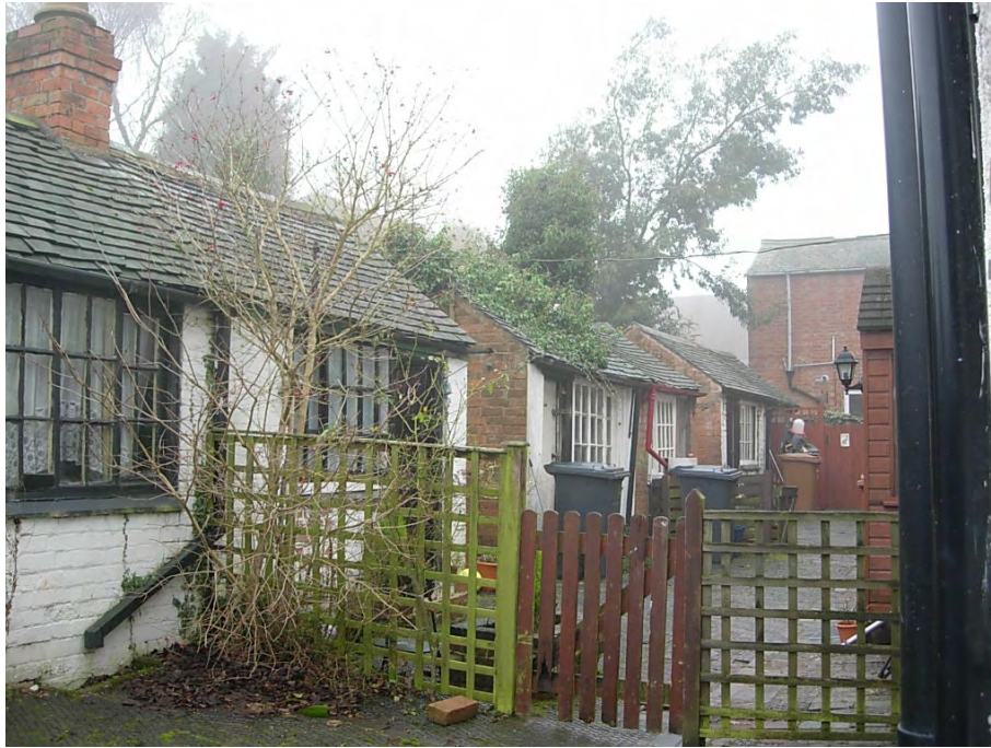
The boot and shoe workshops to rear of Chelsea Row are significant local buildings within the conservation area. The courtyard still retains the original Victorian blue clay floor tiles.
