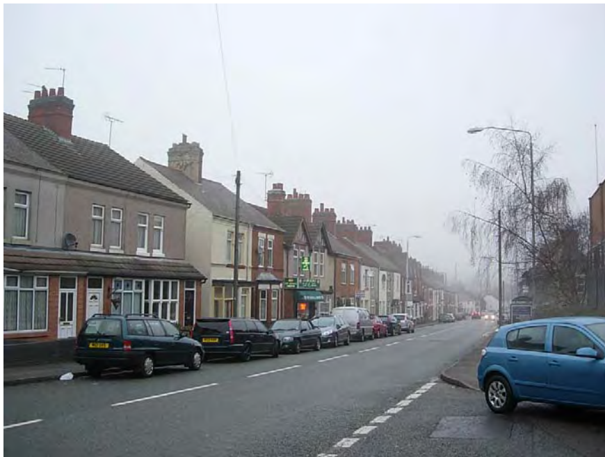
The subtle variations in the building, eave and ridge lines as each section of residential terracing was built can be seen from the view north-eastwards into the conservation area along Hinckley Road. The on street parking does detract from the visual quality of the conservation area.
