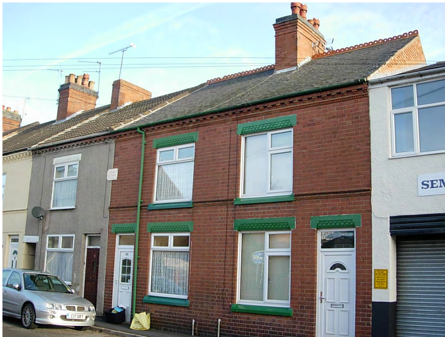
The residential terrace at 49 to 57 New Street was built in 1899 and known as Druid Cottages, as signified by the date stone. The terracotta brickwork and window lintel detail on numbers 55 and 57 New Street can clearly be seen.
