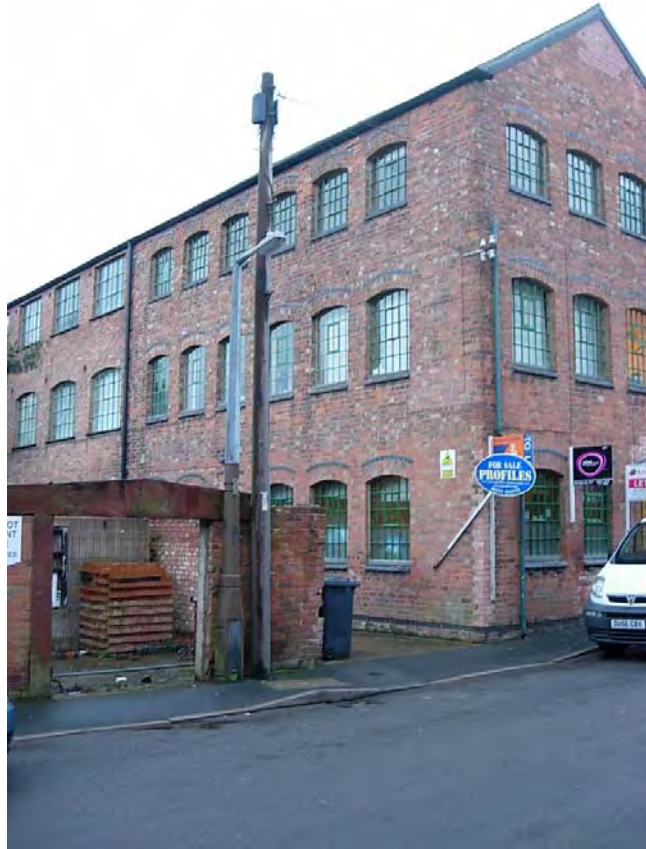
There are a number of concrete and metal lamp posts within the conservation area that should be replaced with a heritage cast iron post, including this concrete lamp post outside 1-5 New Street.
