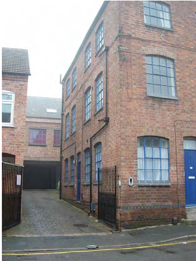
The recently converted boot and shoe factory at 6 New Street retains many original features including cast iron windows and external brickwork detail. Metal gates have been installed and the surface of the courtyard has been treated with concrete pavers.
