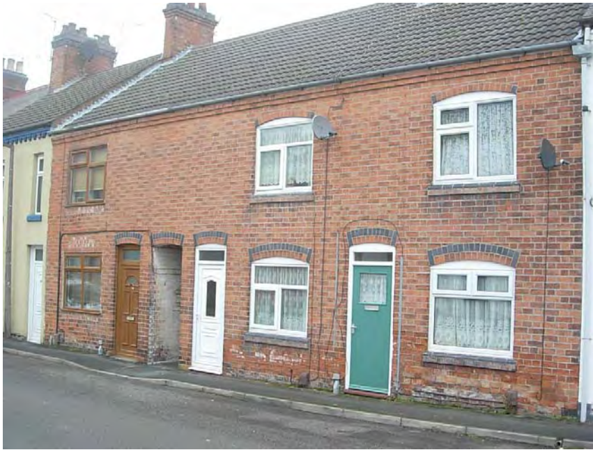
The brickwork on 27 to 31 New Street has been re-pointed and the original window openings retained. The replacement of the concrete roof tiles and plastic windows with traditional materials on these properties would benefit the conservation area.
