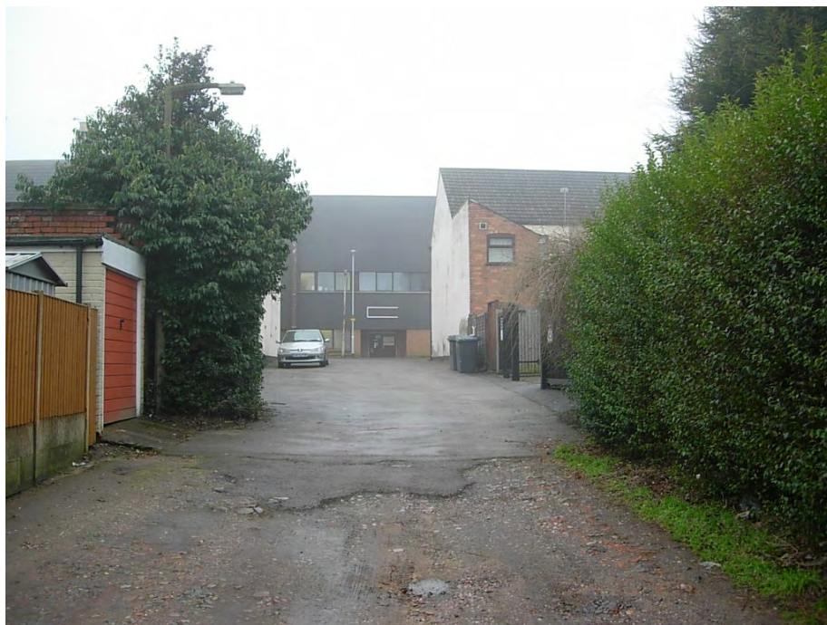
The section of the private road linking New Street with Melton Street has been treated as part of the recent factory conversion at 1-5 New Street. This is a poor view into the conservation area due to the modern materials utilised on the rebuilt Eatoughs factory.
