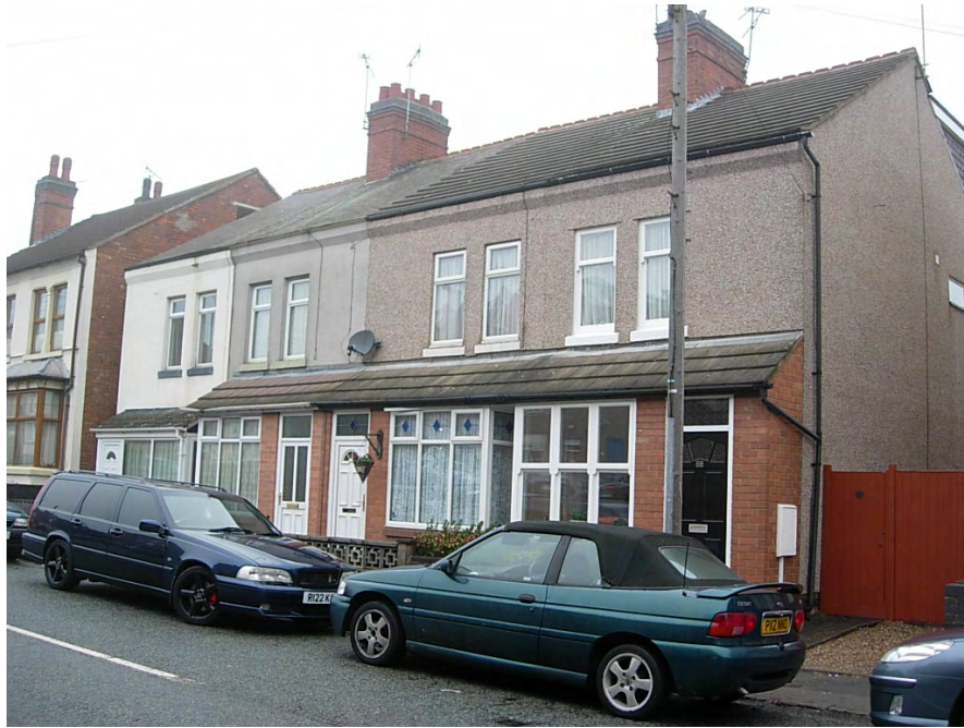
The small front extensions and gardens, rendered brickwork and concrete roof tiles are poor alterations to the terrace at 68 to 74 Hinckley Road. However, the dwellings do retain their original chimney stacks.
