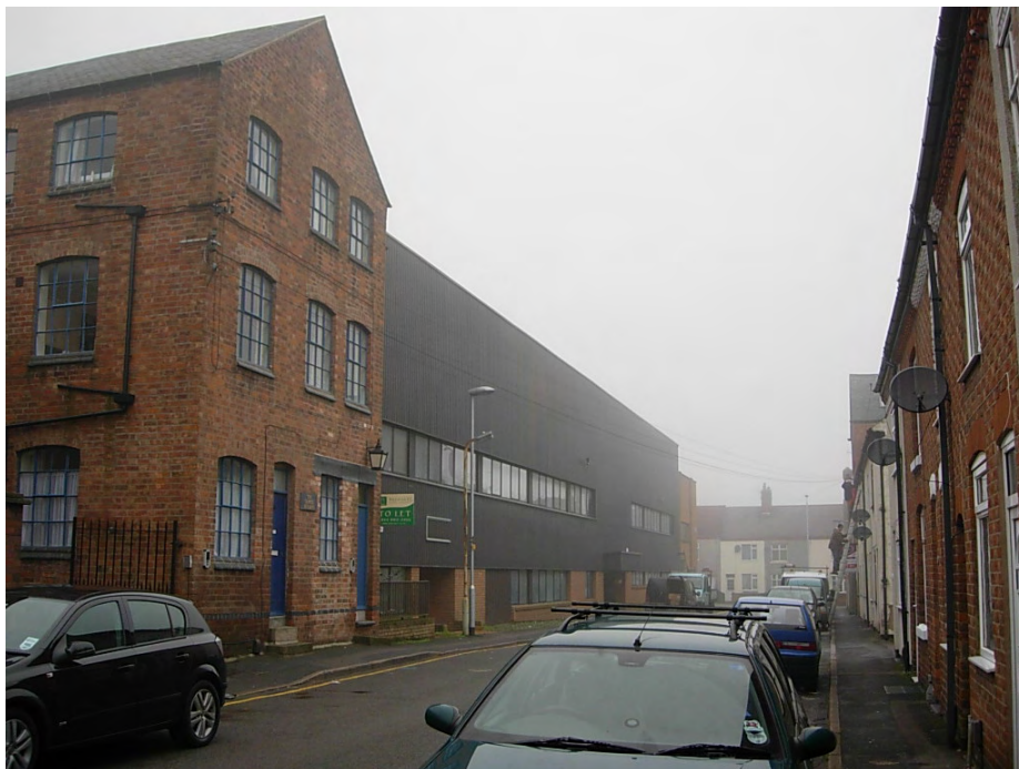
The view north-west from the conservation area along New Street is spoilt by the rebuilt Eatoughs factory (now known as Warwick Buildings), detracting from the visual quality of the converted industrial premises at 6 New Street.
