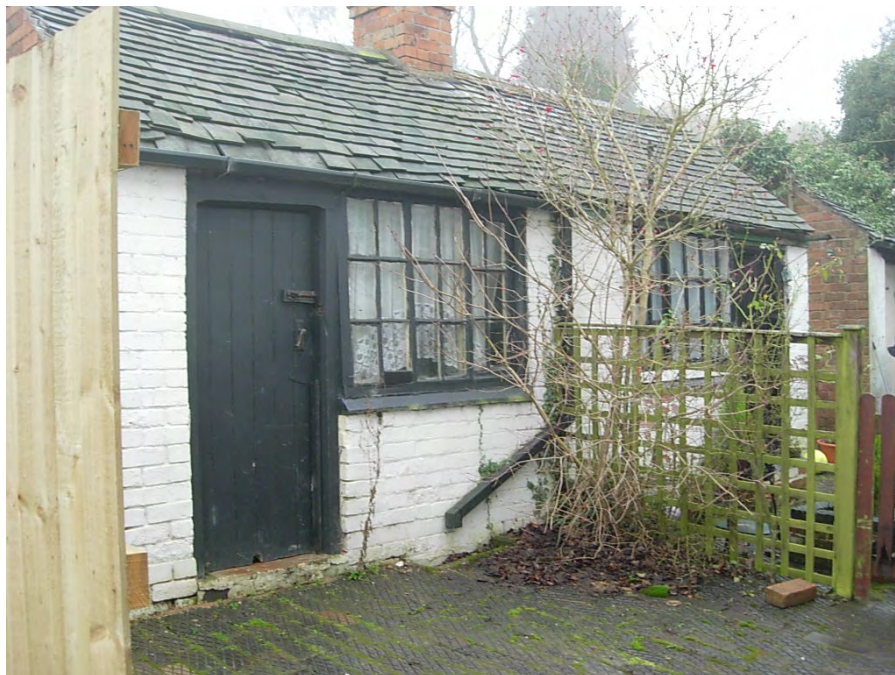
The workshops have some excellent remaining original features including slate roof tiles, a red brick chimney, wooden horizontal sliding sash windows, and internal features including lime plastered timber roofs and in one case a copper boiler.
