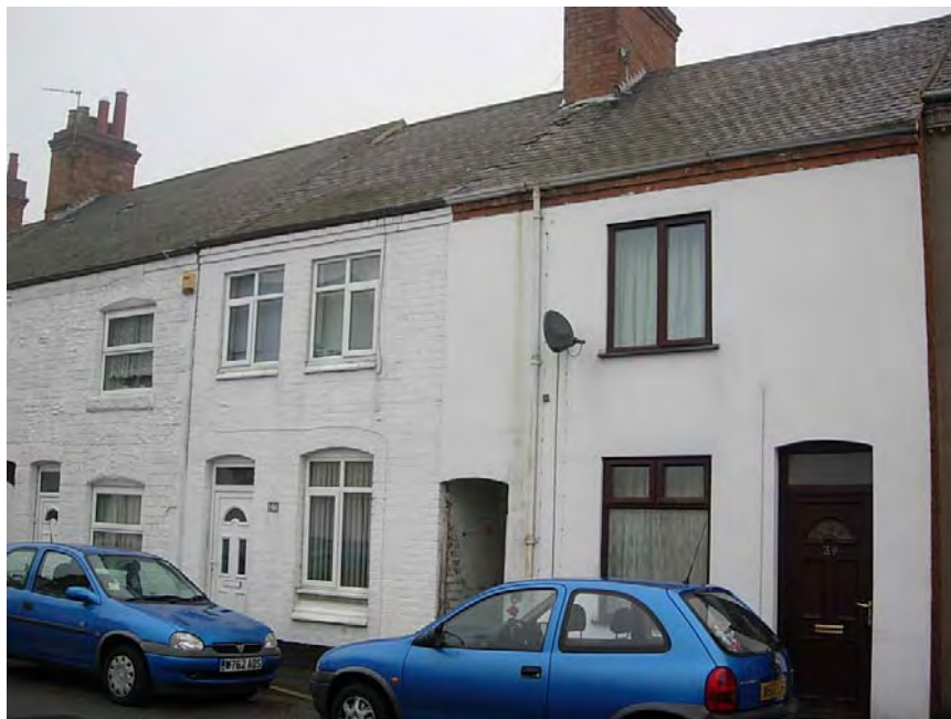
The painted brickwork, window sills and lintels on the row of terraces at 33 to 39 New Street detract from the historic character of the dwellings. The properties do however retain their original slate roof tiles.
