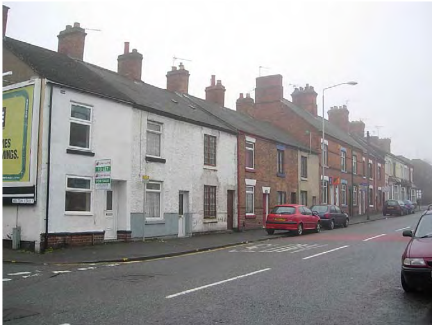
Numbers 9 to 17 Hinckley Road are known as Chelsea Row, a row of six cottages built around 1860 for framework knitting. Few traditional features remain on the front elevations of the cottages.
