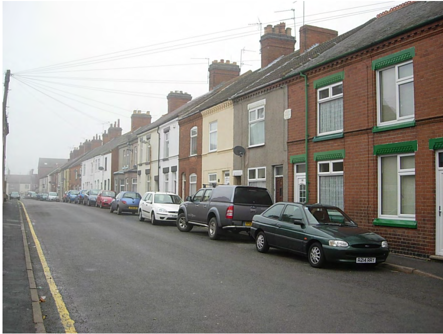
The view into the conservation area of the row of terraces along New Street identifies many excellent details including terracotta brickwork, window lintel details, and brick chimney stacks and stone pots.
