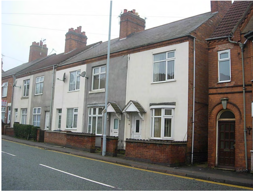
Unsympathetic modern alterations may be identified on the residential terrace at 46 to 54 Hinckley Road, including low boundary walls, plastic windows and downpipes, rendered brickwork, satellite dishes and porches.
