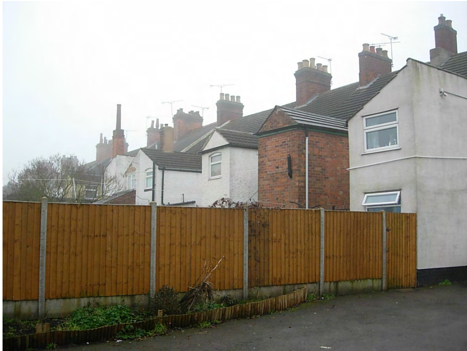
A timber panel and concrete post fence has unfortunately been used to replace a traditional brick wall at the rear of this New Street terrace. However the location does provide an excellent view of the brick chimney stacks and stone and clay pots on the terrace.
