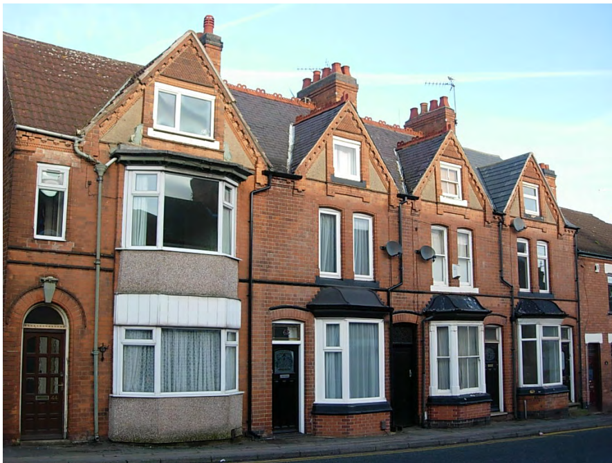
The three storey terraces at 38 to 44 Hinckley Road retain many interesting features, including bay windows, intricate door details, gabled terracotta brickwork, and slate roof tiles. The former balustrading above the second storey bay at number 44 Hinckley Road has been removed.
