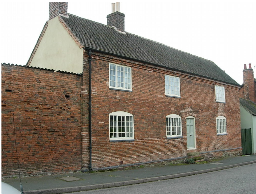
The Grade 2 early to mid-C18 Listed Elms Farmhouse is red brick dwelling built on a Charnwood rubblestone plinth with plain tile roof and steps leading to a central 6 panel door. The farm is now a riding school.
