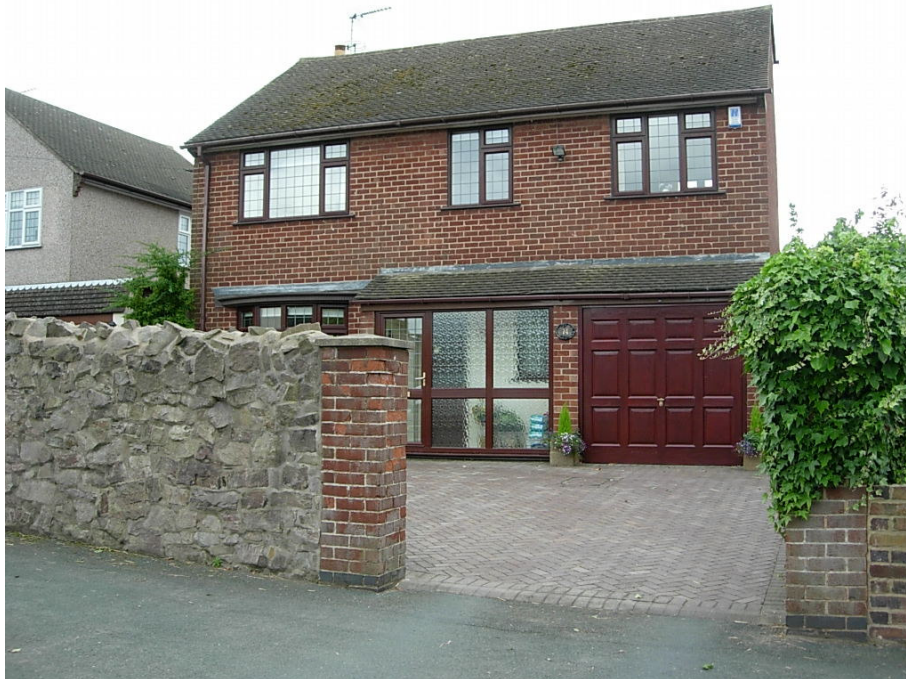
74 Main Street is a modern 2 storey dwelling that has little in character with the villages traditional buildings.
