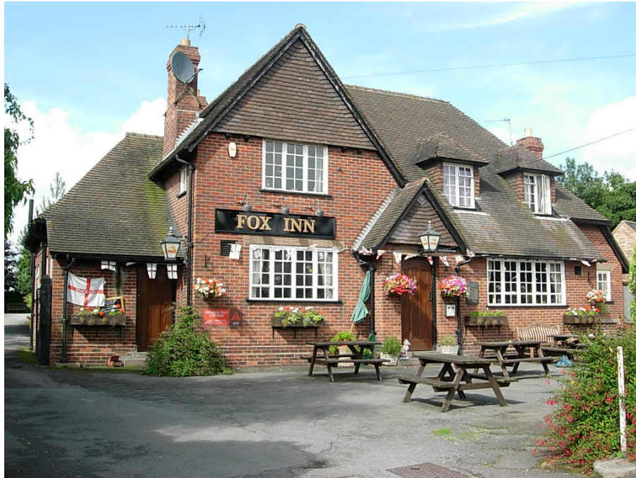
The roof of the Fox Inn built in the 1930's is a visually interesting feature, however the frontage area could be improved.
