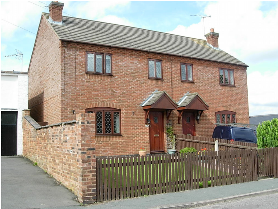
The recently built semi detached dwellings, 35/37 Main Street, are of simple design with small front canopies and picket fence.
