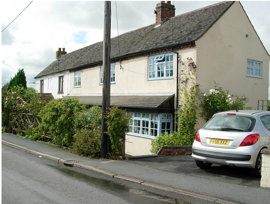
The large canopy that runs at 1 st floor level over the whole length of the property at 19 Main Street is out of character with the original form of the property
