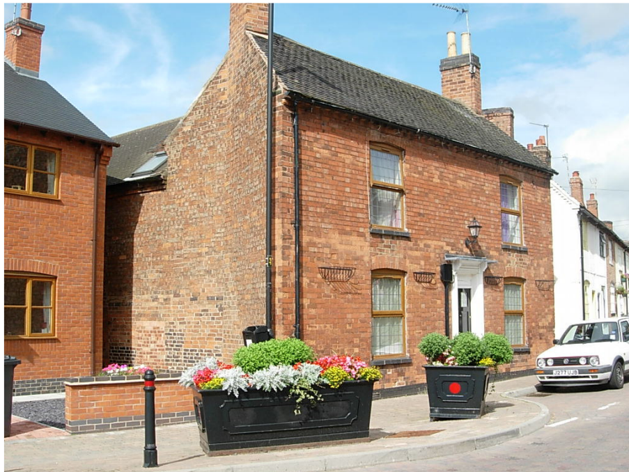
45 Main Street is a pleasant 2 storey dwelling with rosemary roof tiles and panel door. Its front elevation would be improved if the plastic windows were to be replaced with traditional timber sashes.
