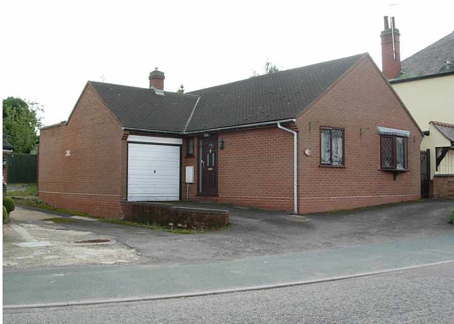
The bungalow 50 Main Street being single storey and built in modern materials has a detrimental visual impact on the conservation area. The area fronting the bungalow is open with the surfacing treatment poor.
