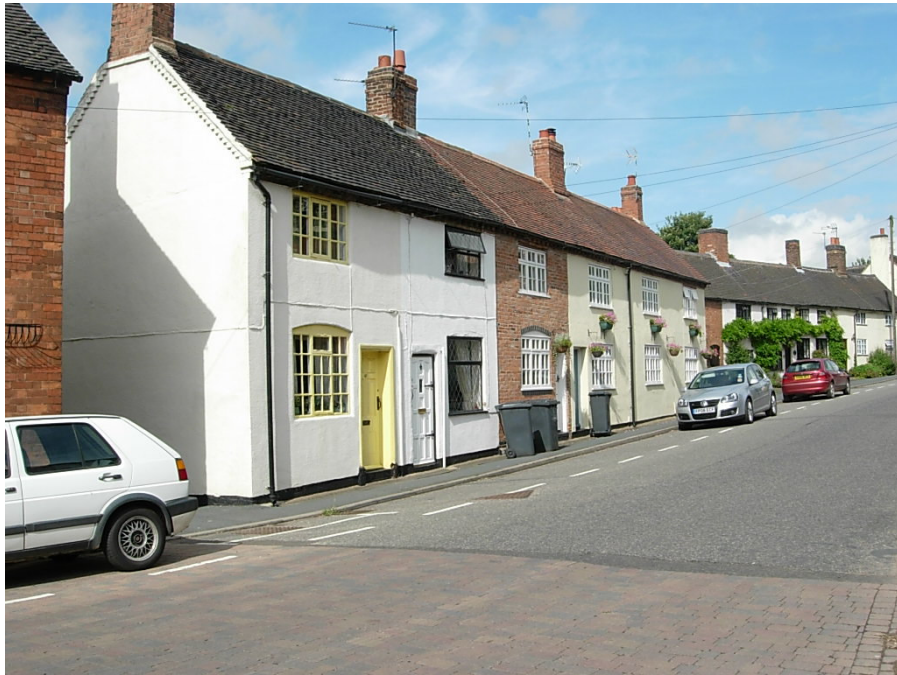
The symmetry of the terrace 47 – 55 Main Street is spoilt with new windows installed at 49 and the roof and ridge tiles changed at 51.
