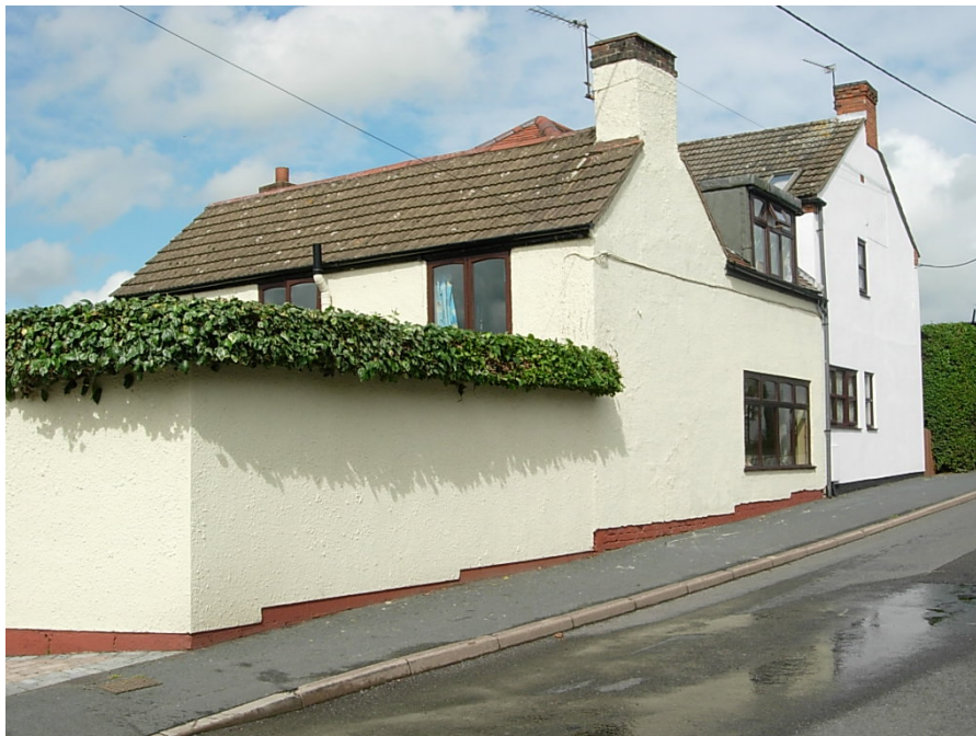
The roof of 23 Main Street could have been improved if the dormer had been set back and its felt sides finished either in tiles or lead. The dwelling has also lost its chimney pots
