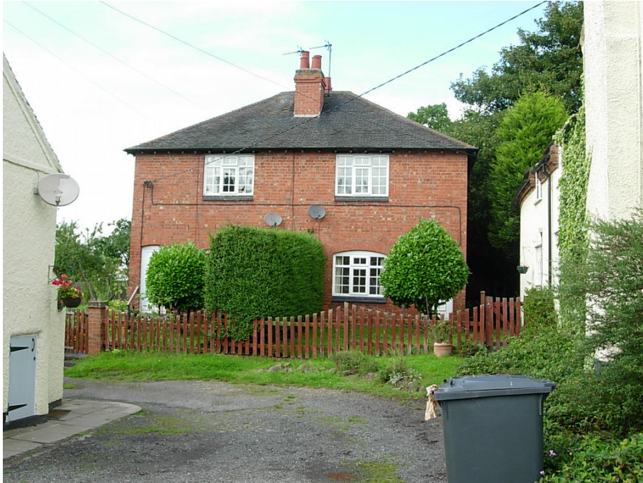
The semi detached dwellings 73 & 75 Main Street which are set well back from the carriageway have been spoilt with the installation of UPVC windows.
