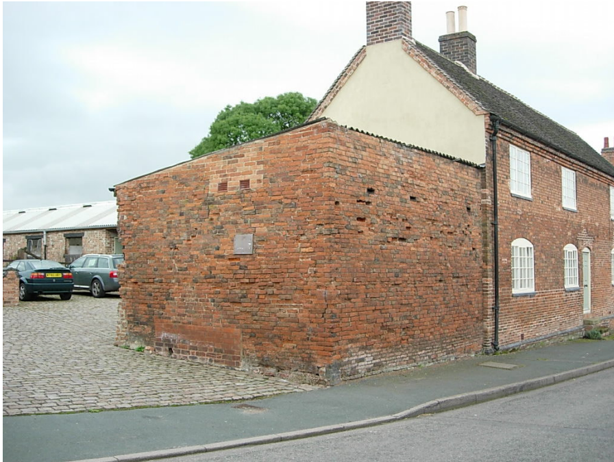
The outbuilding abutting Elms Farmhouse would be improved if the corrugated roof was replaced with a more traditional roof. The brick walls need attention but should be retained where possible.
