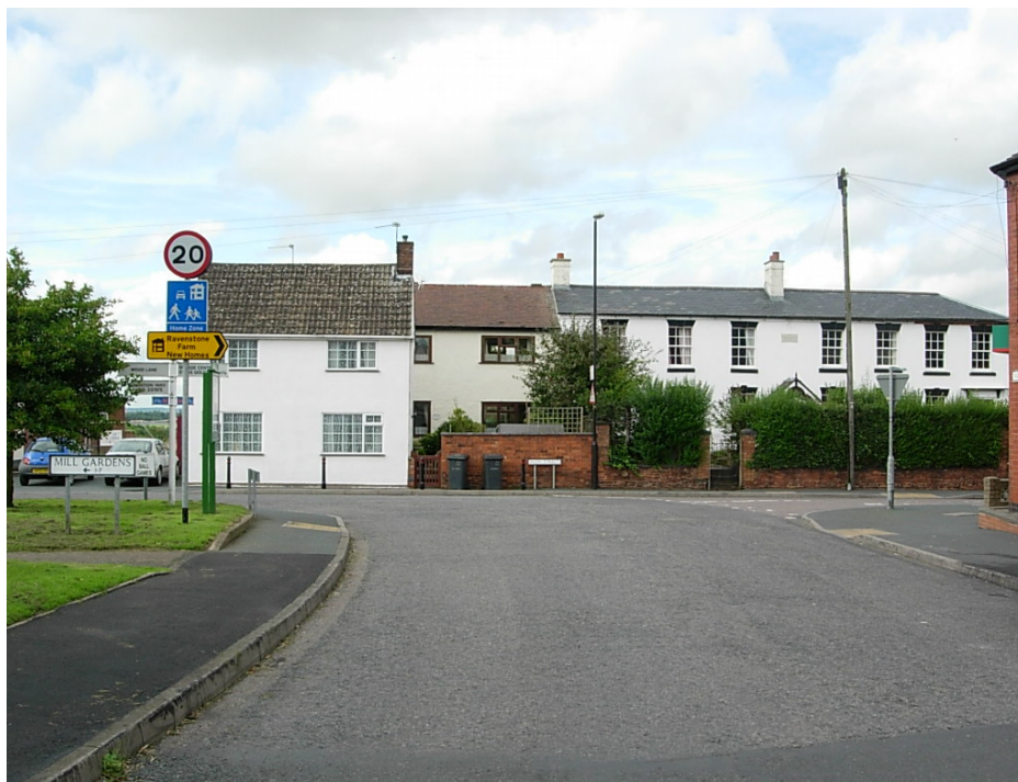
The properties 27 – 33 Main Street provide an excellent visual stop when approaching Main Street from Nuneaton Lane. However, the concrete roof tiles on 27 Main Street not in character.
