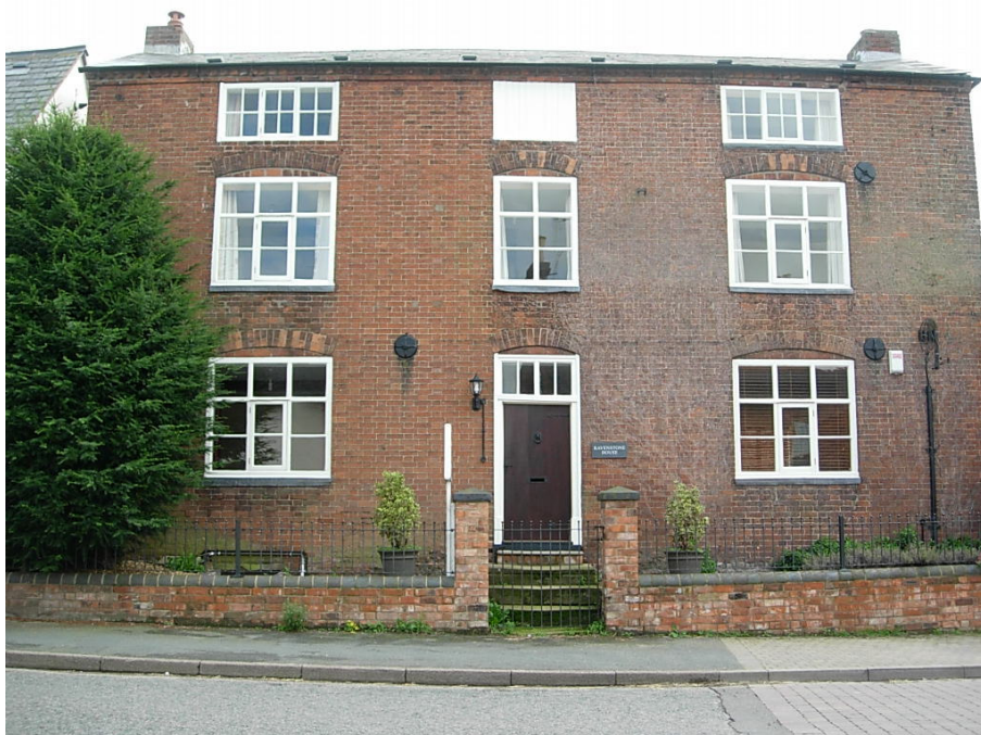
The 3 storey late C18 Grade 2 listed dwelling is one of Higham's important vernacular buildings. The red brick property with slate roof, end chimney stacks and large window casements has steps leading to a flush panel door.
