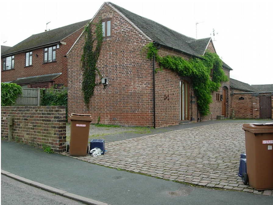
The outbuilding at Elms Farm has been successfully converted to a dwelling with an excellent forecourt surfaced with granite setts. The brick wall fronting the premises needs to be raised up and finished with a traditional coping and the area behind surfaced with granite setts.
