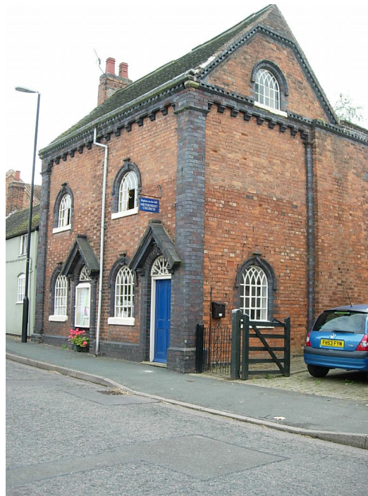
The Grade 2 Listed Methodist Church was originally 'the house that Jack built'. The building which is built of red brick with a purple brick detailing and plain tile roof is a prominent landmark building in the village.
