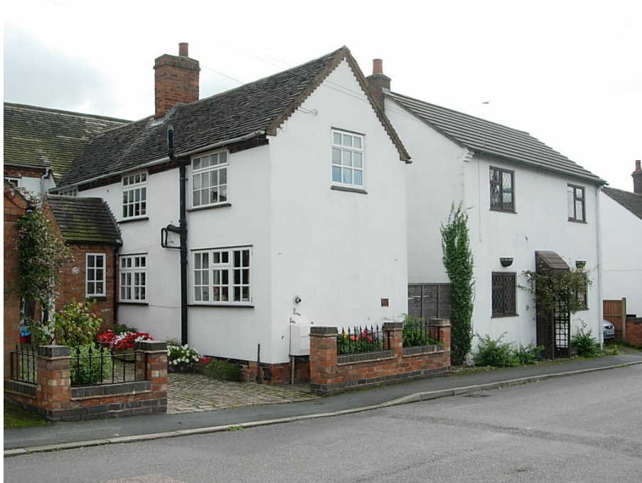
32 & 34 Main Street are an interesting group with 34 having its gable end fronting the road with small pane windows.
