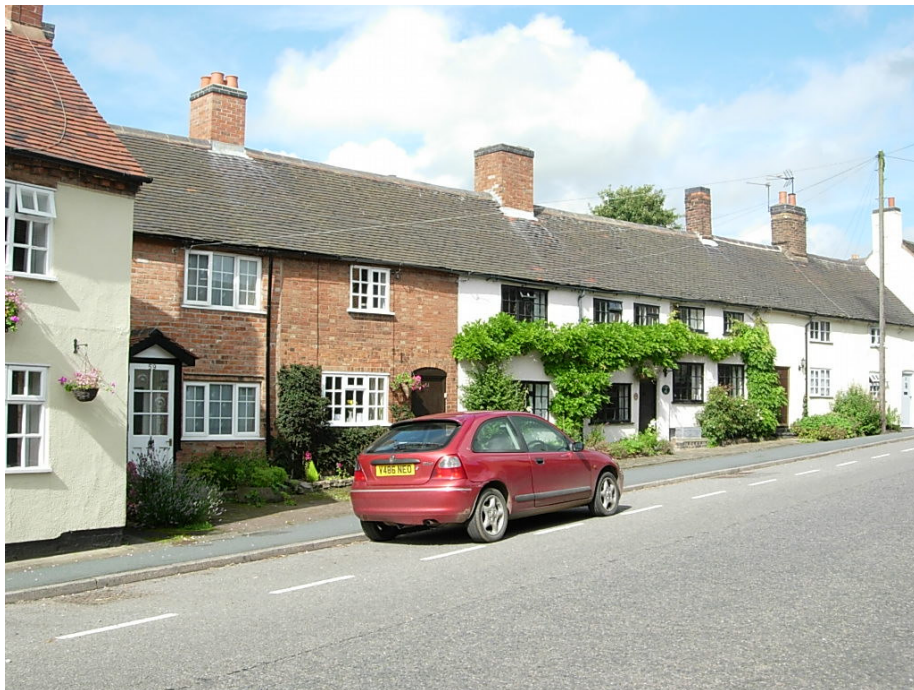
Pump Row is a pleasant group of properties that is spoilt with the loss of some chimney pots.
