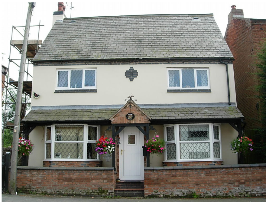
This building that was once a public reading room for men has until recently been used as a doctors surgery. The integrity of the premises has been compromised by recent improvements with a large canopy built over two bay windows and UPVC windows installed.
