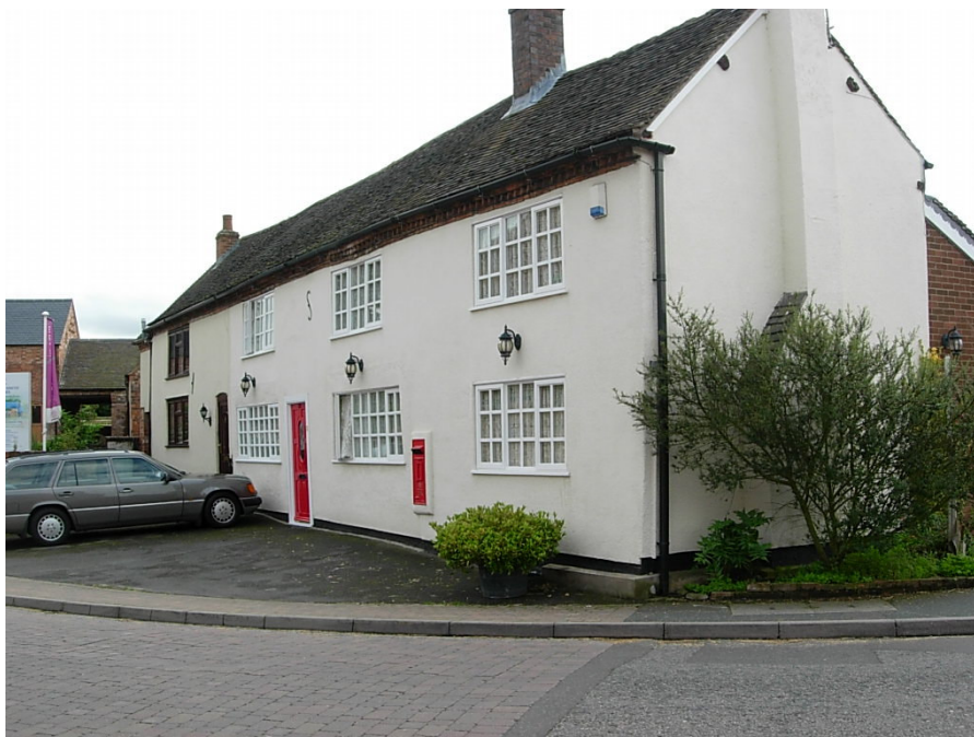
The old post office is sited in a prominent location in the conservation area. The rendered property that has timber windows and rosemary roof tiles has retained its original wall post box.
