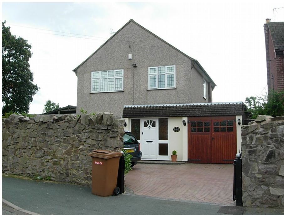
76 Main Street has lost its traditional integrity with recent improvements. The stone wall fronting the dwelling is an excellent feature which has been retained.
