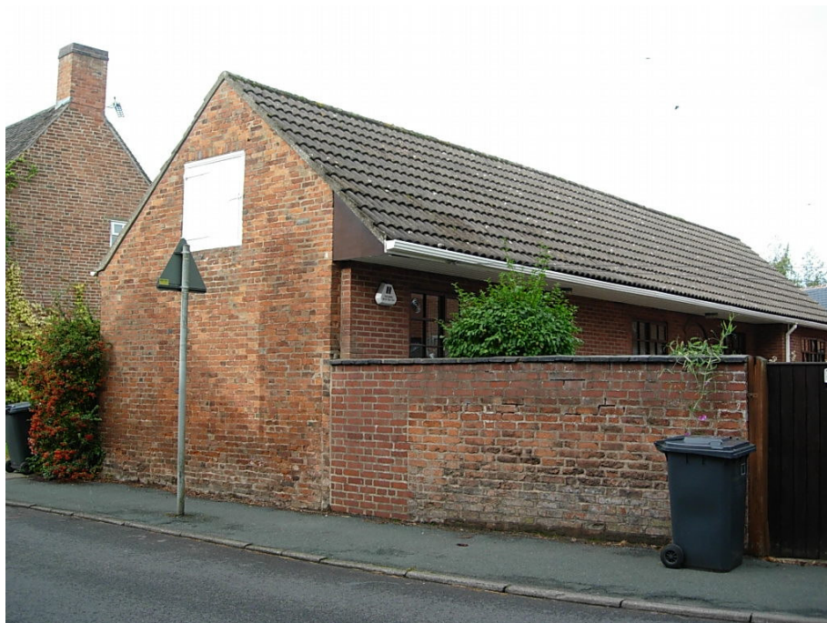
The property 113 Main Street has been converted into a dwelling. Much of the original building has been retained, however, its traditional character has been compromised with the use of concrete roof tiles and plastic guttering.
