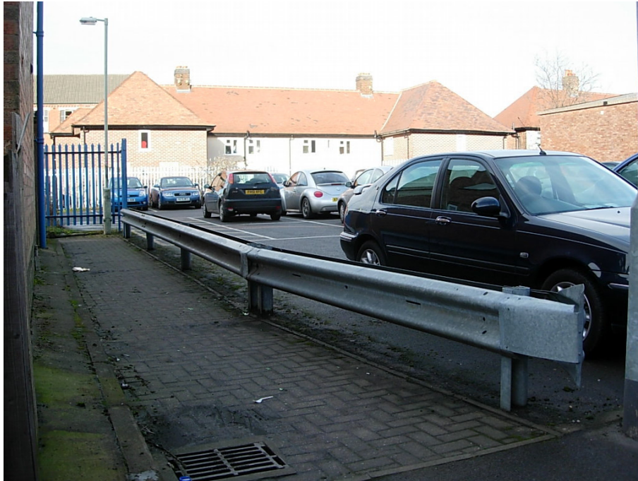
The crash barriers at the side of the Borough Council's car park detract from the appearance of the jitty. They should be replaced or flanked by metal railings.
