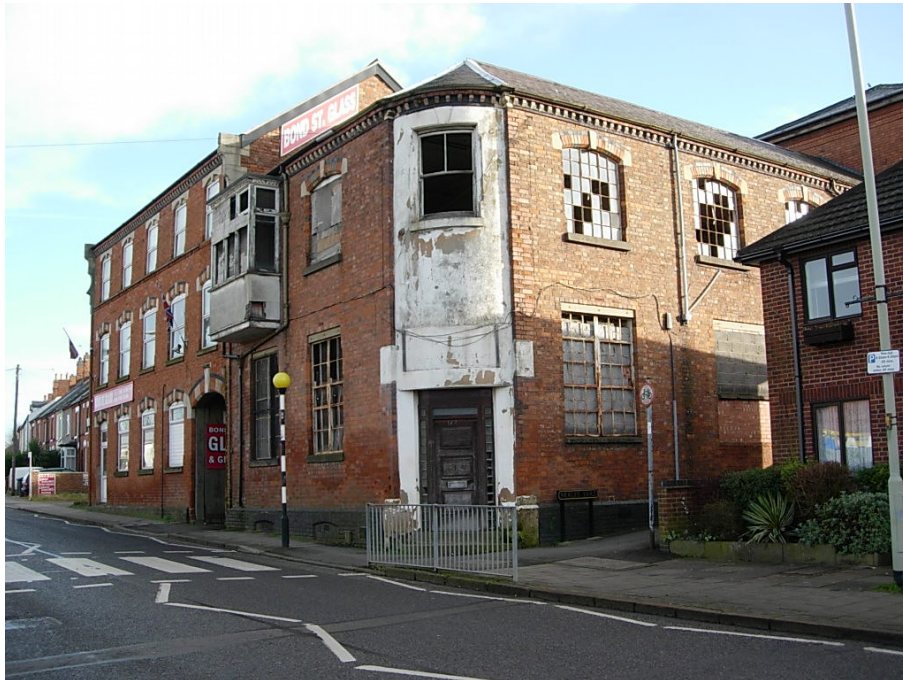
Proposals are in hand to restore Ashcroft House on the corner of Neale's Yard and Upper Bond Street. It is the numerous factories in the conservation area that give it its distinct character
