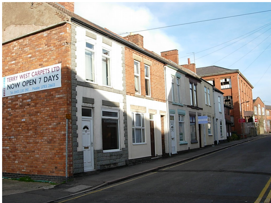
The terrace of dwellings, 50- 60 Druid Street, are traditional red brick properties whose appearance has been spoilt by inappropriate changes. These include the use of rendering, artificial cladding, concrete roof tiles and poorly designed plastic windows.
