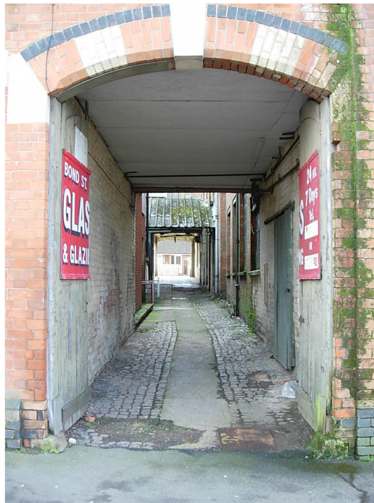
Archway leading to the inner courtyard of the former Puffer factory and Druid Street. The traditional granite sets are still extant
