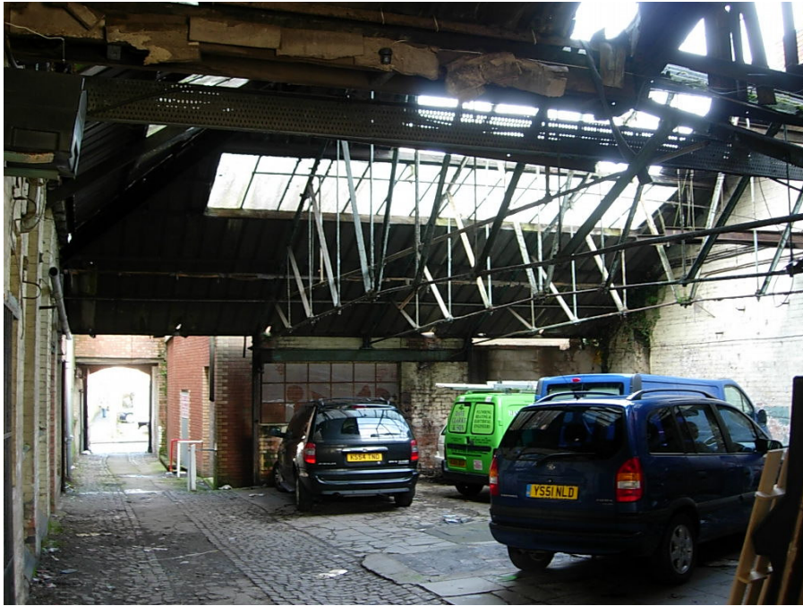
The inner courtyard of the former Puffer factory showing the intricate iron roof trusses
