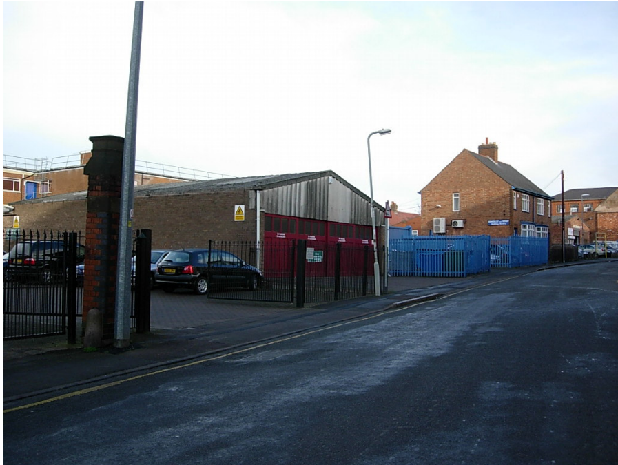
The modern single storey portal framed building and security fencing on the west side of Druid Street although not in the conservation area, have a detrimental visual impact on its character
