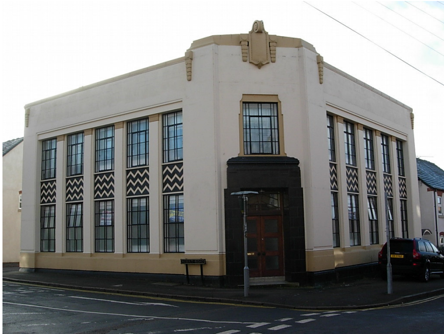
These are the former offices of Moore & Osbourne sited at the corner of Druid Street and Albert Road. It is an imposing building built in the Art Deco style that has recently been converted into 4 flats
