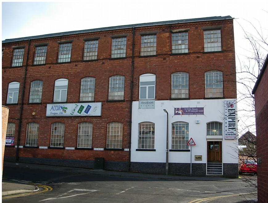
The factory at 55 Druid Street is being utilised by a number of businesses. The loss of several traditional window frames, rendering and advertisements have a negative impact on its Victorian character. Consideration should be given to the restoration of its traditional features.
