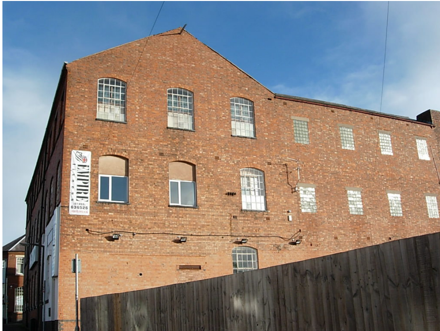
The gable end of the factory at 55 Druid Street is spoilt by the prominent Advertisement board. The replacement of 2 cast iron windows with plastic frames also has a detrimental impact on the appearance of the building.
