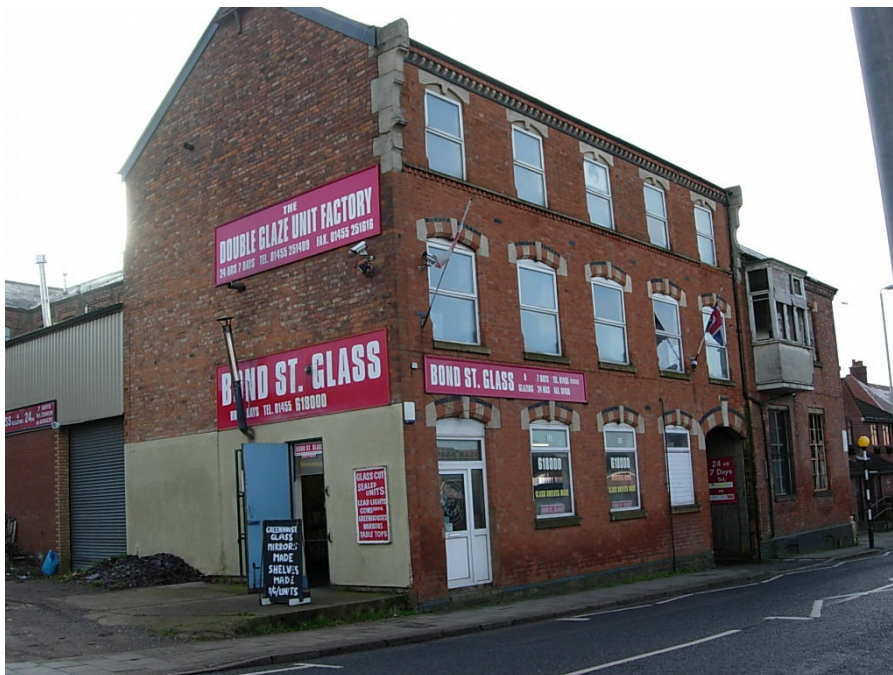
This is a distinctive building at the entrance into the conservation area. The large paned plastic windows and signage detract from its original appearance.
