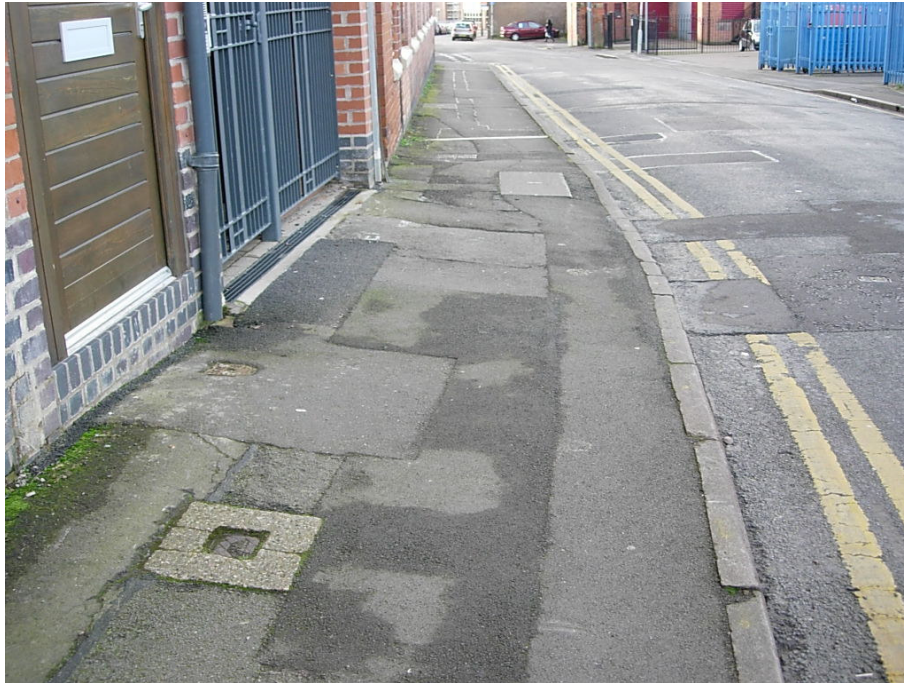
Many of the pavements in the conservation area are in urgent need of resurfacing. It would also improve its character if the concrete kerbs were to be replaced with granite kerbs
