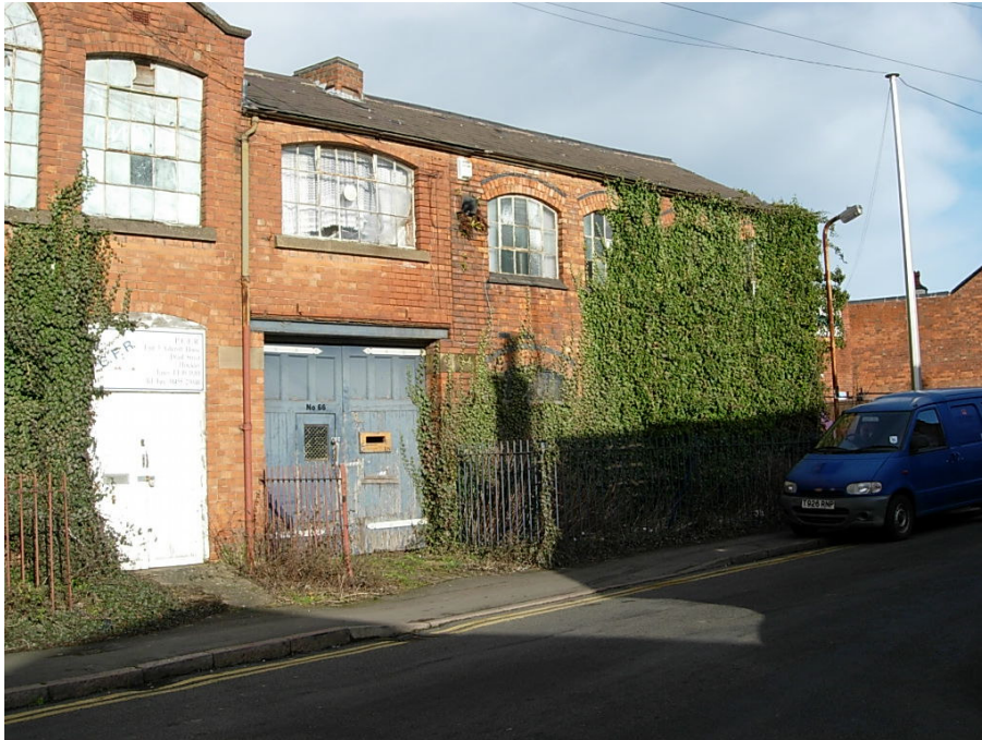
This former Laban Tansey needle factory now forms part of the adjacent premises. Together with the adjacent factory it suffers from neglect and vandalism
