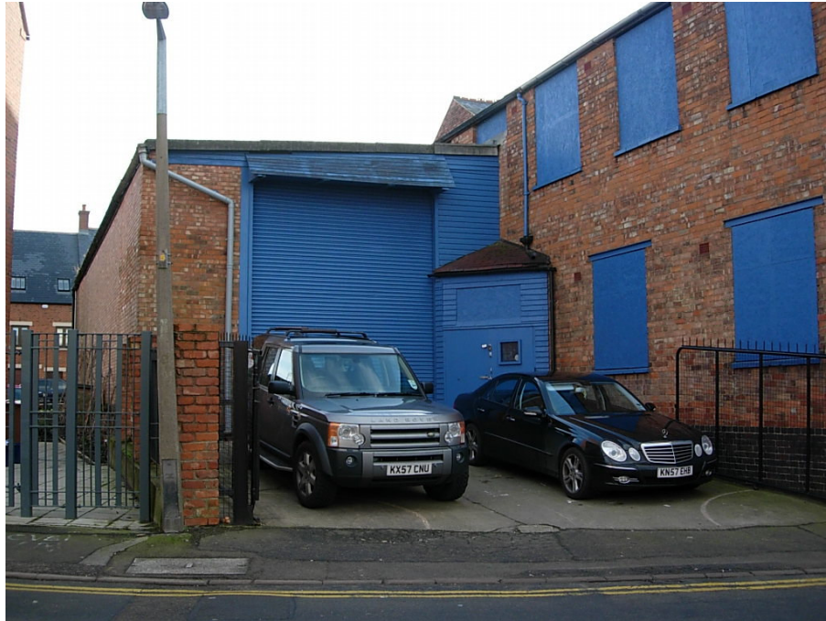
The former Bennett bird seed premises on Druid Street has been brought back into beneficial use
