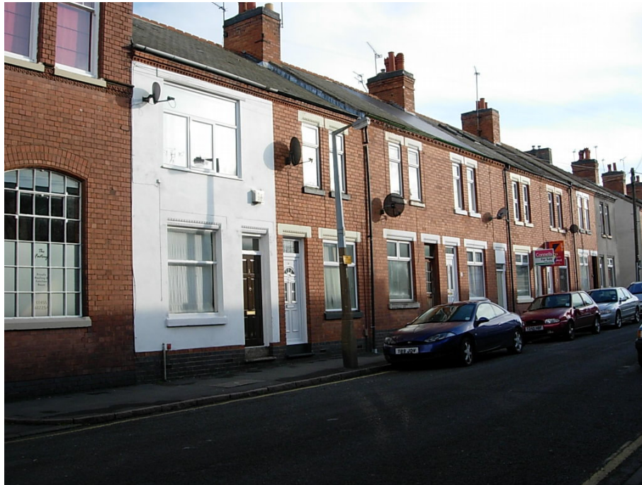
The unity of the terrace of dwellings on Spencer Street has partially been lost due to insensitive improvements and the installation of satellite dishes
