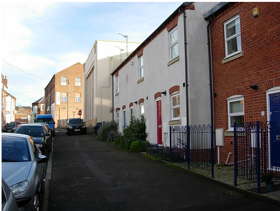
This modern terrace of rendered dwellings fronting the pavement provides a satisfactory setting to the adjacent Art Deco building
