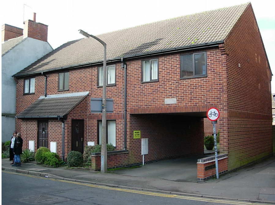
The flats 62-64 Druid Street out of character with the traditional qualities of the conservation area. Of particular concern are its design, choice of materials and siting behind the adjacent terrace.
