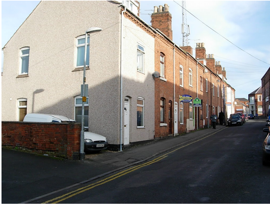
The terrace of dwellings 6-32 Druid Street has lost its original uniformity. Several properties have been rendered, roof dormers installed and window openings altered. Plastic windows, downpipes and satellite dishes also downgrade the quality of the properties
