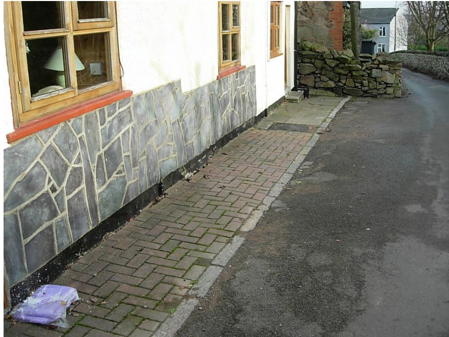
Granite sets would have been preferable to the concrete paviours fronting 14 & 16 Hillside. The slate decorative feature is also gives a cluttered appearance.
