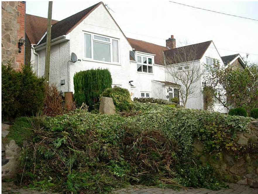
6 & 10 Hillside are well built rendered properties.
