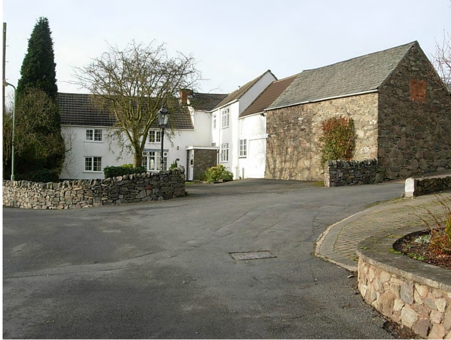
Quarry House and the stone outbuilding are a fine group of buildings on Queen Street although the concrete roof tiles are inappropriate.
