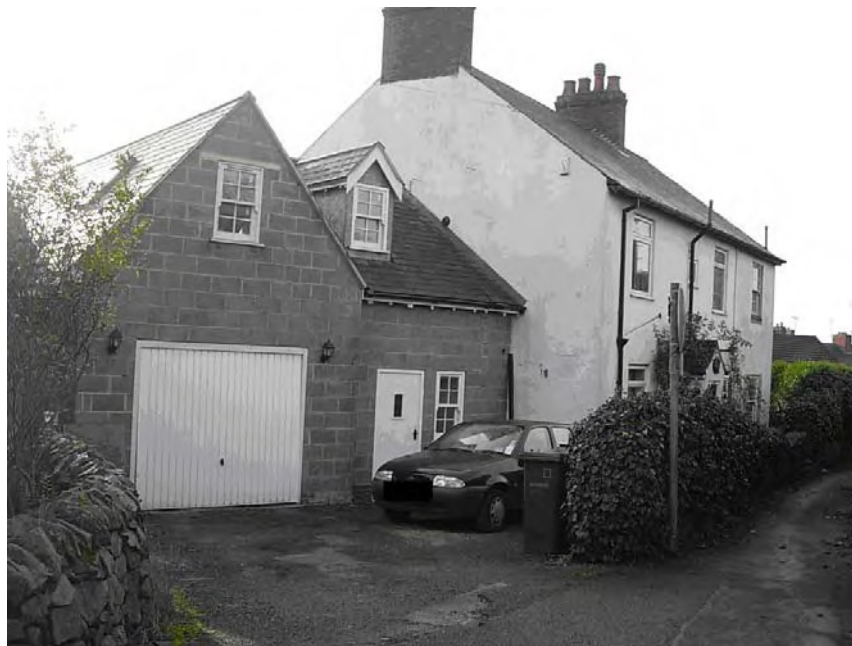
The extension to The Pieces on Queen Street needs to be completed with the block walls rendered to match the main house.
