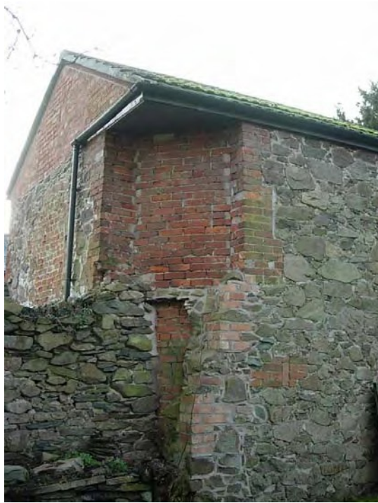
This building sited in the grounds of the Bulls Head Pub has an unusual gable. It appears that there was once a building fronting it.
