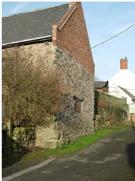
The gable end to Stepping Stone Farmhouse has been heightened utilising red bricks.
