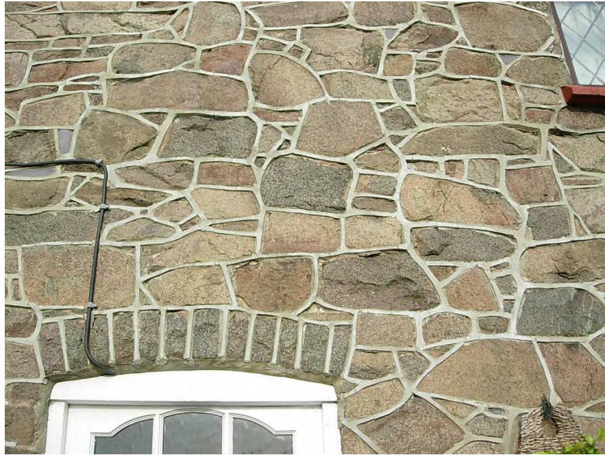
Raised pointing is not a traditional detail and has a detrimental affect on the stonework due to it being too prominent.
