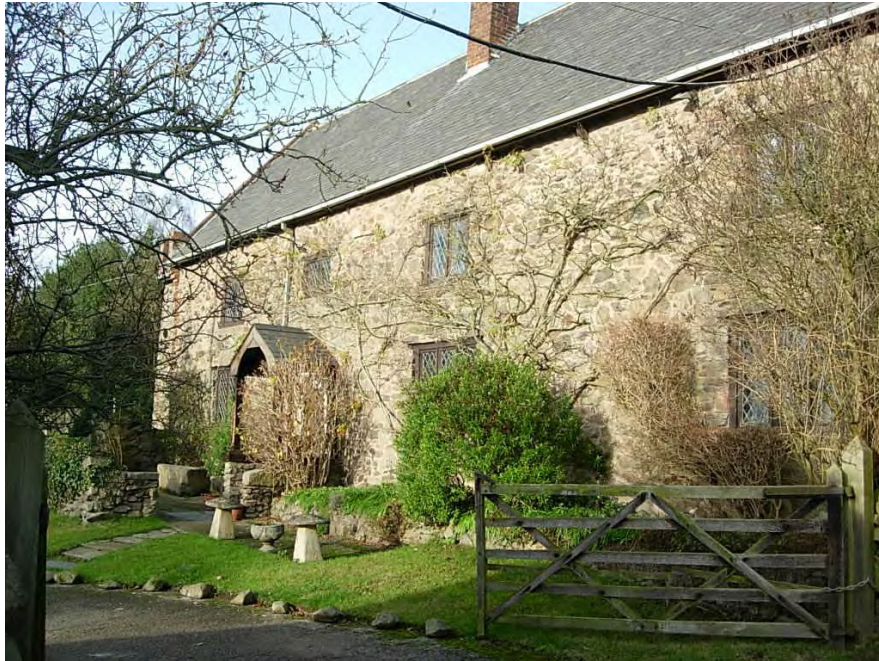
The mid 18C Stepping Stone Farmhouse is an attractive Grade 2 property built in Charnwood granite rubble and red brick with a slate roof.
