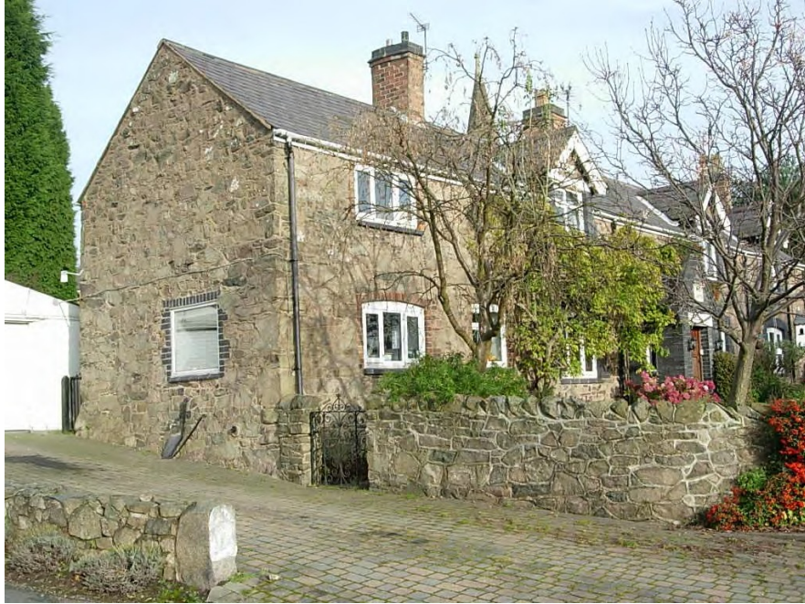
Three Gables on Queen Street is an attractive granite cottage although the insertion of a window in the gable has had a detrimental impact.
