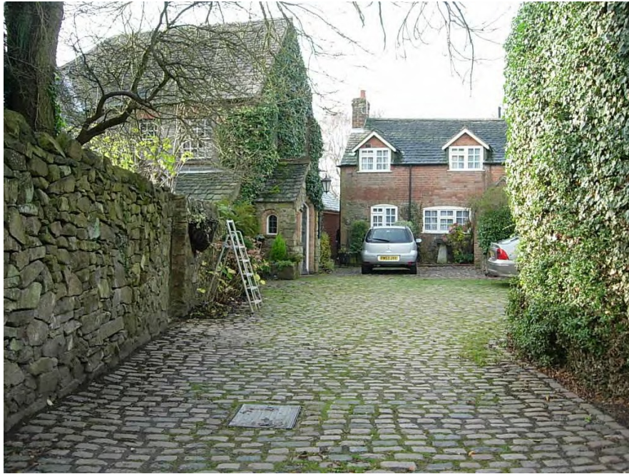
The access to this pleasant group of buildings at 27 Forest Road ( the Manor House) is surfaced with granite setts.
