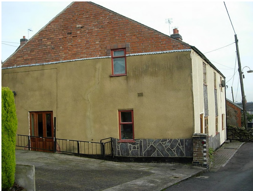
The modern render and other decorative features do not enhance the appearance of 18 Hillside which occupies a prominent position on the road.
