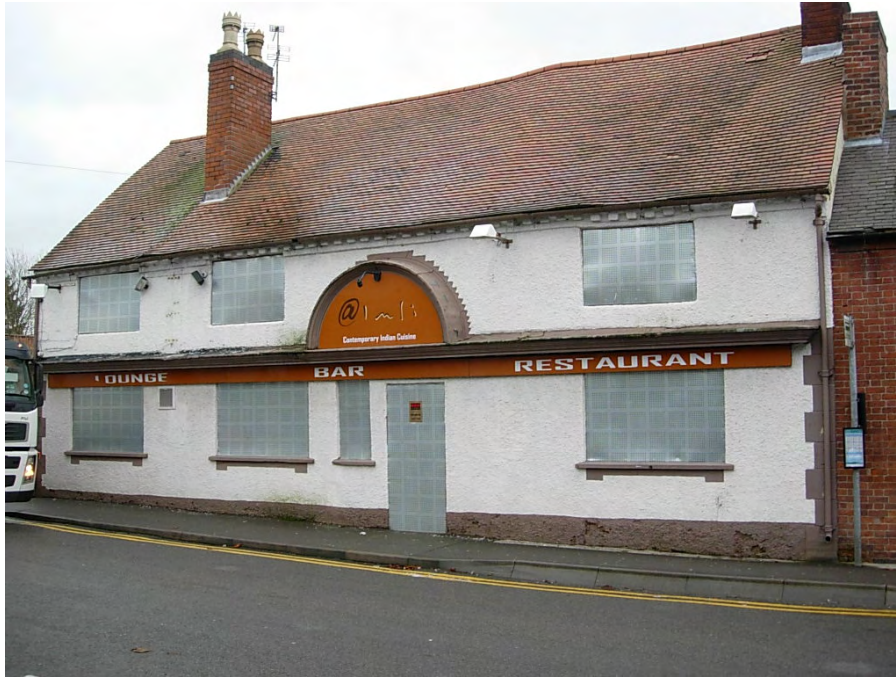
The George Pub is now closed. The land to the rear has development potential but it is important the pub premises front Main Street is retained.
