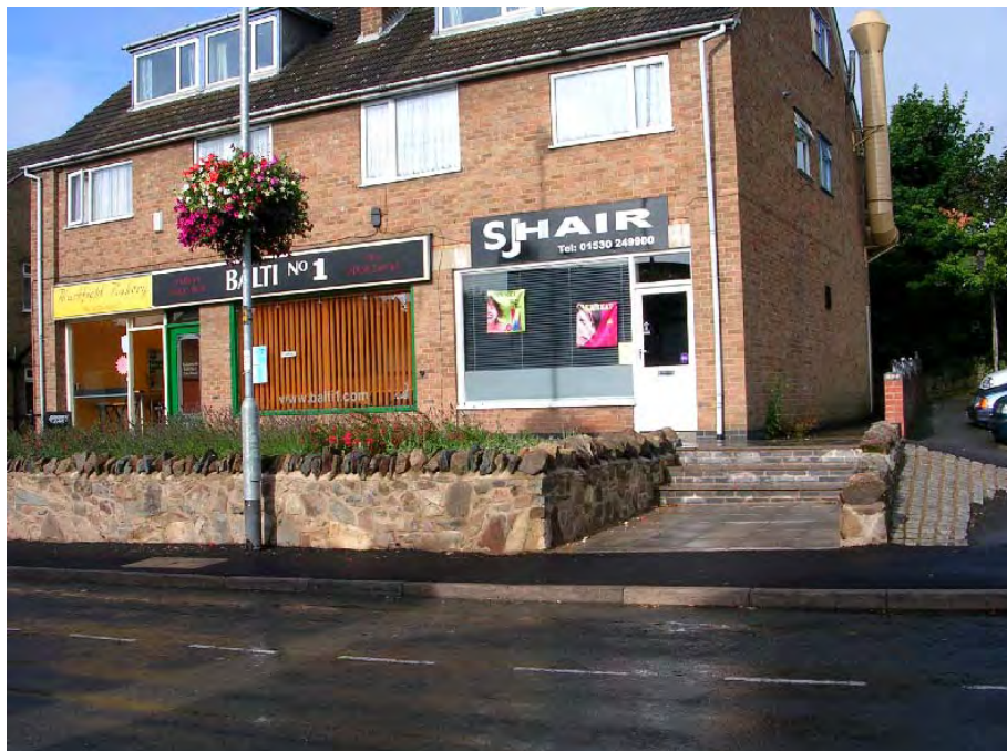
99 Main Street after completion of an enhancement scheme. The scheme comprised the construction of a granite wall fronting Main Street with a planting bed behind and disabled access provided from the adjacent council car park.
