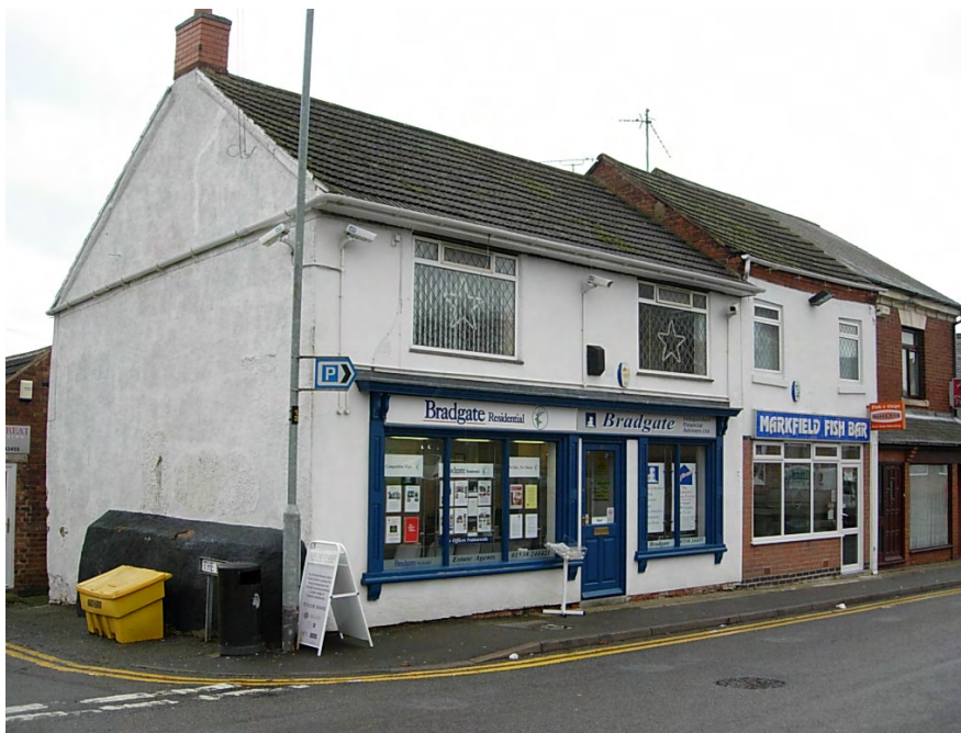
The appearance of 108 & 110 Main Street is satisfactory, although the use of concrete roof tiles and change of window openings at first floor level is unfortunate.
