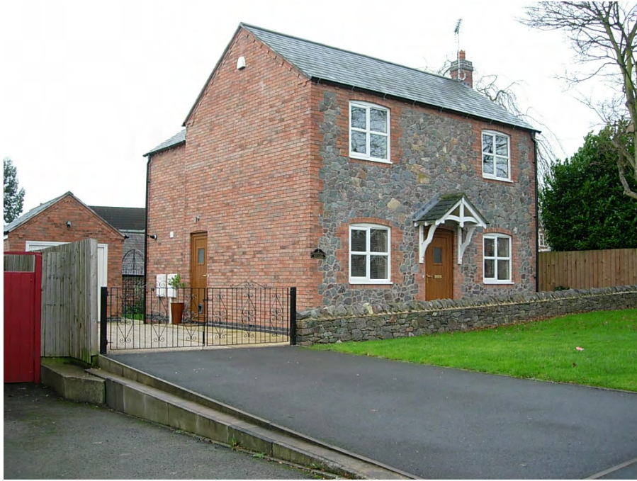
This dwelling on the corner of Neville Drive has only recently been erected and generally has a neutral impact on the conservation area.
