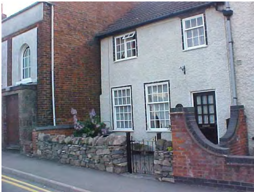
Old Rectory Cottage has had a new granite wall built fronting the property. The wall contrasts with the brick wall adjacent which is unsympathetic by way of its design and choice of materials.
