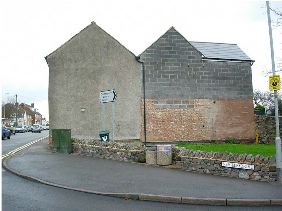
The side wall to the recent extension abutting the open space on Neville Drive needs rendering.
