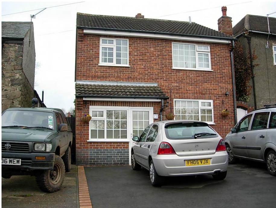
77 Main Street is a dwelling of modern design and materials with an open frontage which detracts from the conservation area.
