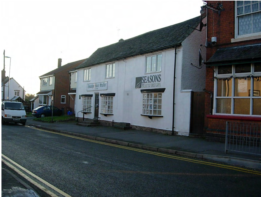
119 Main Street is a vernacular dwelling built in stone. However, the stone has been hidden due to the property being rendered and its chimneys have been lost.
