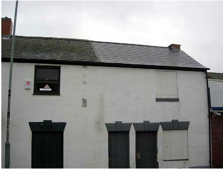
The vacant property on Main Street needs to be brought back into use. The materials used to repair the roof do not match the adjacent property and its chimney has been lost.
