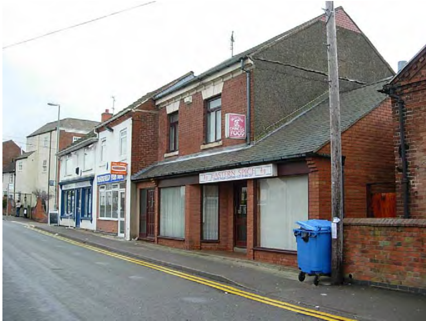
The treatment to 106 Main Street is not in sympathy with the properties either side.
