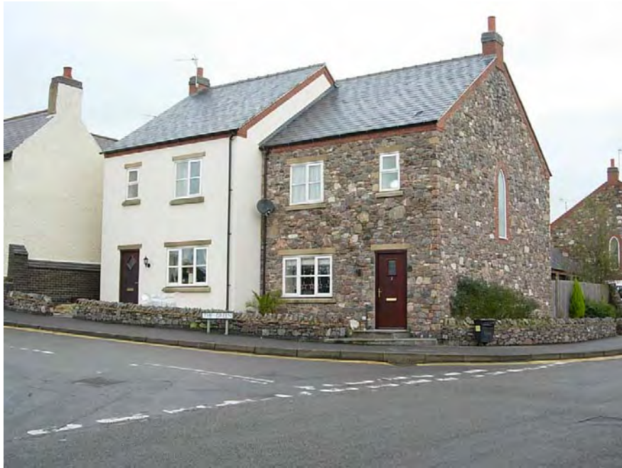
The recently erected semi-detached dwellings at the junction of The Green and Main Street provide a fine setting fronting Saw Pit Green.
