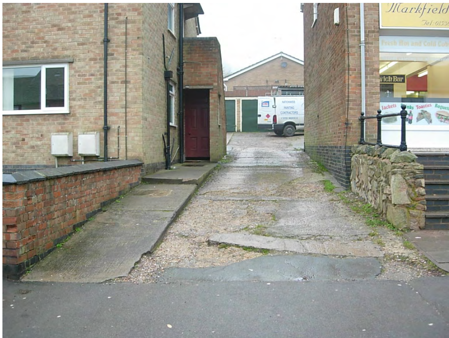
The accesses to both the garage court and 97 Main Street needs re-surfacing.
