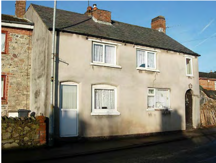
173 Main Street is a rendered property with a slate roof that has lost most of its chimney pots.
