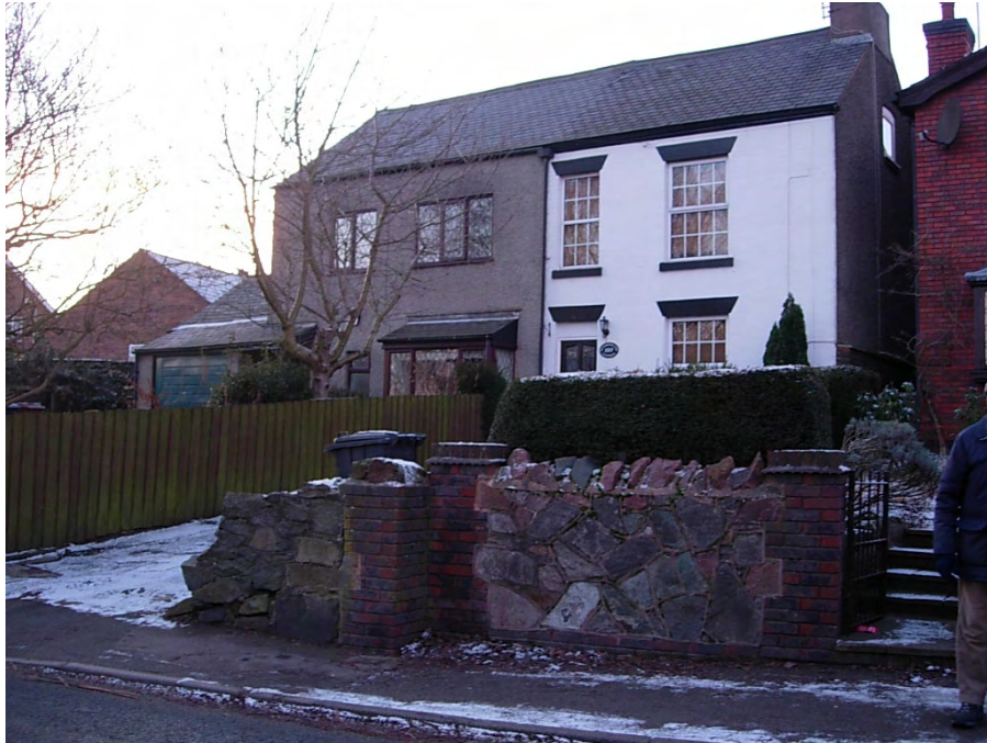
153 – 157 Main Street are properties that still retain their slate roofs but unfortunately have lost their uniformity. 157 has retained its original window openings and stone lintels unlike the adjacent property which has had inappropriate windows inserted and a garage built that needed to be set well back from the front elevation.
