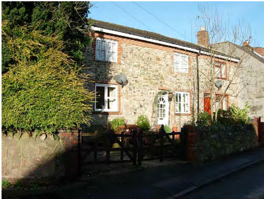
165/167 Main Street is a stone/brick property that has had its roof raised with a shallow pitch and its slate covering replaced with concrete roof tiles.
