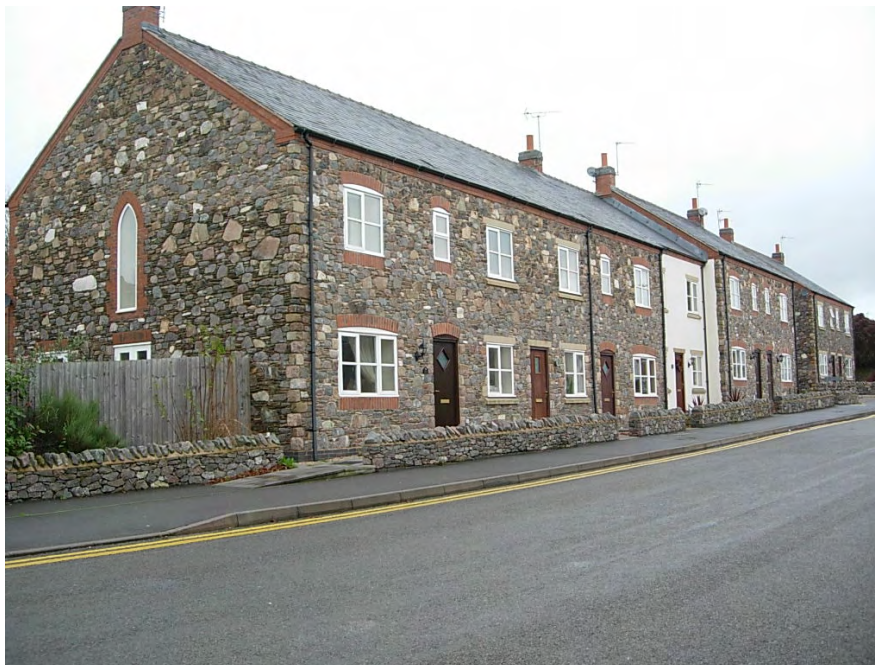
The recent development on Main Street successfully blends with the traditional character of the village by way of design and use of natural materials.
