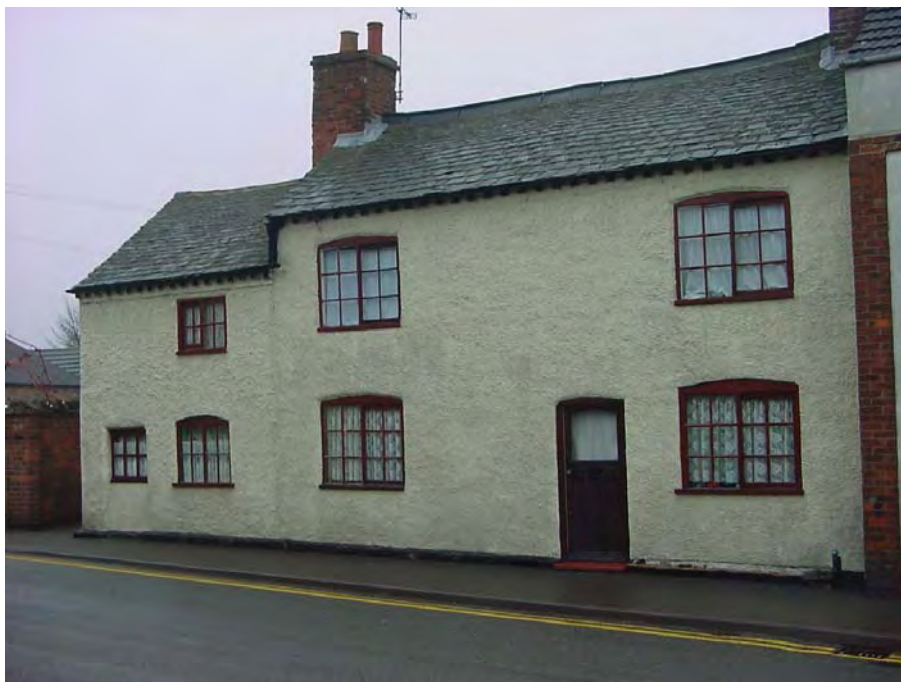
116/118 Main Street is a rendered property with a slate roof.
