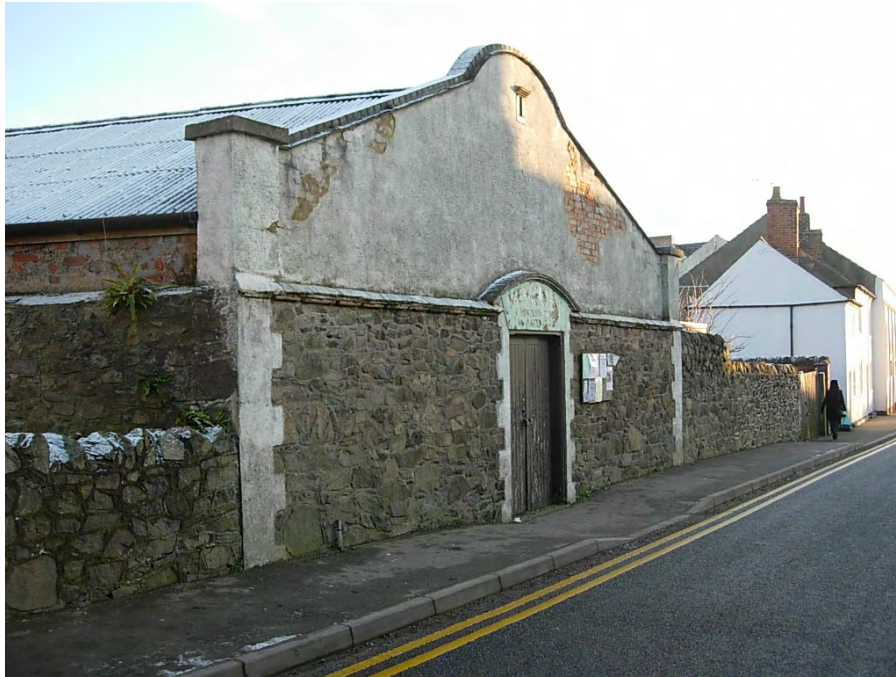
There are proposals to demolish the Miners Welfare Hall on Main Street that was once the village cinema. Redevelopment of the site should respect traditional design elements of the village and materials.
