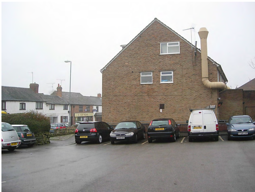
The metal extract flue attached to the gable of 99 Main Street is particularly unsightly. Consideration should be given to reducing its visual impact in this prominent position.
