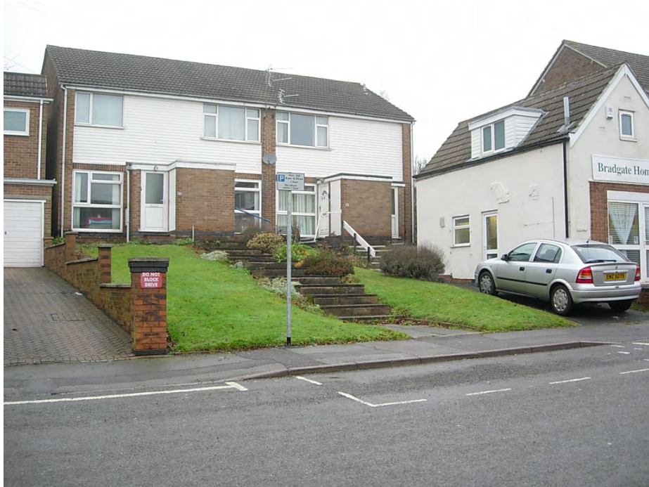
The enclosure fronting the flats at 87 Main Street has been lost. A granite wall needs to be built along the road frontage.
