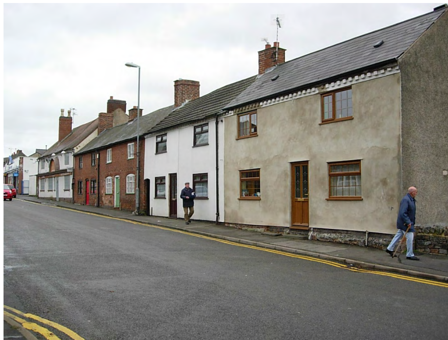
View looking at the east side of Main Street towards The George Pub. This fine terrace of properties has lost some of its traditional character due to insensitive alterations to individual buildings.
