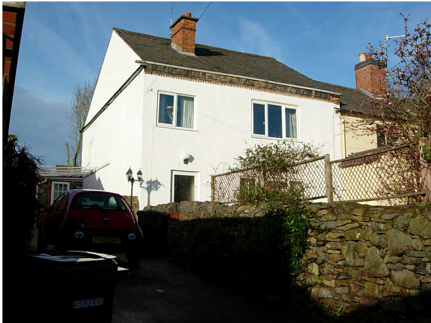
The increase in window openings at 195 Main Street has had a detrimental impact on its appearance.
