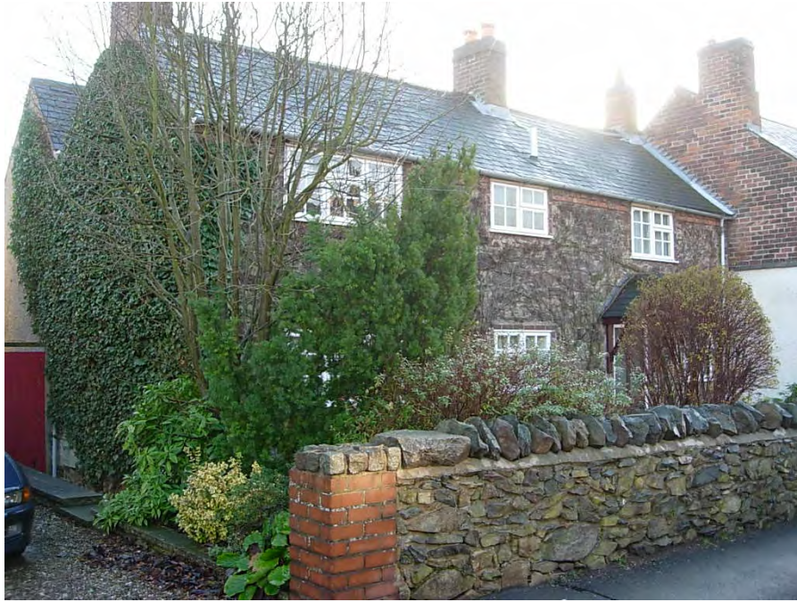
168 Main Street is an excellent stone cottage that has a fine granite wall along its frontage. The property has a slate roof, timber windows and has retained its chimneys.
