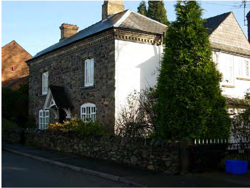
188 Main Street is an attractive property with a slate roof and decorative dentil course along its eaves. Unfortunately, it has lost its chimney pots.
