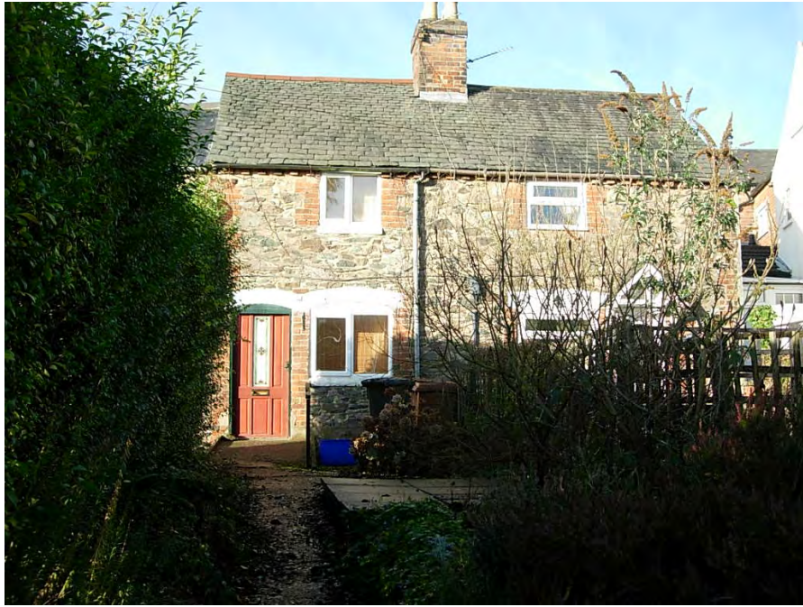
207 - 209 Main Street has retained many original features including a slate roof and chimney, unfortunately its appearance is damaged by plastic windows.
