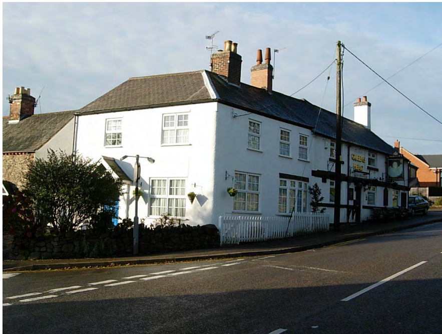
211 Main Street and the Queens Head pub on Ashby Road have retained their slate roof and chimneys but the plastic windows have a detrimental impact.
