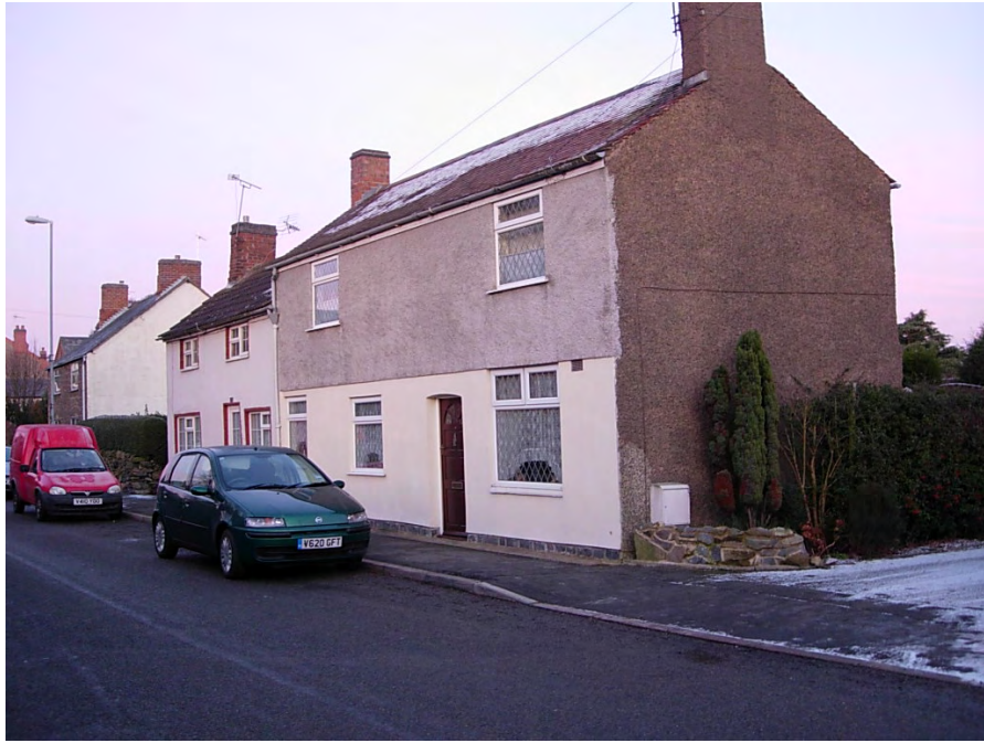
158 and 160 Main Street have different roof heights. Both have had plastic windows inserted. 158 has a Rosemary tiled roof and 160 a concrete tiled roof.
