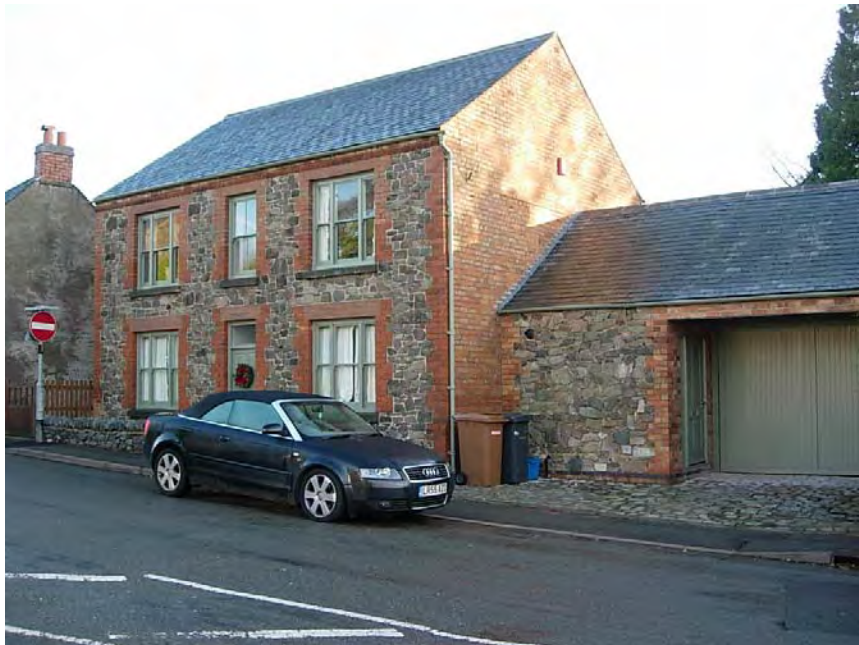
192 Main Street is a fine property that has retained its sash windows but has lost its chimney stacks.
