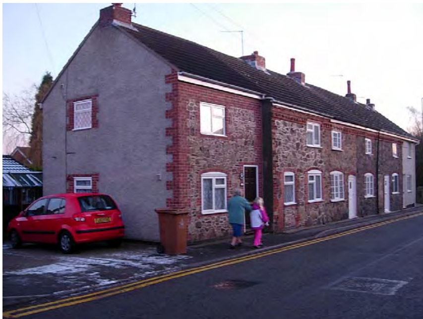
144 – 152 Main Street is still a pleasant terrace despite being considerably modernized and extended. The height of the eaves has been raised, window openings changed and concrete roof tiles used.
