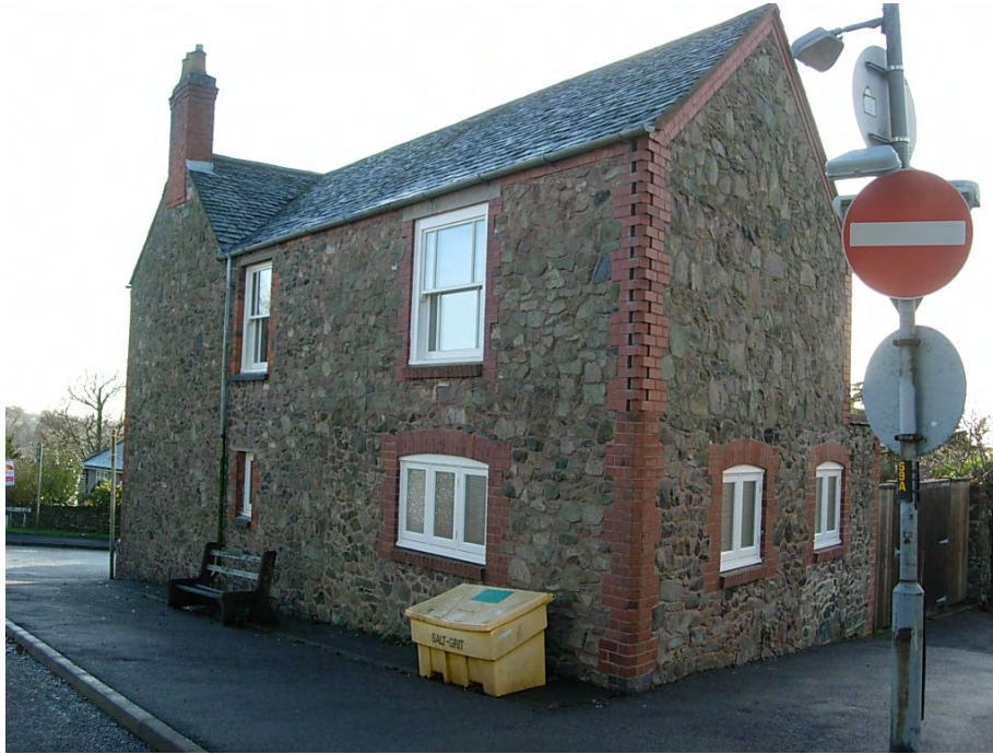
View of the old Police House from Ashby Road. The windows of the property are being replaced with traditional sash windows.
