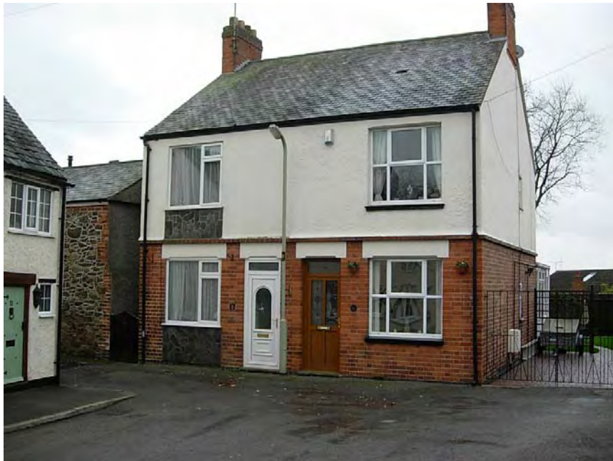
The unity of the semi-detached dwellings, 17–19 The Nook, has been lost with the use of stone cladding under the windows of one of the properties.
