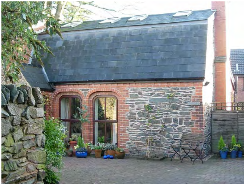
The modern dwelling 186 Main Street is unusual in having a Mansard roof.
