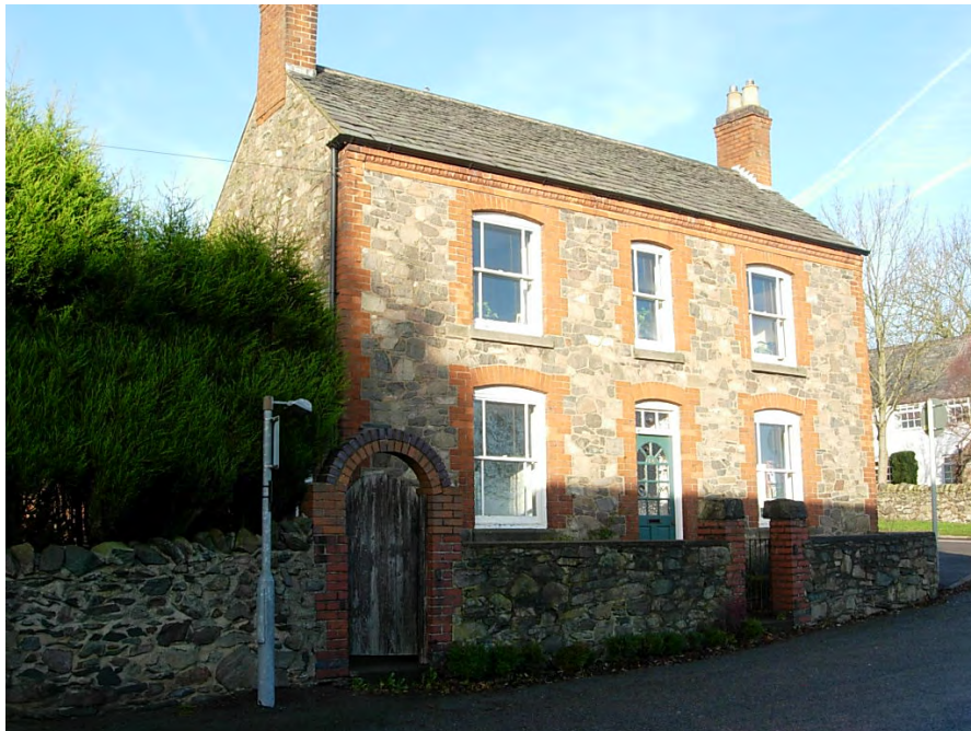
196 Main Street, the village's old police house occupies an important position at the road junction with Leicester Road and Ashby Road. The property has retained its sash windows which are currently being refurbished.
