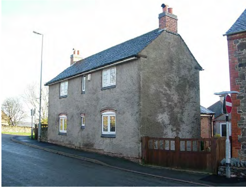
194 Main Street is an interesting property at the junction of Main Street and Leicester Road that suffers from inappropriate render and plastic windows.
