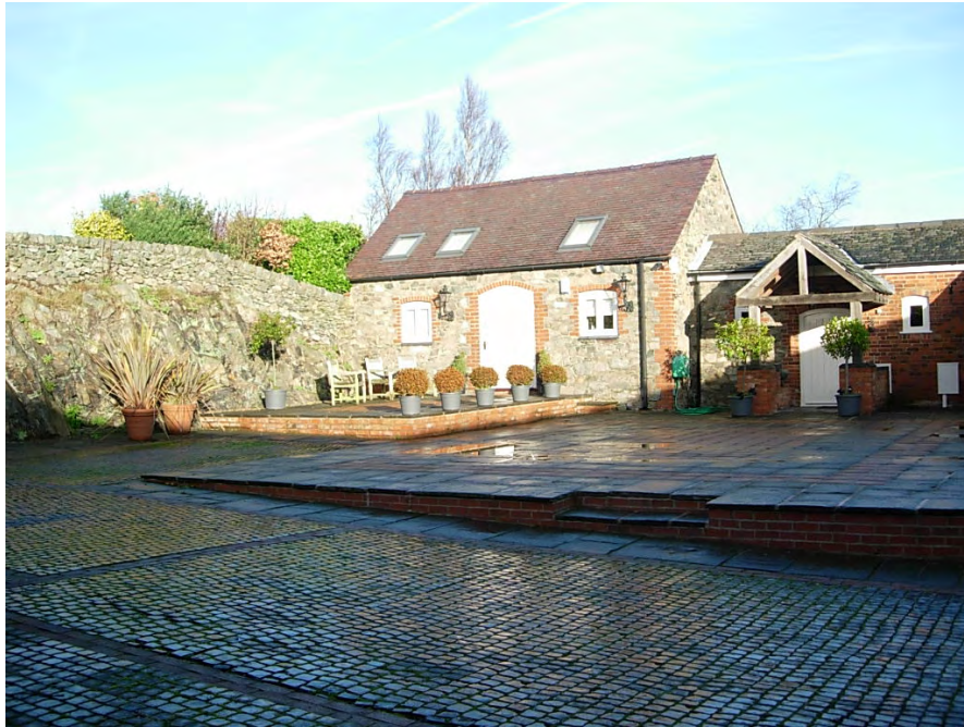
View of the outbuildings at Townhead Farm that have been converted to residential use. The roof lights on the front elevation are very prominent and do not enhance its appearance.
