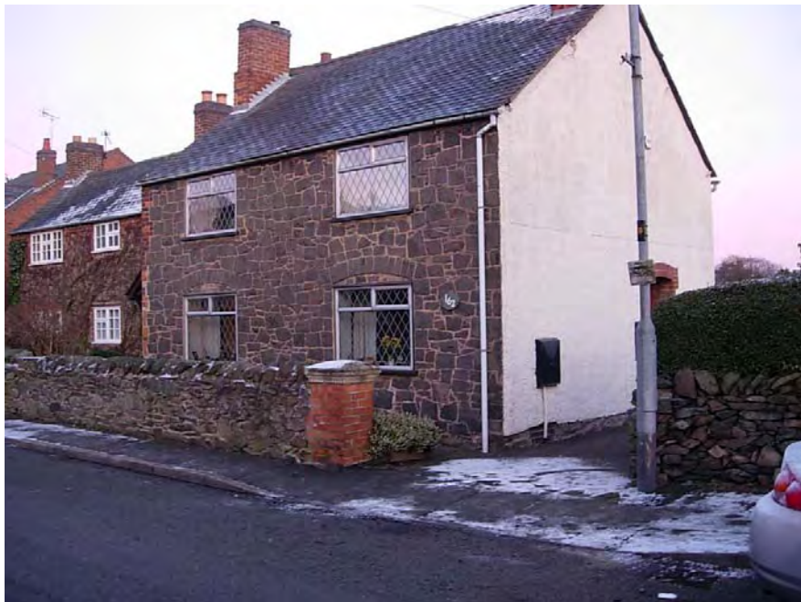
162 Main Street is a stone property rendered on its gable with a slate roof. Its chimney stacks have been rebuilt and new windows inserted.
