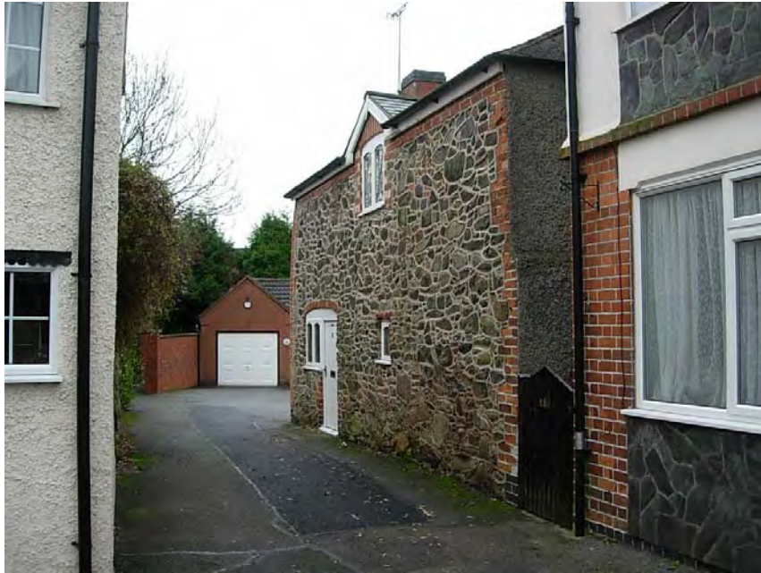
15 The Nook is a stone cottage whose appearance has been altered. The recent addition of a fine stone gable has provided a new feature in the street scene.
