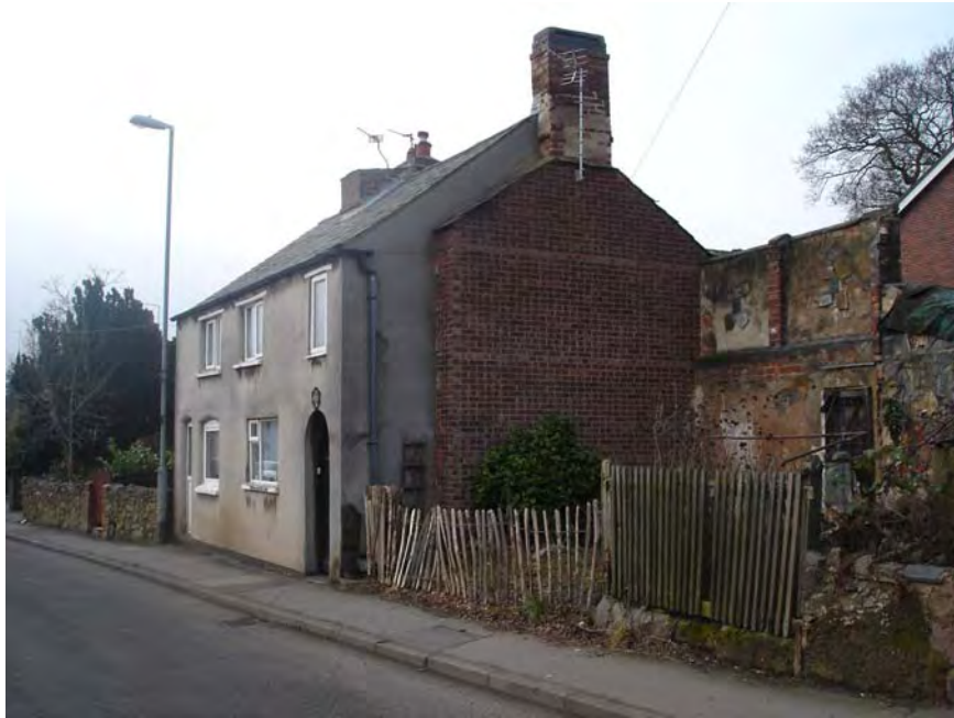
The brick skin built on the end gable at 173 Main Street to stabilise the premises is unsightly. There might be potential to build another dwelling on the adjacent land.
