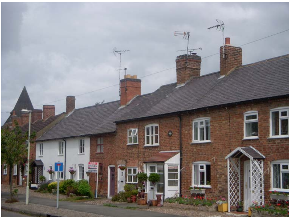
Some rustic features remain on the workers cottages along 21 – 33 Main Street
