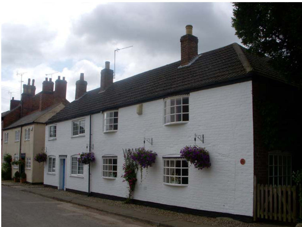
4 and 6 Main Street have had unsympathetic alterations including bow windows, replacement plastic windows with thick frames, and concrete roof tiles. The original cobbled surface outside the dwellings still remains and is fronted by a granite kerb stone
