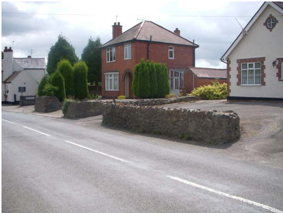
Only the boundary along the road fronting the properties at 26 to 30 Main Street is in the conservation area, but the open frontages and design and setting of the dwellings detract from the character of the conservation area
