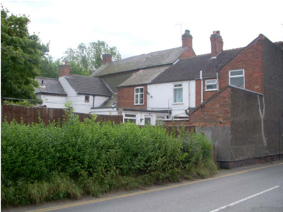
There are mixed floor levels at the rear of the properties on 35 to 41 Main Street
