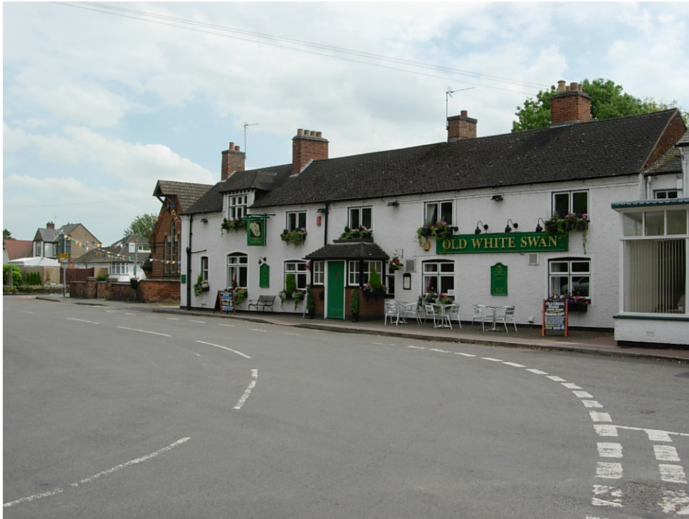
The Old White Swan public house on Main Street is a wide building on the bend of the road. The property could be improved with the concrete roof tiles being replaced with a traditional material
