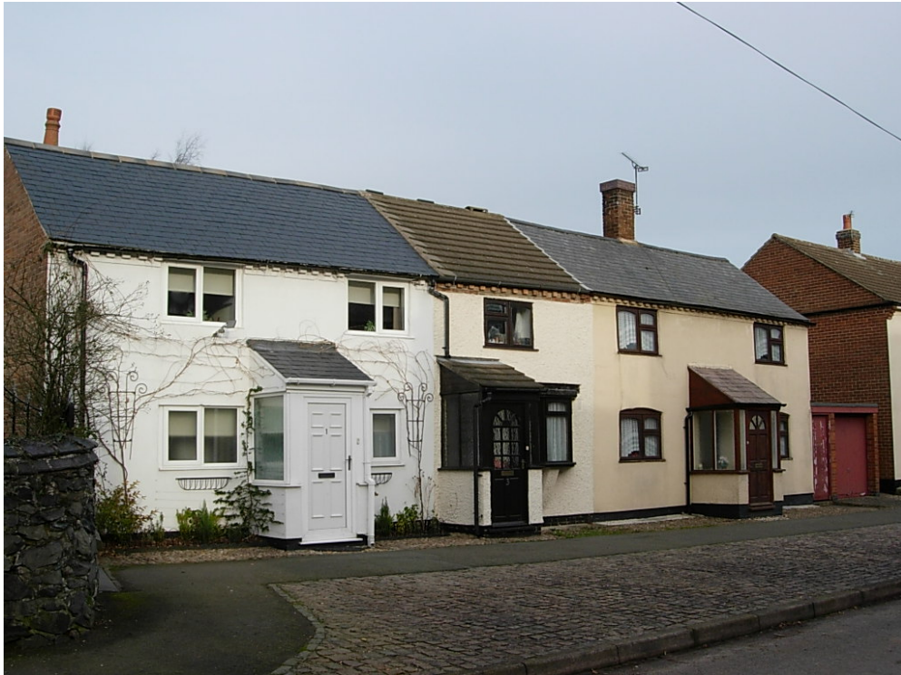
1 to 5 Main Street have been painted and rendered and have had unsympathetic modern additions including porches, plastic windows, and concrete roof tiles
