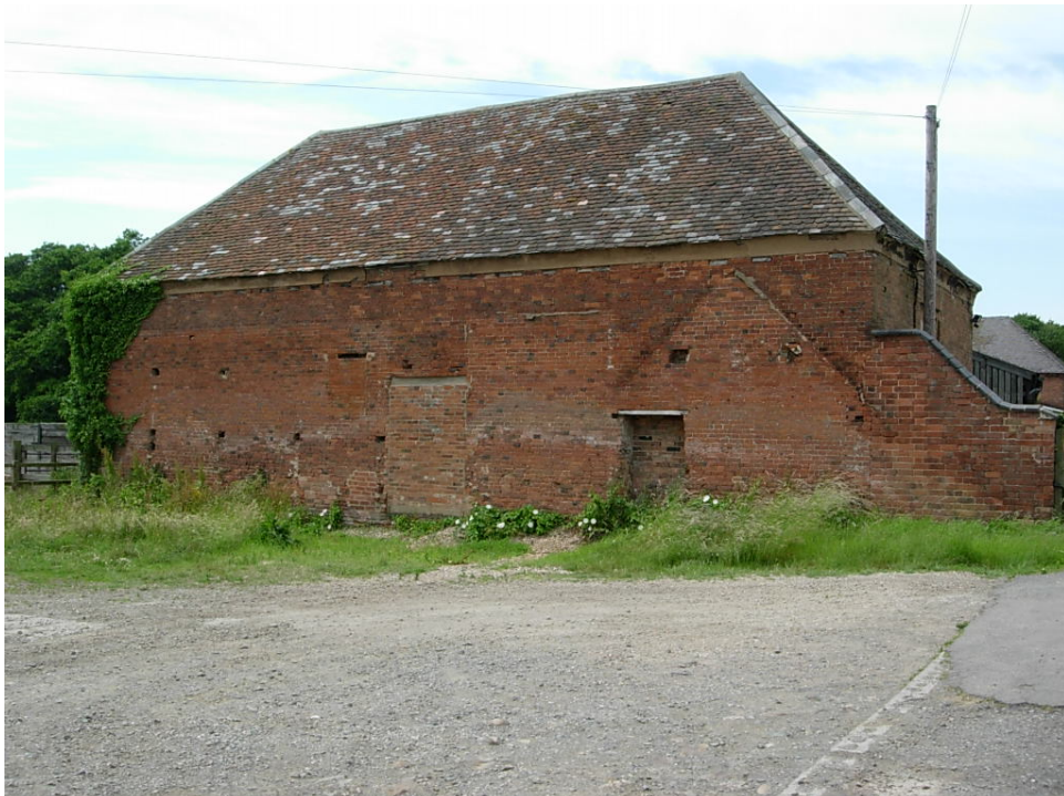
The listed pavilion at the south east corner of Newbold Verdon Hall forecourt is now utilised as a farm building. There is an excellent vista to the south into open countryside over the land fronting the pavilion
