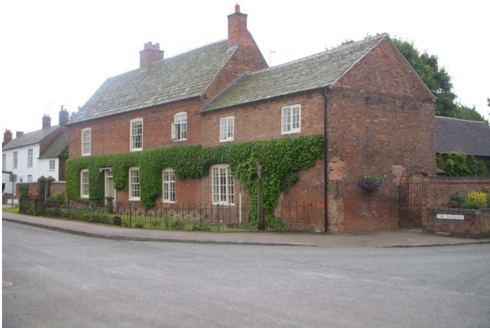
The listed Church Farm has interesting features including Swithland Slate roof tiles and a wrought iron fence along the front boundary. Modern alterations to the dwelling have been sympathetic to the character of the conservation area
