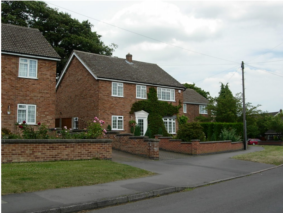
The detached dwellings at 51 to 55 Main Street are set back from the street with large front gardens enclosed by modern walls which go against the traditional feel of the conservation area
