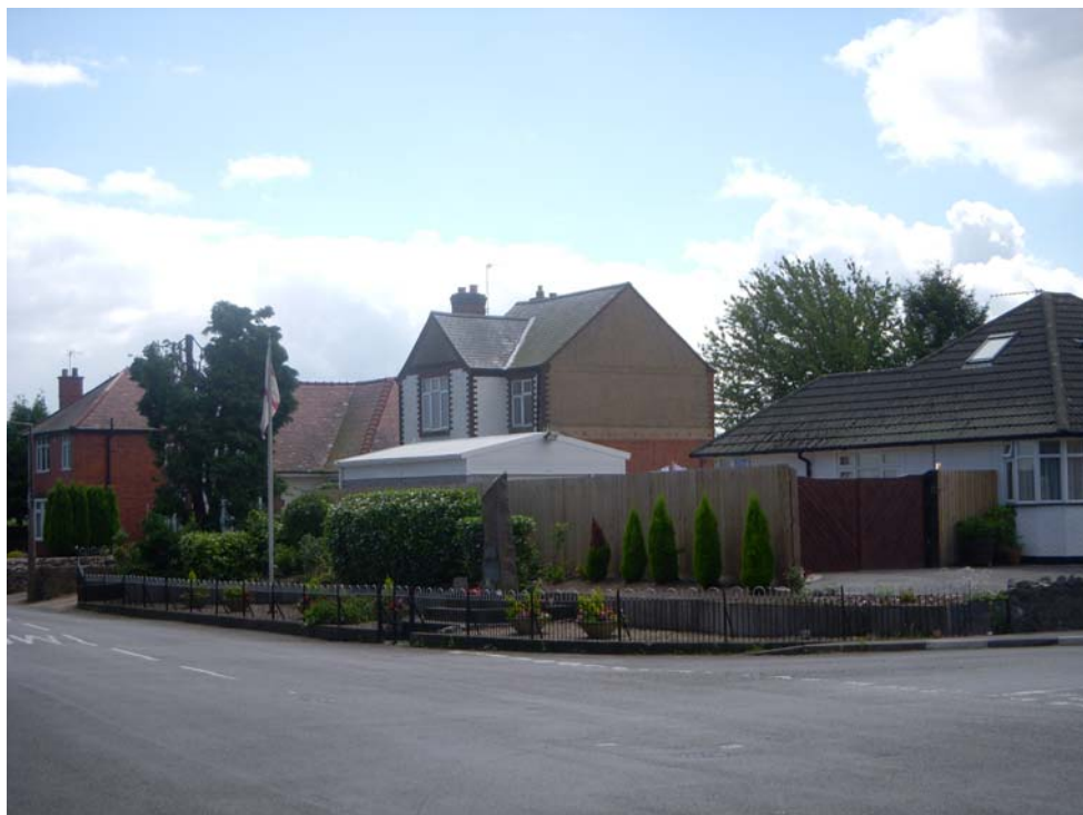
When looking towards the war memorial the unfortunate ground levels make the concrete sectional garage at 2 Brascote Lane too prominent. The war memorial could be improved with traditional hard landscaping and vegetation screening along the rear boundary
