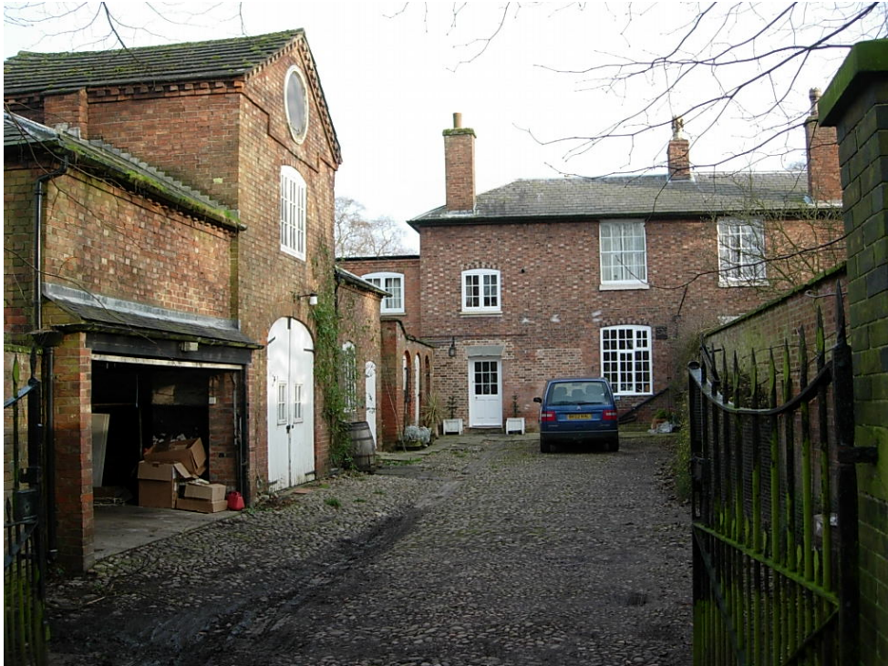
There is an important view from Bells Lane towards the grade II listed old Rectory. The use of the outbuilding as a double garage does detract from original rustic charm of the building.
