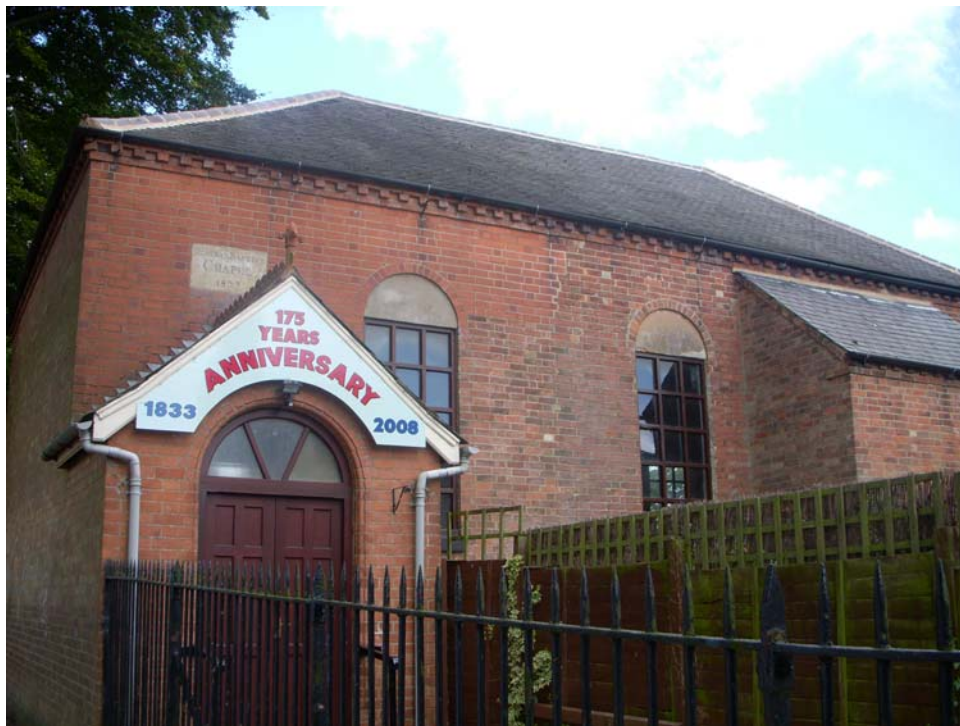
The frontage of the Baptist Church is accessed from Mill Lane. The church would benefit from some minor maintenance including painting the metal fence to the rear of the church bounding the recreation ground
