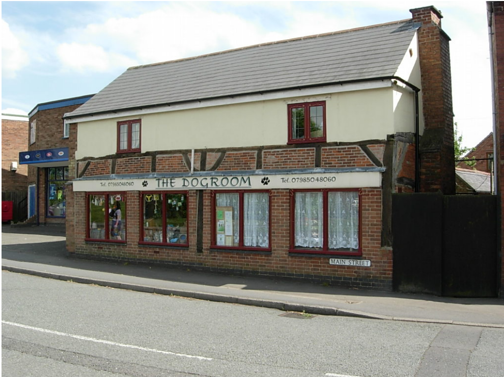
Although not in the conservation area, 62 to 64 Main Street is an interesting building with the original timber frame still remaining
