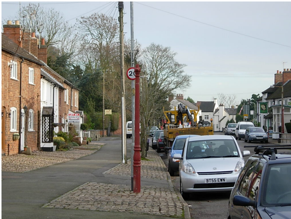
As part of the Environmental Improvement Programme (EIP) heritage cast iron lamp posts have been installed, replacing their modern counterparts
