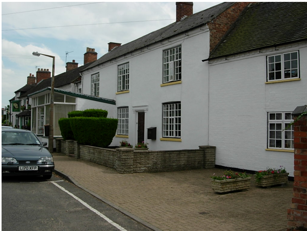
The frontage of 18-20 Main Street could be improved by the modern wall being replaced with a traditional wall, enhanced hard landscaping, and the removal of the 1950s office extension
