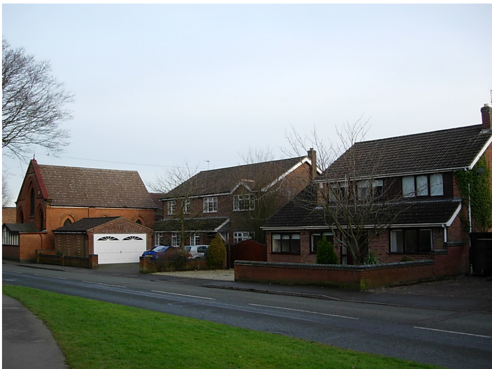
The modern dwellings at 38 and 50 Main Street detract from the traditional feel of the conservation area. The large double garage at 50 Main Street hinders views of the Methodist Church
