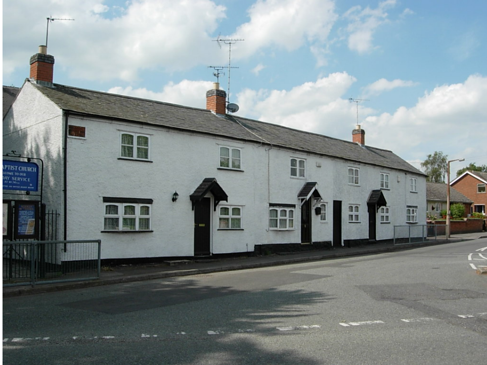
The traditional character of the cottages at 1 to 7 Mill Lane has been compromised by the addition of wooden canopies, modern and bow windows and a satellite dish
