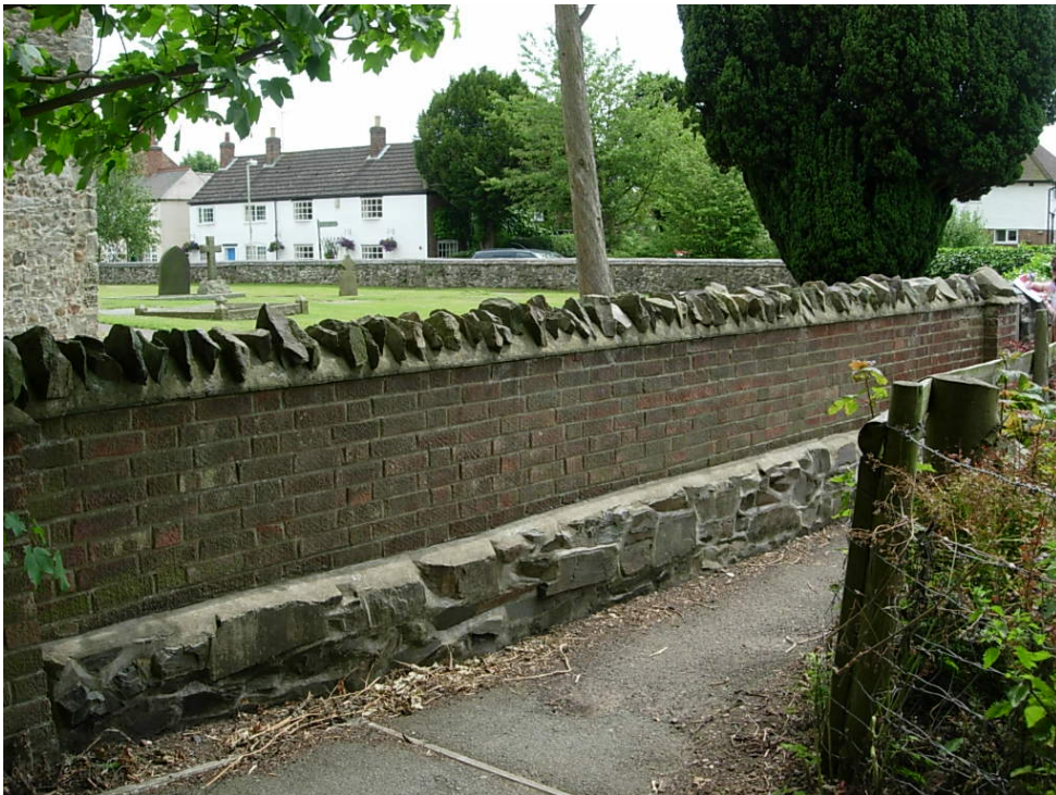
The modern wall bounding the footpath in St James's church yard could be improved by being replaced with a traditional stone wall with saddleback coping
