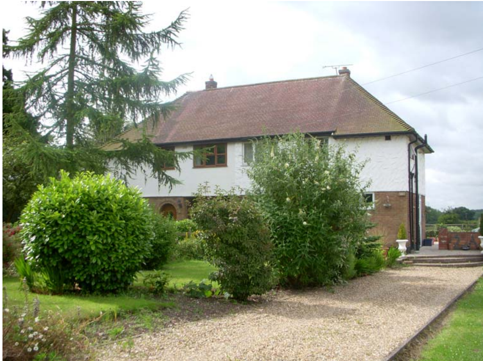
2A and 4A Main Street are a pair of semi-detached dwellings out of keeping with the character of the conservation area
