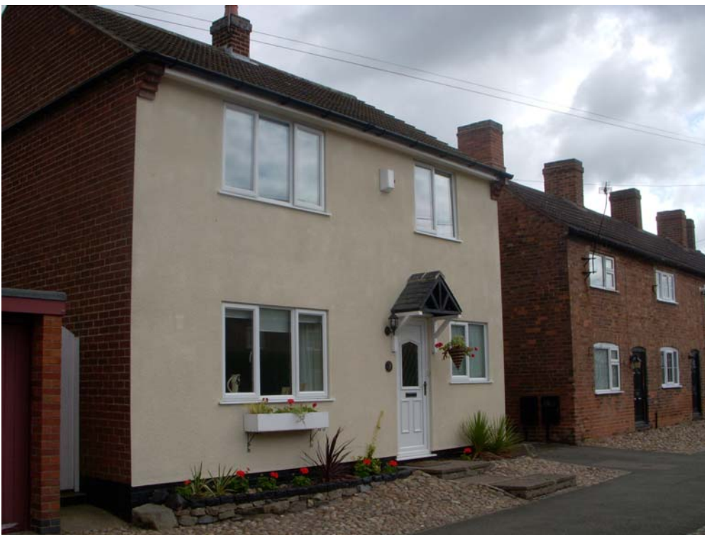
7 Main Street has not been built to the street line with the scale too large and the ridge and eave level too high
