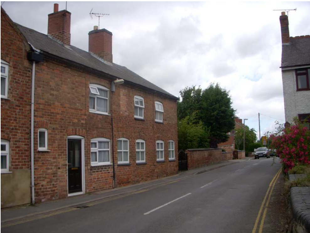
The windows at 1 to 5 Dragon Lane are modern additions with frames that are too large, though some are wooden. The modern wall adjacent to 5 Dragon Lane has been constructed in a traditional manner with reclaimed red brick
