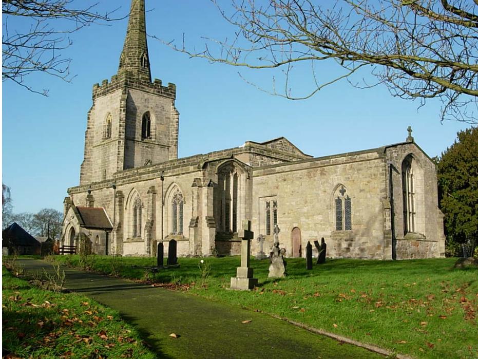
The parish church of St Edith is an early C14 grade 1 listed church with its tower and spire built of ashlar stone with low pitch roofs.
