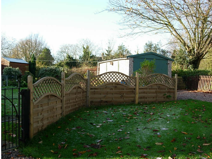
The timber fence and pre-cast concrete garage are unattractive features that tend to spoil the area around the parish church. The fence needs to be replaced with a privet hedge
