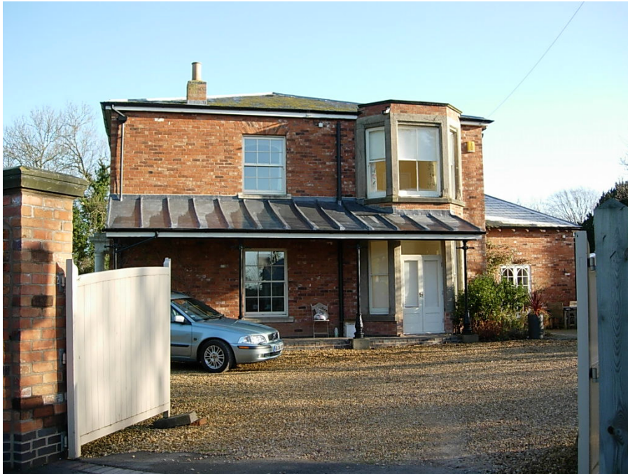
The property, Highlands which is set back from Warton Lane is a period dwelling that has an unsympathetic canopy attached to its front elevation.
