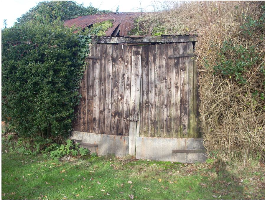
The garage that fronts onto the village green is an unattractive feature in need of maintenance or removing.
