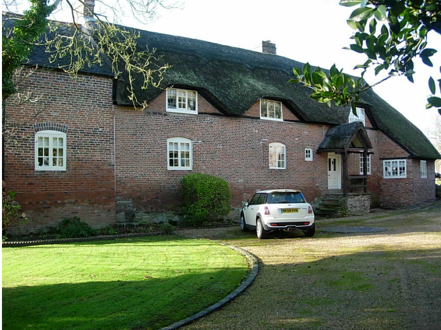
Church Farmhouse is a Grade 2 listed property that has a timber framed core of cruck construction with outer walls of red brick, thatched roof and brick ridge stack.
