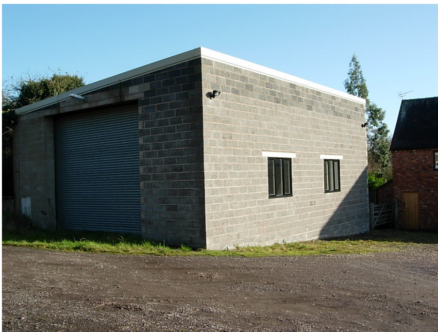
The large garage at Hall Farm built in concrete blocks tends to detract from the setting of the Farms setting.
