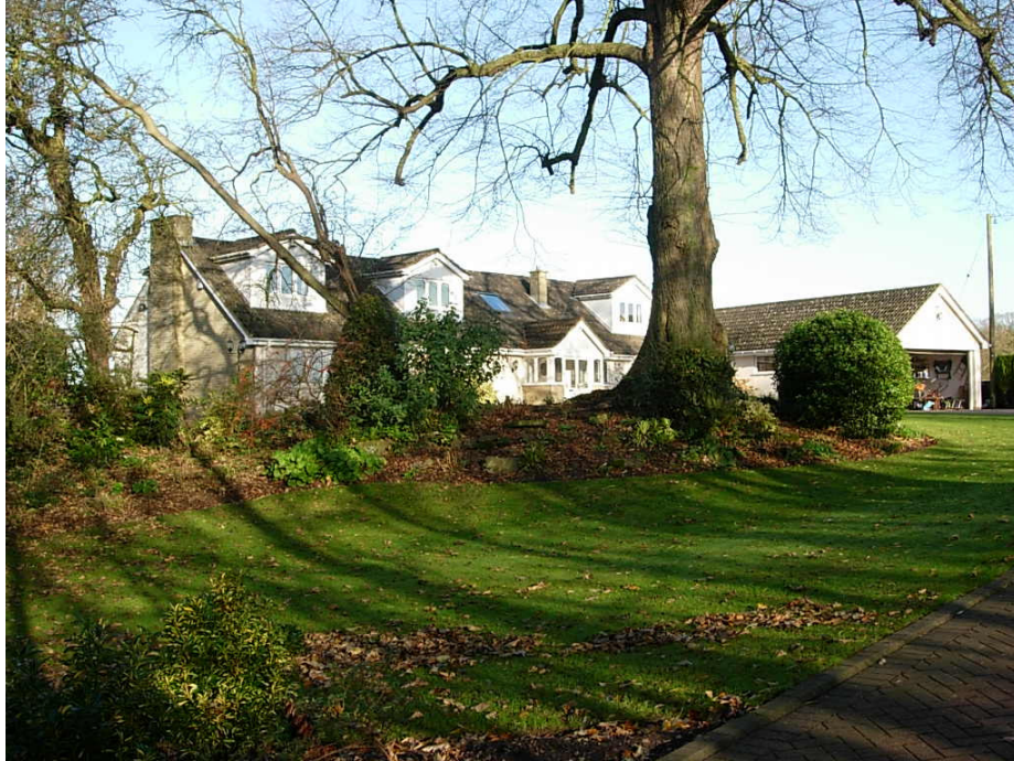
The rear of 1 The Green. The use of dormers is not a traditional feature in Orton.
