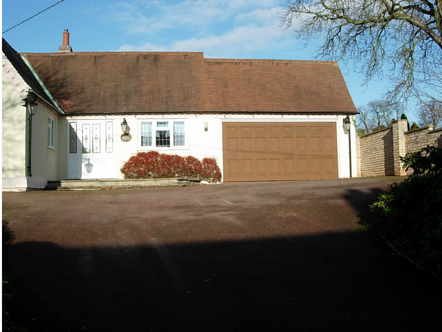
The double garage at 10 Pipe Lane is out of scale with the property. Its impact could have been reduced considerably if a pair of garage doors had been utilized.
