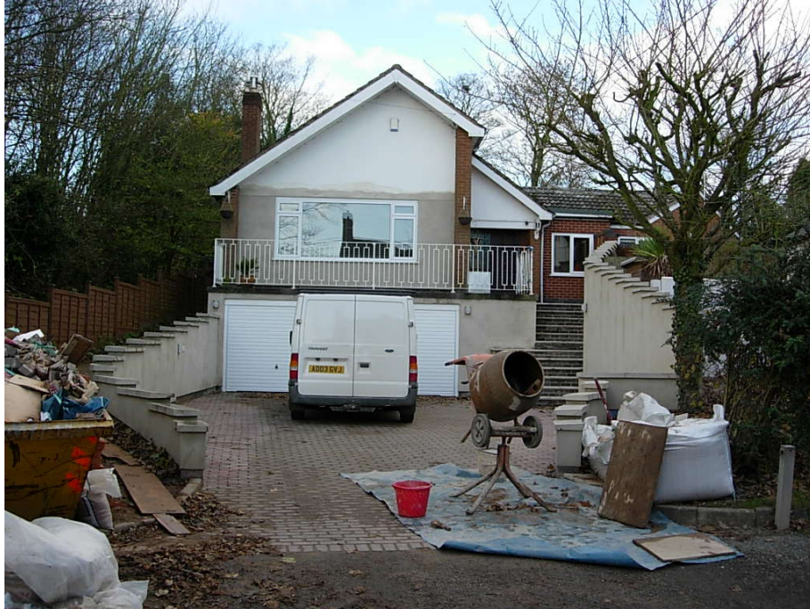
The modern design of 15 Main Street, which includes an integral Garage, verandah and rendered walls, is totally out of character with the traditional core buildings and walls in the conservation area.
