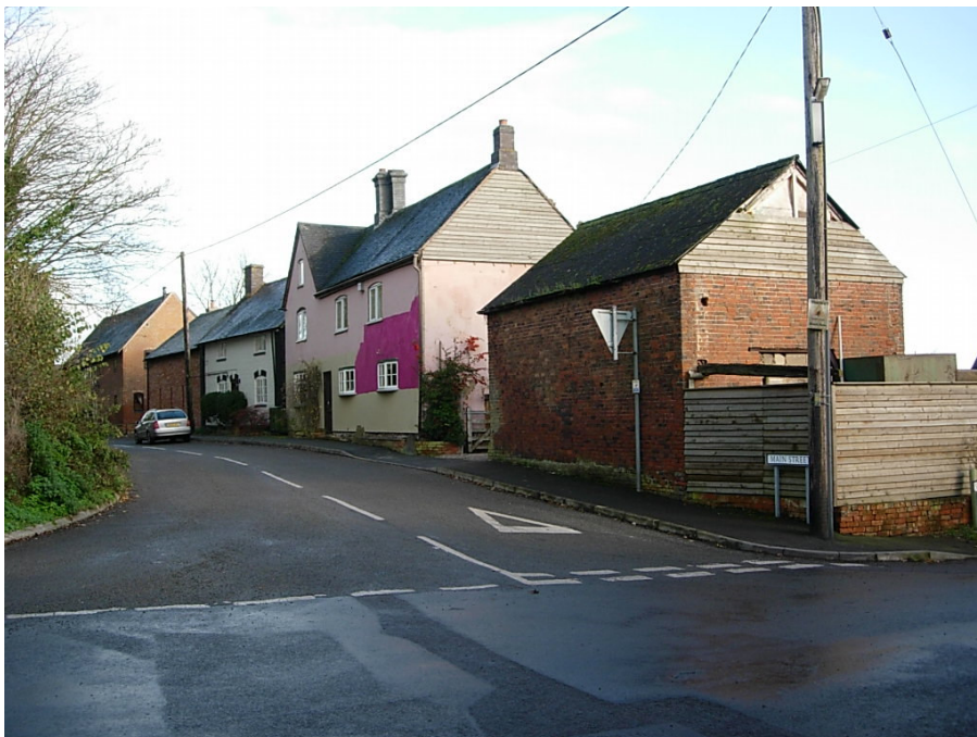
This pleasant group of properties on Main Street is spoilt by the unsympathetic treatment to the gable ends with timber planks used as cladding and corner fence. The colour of the rendering and use of bow windows is also unfortunate.
