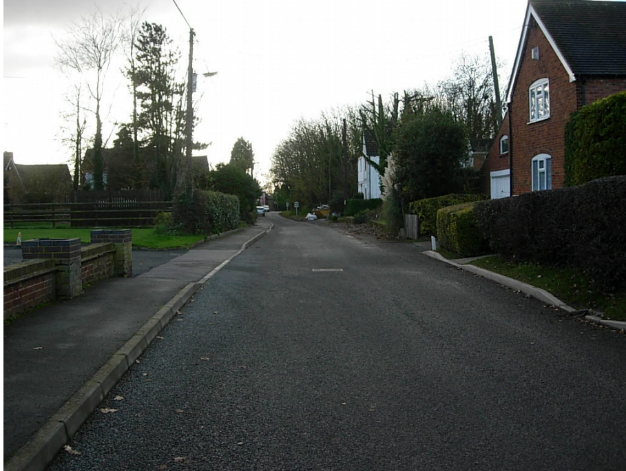
View looking down Main Street showing how the construction of a footpath and use of concrete kerbs can have a marked detrimental effect on the visual quality of a conservation area.
