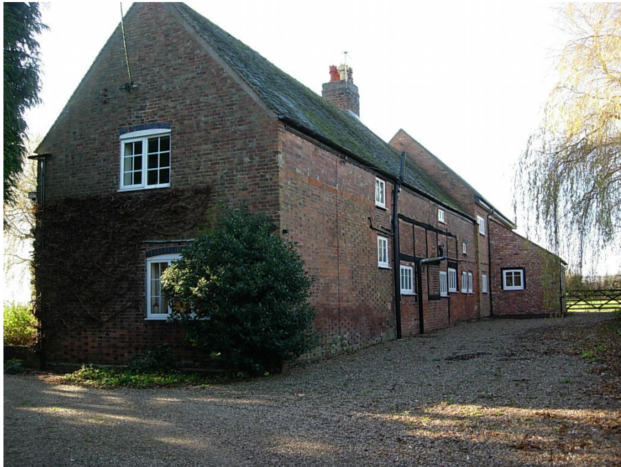
The plastic drainage pipes on the side of Peggs Farm spoil the visual quality of this property.
