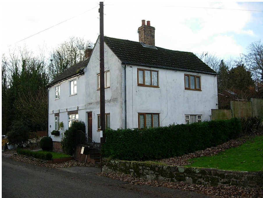
The concrete roof tiles at Ivy Cottages are a modern material that detract from the character of the conservation area.
