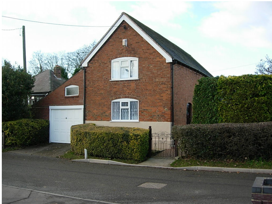
The pitched garage roof at 21 Main Street runs in the same plain as the main dwelling which gives rise to an unusual appearance.
