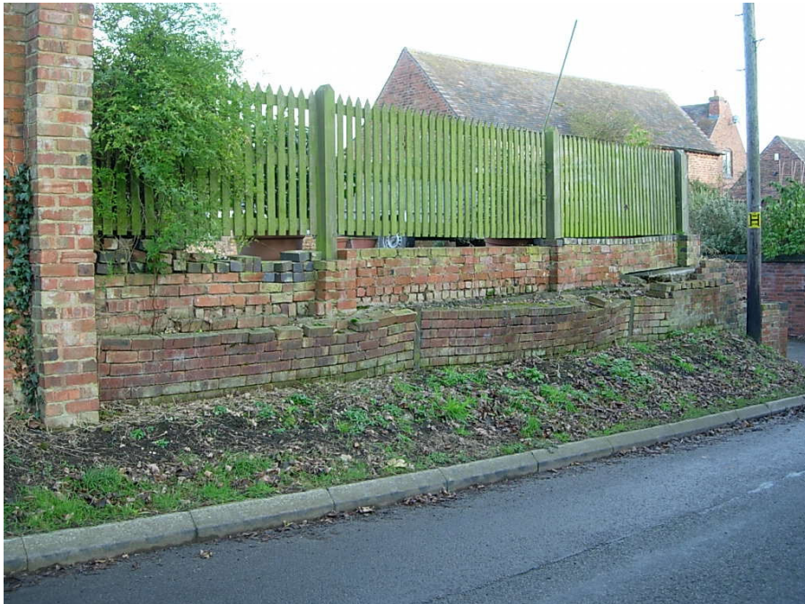
This area on Sheepy Lane could also be improved with the rebuilding of the brick wall.
