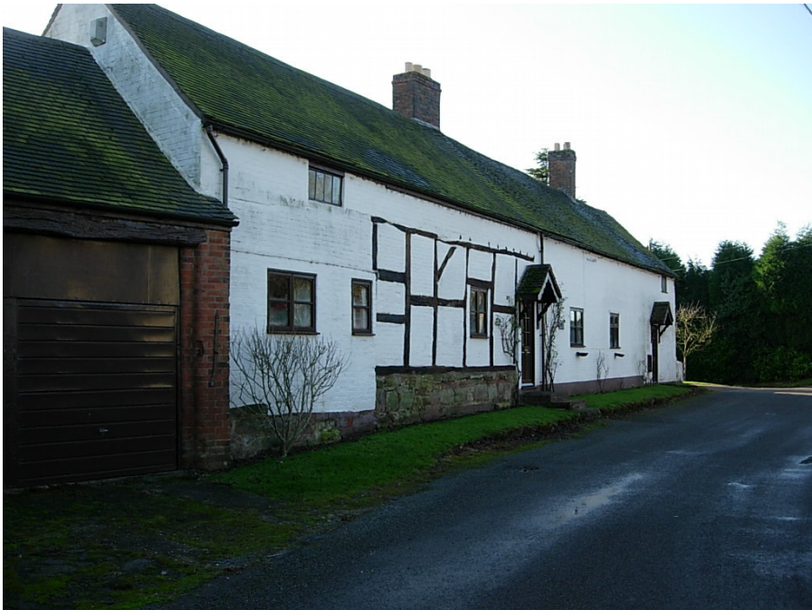
Lower Farmhouse is an excellent C17 Grade 2 listed property, timber framed on a stone plinth with painted brick infill panels and plain tiled roof. The property forms part of a picturesque group of dwellings.
