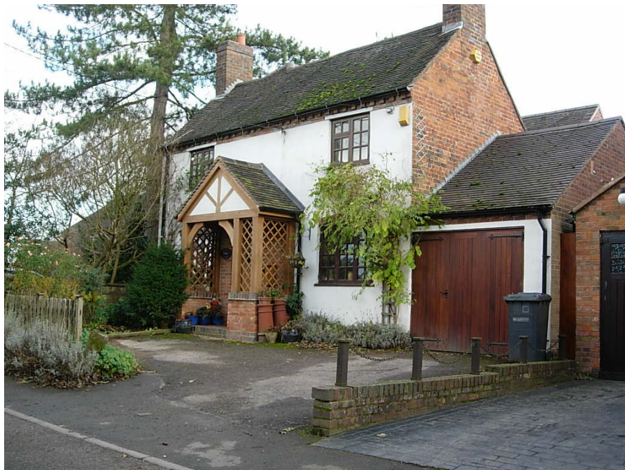
The front porch at Yew Tree Cottage has an overbearing impact on the property.
