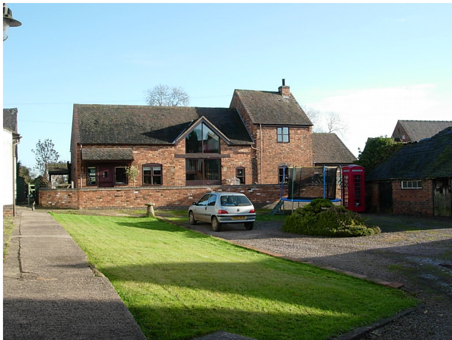
The inner court yard at Lower Farm showing the conversion and modernization of one of the farms outbuildings that incorporates features which are out of character with traditional buildings in Orton.
