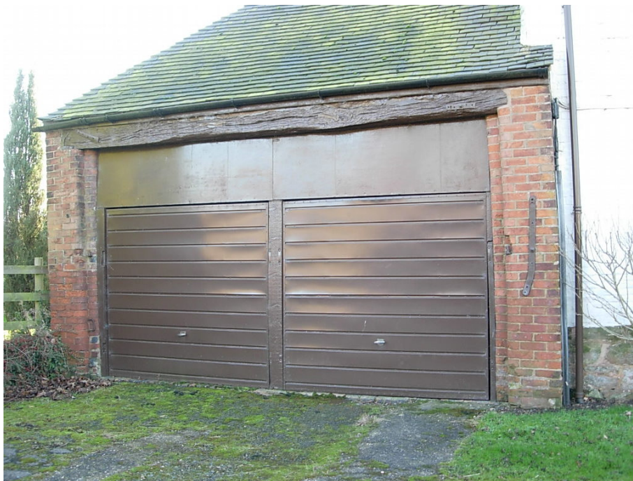
The double garage that adjoins Lower Farmhouse detracts from the traditional character of the listed vernacular building because of the use of modern garage doors.
