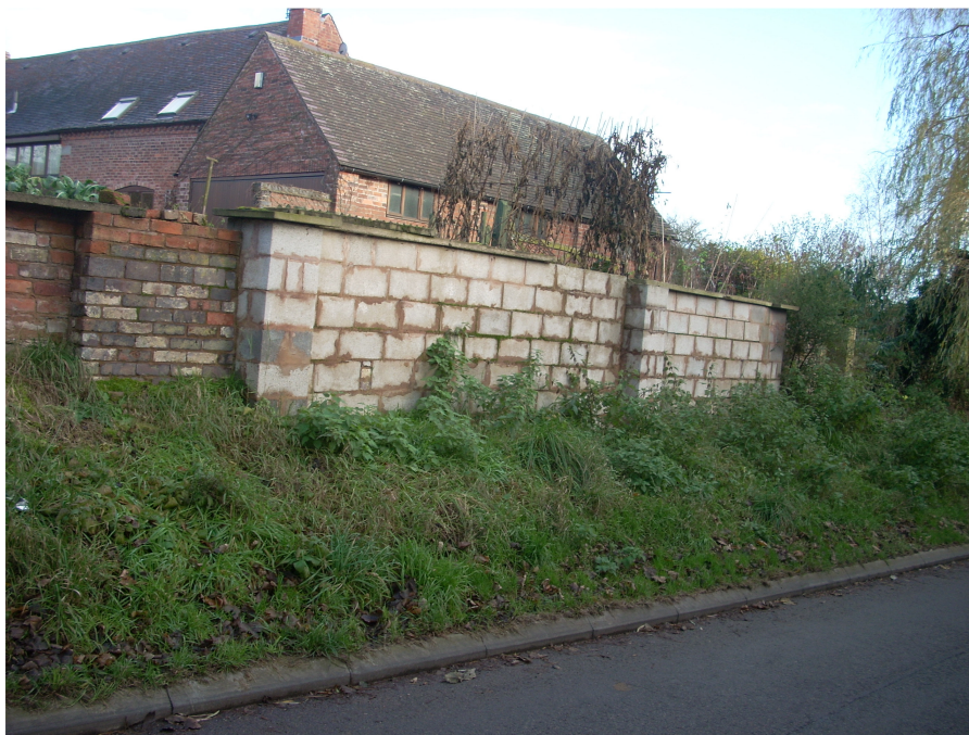
The block wall on Sheepy Lane at the entrance to the village and conservation area is a poor visual feature. A brick course built in front of the wall or its re-building would be of benefit.
