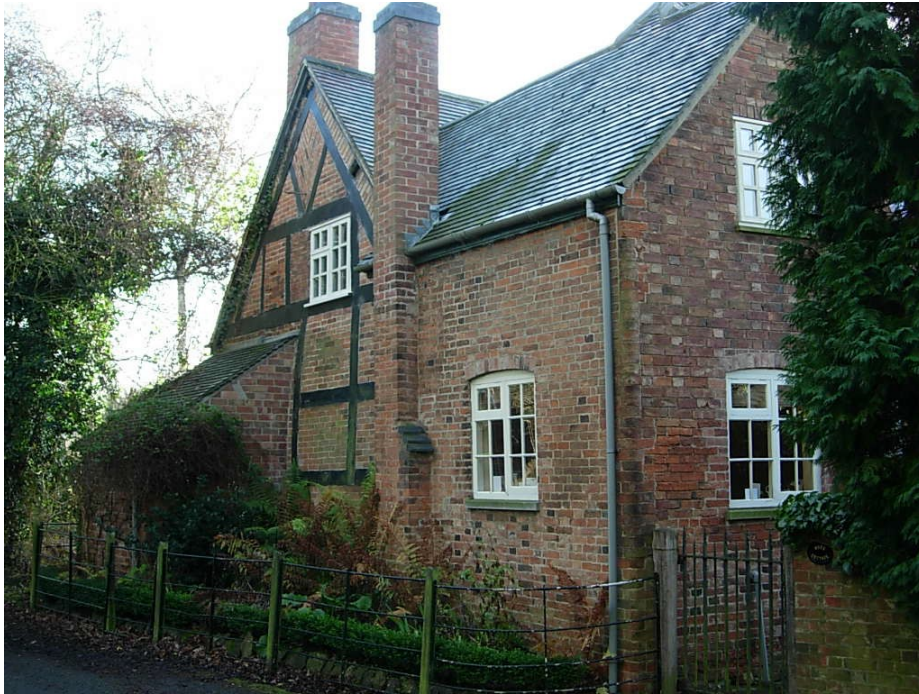
Moss Cottage has been considerably extended with dormers added on both side elevations.
