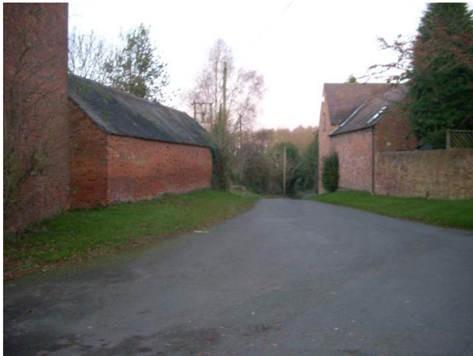
The Home Farm outbuilding and White Boar Barn help to funnel views down Goatham Lane.
