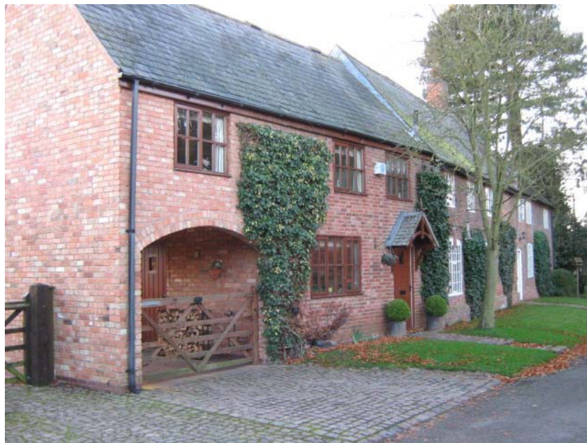
Hall Farm Cottage, once a barn attached to the eastern gable of Hall Farm, has almost been rebuilt into a 2 storey dwelling. Similar to several other dwellings in Osbaston, granite setts, have been utilized to surface its vehicular access.
