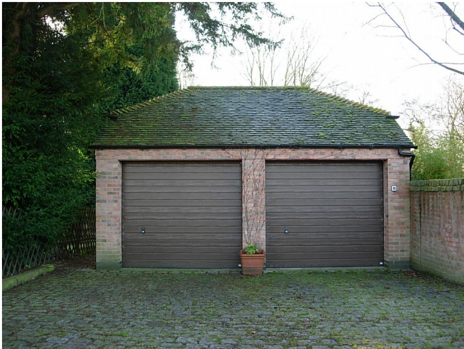
The visual impact this double garage on Gotham Lane is considerably reduced as a result of its roof being hipped and doors painted a darker colour. Granite sets have been sensitively incorporated as a surface material.
