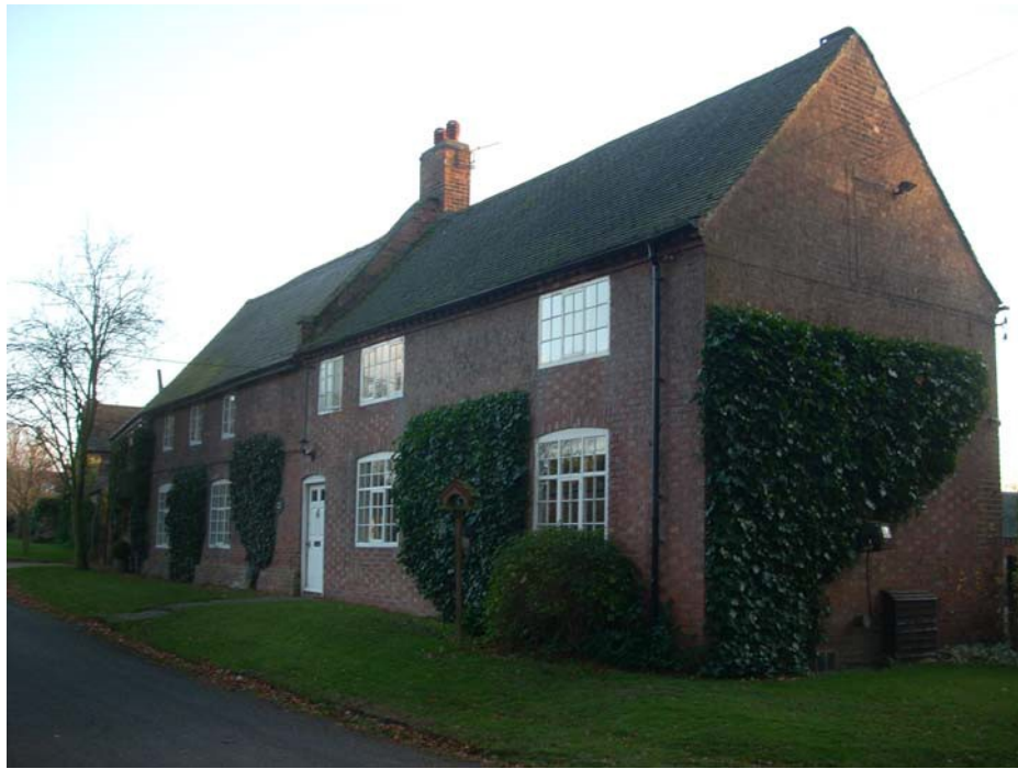
Hall Farm still has one of its original parapet walls that runs up to its chimney stack. The photograph shows how the original farm dwelling has been extended along its frontage.
