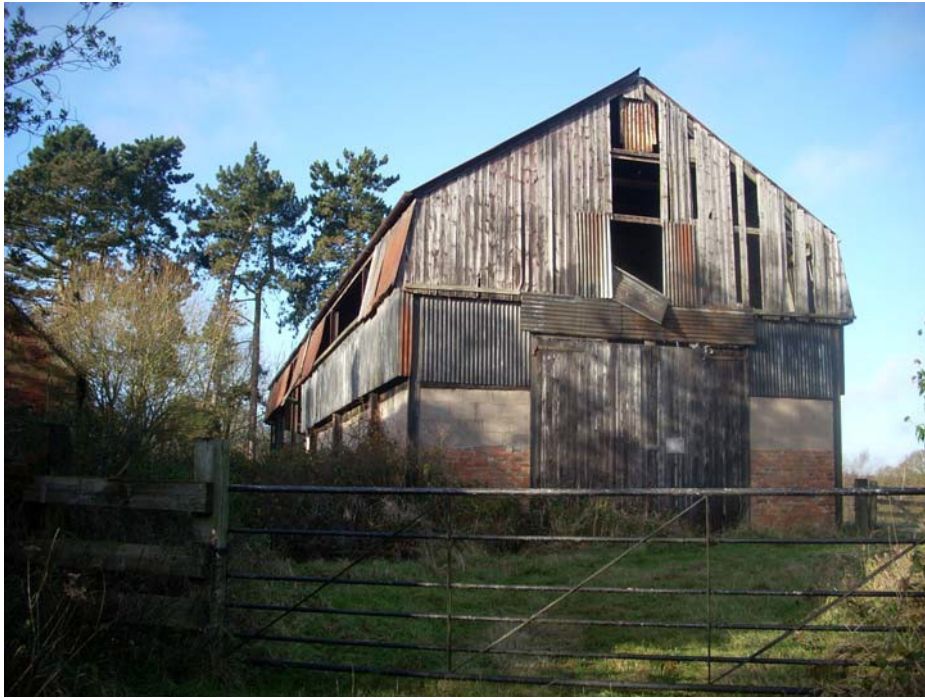
This excellent barn at Home Farm is in urgent need of maintenance.
