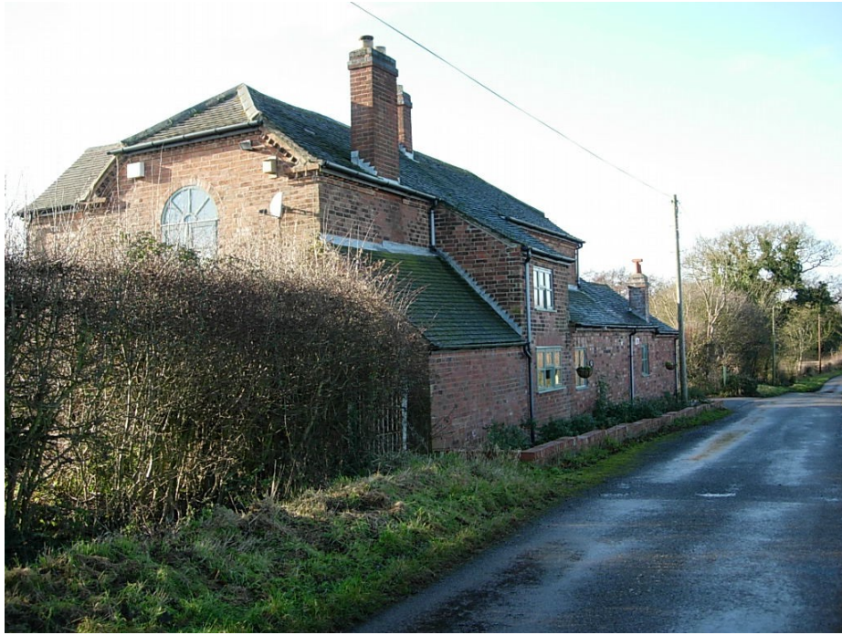
The architectural integrity of Gotham Cottage has unfortunately been lost due to numerous extensions being carried out on the property producing a complex elevation to the street scene.
