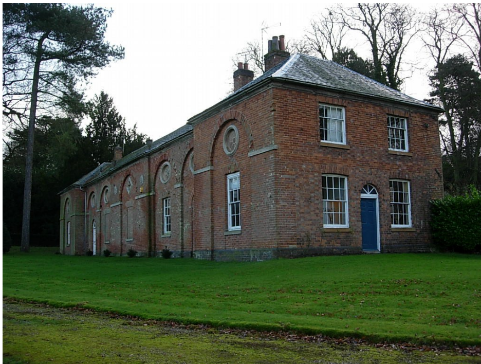
The grade 2 listed stable block and cottage, a late 18 th century brick building with stone dressings and plain tiled roof situated in the grounds of Osbaston Hall.
