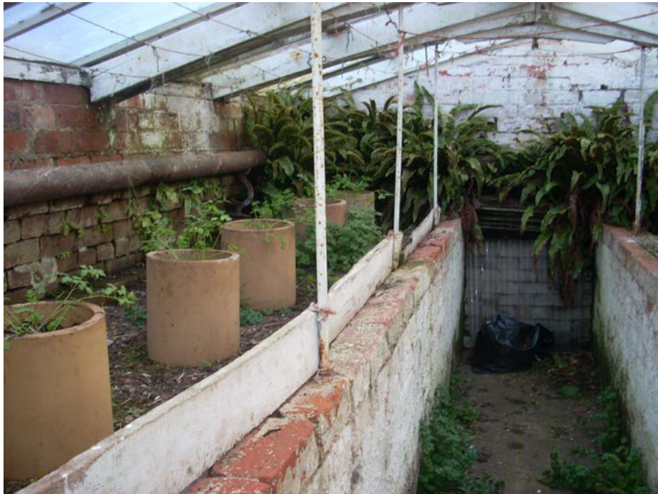
The sunken Victorian greenhouse situated in the walled Garden at Osbaston Hall is in urgent need of restoration.
