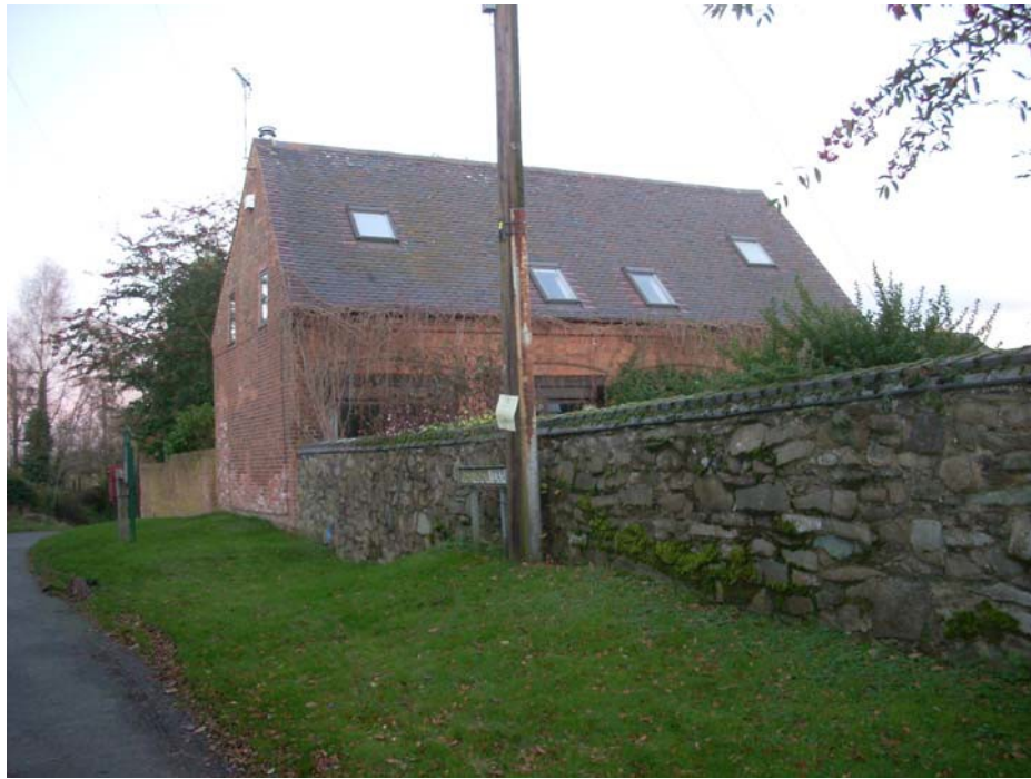
The roof lights on Bloomfield Barn are features that are at discord with its traditional character. The property however, is bounded by an excellent stone wall and wide grass verge.
