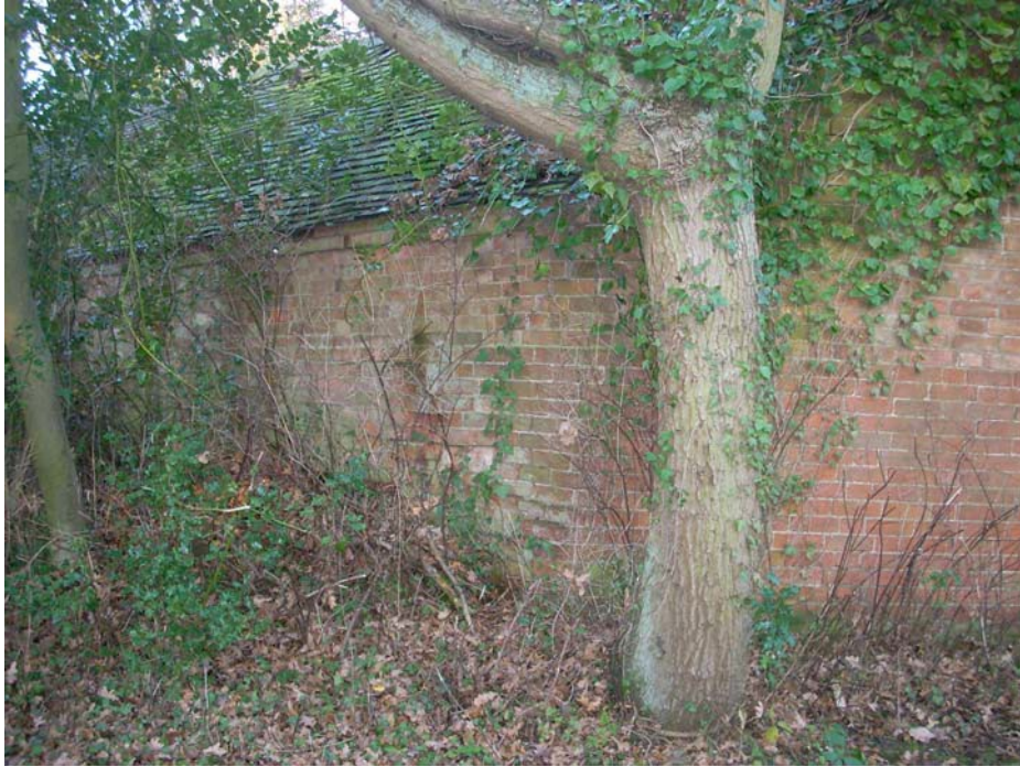
The tree growing adjacent to the derelict barn on Hall Lane should be removed as it is starting to damage the walls.
