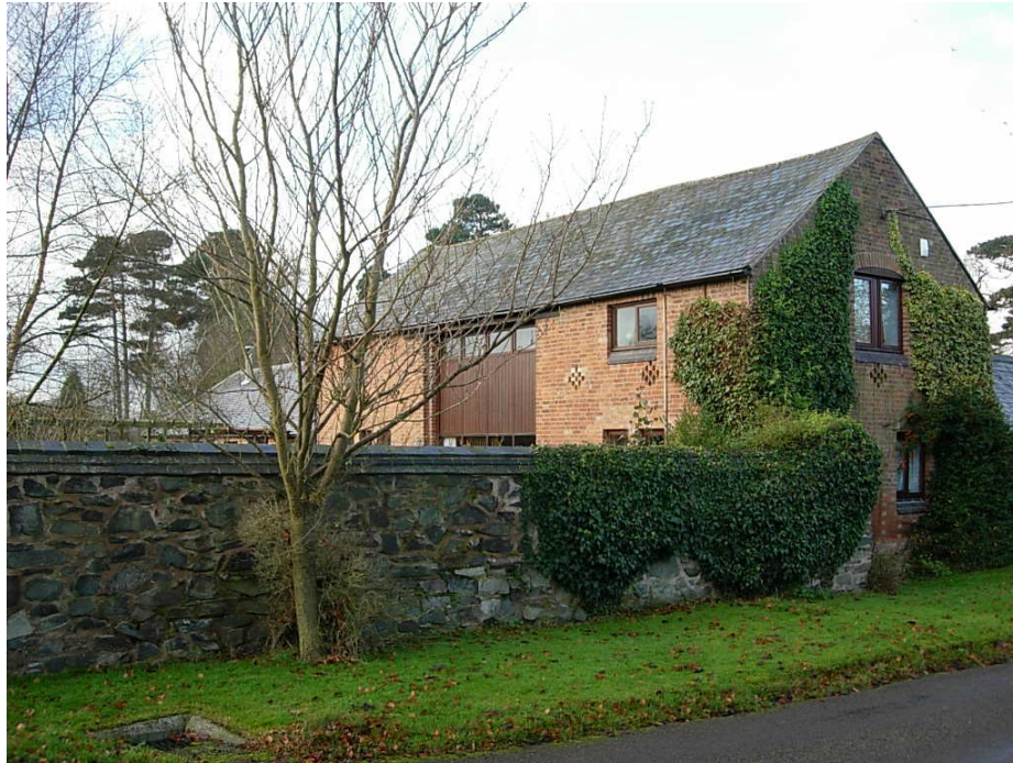
Hall Barn has been converted from a hay barn into a dwelling. The barn's ventilation openings in its side walls are still evident at first floor level
