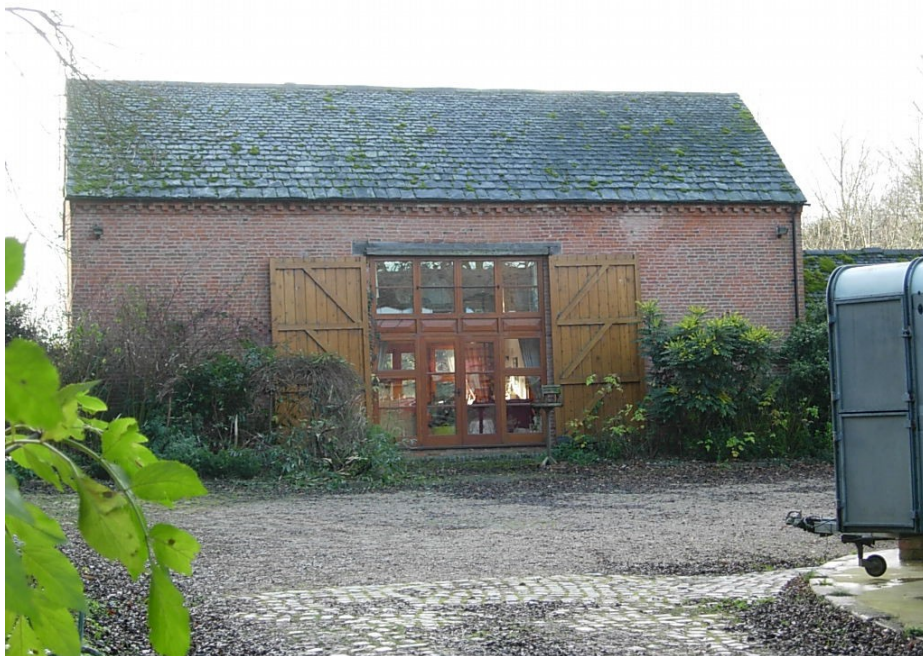
Rookery Barn, like many barns in Osbaston, has been converted into a dwelling. Granite setts have been utilised to surface the courtyard.
