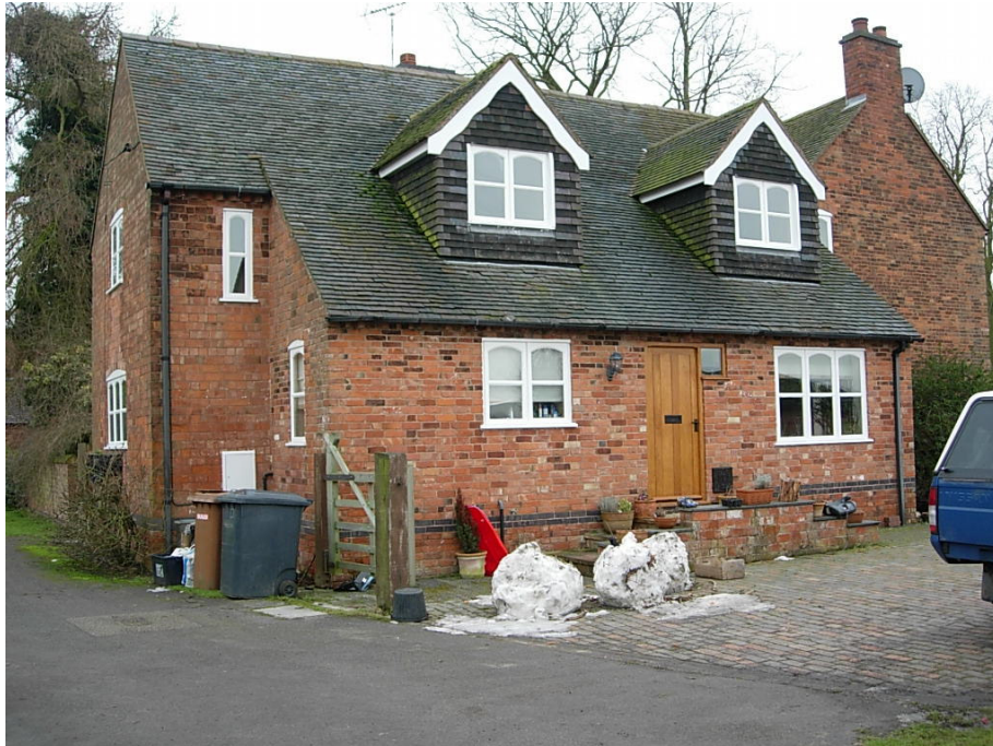
Elmside House is a dwelling sited at the end of Allotment Lane built side ways to the lane. The property has been considerably modernized in recent years and has lost its traditional character. The dormers are out of character and the windows although timber do not follow traditional detailing
