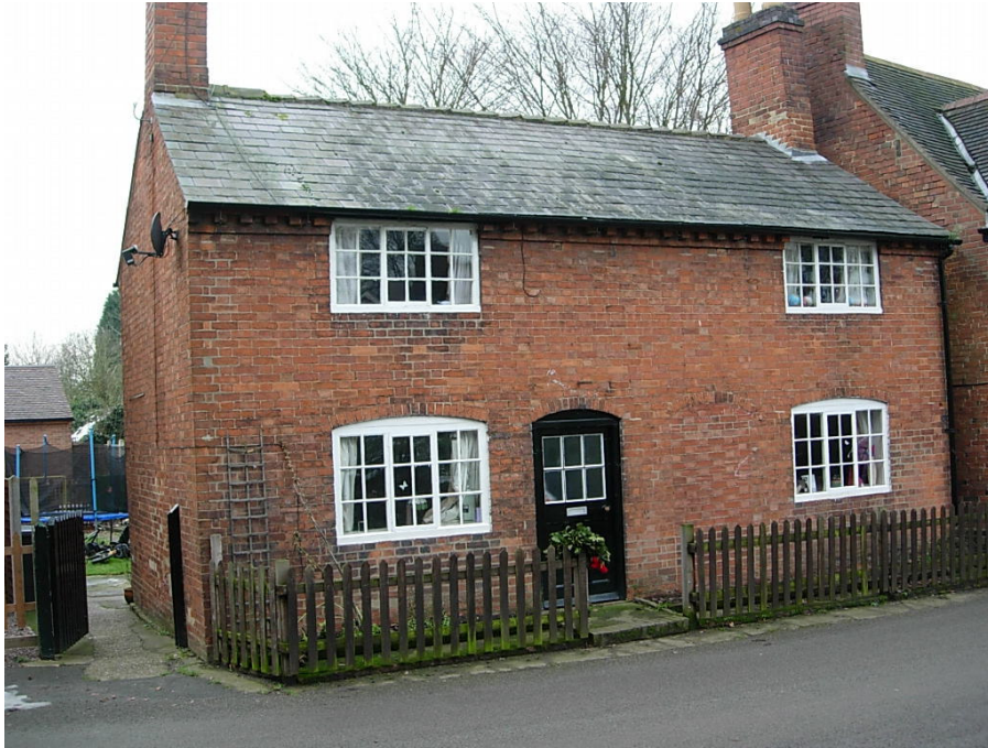
67 Church Road, a quaint cottage that retains its traditional character
