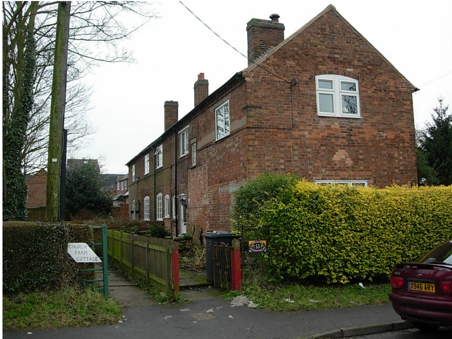
The traditional farm cottage 53 Congerstone Lane has been spoilt with the installation of UVPC windows which should be replaced with timber windows.
