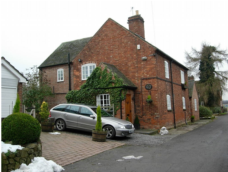
The property Cartwheel Cottage is a typical two storey core building on allotment Lane sited on the back edge of the footpath
