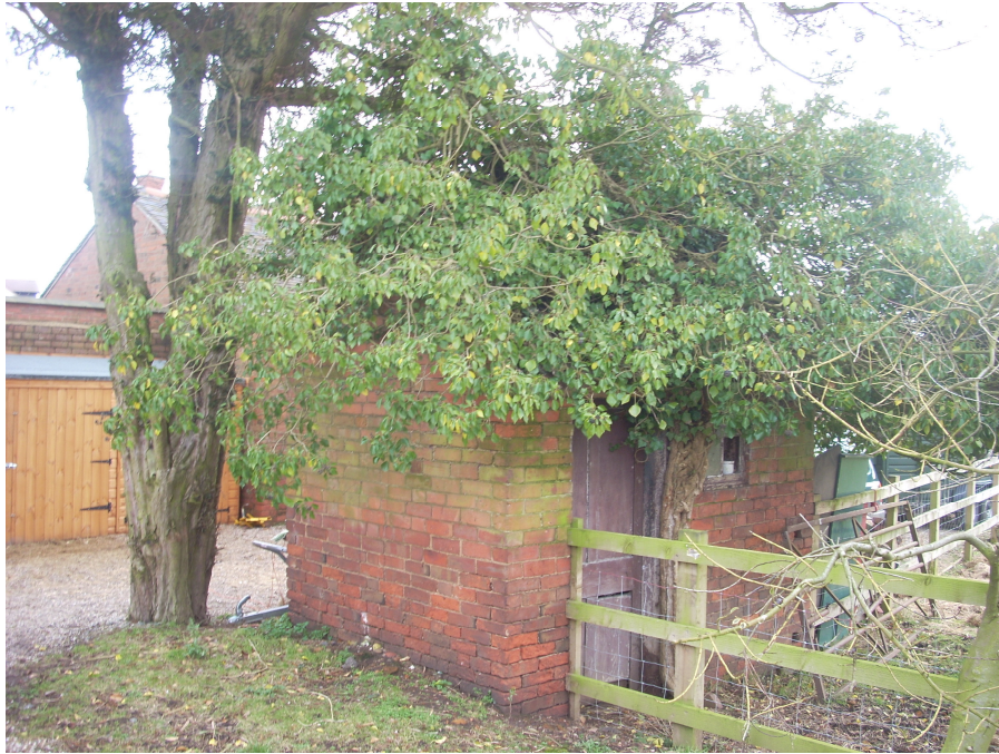
The three hole privy at the former Arnolds Farm is an important historic feature in need of repair
