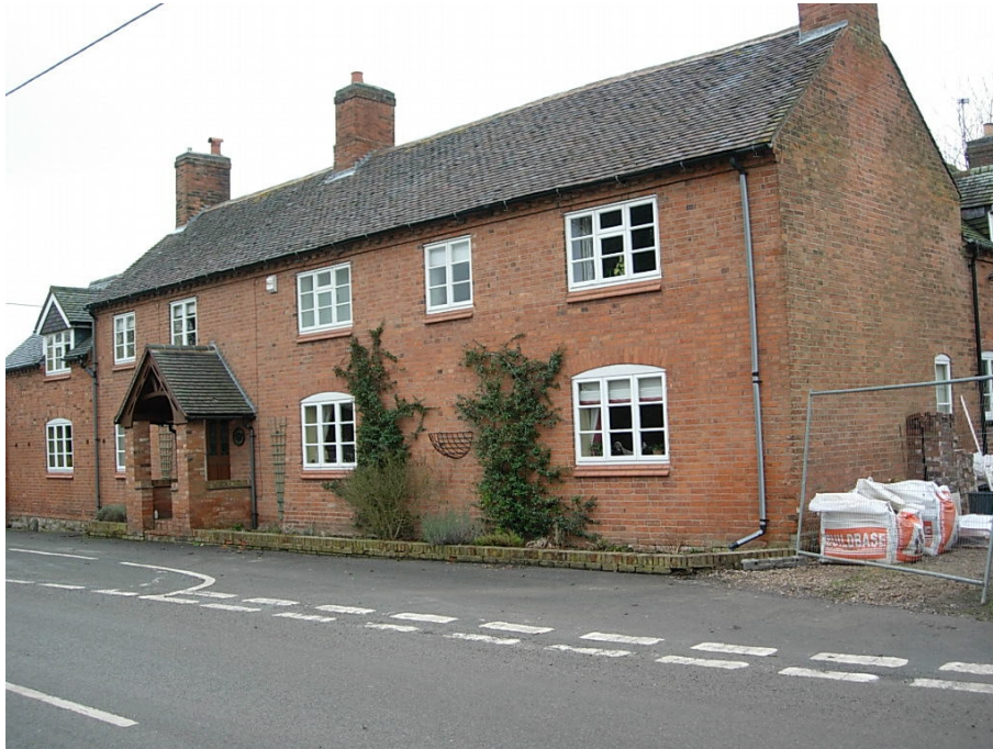
Cattows Farm Cottage sited at the junction of Insley's Lane and Main Street. It has retained its traditional appearance with the exception of the dormer
