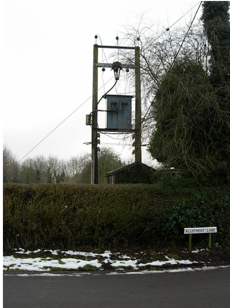
This overhead transformer is an unsightly feature at the entrance to Allotment Lane. The overhead power cables throughout the village have a negative impact on the conservation area. To underground the cables, however, will be costly
