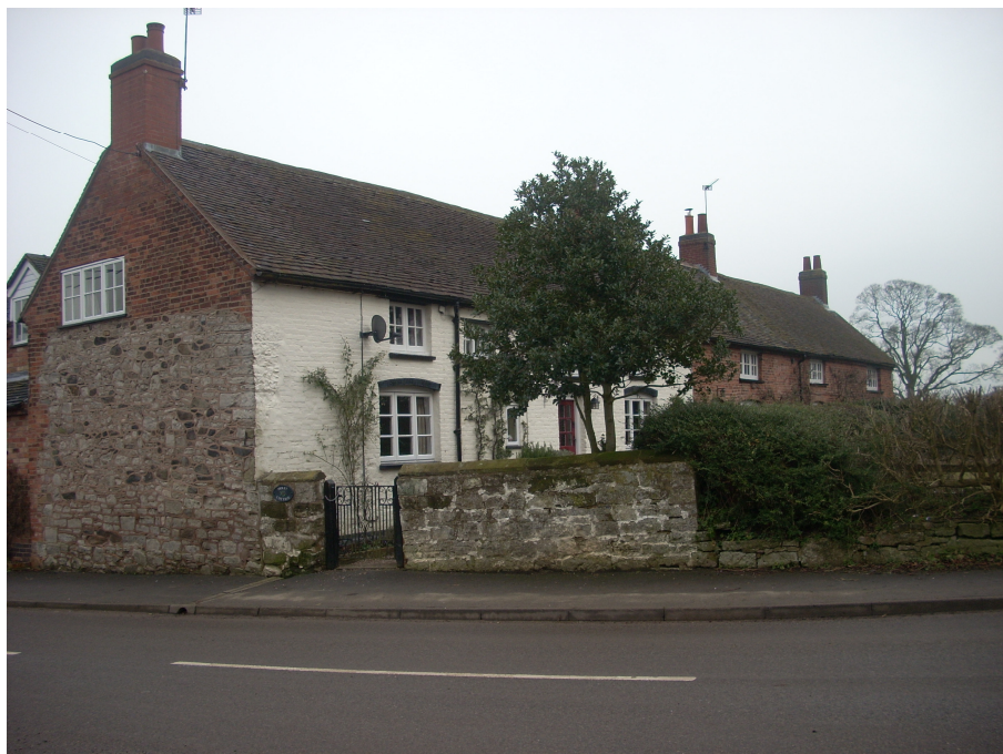
Post Office Terrace sited side on to Main Street is unusual in having most of its gable end and boundary wall built in stone
