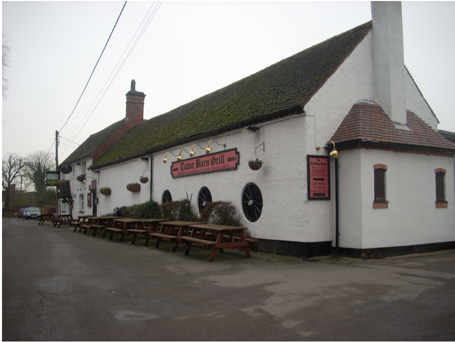
The Rising Sun pub on Church Road was probably a farm dwelling when it was originally built. The plastic windows should be replaced with timber windows
