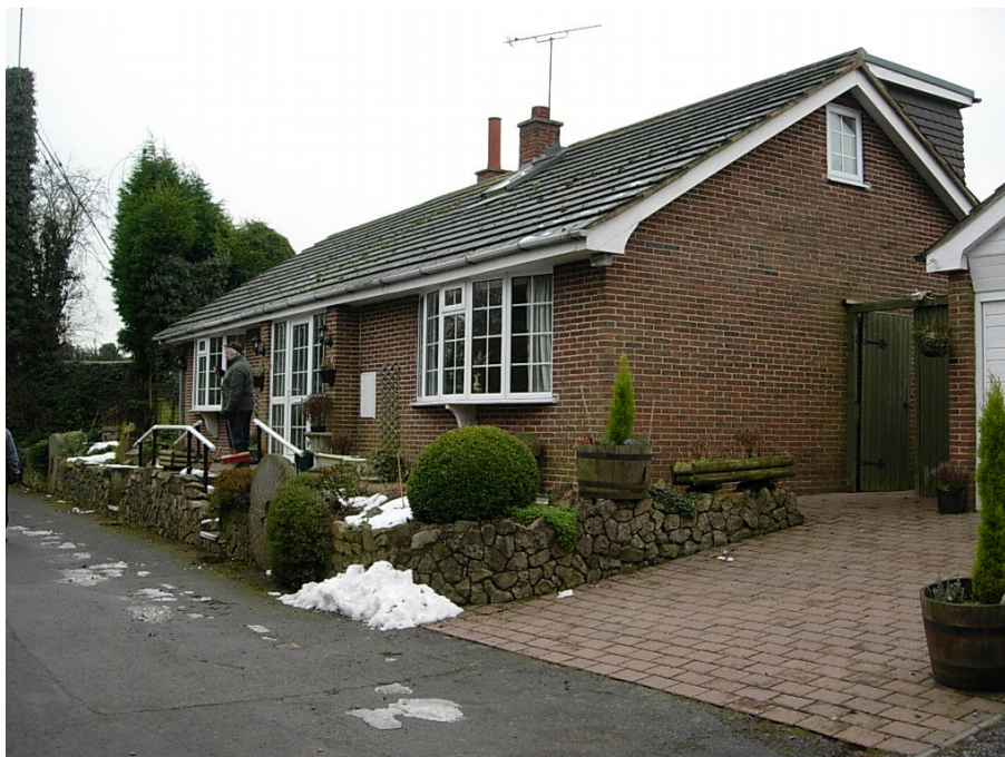
This modern bungalow on Allotment Lane is out of character with the traditional buildings in Shackerstone by way of being single storey, its design and choice of materials
