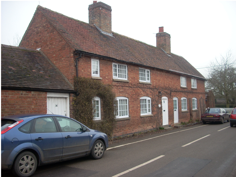
The properties 31 & 36 Main Street have lost some of their traditional character with the unsympathetic use of UPVC windows and doors
