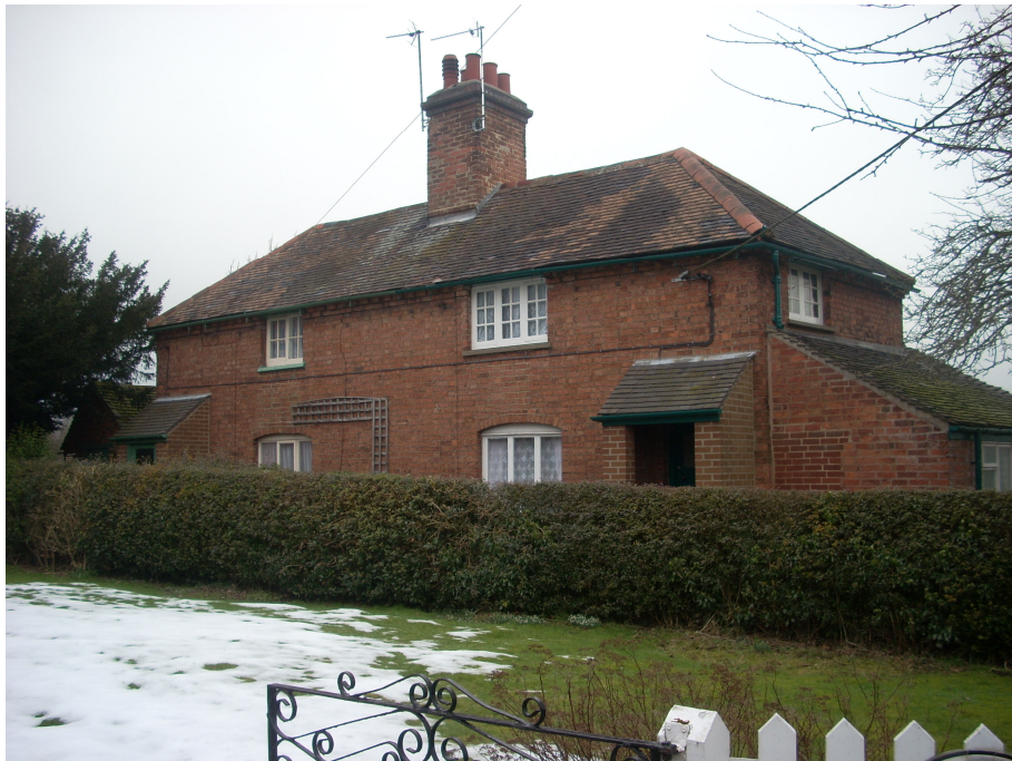
Oaklands Farm Cottages on Main Street still retain their chimney stacks. The hipped roof is not a traditional in the conservation area
