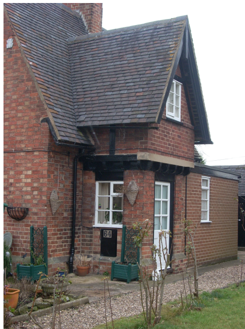
The property 64 Church Walk has some excellent detailing on its side elevation. The flat roof extension to the rear is, however, unsympathetic to the character of the dwelling.
