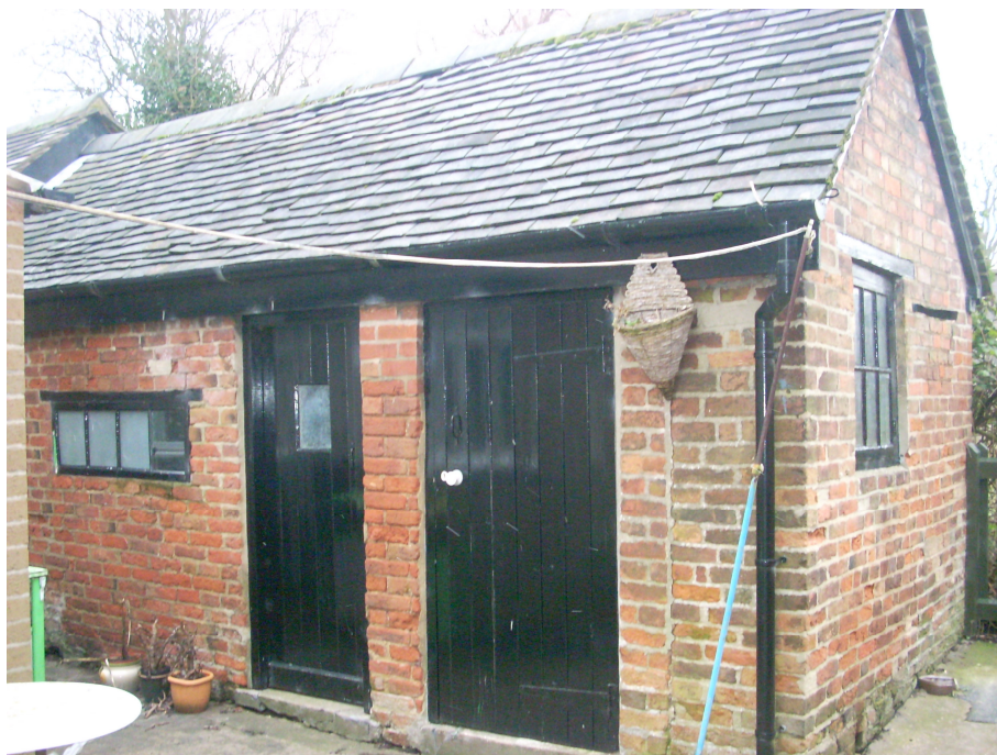
The former estate dwellings originally had their own outhouses for washing and storage. They are important features which should be retained.
