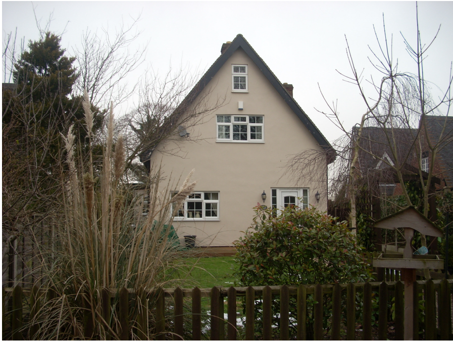
Although Rose Cottage on Church Walk has a steep pitched roof, the dwelling is generally out of character with the rest of properties on the walk by way its rendering, use of UPVC windows and design. Any new dwellings built in Shackerstone should respect the traditional character of the settlement.
