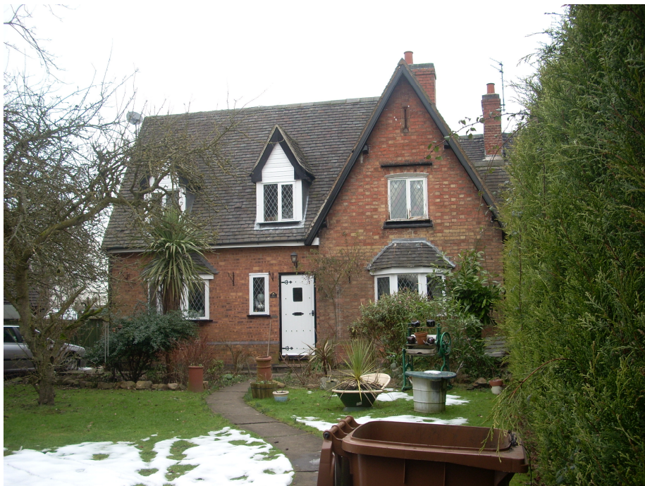
57 Church Walk built in the Arts & Crafts style. Unfortunately, the white painted door and dormers are too visually prominent and the window openings appear to have been modified without retention of any of its original detailing.
