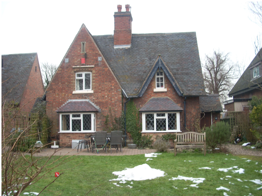
61 Church Walk is a fine example of a Gopsall Estate workers property, the traditional character of which has been spoilt due to its inappropriate bays and windows
