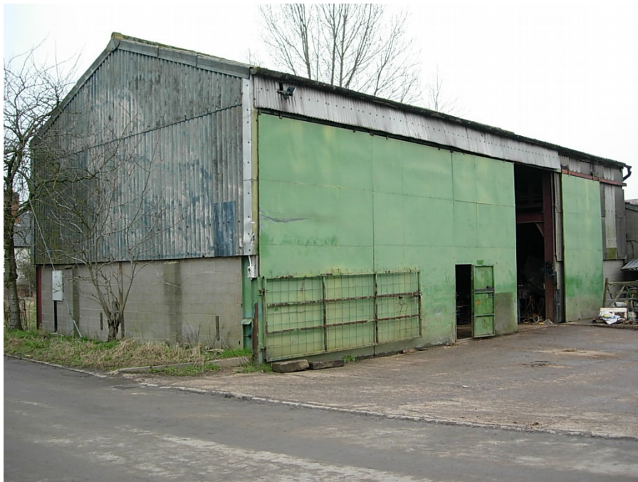
The corrugated iron barn at Wharf Farm still shows Shackerstone's rural links with the past
