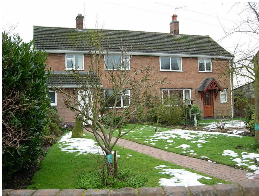
The dwellings 3 & 4 Council Houses is one of three blocks of semi detached houses on Church Road. The dwellings are of modern materials and design which are out of character with the traditional buildings in the settlement. Fortunately, several dwellings are still fronted by traditional brick walls.
