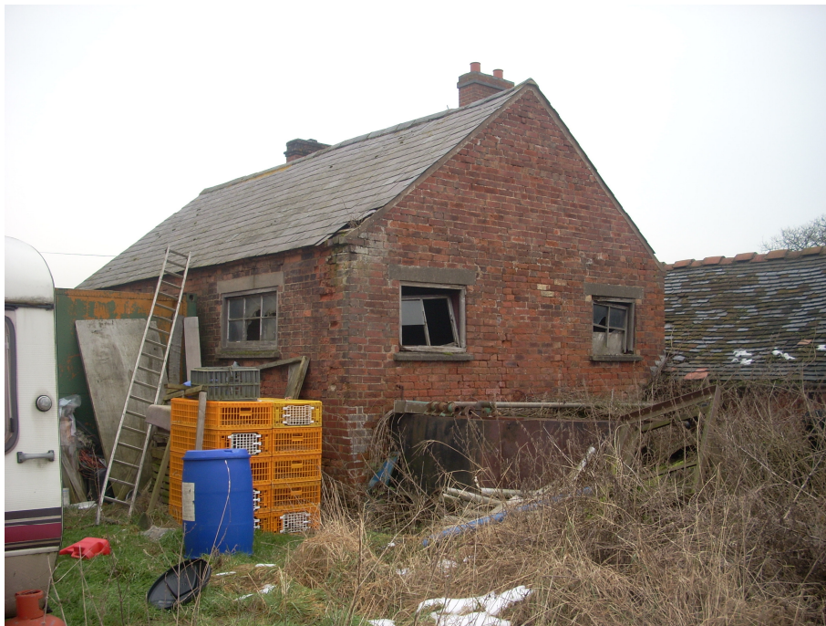
This derelict building to the rear of Bridge Farm Cottage was once the village bakery. Every effort should be made to retain this vernacular building
