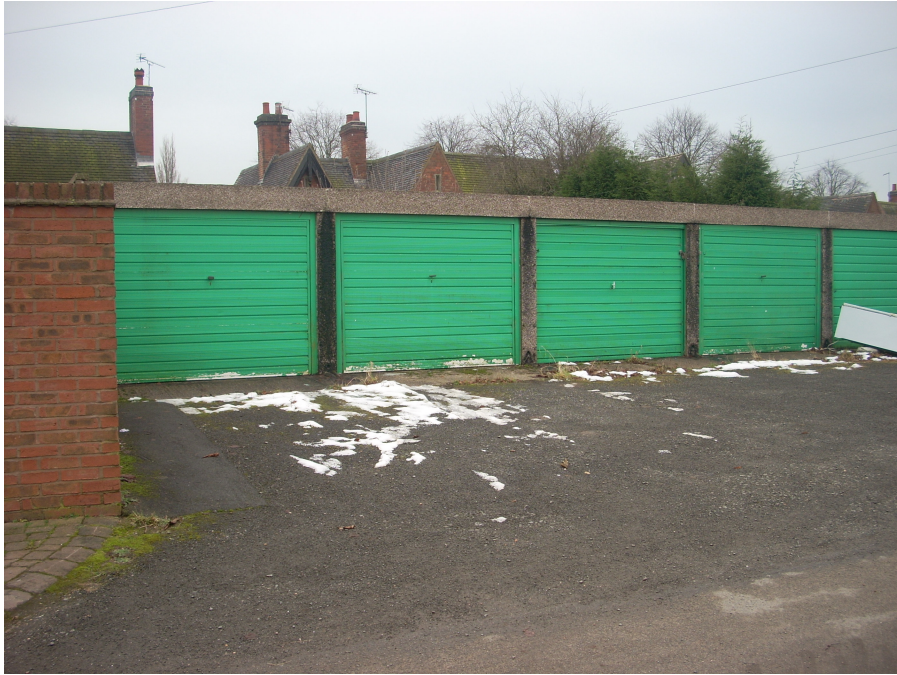
The block of garages and large area of tarmacadam on Station are a poor visual feature and should be replaced with a more appropriate structure.
