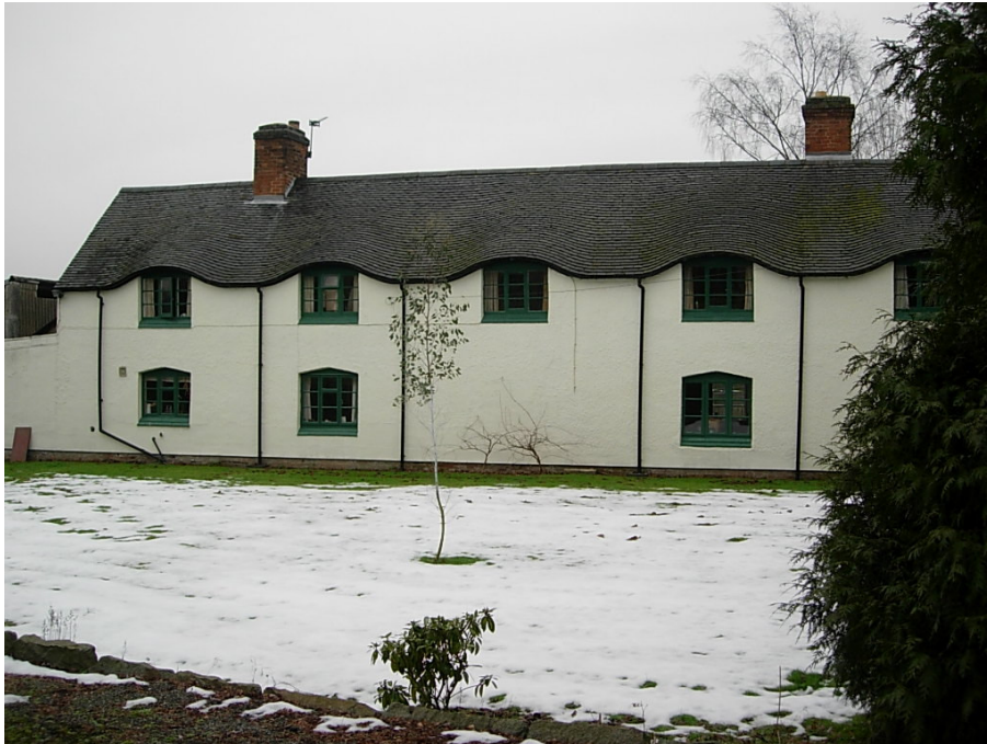
The side elevation of Wharf Farm on Station Road has subsequently been rendered which detracts from its original appearance.
