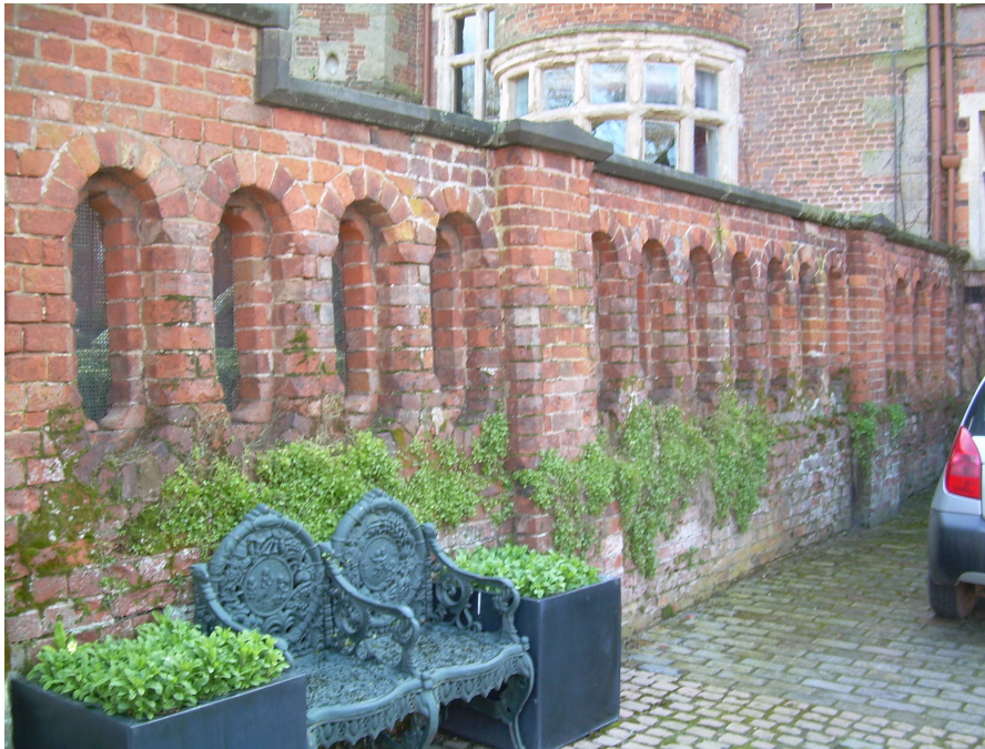
One of the fine decorative walls at Shenton Hall
