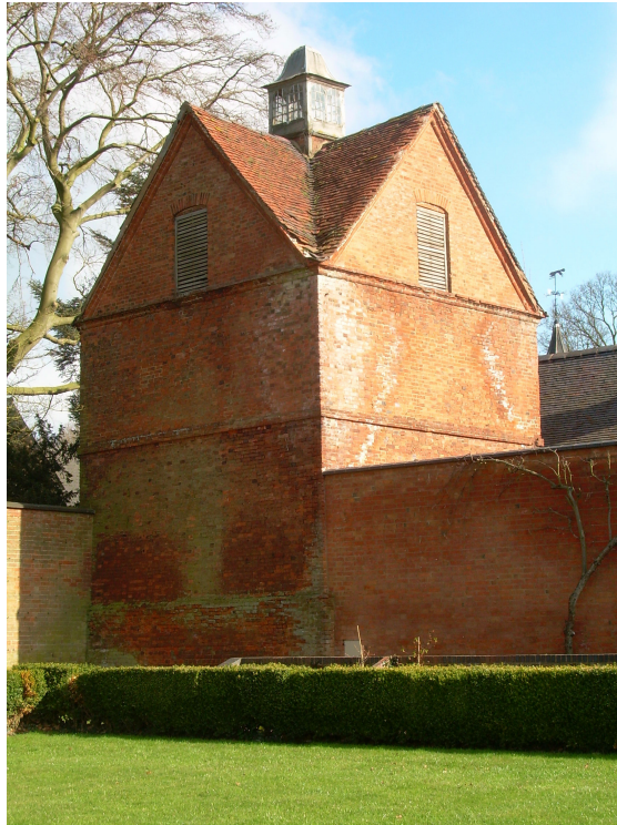
The listed Dovecote at Shenton Hall dated 1719 has benefited from recent conservation repairs.
