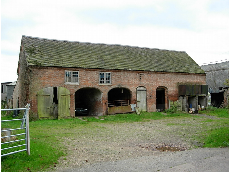
The mid 19 th century cart shed with loft above situated to the rear of Fomer Farm is a Grade 2 listed building built in the ‘Shenton Estate’ style.
