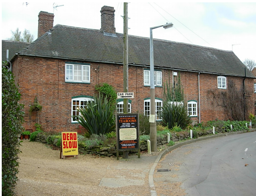
The listed White Moors located at the bend on Mill Lane has been converted into an arts and craft centre. The notices, telegraph pole and light column add to the clutter fronting the property. The UPVC windows at 1 st floor level should be replaced with timber windows to help retain the traditional character.
