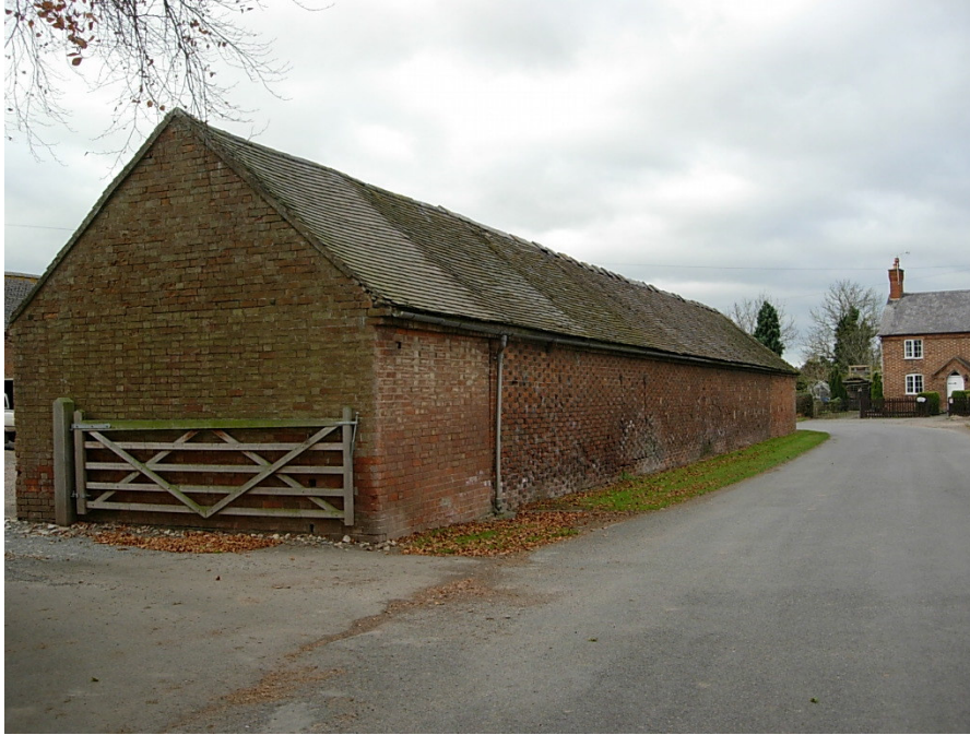
Another view of the Stud Farm cattle barn showing diaper brickwork on its north-eastern elevation. 'The Poplars' can be seen in the distance closing views up Sibson Lane towards the start of the bend.
