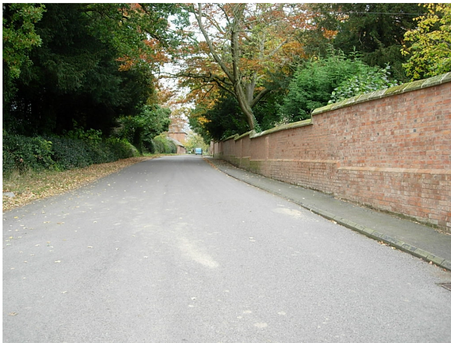
View looking north eastwards up Bosworth Road showing the boundary wall to Shenton Hall which has recently been repaired.
