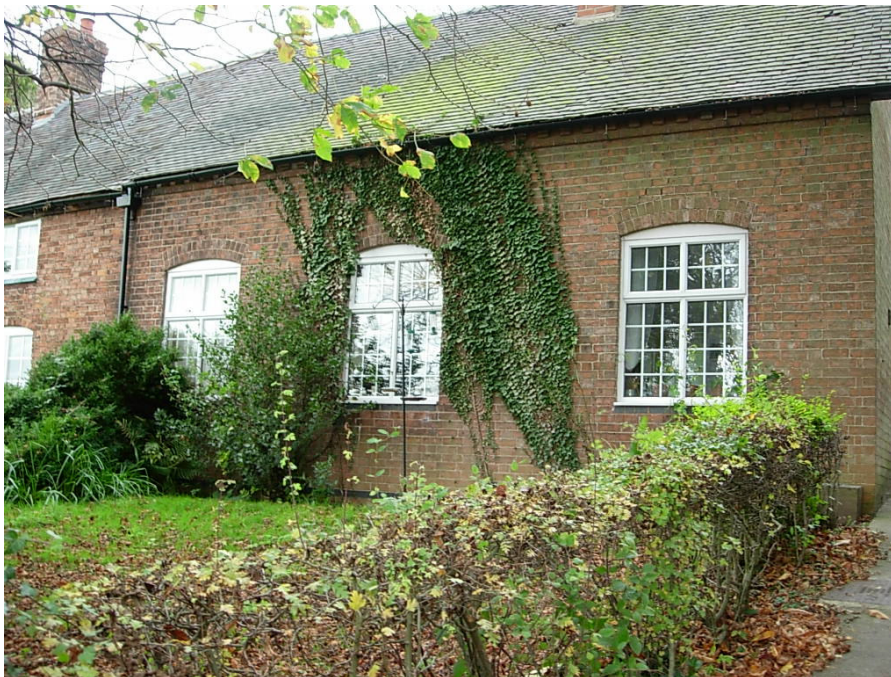
Number 7 Pump Lane is a single storey property attached to a two storey dwelling. The plastic windows detract from its appearance.
