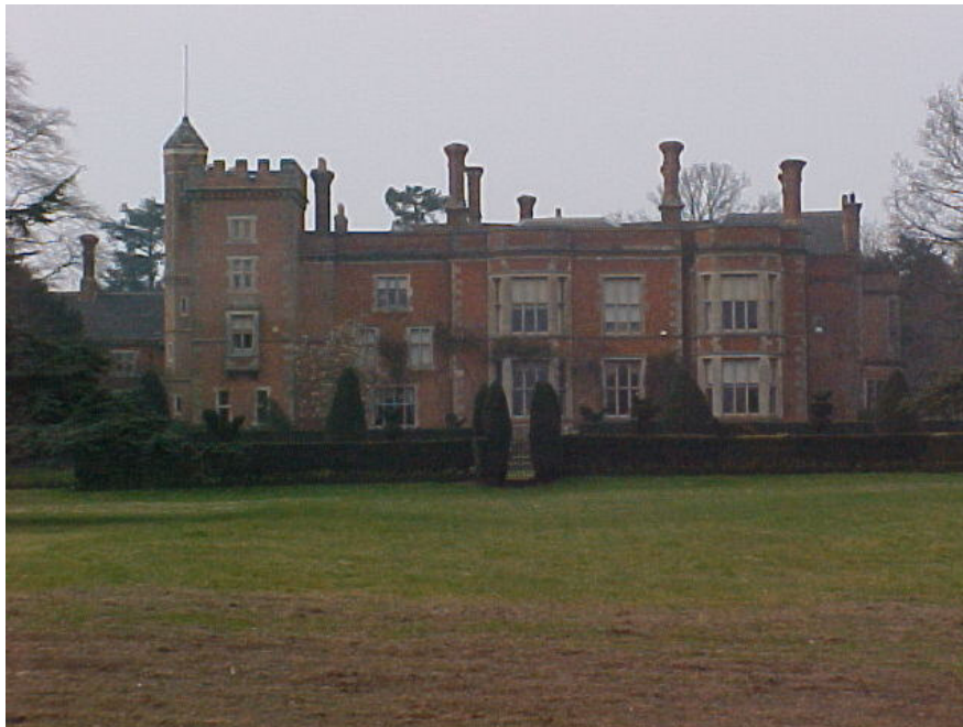
South eastern elevation of Shenton Hall. Although building work started in the 1620's, the Hall had doubled in size by the mid 19 th century. The property is listed Grade 2* built in brick with stone dressings and plain tiled roof.
