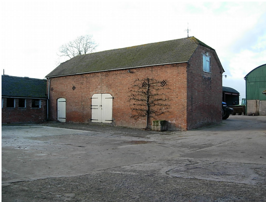
Traditional barn at Top House Farm built with a dental eaves course and tiled roof. A horse mounting block fronts the building.
