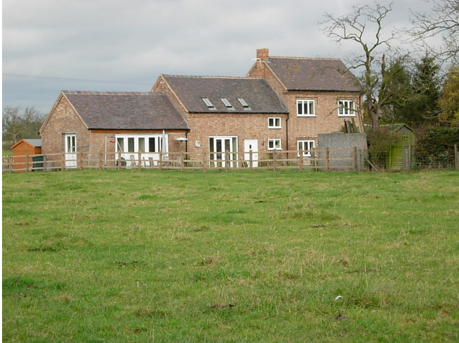
View of Brookfield Barn from Sibson Road. The use of white paint makes the windows particularly prominent when viewed from a distance. Dark brown or green is more appropriate on barn conversions.
