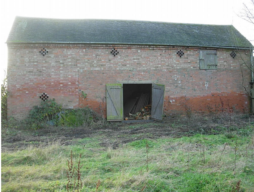
This fine barn on Mill Lane is suffering from poor maintenance.
