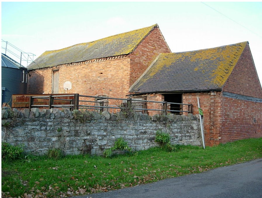
These fine barns at Aqueduct Farm are important buildings in the conservation area which need to be retained
