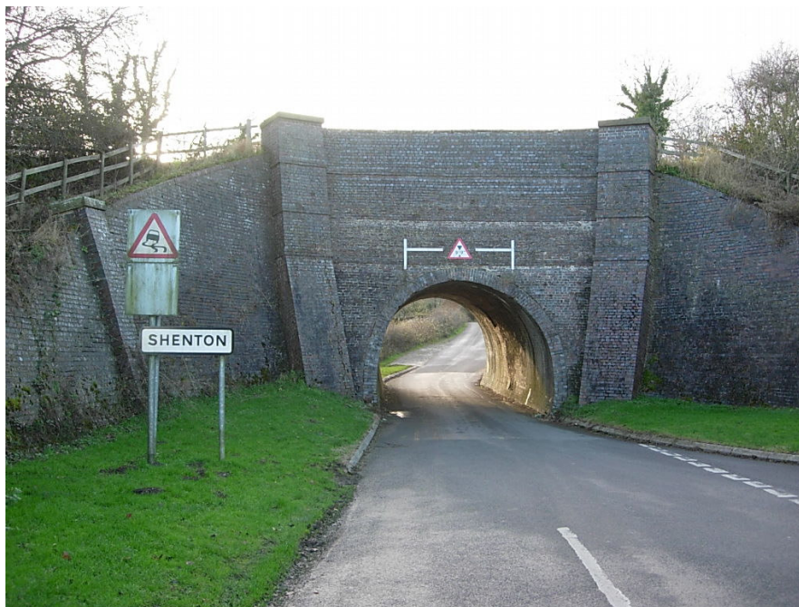
Entrance into Shenton along Bosworth Road is obtain through the narrow archway of an aqueduct on the Ashby Canal. The aqueduct is built with brindle blue bricks with covered parapets flanking the canal.
