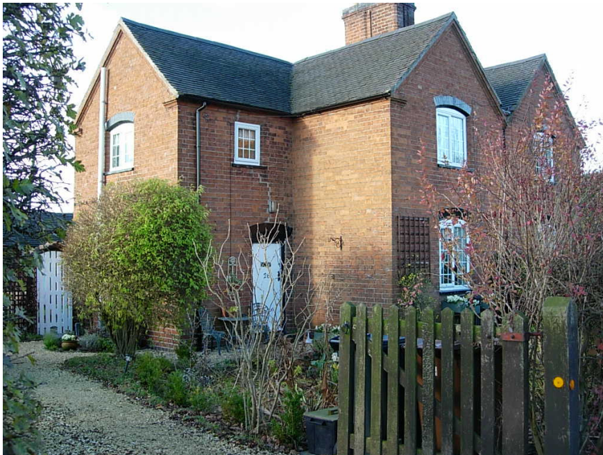
The replacement plastic windows fitted in 26 Mill Lane detract from the traditional appearance of the dwelling.
