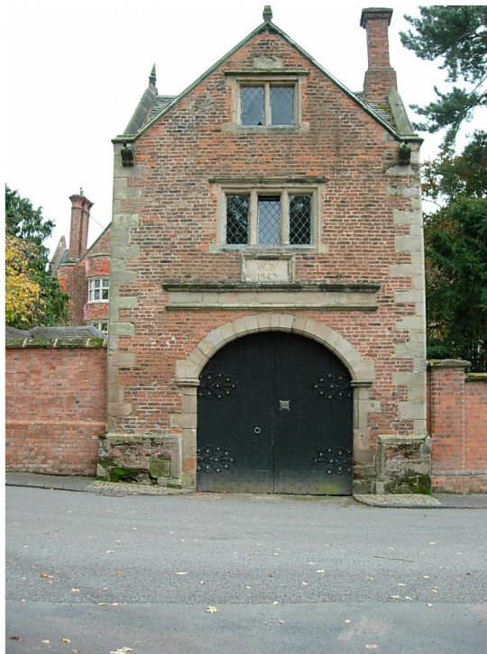
The listed gatehouse at Shenton Hall dated 1629 is an important building fronting Bosworth Road.
