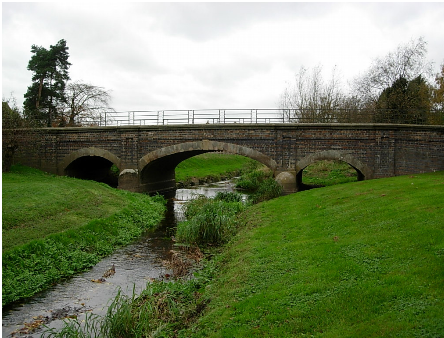
The picturesque road bridge that spans the River Tweed on Bosworth Road is flanked by low parapet walls with iron railings running along their top. The bridge and adjacent marshes are important features in the conservation area.
