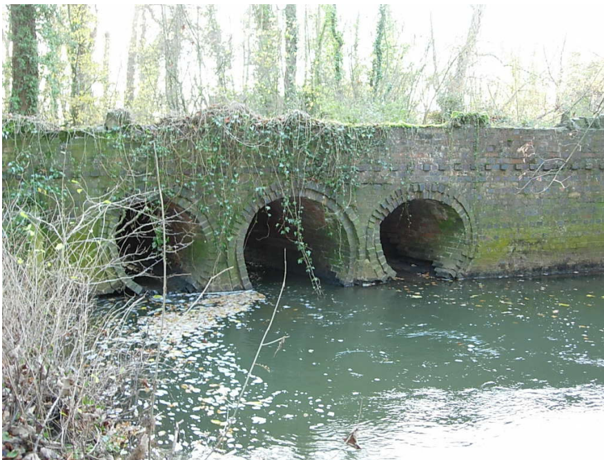
The bridge that leads to New Barn Farmhouse requires urgent maintenance. Part of the stone copings are missing and the brickwork is in need of repair.
