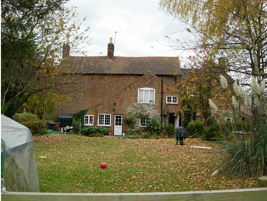
The side elevation of Ivy House Farmhouse on Main Street. The listed Farmhouse which is sited at right angles to the carriageway has had several of its windows replaced with modern plastic ones to the detriment of its traditional character.
