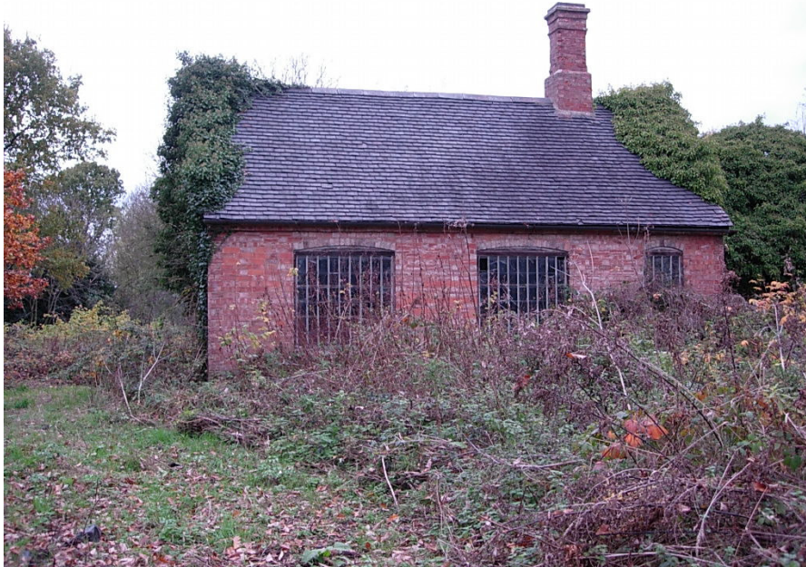
This building is situated within a small copse fronting Pump Lane. The property, now derelict, was once used as a joiner's workshop but is now in need of repair or it will be lost.
