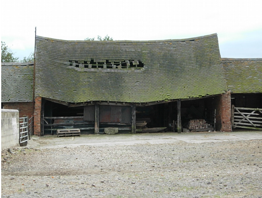
Several of the outbuildings at Stud Farm are important to the character of the conservation area but are in urgent need of maintenance.
