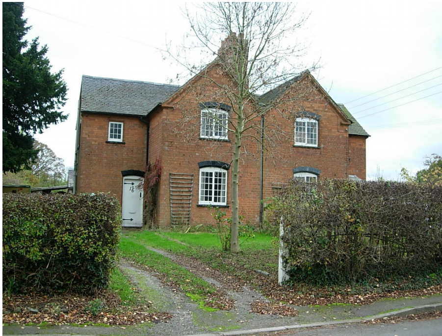
The properties 15 and 16 Sibson Road still have their original timber windows and rosemary roof tiles.
