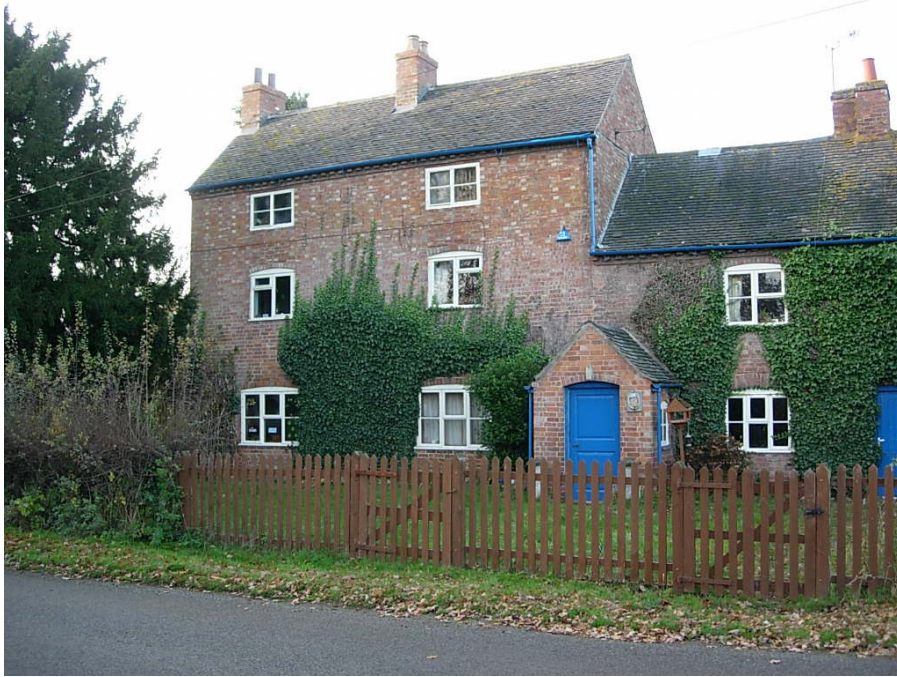
Aqueduct Farm would benefit from the re-placement of its first floor windows with traditional designed windows.
