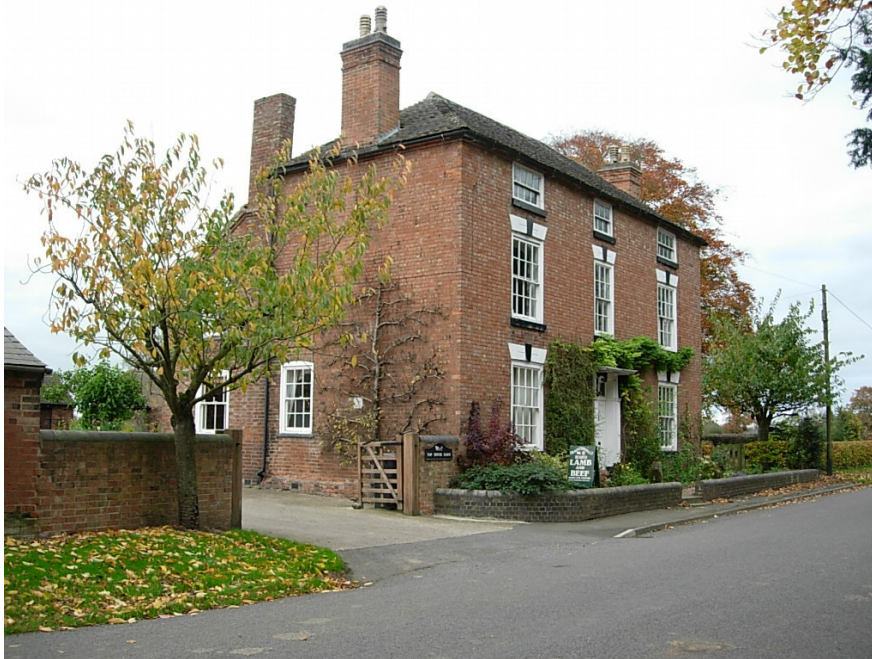
The listed early 19 th century Top House Farmhouse, built in brick with a hipped plain tiled roof. There are very few properties in the settlement that are 3 storey.
