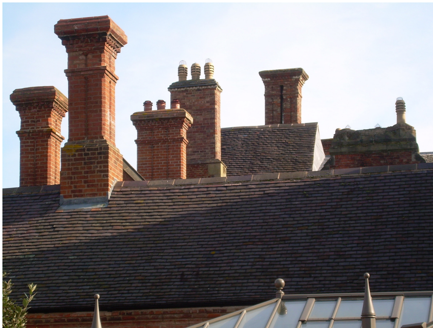
Shenton Hall showing a number of its embellished chimney stacks. These are important 'roofscape' features in the village.
