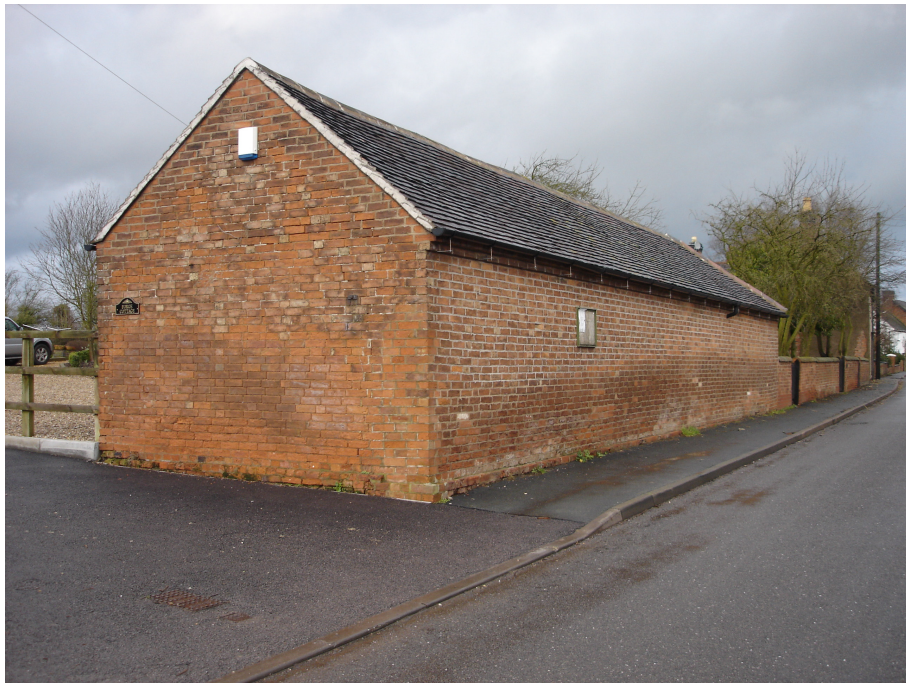
The former farm building on Main Street has been retained by successfully converting it into garages and storage accommodation. The building is one of numerous red brick buildings dispersed within the settlement.
