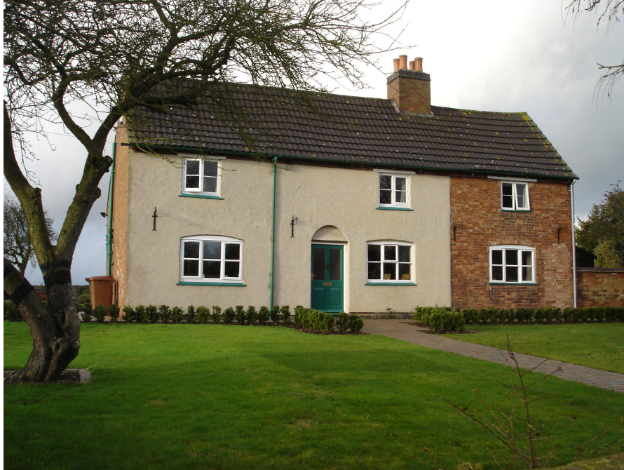
Forge Cottage, a part brick /rendered dwelling set back from the highway. The use of concrete roof tiles tend to detract from its traditional character.
