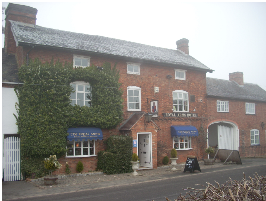
The fixed blue canopies, bow windows, signs and planting tubs fronting the pub tend to detract from the character of the conservation area.
