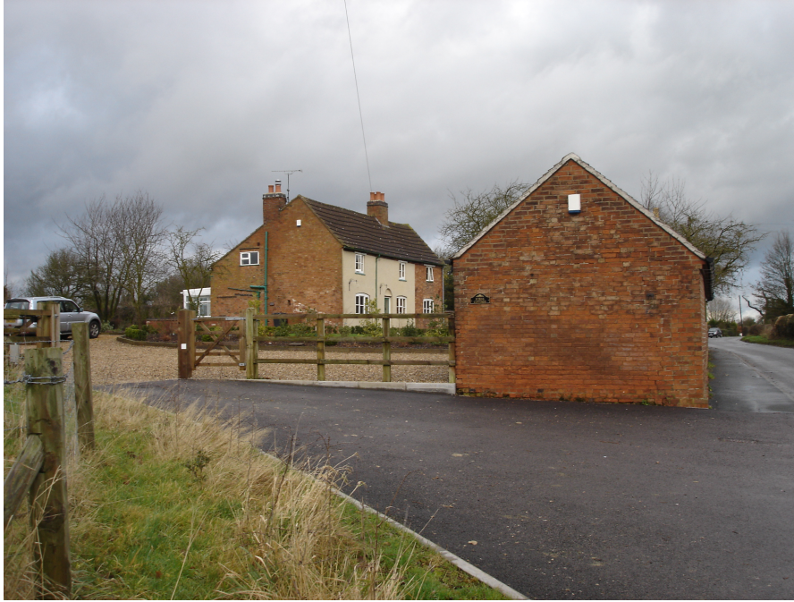
This area on Main Street has lost its enclosure and would benefit with the timber fence replaced with a traditional wall or hedge.
