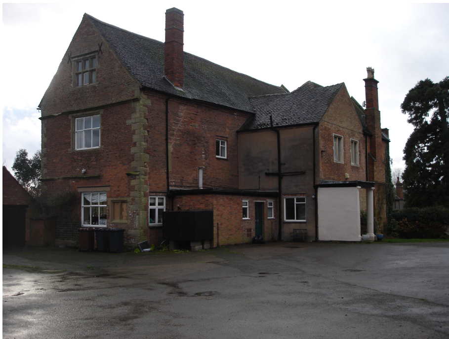
Rear of Hall Farmhouse showing stone corner dressings.
