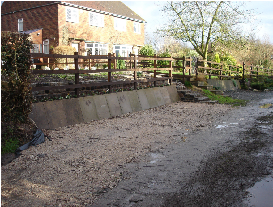
The concrete retaining slabs fronting 2 & 3 Blacksmith Lane are a poor visual feature. Consideration should be given to replacing the slabs with a wall of traditional character.
