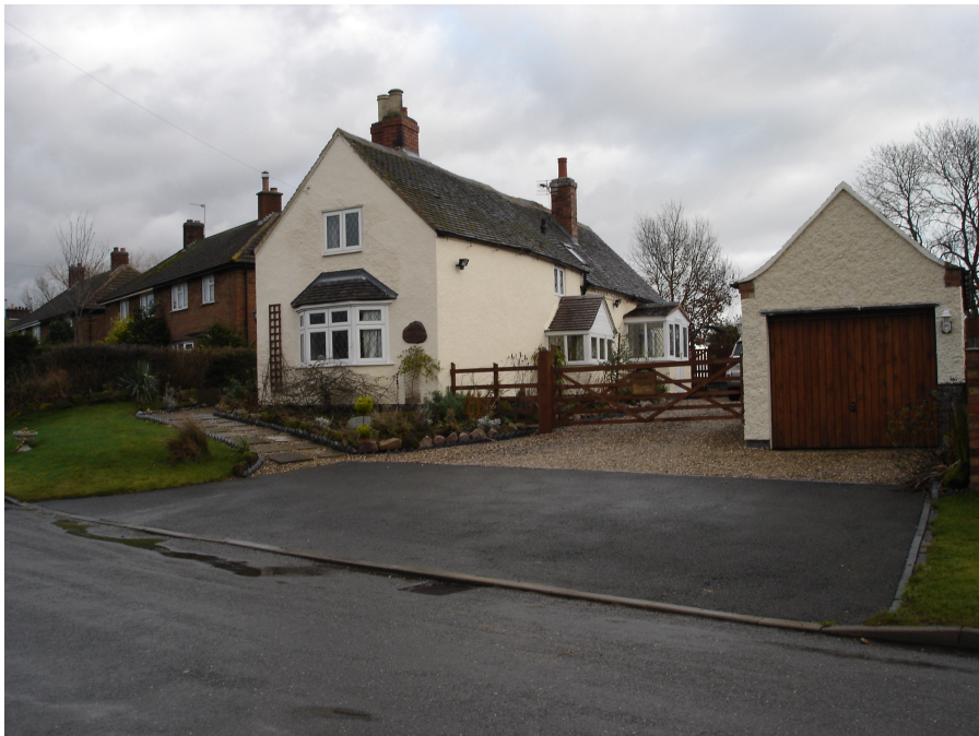
Ambion Cottage, a rendered property with a rosemary tiled roof that has had its windows modernized.
