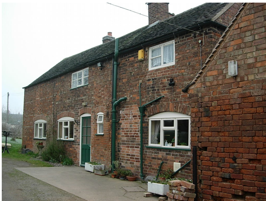
Rear of The Old Bakery showing numerous alterations that have taken place to the dwelling. The blocking up of doorways and openings with an inappropriate brick type has had a detrimental visual impact on the premises.
