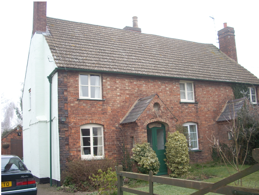
Applewine Cottage and Sunnyside Cottage sited at the end of The Square. The use of concrete roof tiles tends to spoil the character of these properties.
