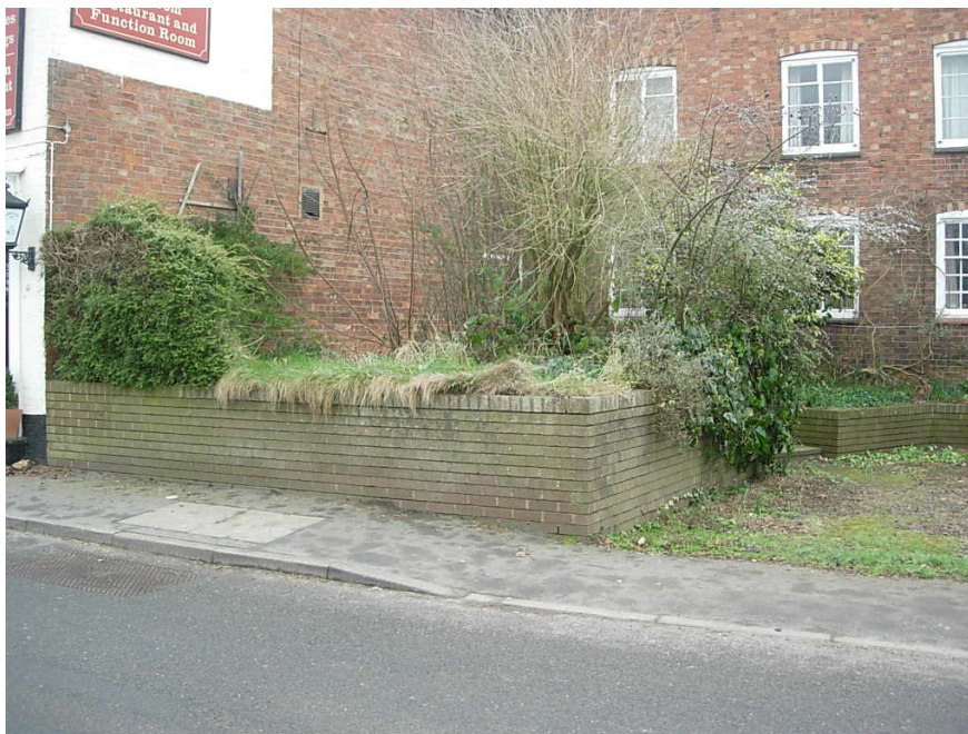
The listed grade 2 property to the south-west of the Hercules Inn has a doorway built with a round headed archway and hipped roof. The property would benefit visually if the modern brick wall was to be replaced with a traditional wall.
