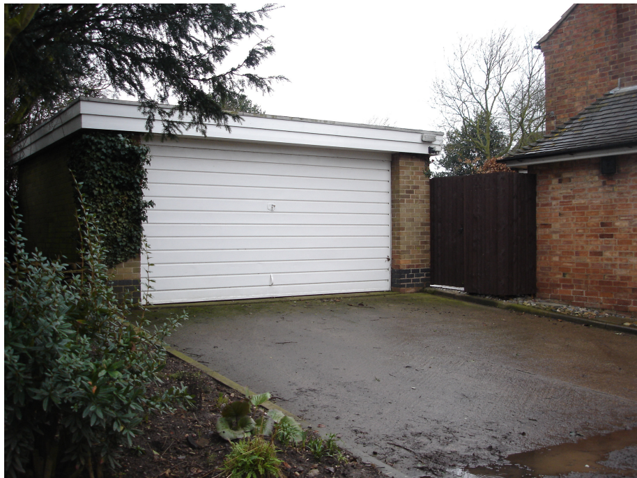
The flat roofed double garage adjacent to Keepers Lodge is unsympathetic to the traditional character of the conservation area.
