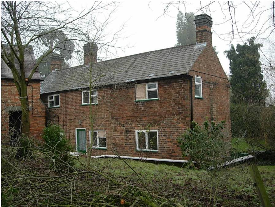
Rear elevation of The Old Post Office showing the prominence of re-constituted wall copings. The introduction of re-constituted building materials in parts of the conservation area is starting to have a negative effect on its character.
