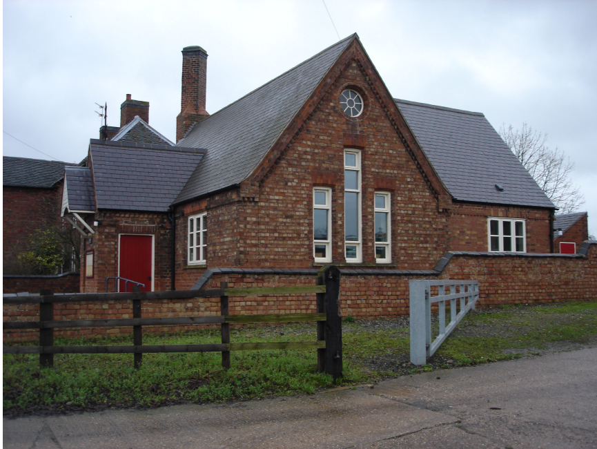
Sutton Cheney's Church Hall has a fine traditional boundary wall.
