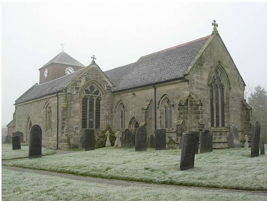
Grade 2* St James's Church principally of the early C13 but with perpendicular features. Built in limestone with some ashlar work and plain tiled roof.
