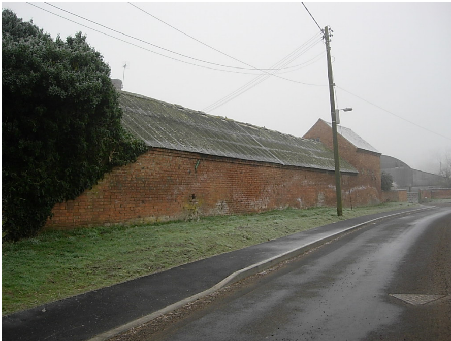
The farm buildings to Townshead Farm help channel views down Bosworth Road. Together with the grass verge there is a rural feel to the road which has been spoilt with the introduction of concrete kerbing.
