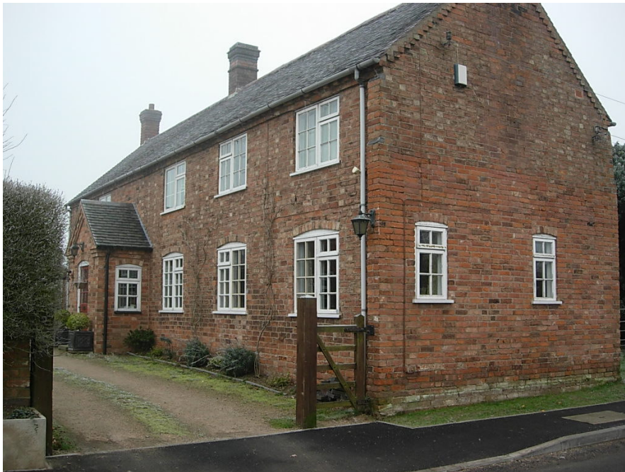
Moores Cottage that has its gable end fronting Bosworth Road has lost some of its chimney pots.
