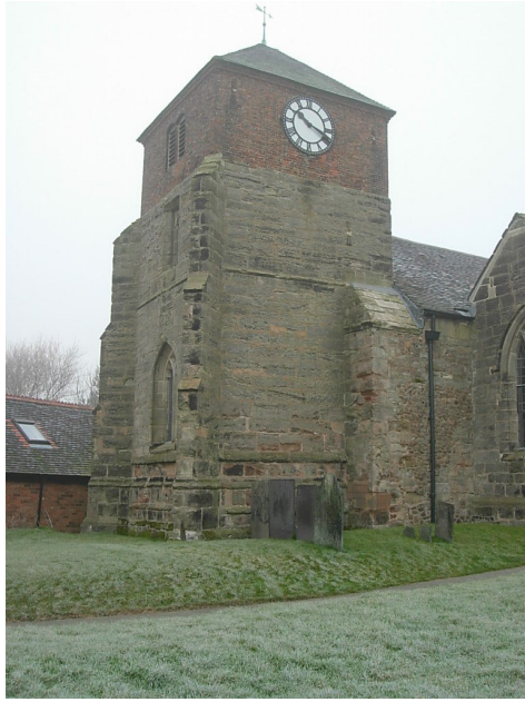
St James's Church Tower showing its angle buttresses and plinth that has been raised using bricks.
