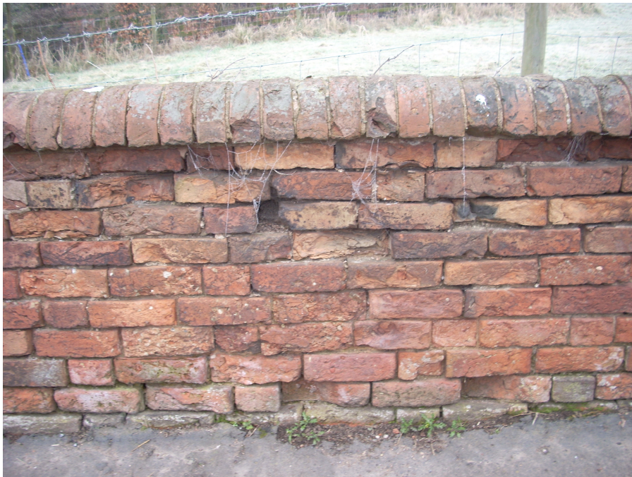
A traditional brick wall found in the Sutton Cheney Conservation Area. Built utilizing a nine inch bond with saddleback copings, the loss of these walls would have significant visual impact on the village's traditional character.
