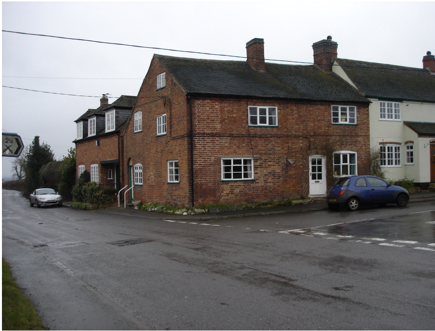
Corner Cottage at the junction of Wharf Lane and Bosworth Road.
