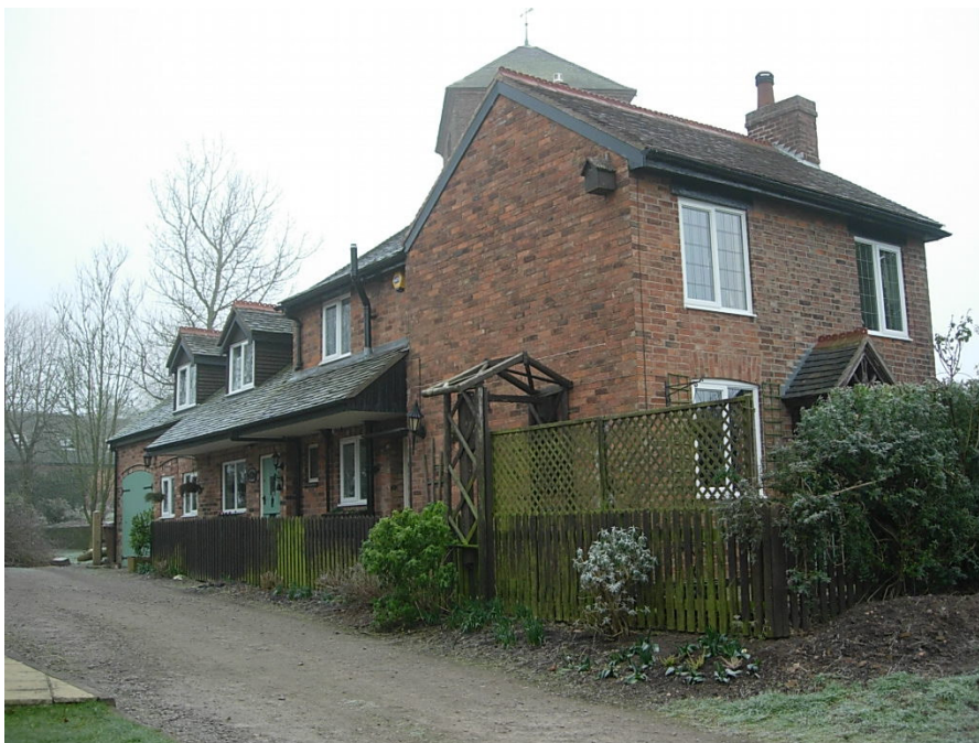
Bumblebee Cottage has been considerably modernized. The dwelling is one of few properties in the village that has barge boarding. With the introduction of plastic windows, roof lights, canopy and satellite dish, it provides a poor setting to the parish church.
