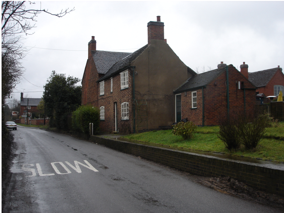
Field View is at the southern entrance of the conservation area on Wharf Lane. Enclosure has been lost due to the open nature of the garden. Some form of enclosure is needed, preferable with the building a traditional brick wall.
