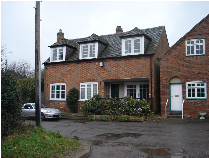
The Old Chapel on Wharf Lane has had improvements made to it. The dormers on the front elevation are out of scale with the property.
