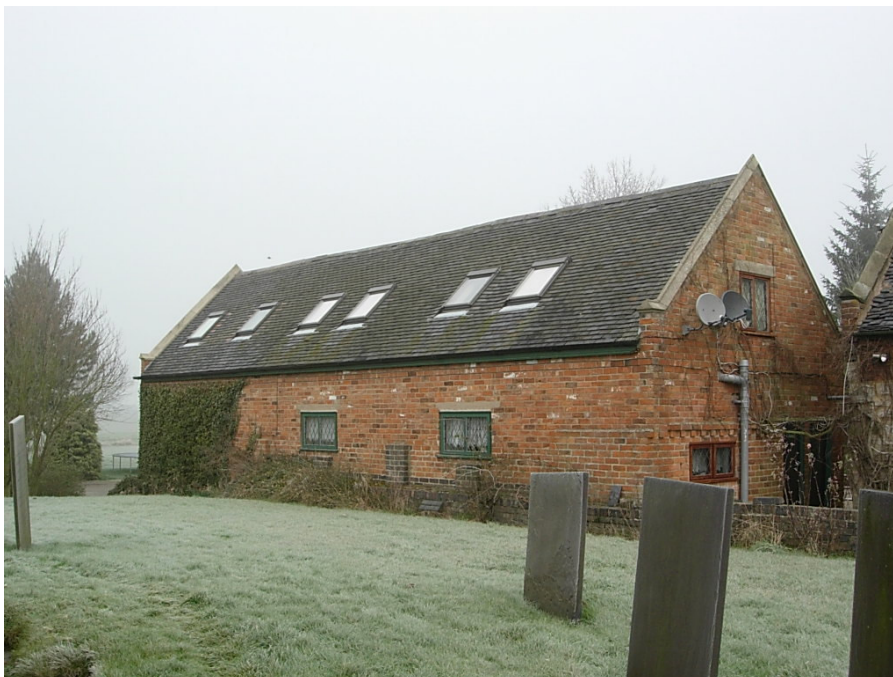
The side elevation of Sutton House viewed from the parish churchyard. The roof lights, concrete lintols to the windows and satellite dish are unsympathetic features adjacent to the historic church and alms house.
