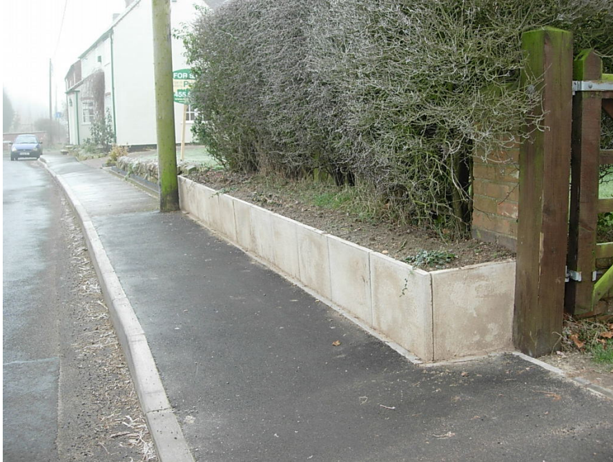
The concrete retaining slabs on Bosworth Road are a poor visual feature which should be replaced by a brick wall.
