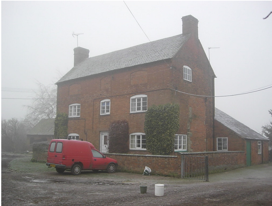
Townshead Farmhouse, a Grade 2 listed building built early C19 that has some limestone visible in the gable wall suggesting a possible earlier core. The dwelling is three storey with blind lights to the attic.
