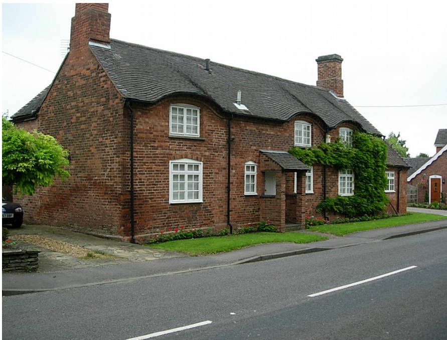
7 Church Street has also been converted into one cottage which has resulted in the loss of one of its original doors and chimney pots.
