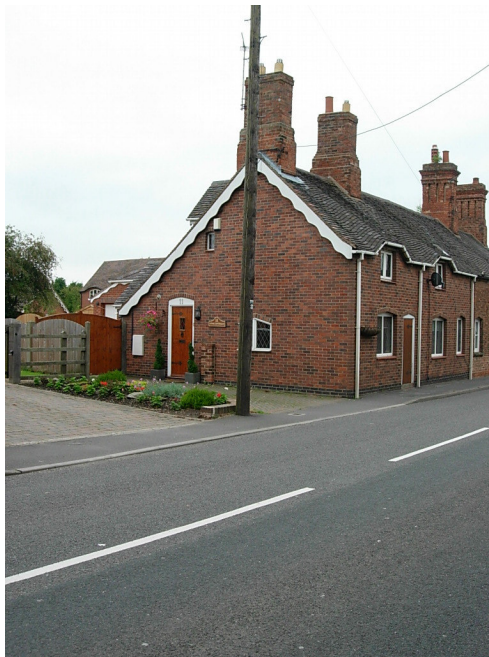
The barge boarding on the gable end of 11 Church Street is prominent incongruous feature on Church Street.
