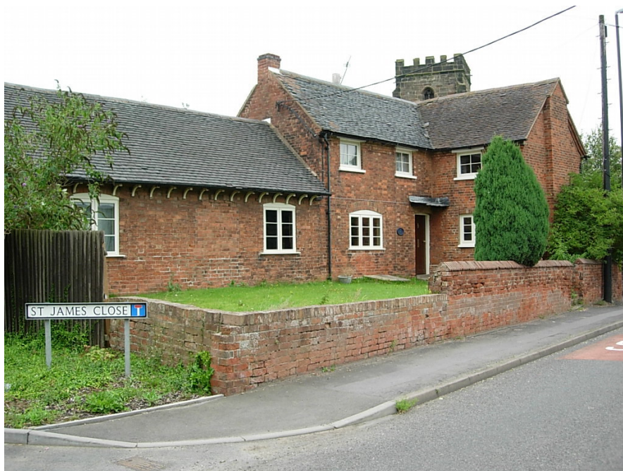
19 Church Street is an attractive dwelling which generally retains its rustic charm although it would benefit from a traditional saddleback coping running over the whole length of its boundary wall and having the chimney stack replaced on its gable end.
