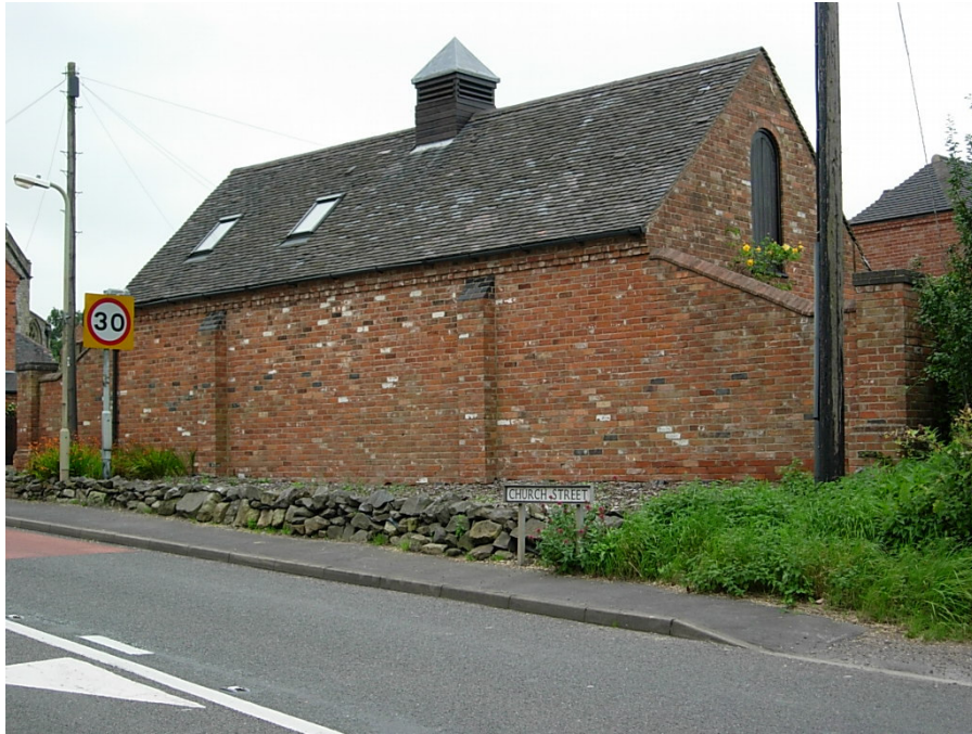
This existing building has been converted into garages/store. The roof lights on the front elevation should have been restricted to the rear elevation only
