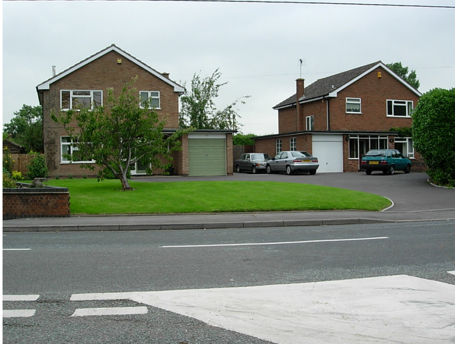
The two modern dwellings 4-6 Main Road are out of character with the traditional 'core' buildings in the conservation area. Enclosure is also lost with their open aspect fronting the carriageway. Consideration should be given to the building of a brick wall of traditional materials and brick bond.
