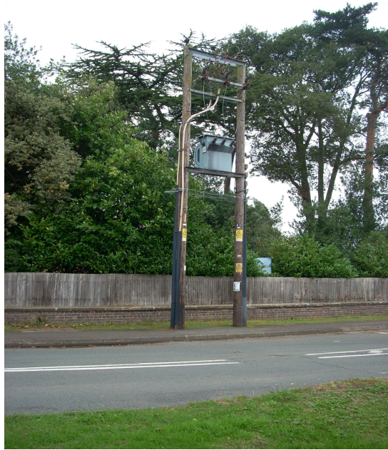
The pole transformer on Main Road is an incongruent feature that needs to be removed and the overhead electric cables in the conservation area undergrounded.
