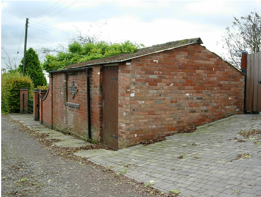
Significant changes to this small Victorian outbuilding on Flax Lane has had a detrimental impact on its character. The pitch of the roof has been reduced and the roofing material changed from its original.
