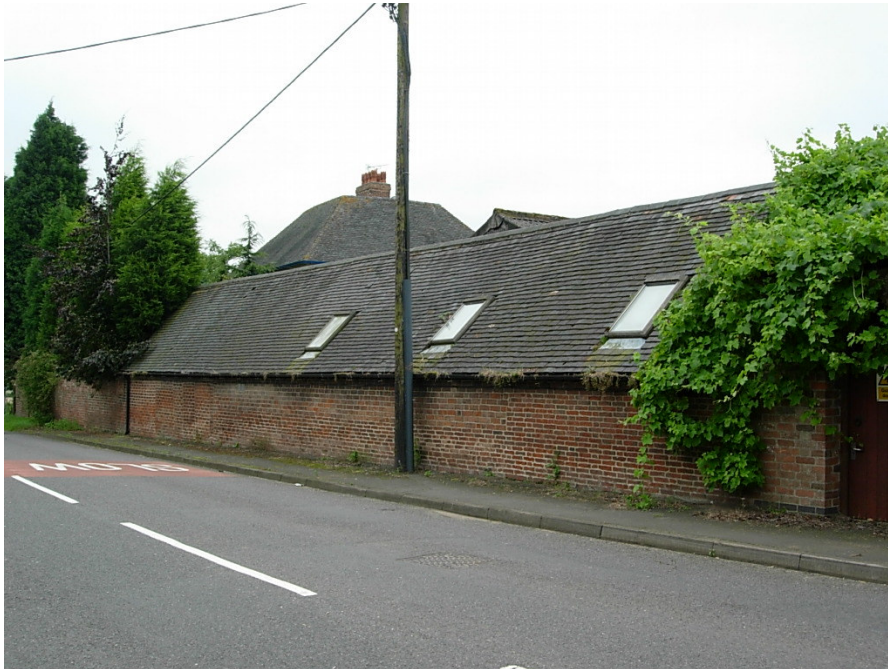
The single storey building fronting Church Street is located within the curtilidge of the listed Grade 2 Manor Farmhouse. The insertion of three large roof lights detracts from its appearance and former agricultural use.
