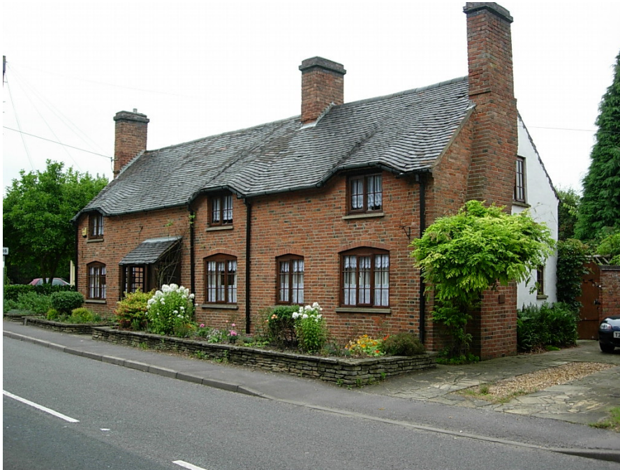
3 Church Street has been converted into one dwelling generally utilizing natural materials. Although the chimney stacks have been retained, the chimney pots are a missing element.
