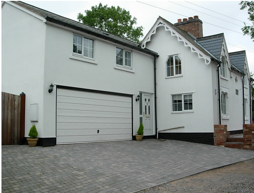
A large unsympathetic side extension / integral garage has been built at 15 Sheepy Road which is out of scale and character with its period dwelling.
