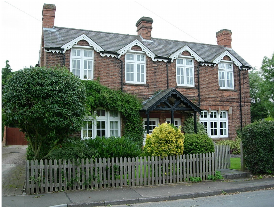
9 & 11 Sheepy Road, a pair of semi-detached dwellings showing 'gables' as features above their bedroom windows
