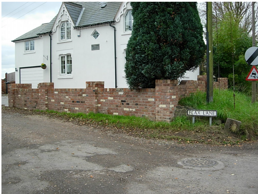
The design of this recently built wall fronting 15 Sheepy Road is out of character with other traditional boundary walls in the conservation area.
