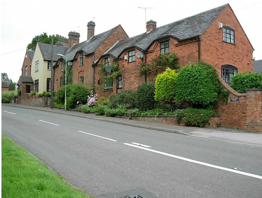
The properties situated at the entrance to the village that step up Church Street form an attractive terrace. Unfortunately, several satellite dishes mounted on their front elevation detract from its appearance.
