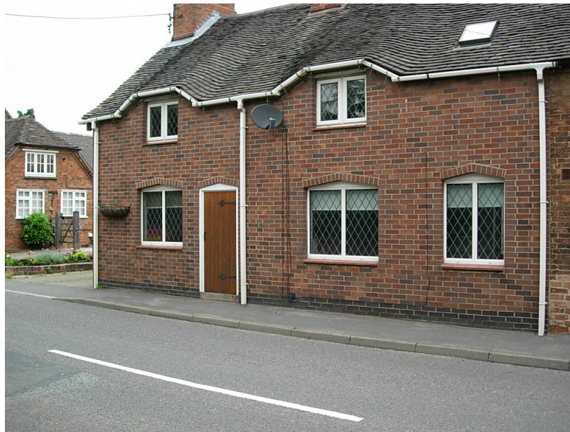
11 Church Street has been modernized utilizing; a modern brick laid stretcher bond, whiteUPVC guttering and down pipes, roof light and satellite dish mounted on the front elevation. The property is at discord with the rest of the terrace and should have been modernized utilizing natural materials and traditional building methods.
