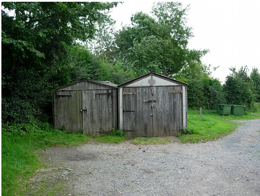
The two garages and surface dressing of the carriageway are unattractive features that tend to detract from the appearance of Flax Lane.
