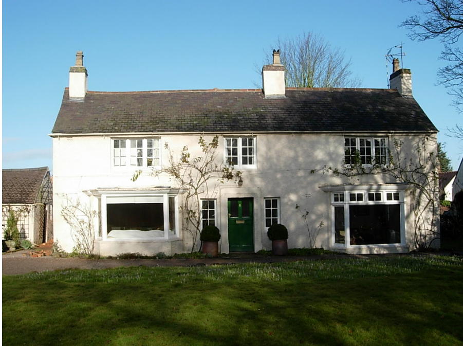
8 Cottage Lane, although not sited in the conservation area, the dwelling and mature trees sited in its large garden have a significant visual impact. The property was once used as a chapel and charitable school. The dwelling has timber windows. Its slate roof and chimney pots have recently been restored.
