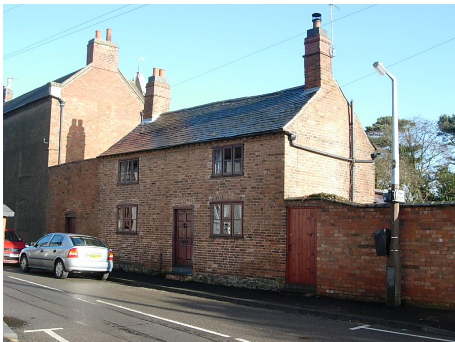
68 Main Street is a small attractive cottage with a slate roof and two fine chimneys on its gables.
