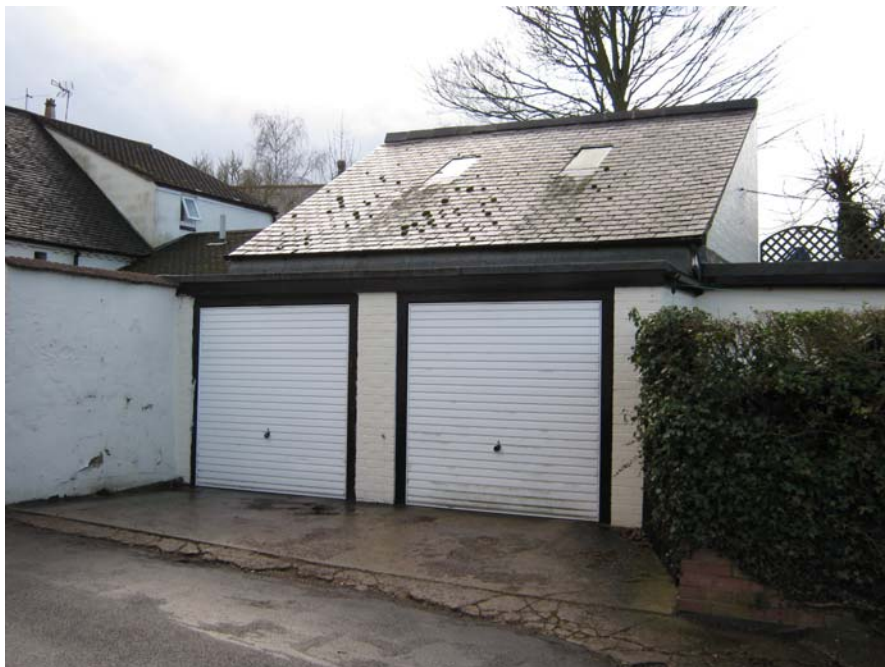
The double garage on Cottage Lane with its up and over doors does not particularly enhance the street scene.
