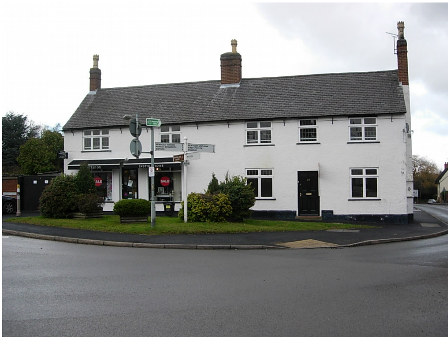
The properties 37 High Street and 2A Main Street are attractive buildings that restrict views along High Street at an important intersection.
