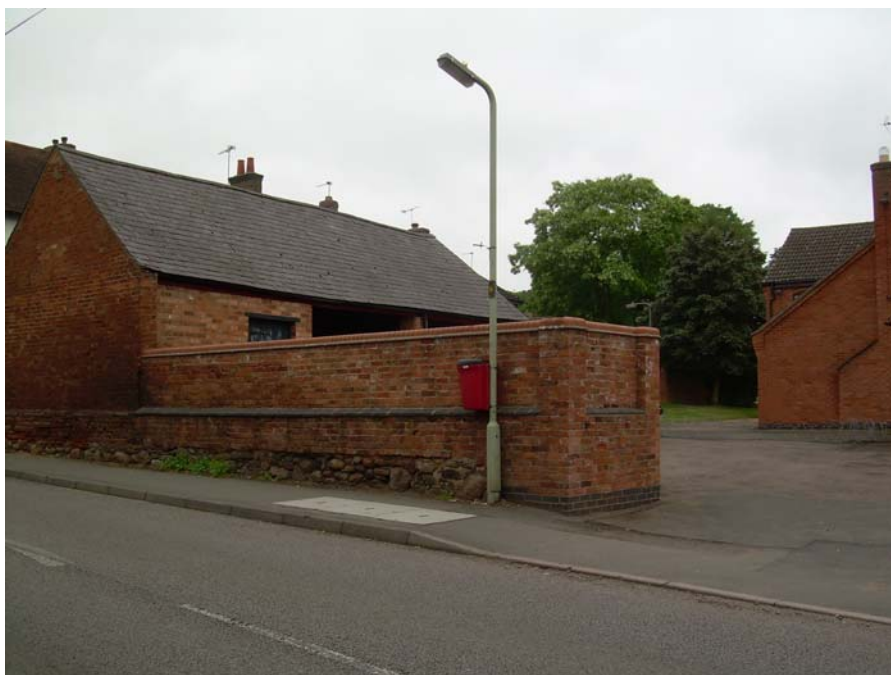
The barn, sited at the junction of Church Lane and High Street, was probably built around the same time as Old Manor Farm. It still has late mediaeval arched foundations. The building was once listed as it was sited within the curtilidge of the adjacent listed property.
