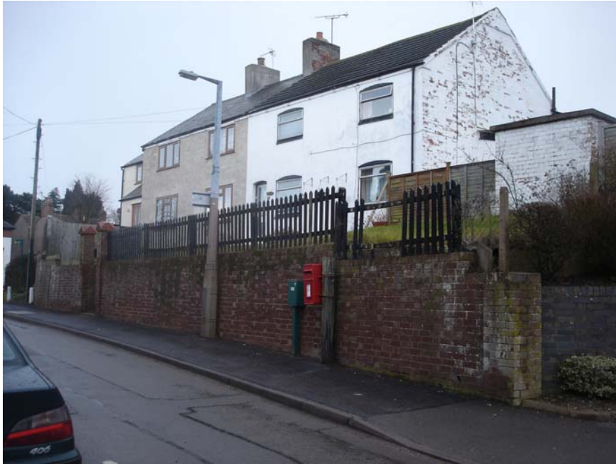
The properties 5-11 Newbold Road occupy a prominent position on the road sited behind a tall retaining wall. The terrace has been modernised to its visual detriment.
