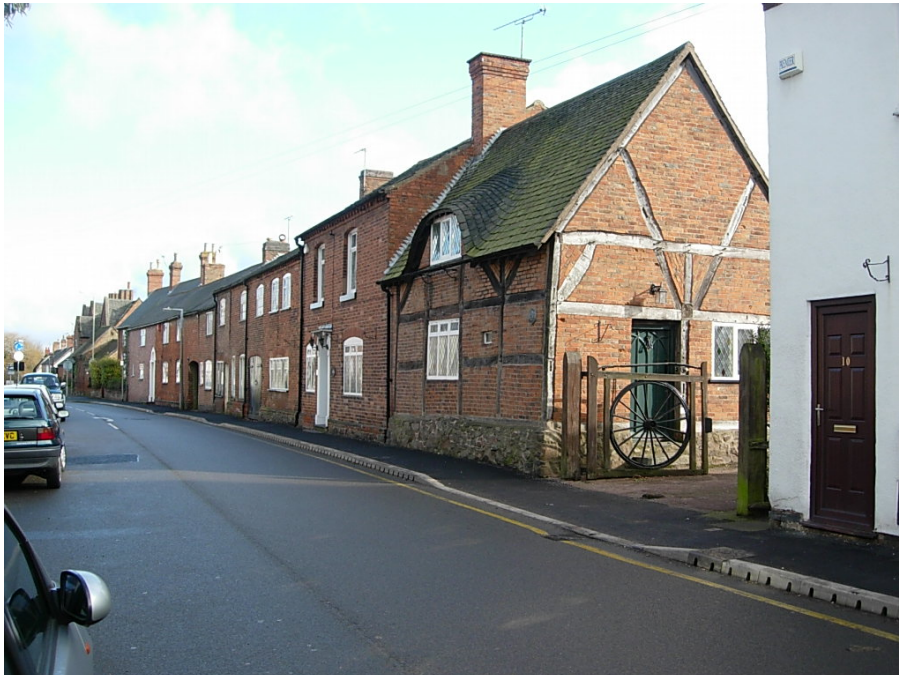
View showing the different roof heights and impact of chimneys on High Street. 16 High Street is a late C18 timber framed property with a eyebrow window. The dwelling is constructed in red brick and Flemish bond, with a Swithland slate roof.
