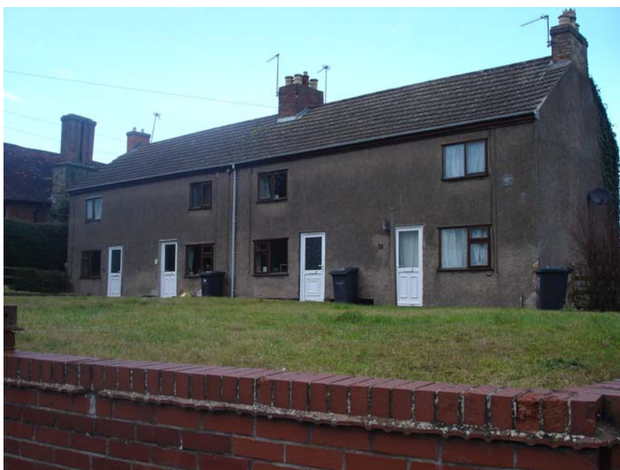
The terrace, 30-36 Newbold Road, has lost some of its traditional character due to insensitive alterations with the installation of plastic window, doors and concrete roof tiles.
