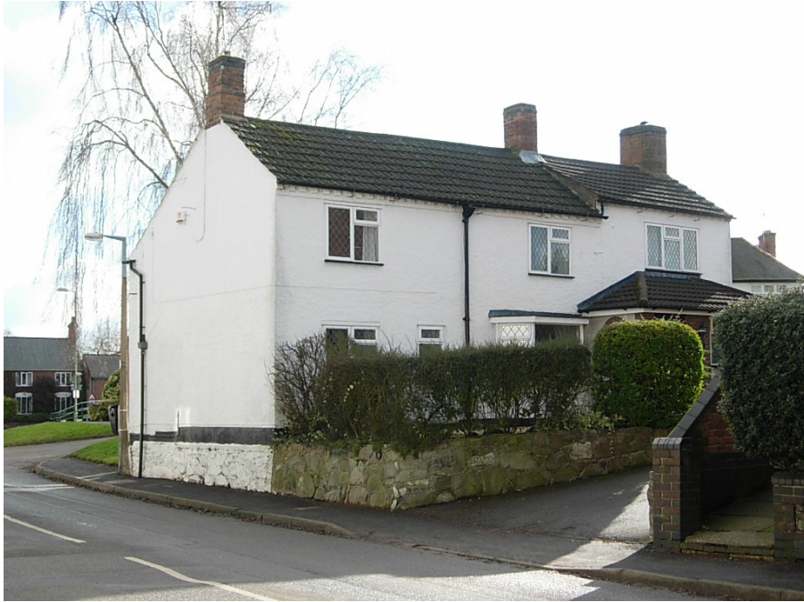
9 Main Street is a fine rendered property with its gable fronting the road that is spoilt by the choice of concrete roof tiles.
