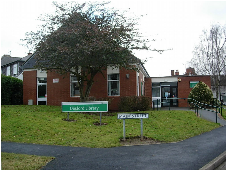
Desford Library is a modern building sited in a prominent location at the junction of Main Street and Manor Road. Unfortunately, the building does not reflect the traditional character of the conservation area.
