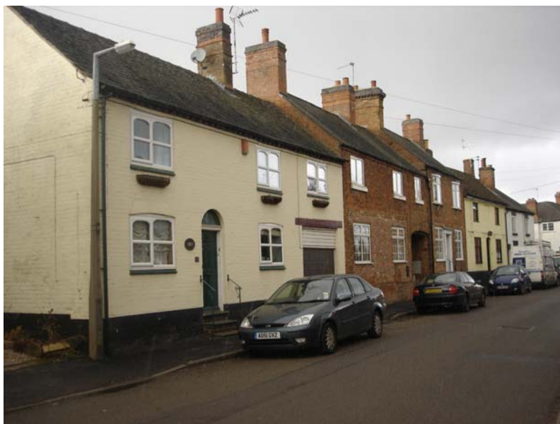
The properties, 53-59 Main Street, are attractive as a group but are spoilt by the modernisation of individual dwellings. The choice of plastic windows and the building of an integral garage tend to spoil the appearance of the terrace as a whole.
