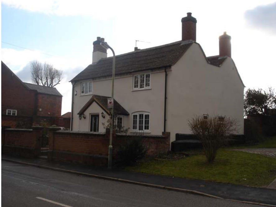
23 Main Street is a period property that has retained its attractive chimney stacks. It is tiled with Staffordshire Blue clay tiles.
