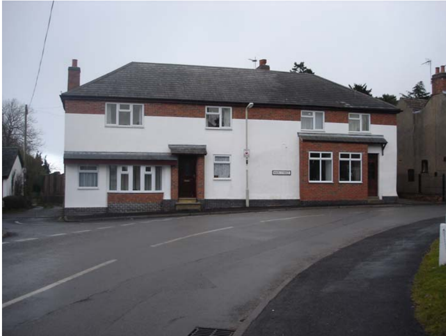
The elevation treatment of 80 Main Street is out of character with the traditional features of the conservation area.
