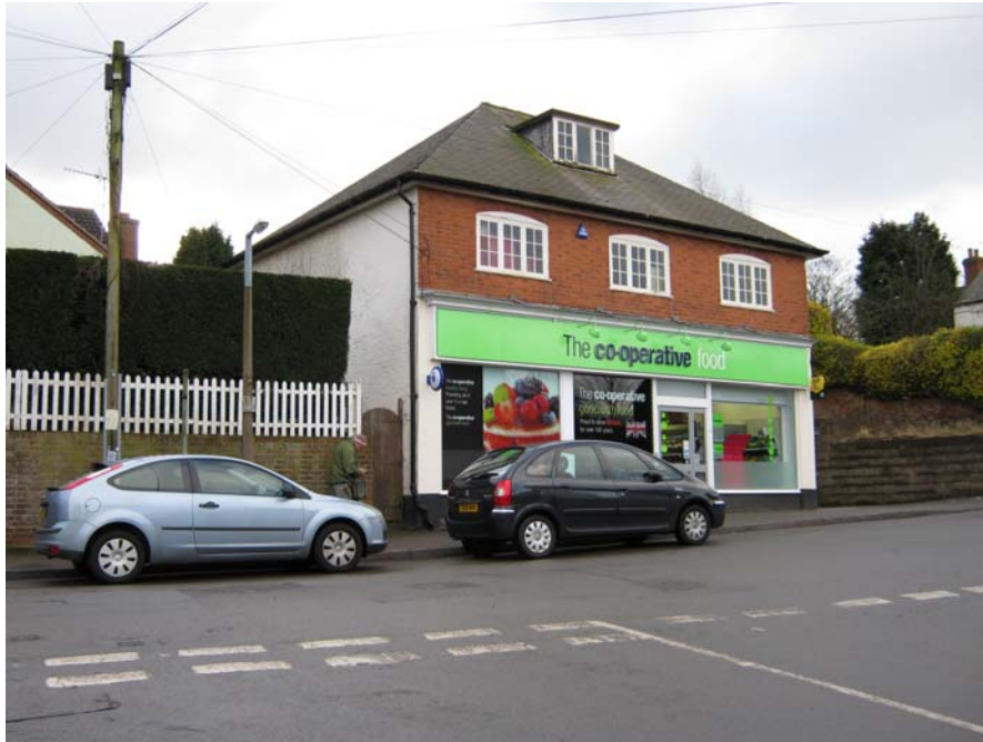
The shop front treatment to the Co-Op store on Newbold Road is too brash and prominent. Consideration needs to be given to reduce its visual impact in the street scene.
