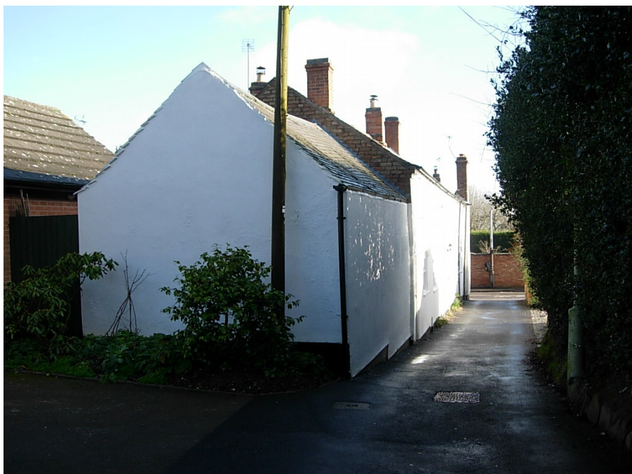
The properties, 2-6 Chapel Lane, were once framework knitters cottages.
