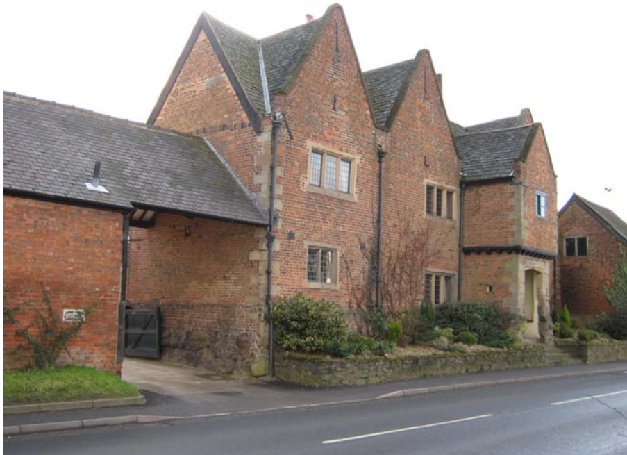
The Old Manor House on High Street is an early C17 Grade II* listed farmhouse built in red brick in English bond. The property has sandstone ashlar quoins and dressings and Swithland slate roof. The windows are stone mullioned with square leaded casements that have rectangular ashlar surrounds. To the left is a brick barn that has been converted into a dwelling and to the right, forward of the house, is an early C18 service block built in Flemish bond.
