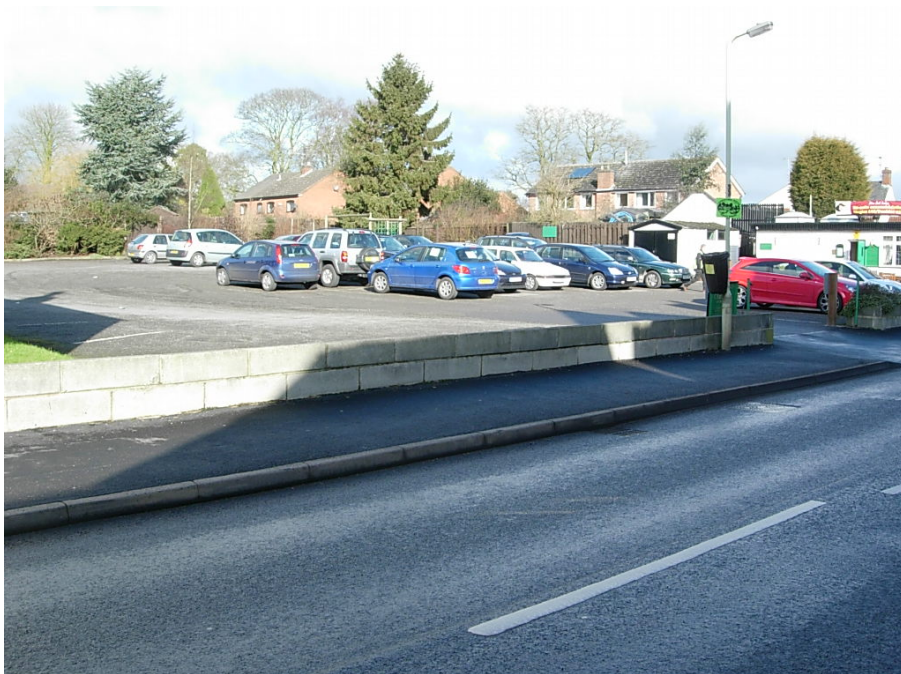
The block wall fronting the Bluebell Pub Car Park is an unattractive feature that needs replacing with a traditional brick wall.
