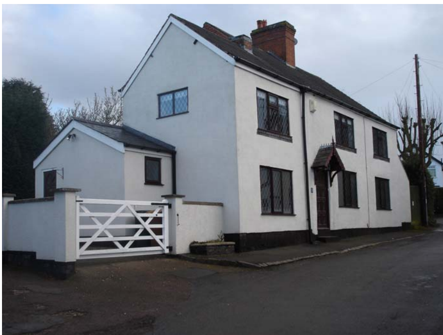
3-7 Cottage Lane is typical in design and treatment with the dwellings sited at the northern end of the Cottage Lane.
