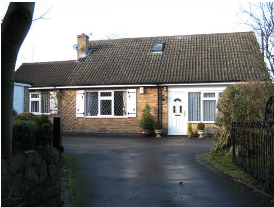
12 Chapel Lane is a dwelling of modern design and materials that has a negative impact on the conservation area.
