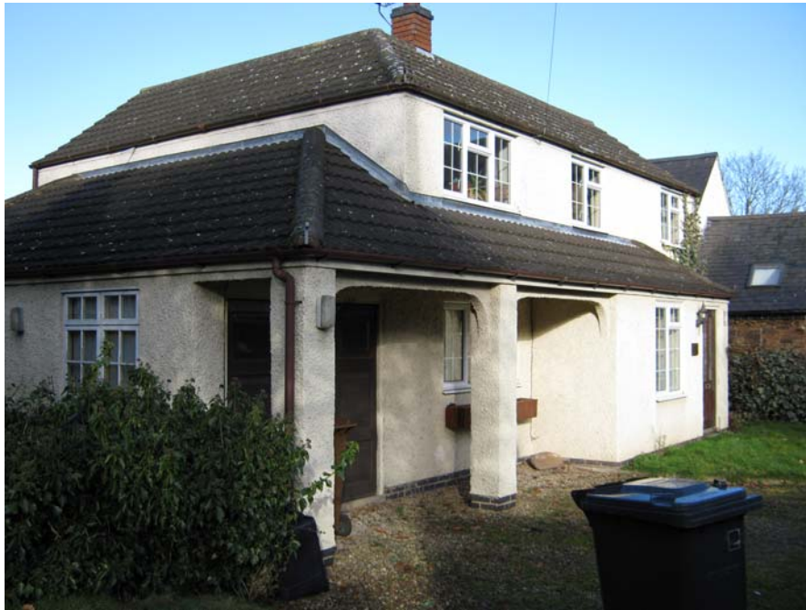
The dwelling, 19 Cottage Lane, does not respect the traditional character of the conservation area by way of its design and choice of materials. The canopy is a particularly incongruous feature.
