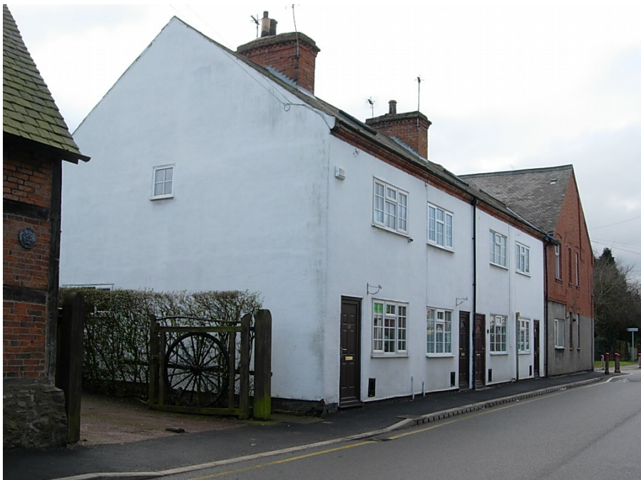
The rendered terrace 4-10 High Street has been spoilt with the insertion of roof lights and plastic windows.
