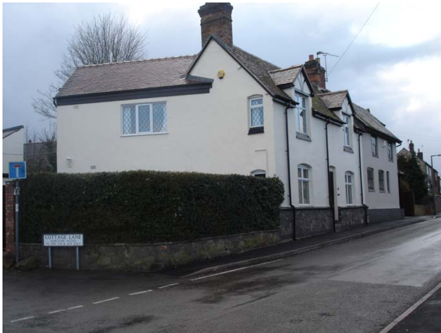
The dwellings, 33-35 Newbold Road, are attractive rendered properties sited at the entrance into the conservation area on Newbold Road.
