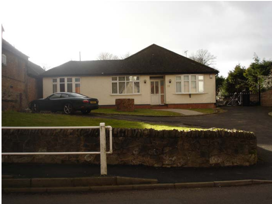
This modern bungalow, 35 Main Street, does not reflect the traditional character of the village by way of design, materials and siting.
