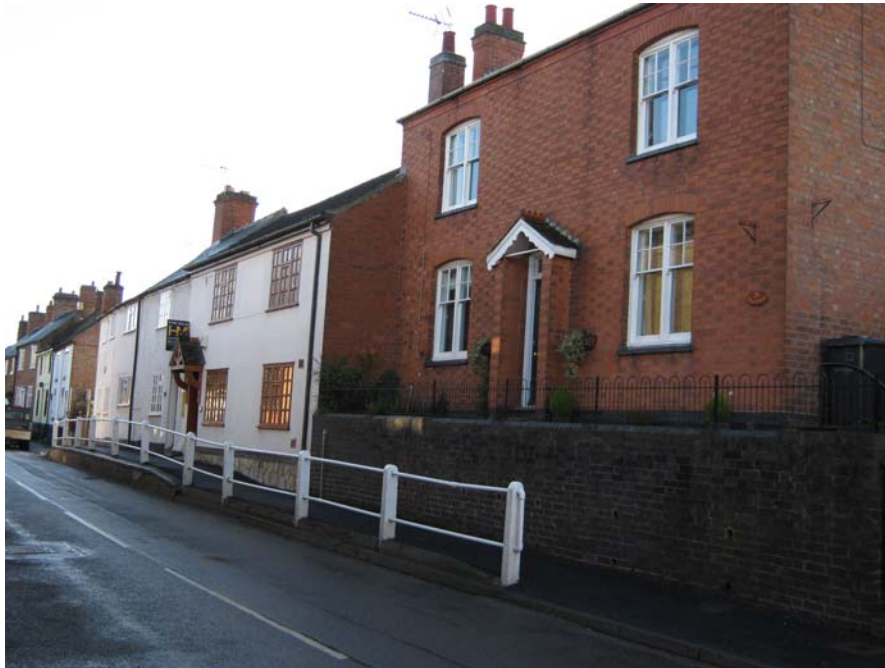
75 Main Street is an attractive property that occupies a prominent position in the street scene sited behind a blue brick retaining wall.
