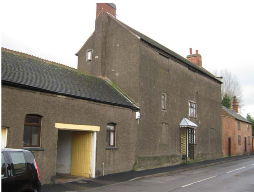
Prior Farm on Main Street is one of only a small number of three storey buildings located in the conservation area. This rendered property that has had several of its windows blocked in on its front elevation, has an attractive rear elevation.
