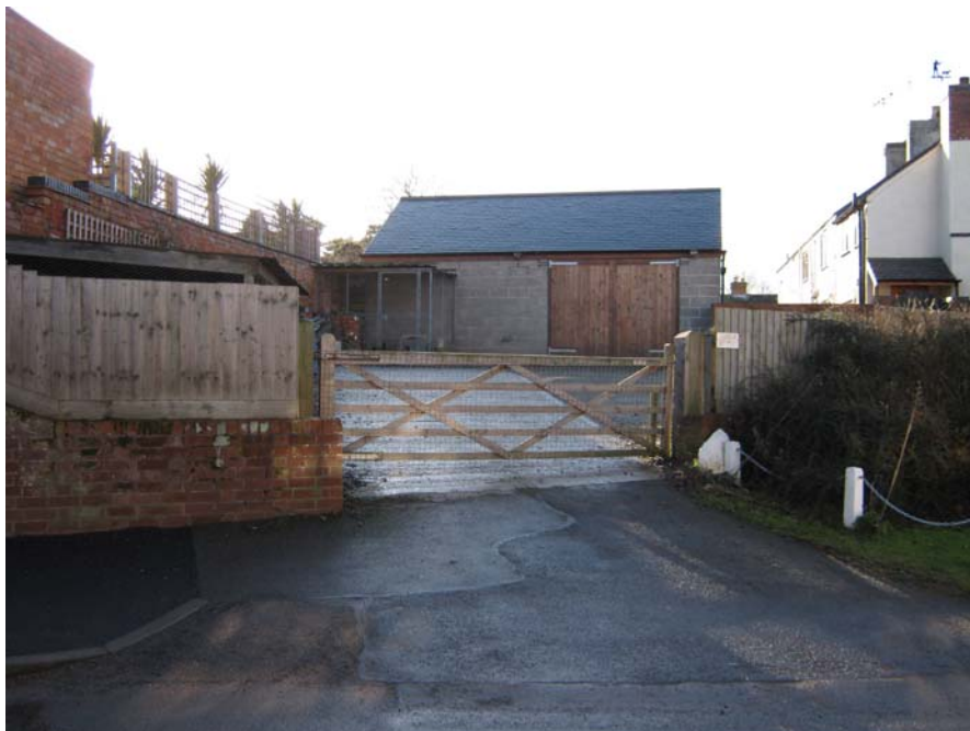
This small holding sited at the northern end of Main Street with its agricultural gate is a remnant of the past. It is unfortunate that the outbuilding has been built with concrete blocks. The site has development potential.
