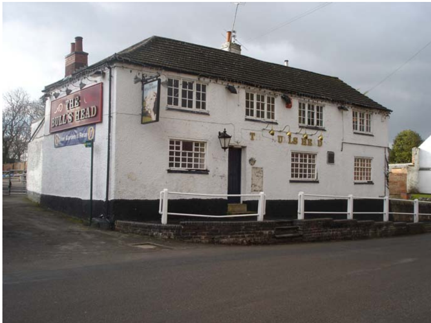
The Bulls Head pub is currently being converted to a dwelling and will probably lose its pub signs. The raised pavement and post and rail fence is an appealing feature fronting the premises.
