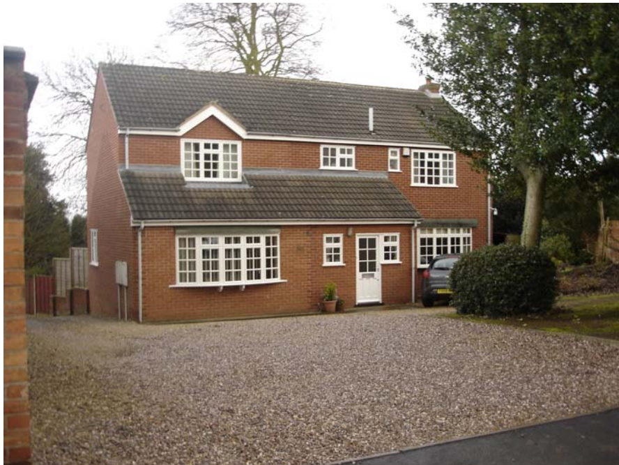
This modern dwelling, 56 Main Street, does not reflect the traditional character of the village by way of design, materials and siting.
