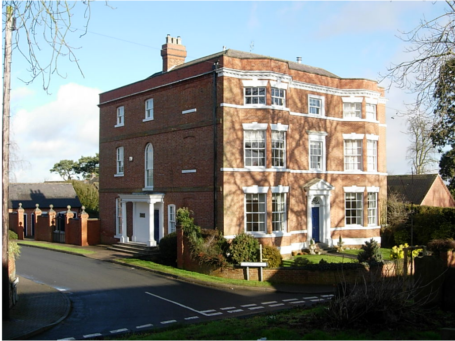
The Grange on Church Lane is a Grade II listed building built in 1799 with some C19 and C20 alterations. The red brick walls are built in Flemish bond with stucco dressings and slate roof. The central doorway has a traceried fanlight and pedimented doorcase.
