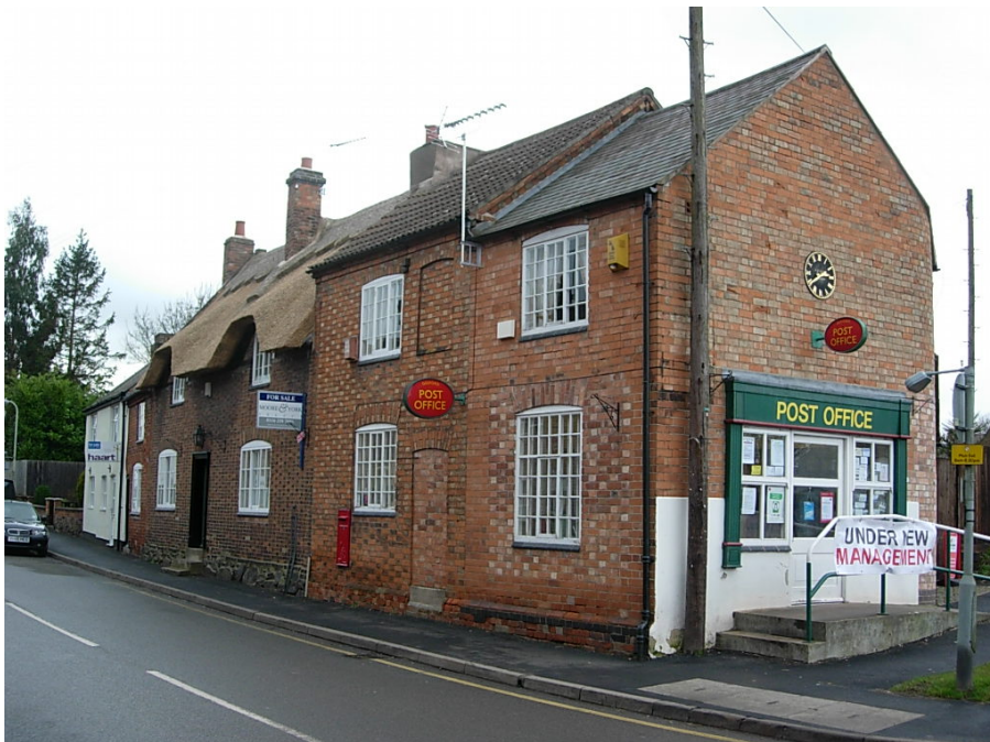
19, 21 and 23 High Street are late C18 to mid C19 Grade II listed properties with a combination of thatch, slate and concrete roof tiles. Consideration needs to be given to replacing the concrete tiles with Swithland tiles. The insensitive use of the concrete ramp into the Post Office is also unfortunate.
