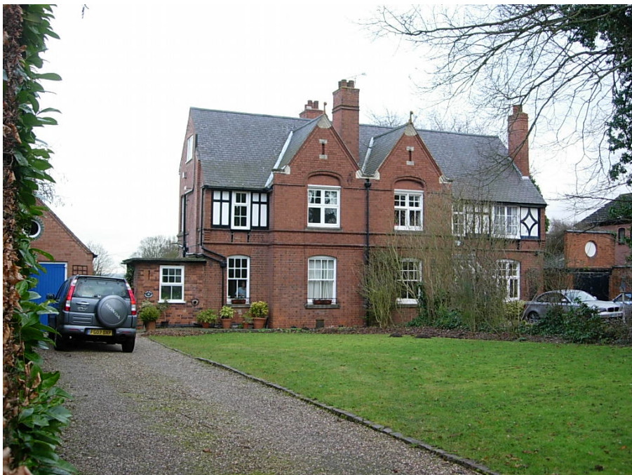
23-25 Church Lane are a fine pair of imposing semi detached properties set back a considerable distance from the carriageway.
