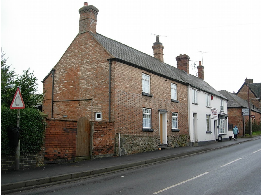
40-44 High Street is an attractive terrace that still retain its chimneys.
