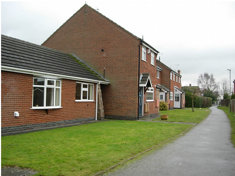
The modern terrace, 7-13 Stewards Court, fronts the footpath. The properties help to give enclosure along the footpath, however their design and choice of materials do not enhance the character of the conservation area.
