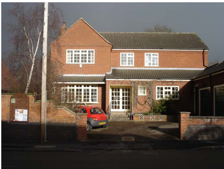
44 Main Street is a modern dwelling that would have been better sited outside the conservation area due to its design and choice of materials.
