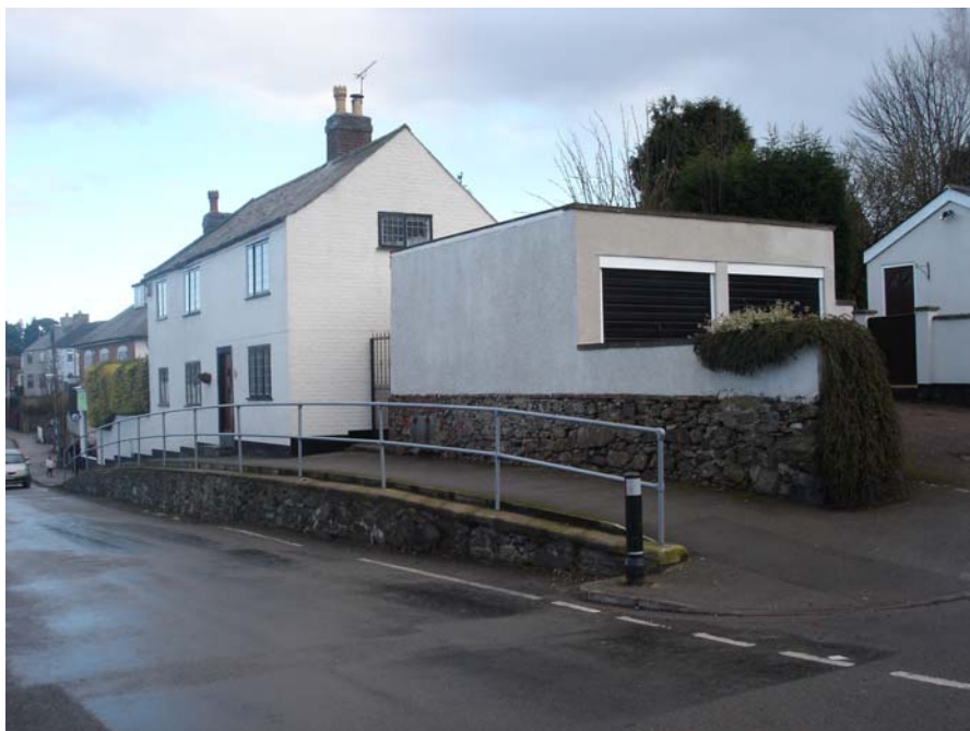
The new railings installed fronting 29 Newbold Road do not have the same visual appeal or match the rest of the post and rail fences sited in other parts of the village. The flat roof double garage does not respect the traditional character of the conservation area.
