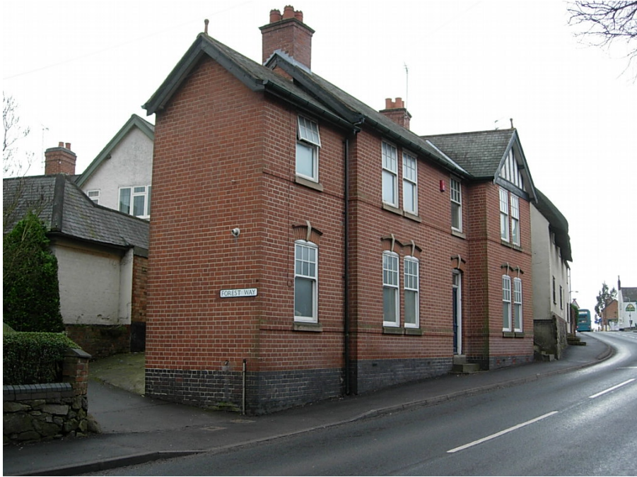
The property, 54 High Street, is a tall imposing building built in red brick and slate roof.
