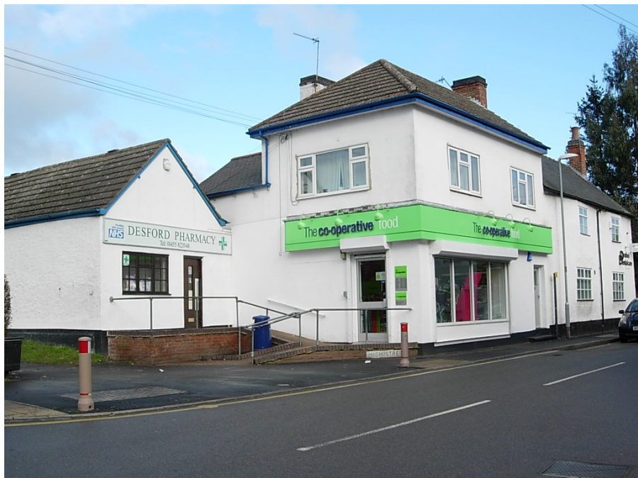
The shop fascia to the Co-Op store is too visually dominant and the building's original features have been lost.
