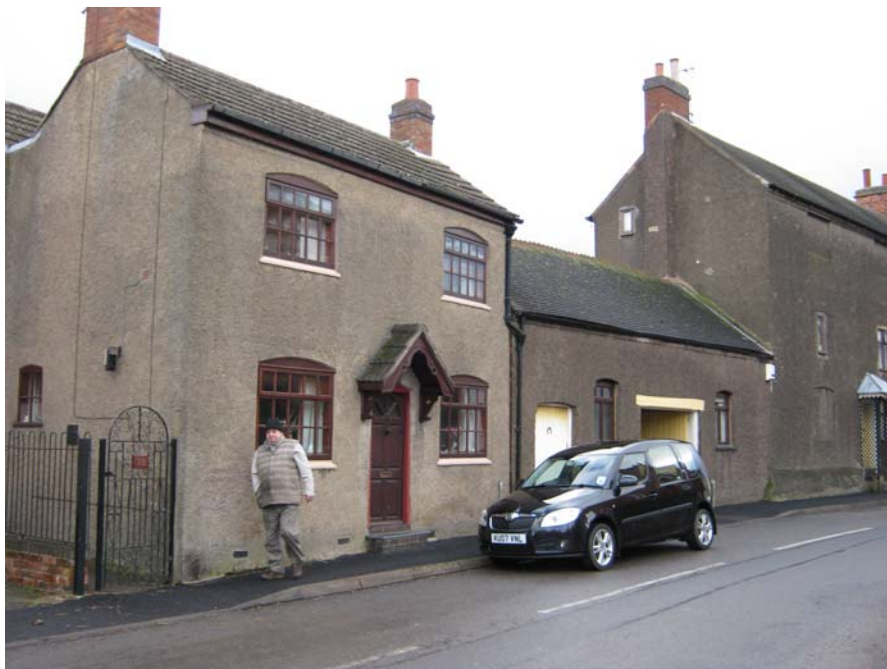
76 Main Street is a small period cottage spoilt by the use of concrete roof tiles.
