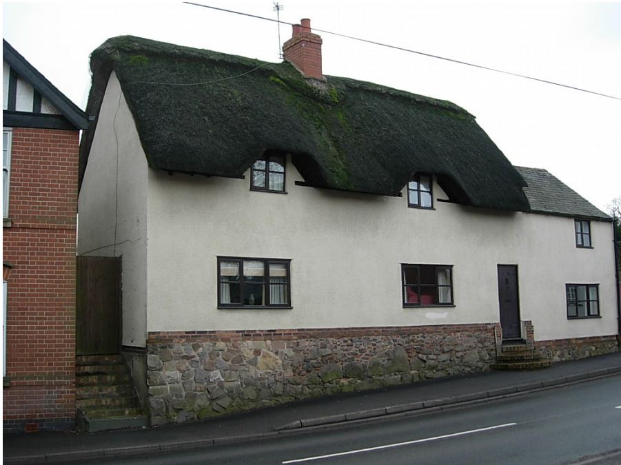
52 High Street is an excellent traditional cottage with eyebrow dormers and thatched roof that stands on a granite base.
