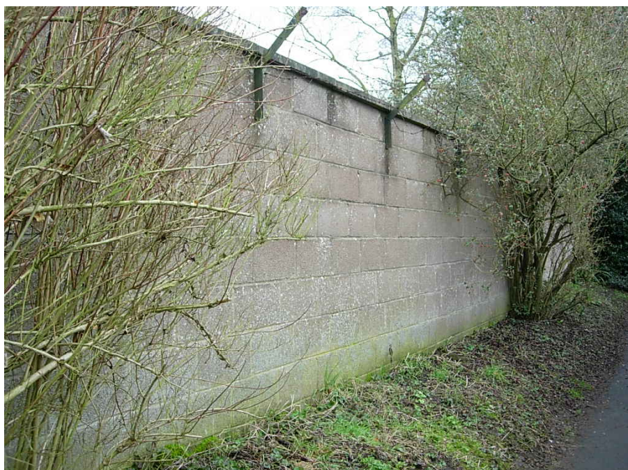
The concrete block boundary wall to the Desford Free Church is an unattractive feature running along the footpath leading to the Pickard Recreation Ground. It needs to be finished with render.
