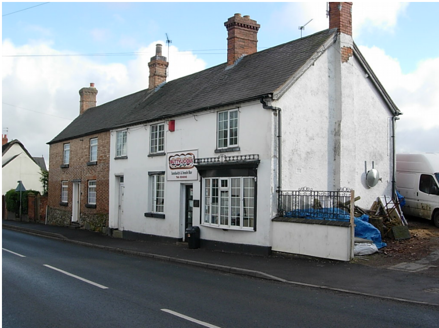
The bow window and wall fixed sign to the shop at 40 High Street are out of character with other traditional properties on the road.
