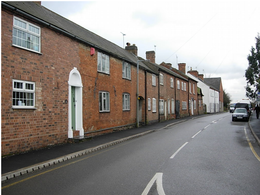
Excellent view of the terraced properties that run up the southern side of High Street.
