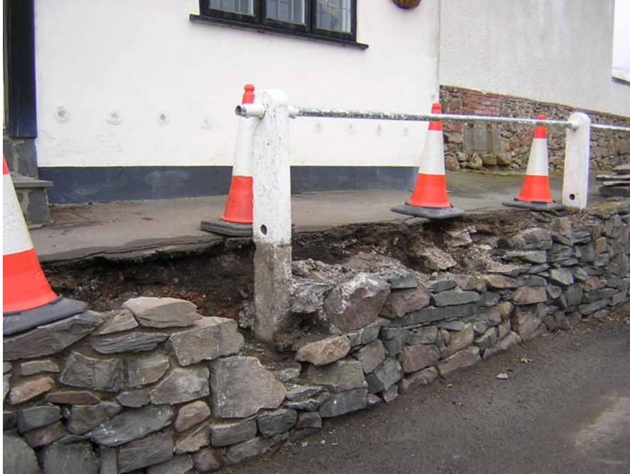
The raised pavement fronting 29 Newbold Road before the stone retaining wall was rebuilt shows the concrete post and rail fence before it was replaced.
