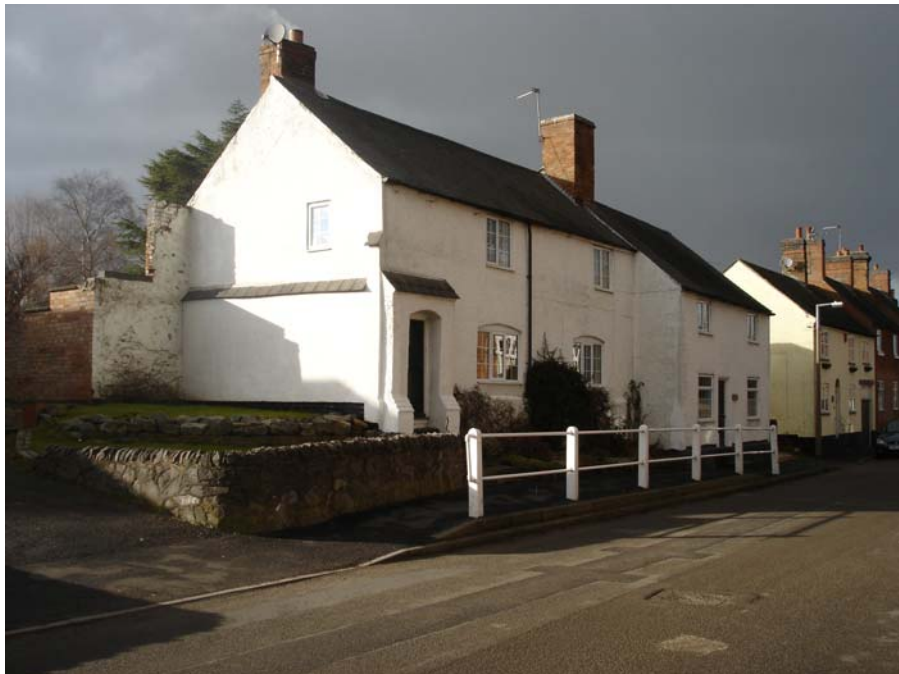
The attractive terrace, 47-51 Main Street, showing the end of the property sited forward. The post and rail fence enhances the setting. Unfortunately one of the properties has lost its chimney pot.
