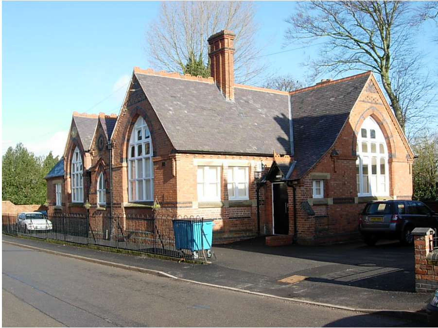
Desford School on Main Street is a Grade II listed property built in 1876. The former school is built in the same style and materials as the adjacent School Master's house.
