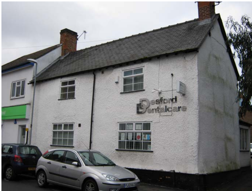
3 High Street is a period building and its timber frame is still evident in the property's gable wall.
