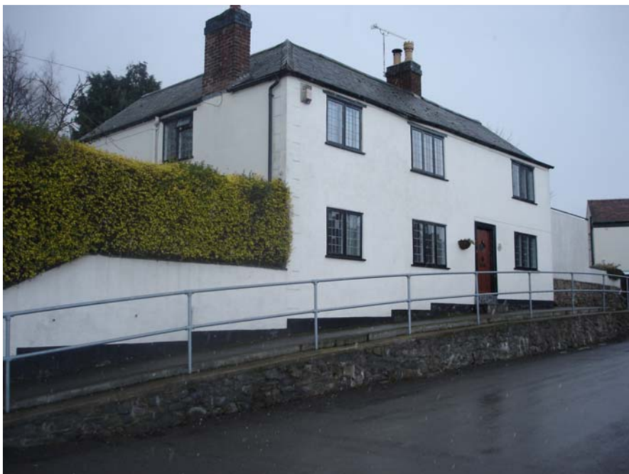
29 Newbold Road is an attractive rendered dwelling fronting a raised pavement. It is unfortunate that the original railings have been replaced with modern railings.
