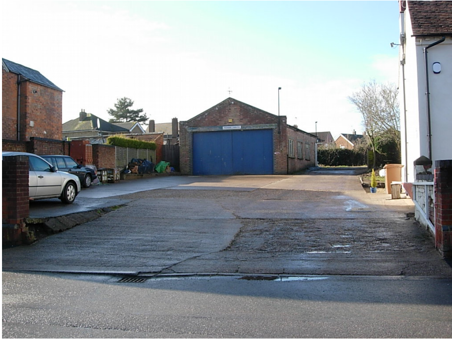
The haulage depot with its large concrete forecourt is an unattractive feature on Main Street. The site has re-development potential.
