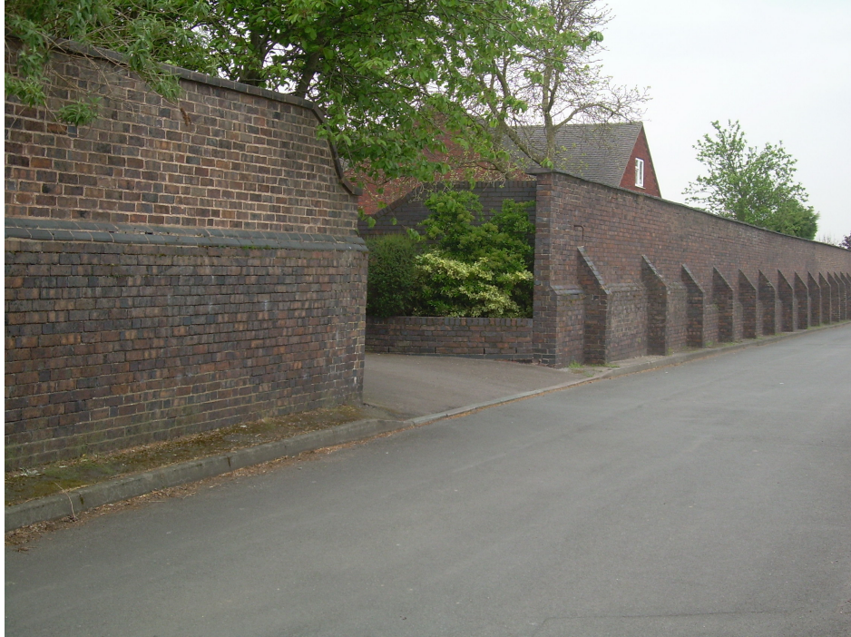
The high buttressed wall delineates the conservation area boundary
