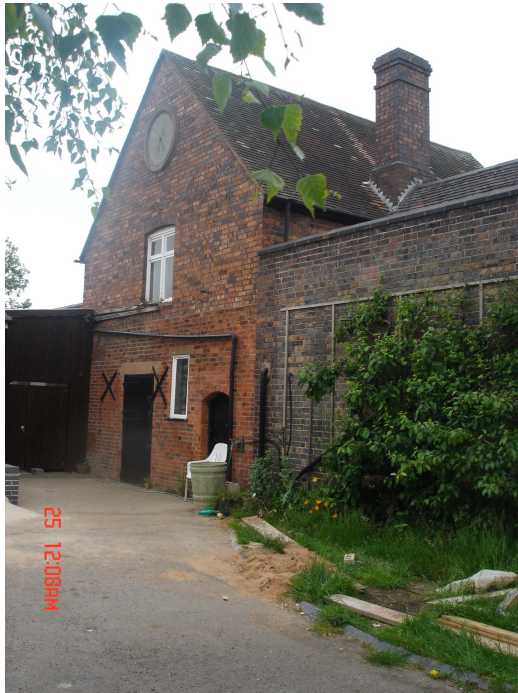
Interesting building with clock on the gable end that was once accessed from the walled garden Used as a store and hay loft and possibly by the estates farrier
