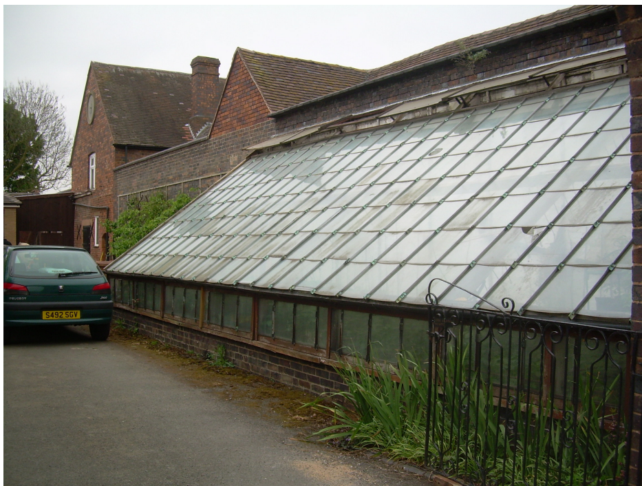
Greenhouse that was originally part of the walled garden to Witherley Hall
