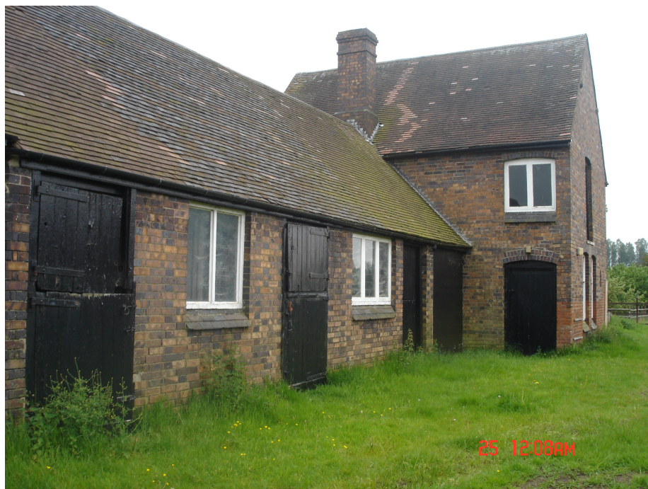
The store and hay loft from its north eastern side showing the stables. The property has planning consent for conversion to a dwelling
