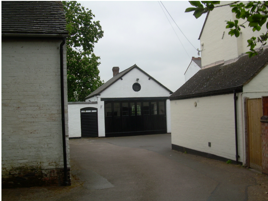
A double garage on Hall Gardens which is in sympathy with its dwelling in both scale and use of materials with a glazed timber door that folds into several sections
