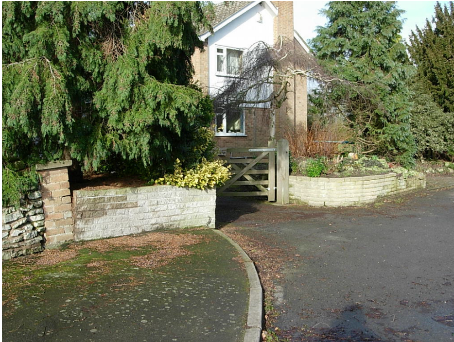
(3) The block wall on Shackerstone Road needs replacing with traditional Carlton stone wall
