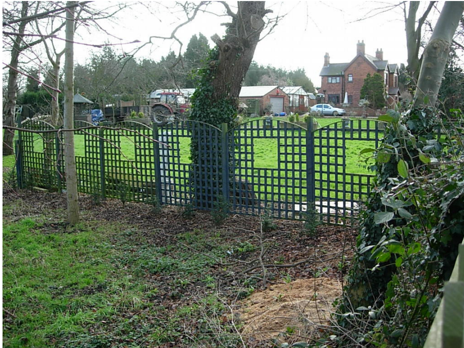
(1) Existing fence at the entrance to the conservation area on Shackerstone Road is an incongruous feature which needs replacing with a more traditional fence
