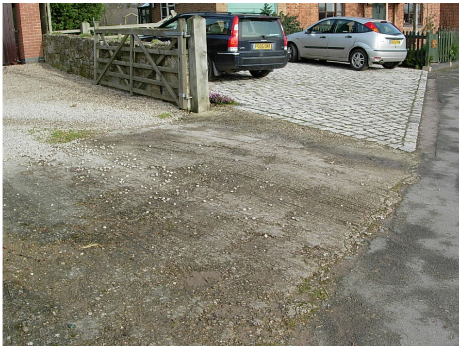
(8) Area would be improved on Barton Road if the unsightly concrete apron was replaced with granite setts to match the adjacent property
