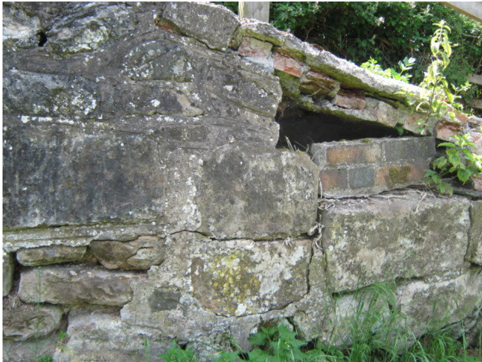
Bridge 23 showing the towpath access needs repairing
