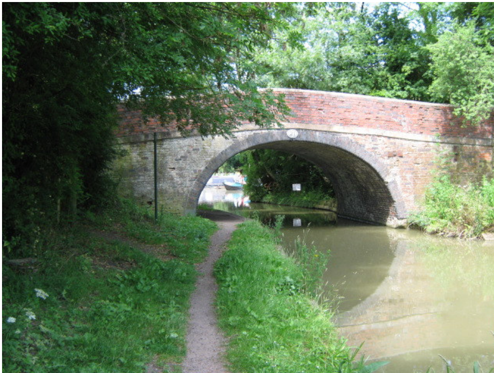
Bridge 21 South Elevation
