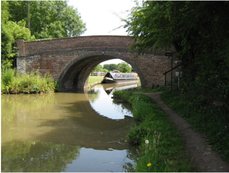
Bridge 22 (Basin Bridge) North Elevation This bridge is in need of repairs
