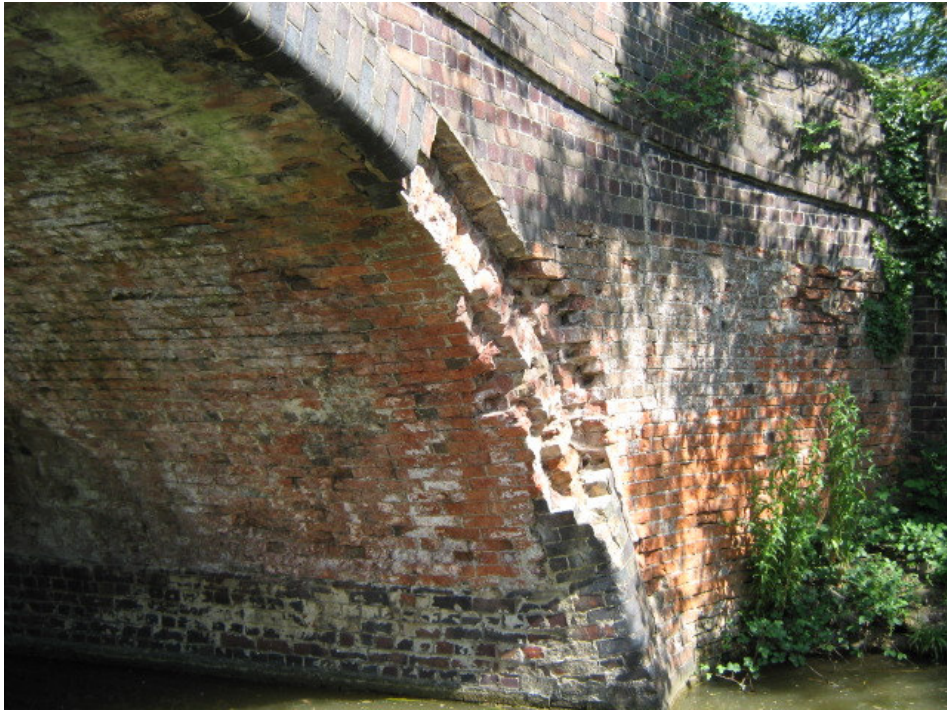
Bridge 26 South Elevation The arch's brickwork is collapsing and in need of repair
