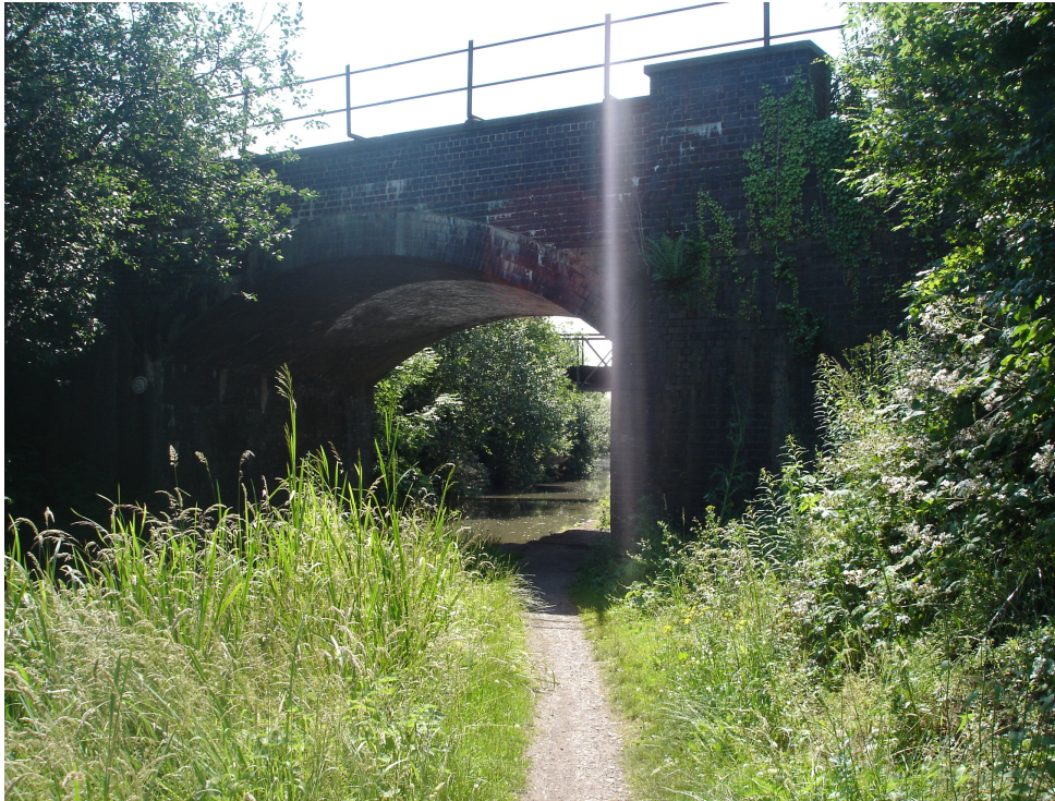
Leicester to Nuneaton Railway Bridge, Northern Elevation This railway bridge is a fine brick structure in good condition. Unfortunately, the modern safety railings that have been added to the parapet detracts from its appearance
