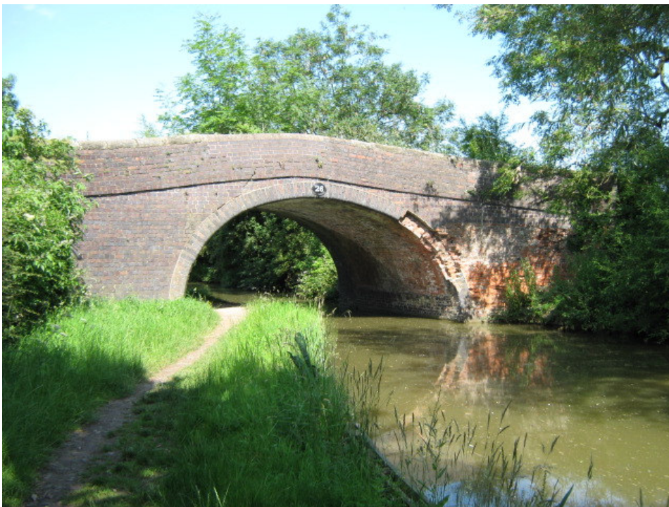
Bridge 26 South Elevation
