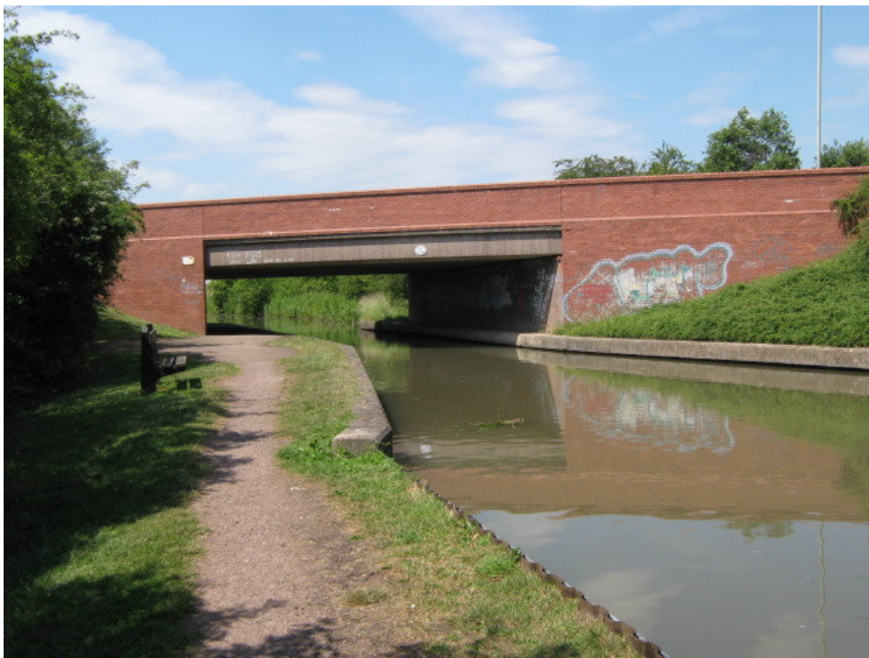
Bridge 17a Southern Elevation
