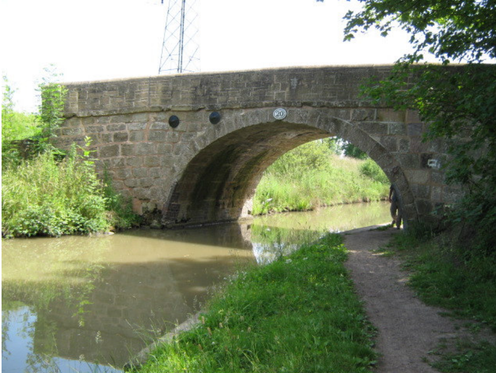
Bridge 20 (Frieston's Bridge) North Elevation
