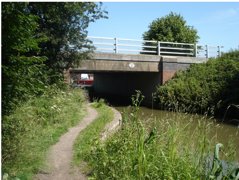
Bridge 17 Southern Elevation The bridge has two different styles of railings on its opposite elevations. This could be improved by the adoption of a consistent approach to this feature
