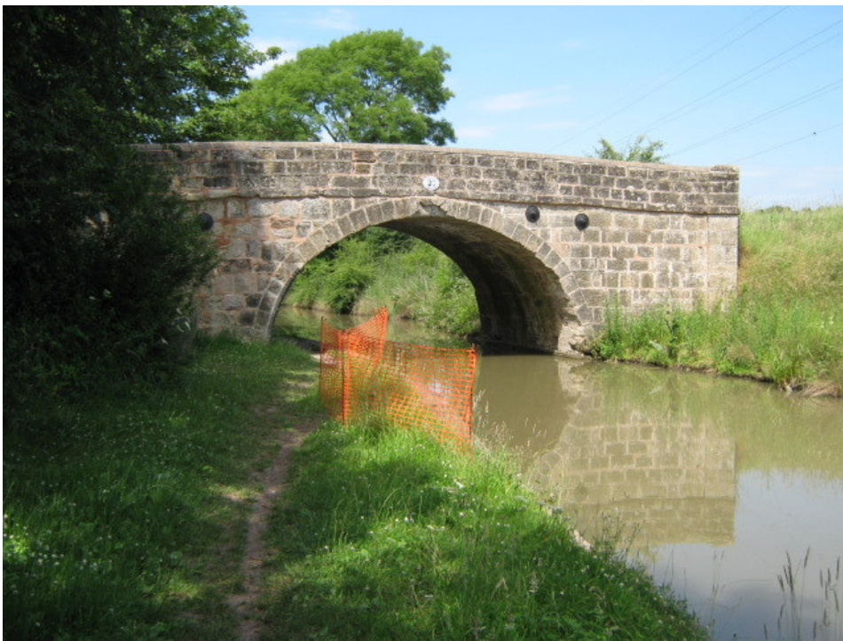
Bridge 20 South Elevation
