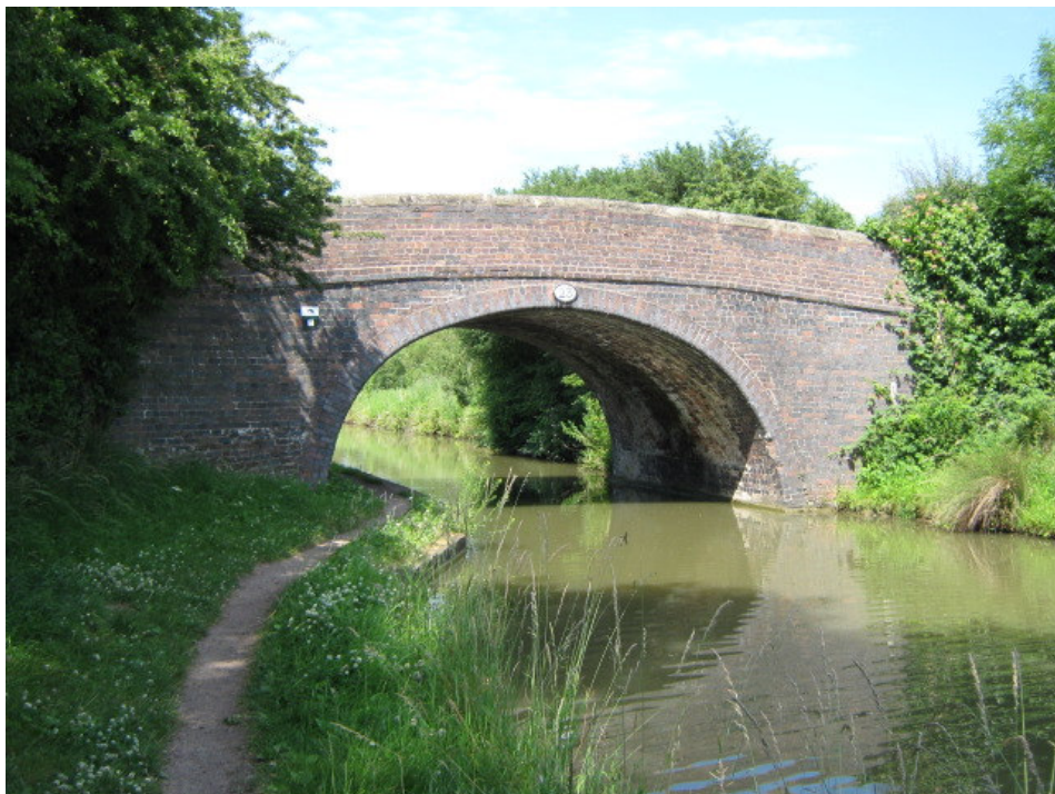
Bridge 23 South Elevation
