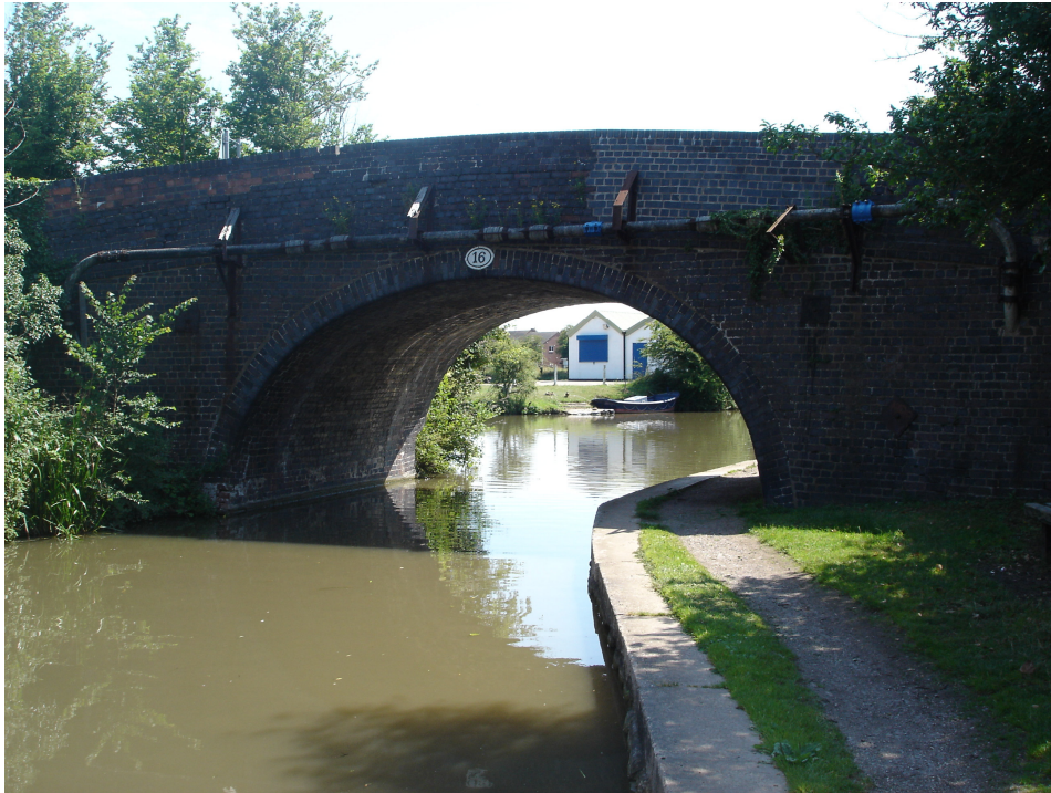
Bridge 16 (Nutt's Bridge) North Elevation
