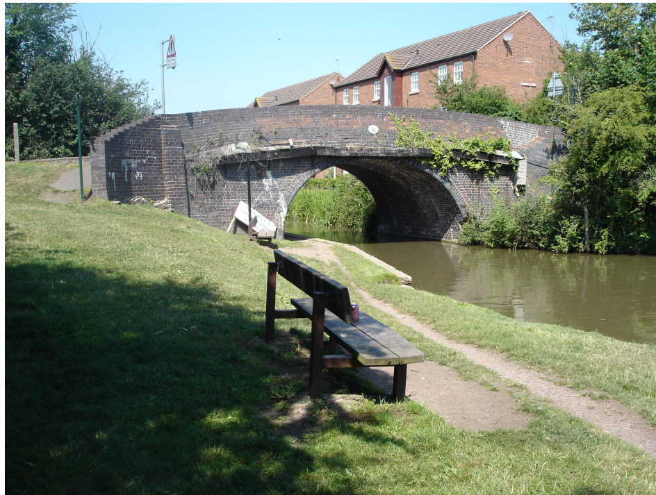
Bridge 16 Southern Elevation
