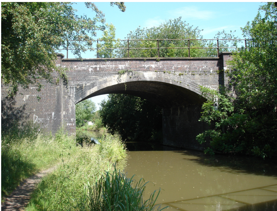
Leicester to Nuneaton Railway Bridge, Southern Elevation
