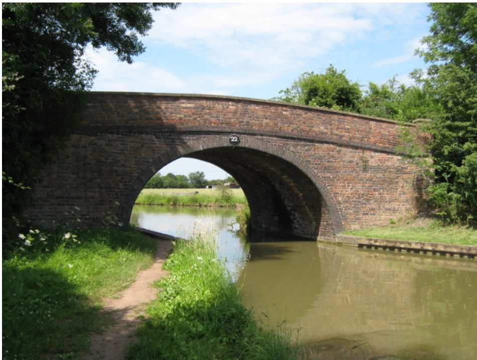
Bridge 22 South Elevation
