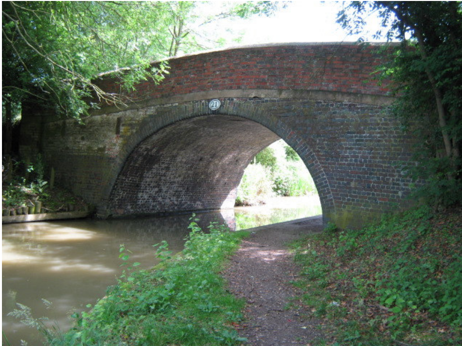
Bridge 21 (Wykin Bridge) North Elevation This bridge is in fair condition with no obvious repairs needed
