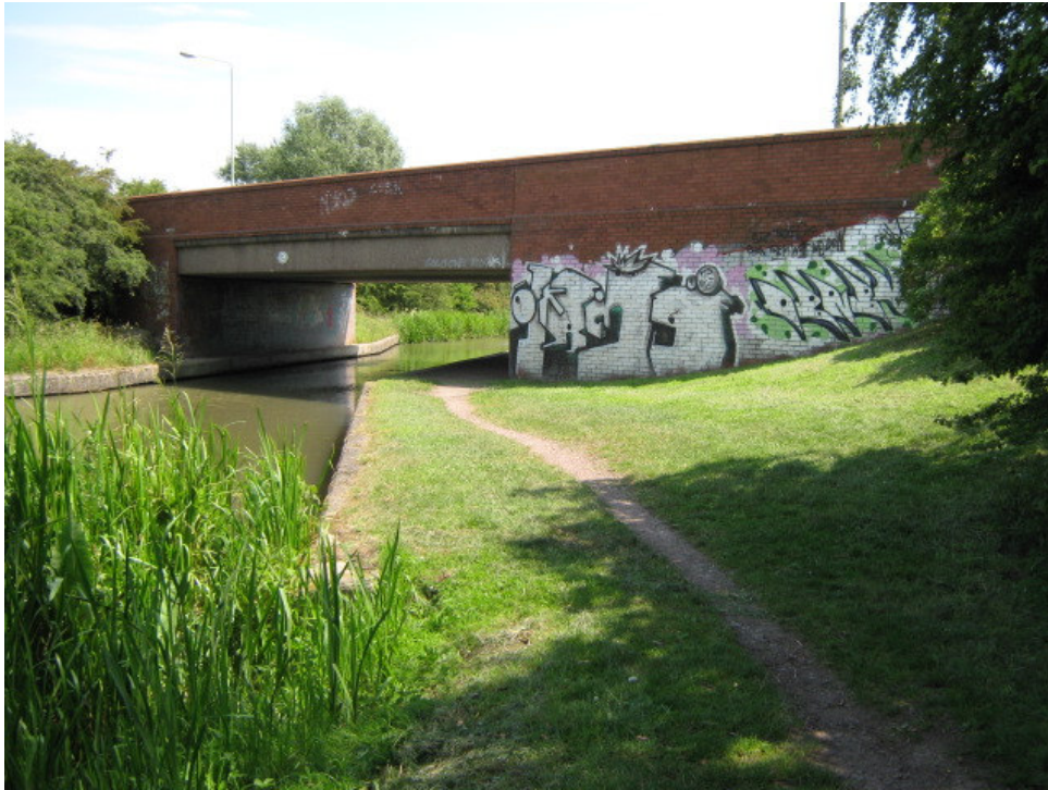
Bridge 17a (Dodwell's Road Bridge) North Elevation This modern concrete road bridge is out of character with the canal. The bridge was built in the 1970's and forms part of the Hinckley Northern Perimeter Road. It has been heavily painted
