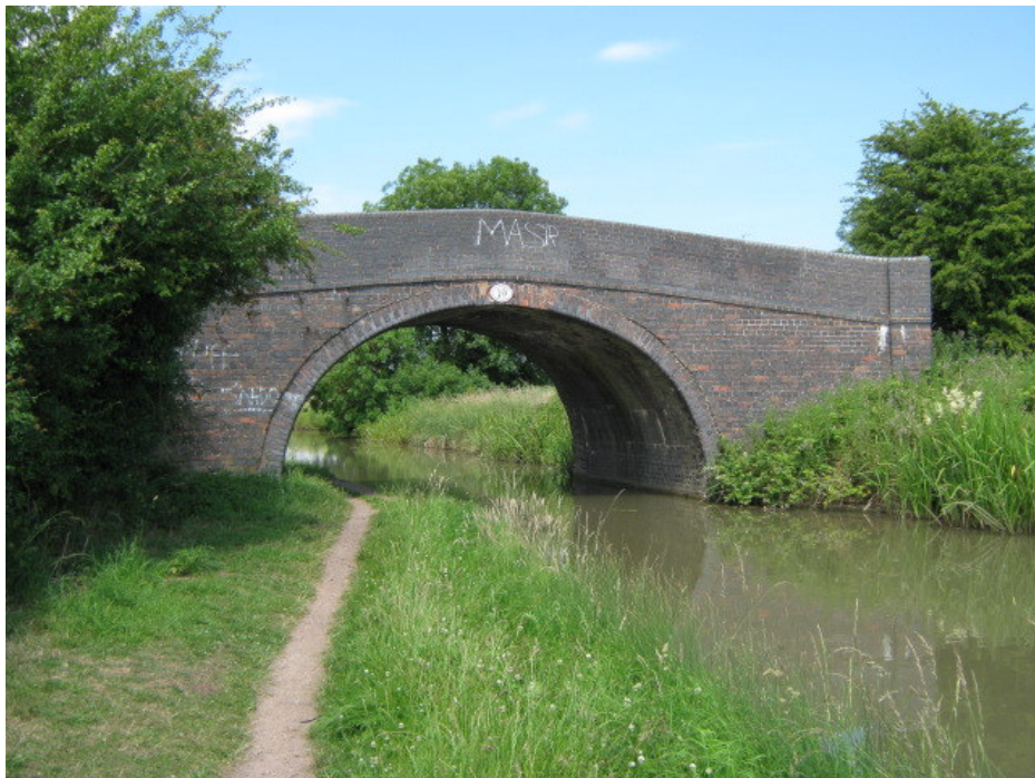
Bridge19 South Elevation
