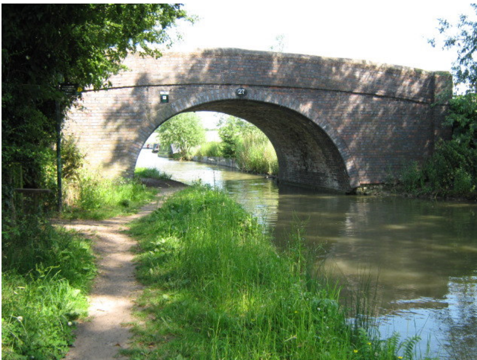
Bridge 27 South Elevation
