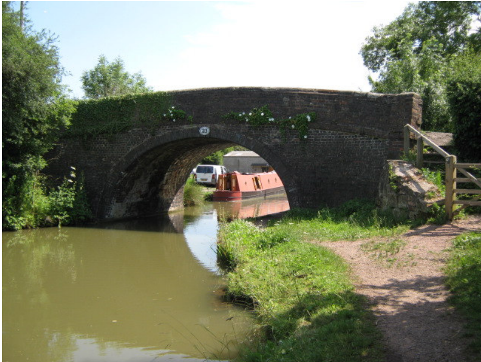
Bridge 23 (Higham Bridge) North Elevation This brick road bridge is generally in fair condition although the wall needs repairing
