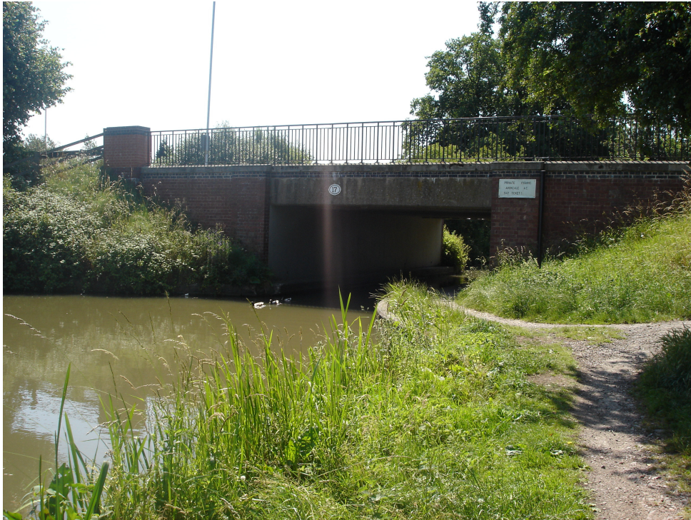
Bridge 17 (Coventry Road Bridge) Northern Elevation This modern concrete road bridge that takes traffic on Coventry Road is out of character with the canal.
