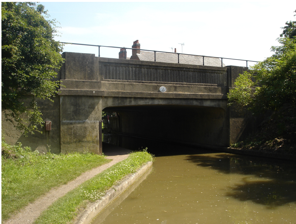
Bridge 15 Southern Elevation Although the bridge is not a brick structure, it has a neutral impact on the canal
