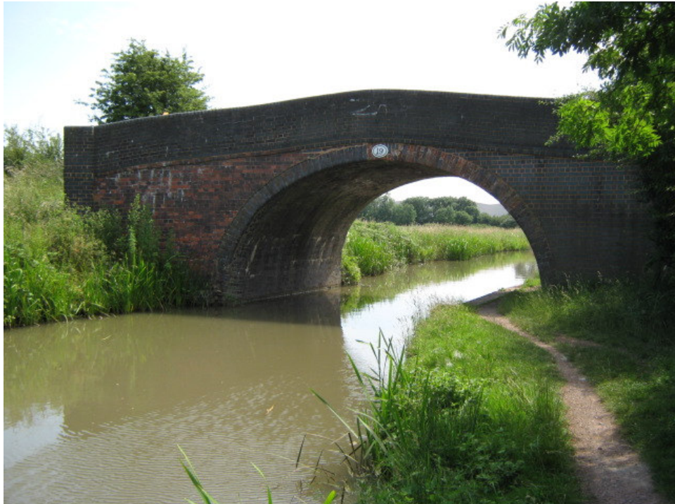
Bridge 19 (Barn Lane Bridge) North Elevation
