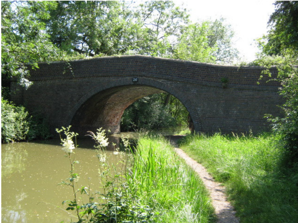
Bridge 26 (Foxwell's Bridge) North Elevation The bridge needs repairs at water level
