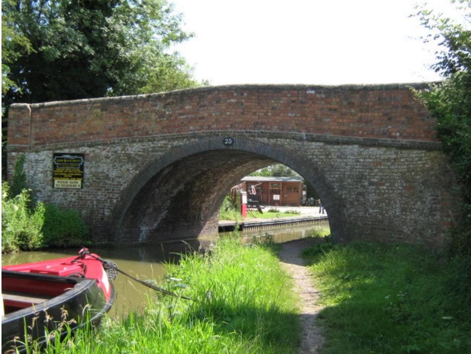
Bridge 25 (Stoke Golding Wharf Bridge) North Elevation Although this road bridge is in a good state of repair, its parapets have been replaced with non matching brick work
