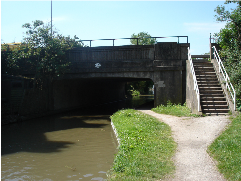
Bridge 15 ( Watling Street Bridge) Northern Elevation The bridge is a major concrete structure that carries the A5 Watling Street over the canal
