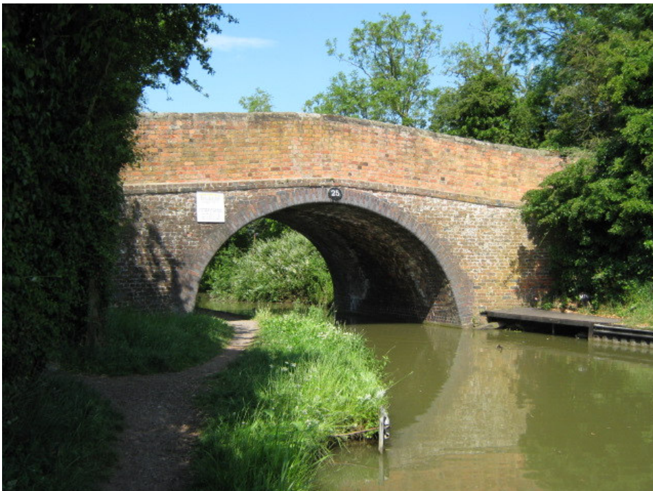
Bridge 25 South Elevation
