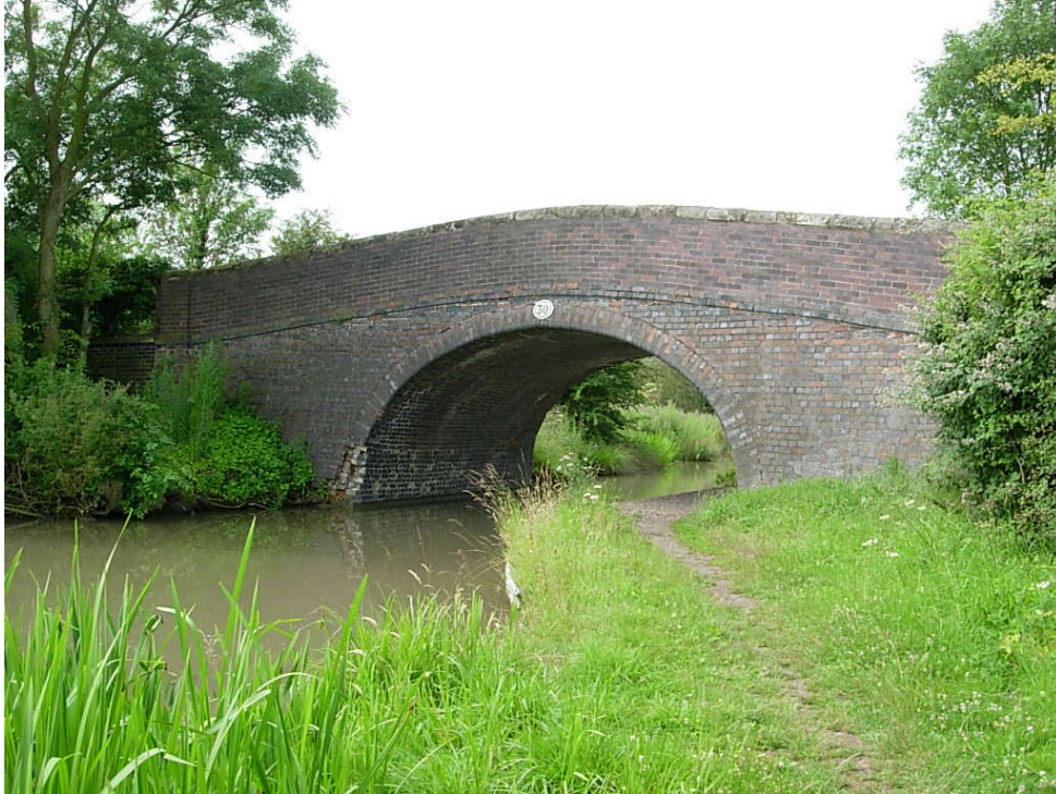
Bridge 30 (Dadlington Wharf Bridge) North Elevation This road bridge has had significant repairs. Unfortunately, the parapets have been rebuilt in stretcher bond although the stone copings have been re-seated and are complete
