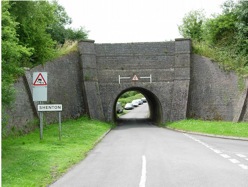
Shenton Aqueduct East Elevation
