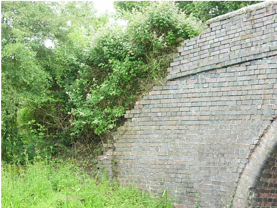
Bridge 29 North Elevation
