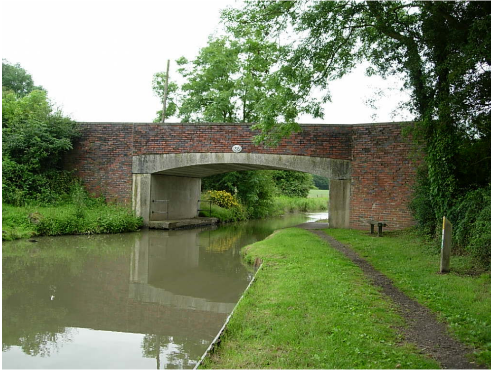
Bridge 35 (Bradfields Bridge) North Elevation A modern concrete road bridge in good condition
