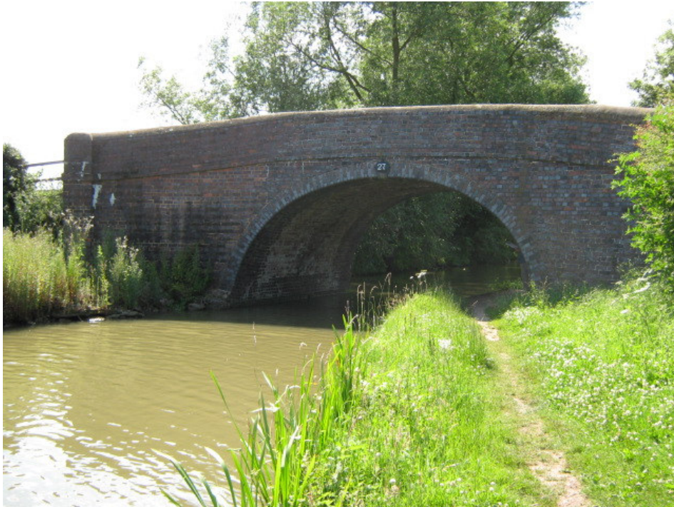
Bridge 27 (Foster's Bridge) North Elevation
