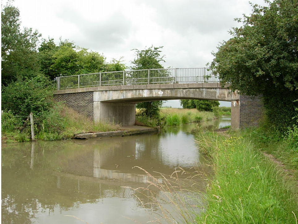
Bridge 32 (Dadlington, Sutton Lane Bridge) North Elevation This modern concrete road bridge with metal railings is out of character with the canal
