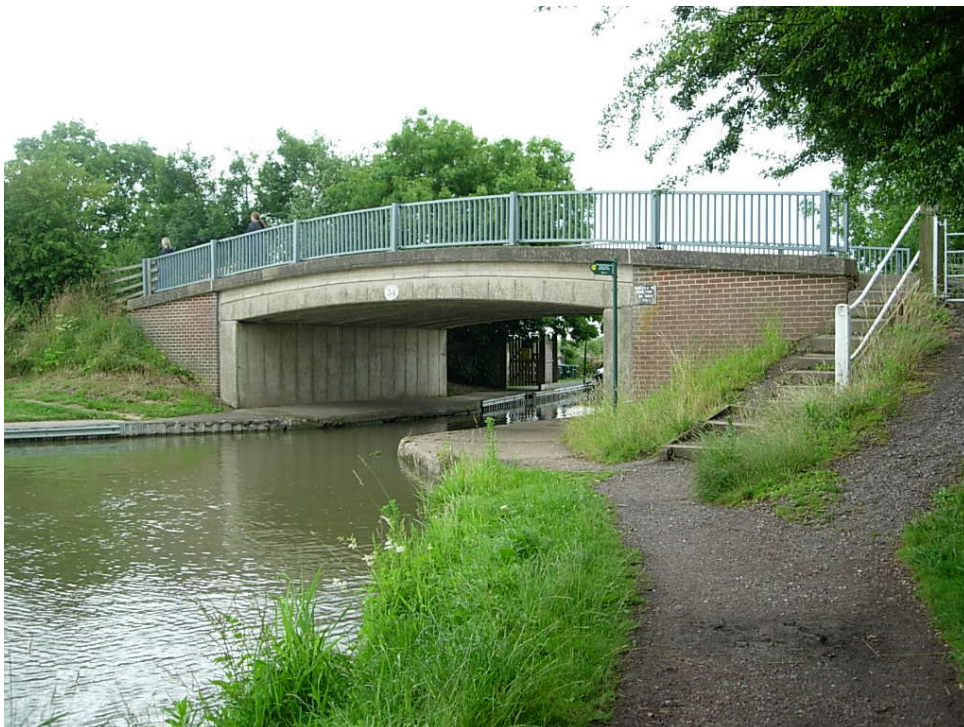
Bridge 34 North Elevation Insensitive modern railings protect the edge of the steps down to the canal towpath
