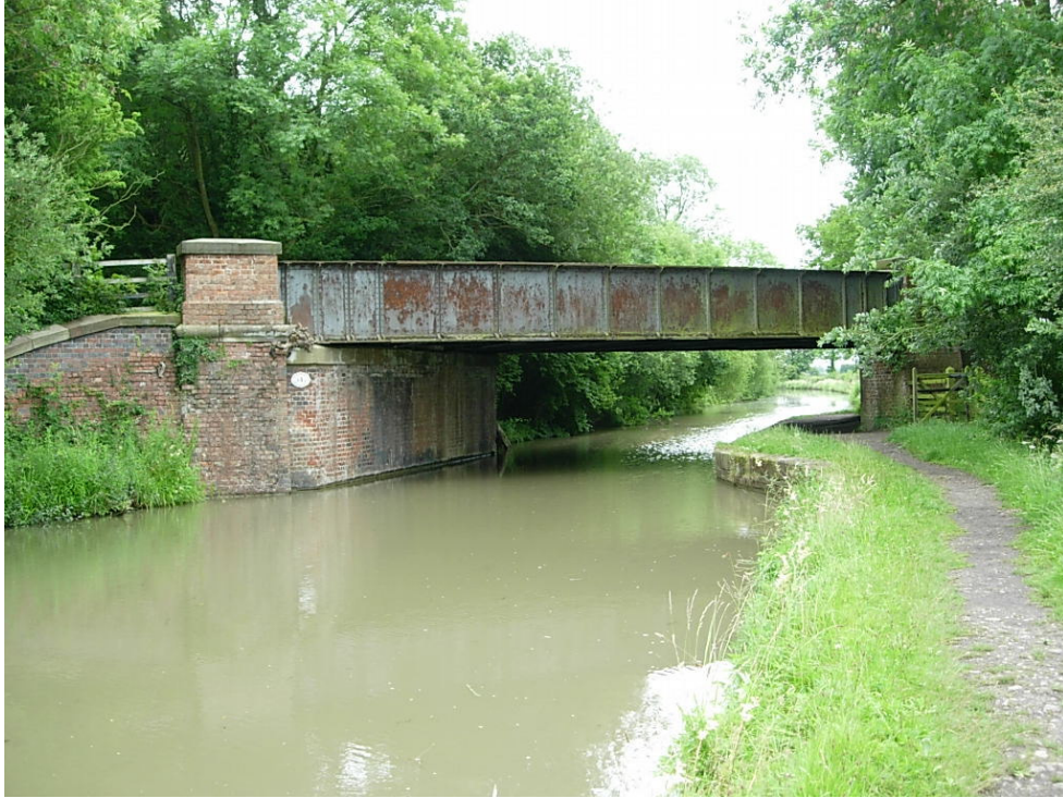
Bridge 34a North Elevation
