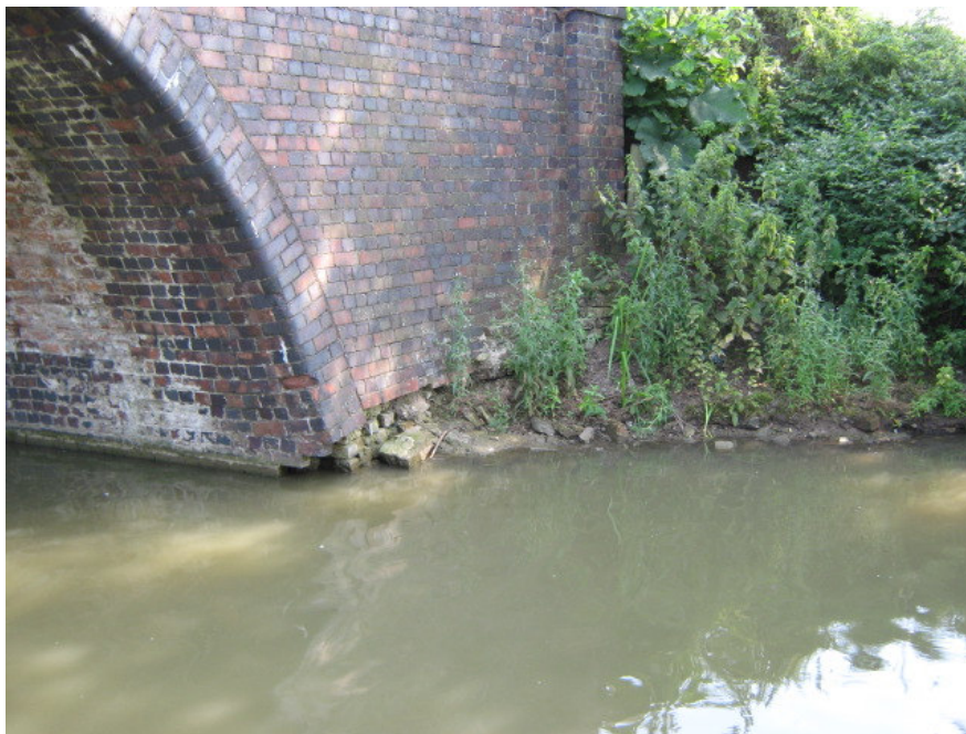
Bridge 27 Some repair work is needed at water level
