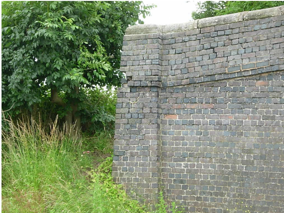
28 North Elevation The abutments and copings need major repairs
