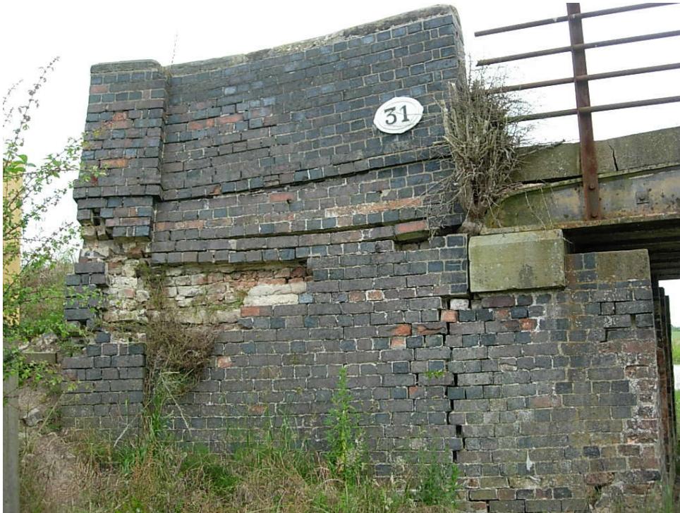
Bridge 31 Showing the parapet which has recently been taken down
