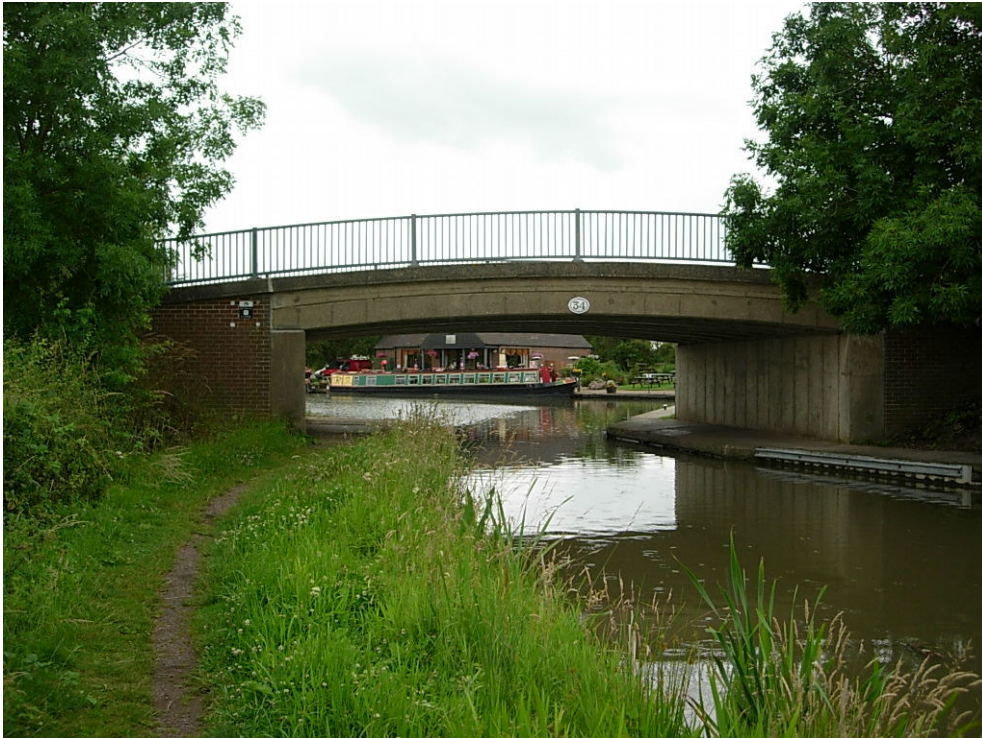
Bridge 34 (Sutton Wharf Bridge) South Elevation This concrete road bridge has steel railings. Although it is in good condition, its modern appearance detracts from the character of the canal at this very important location.
