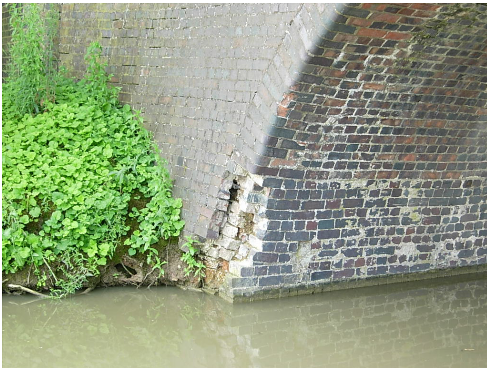
Bridge 30 The springing point of the arch is in need of repair
