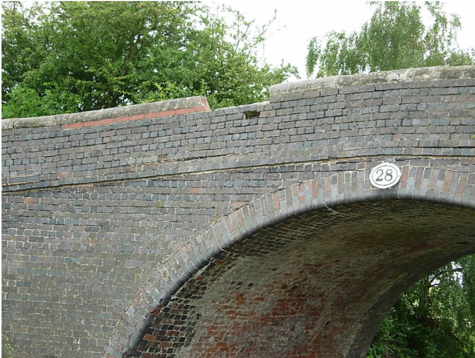
Bridge 28 (Dadlinton Bridge) North Elevation This bridge needs major repairs. The copings are a mixture of concrete and original stone
