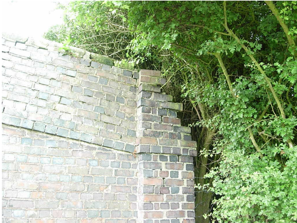
Bridge 29 North Elevation
