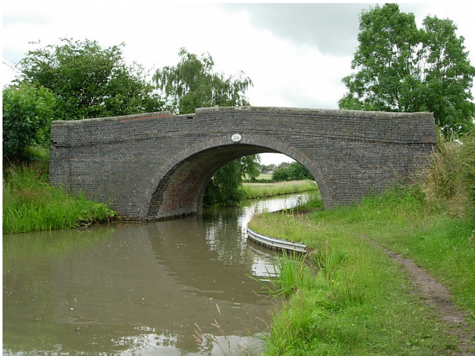
Bridge 28 North Elevation
