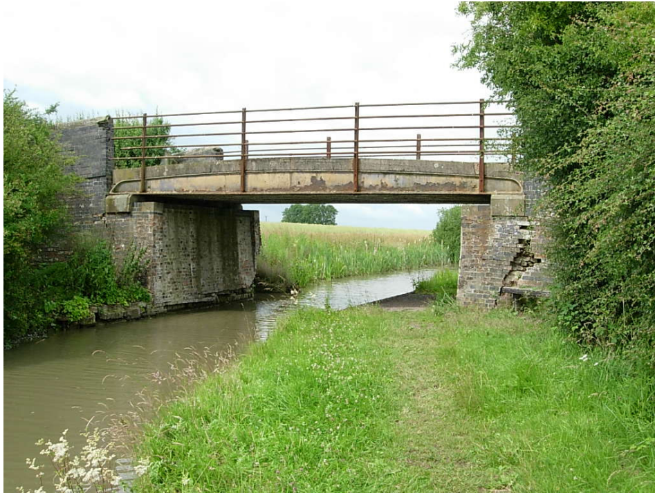
Bridge 31 ( Wooden Top Bridge) North Elevation The arch on this accommodation bridge has been replaced with a modern concrete and steel structure
