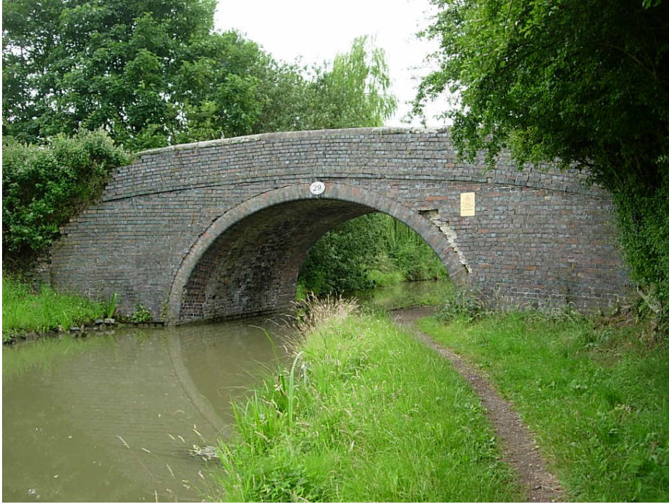
Bridge 29 (Allotments Bridge) North Elevation This private accommodation bridge is in poor condition and repairs are required to the brickwork
