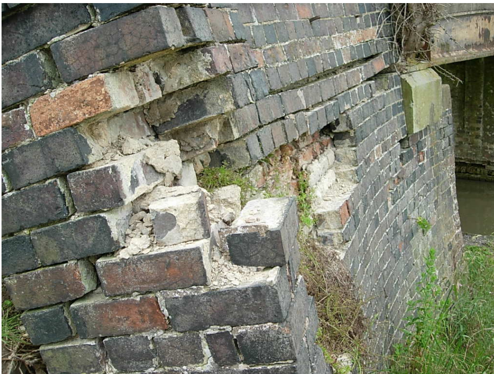
Bridge 31 The abutment requires major repair work
