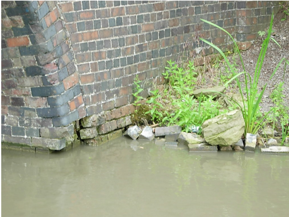
Bridge 28 Urgent repair works are required to the arches and abutments at water level
