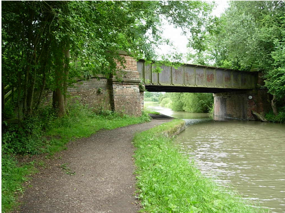
Bridge 34a South Elevation
