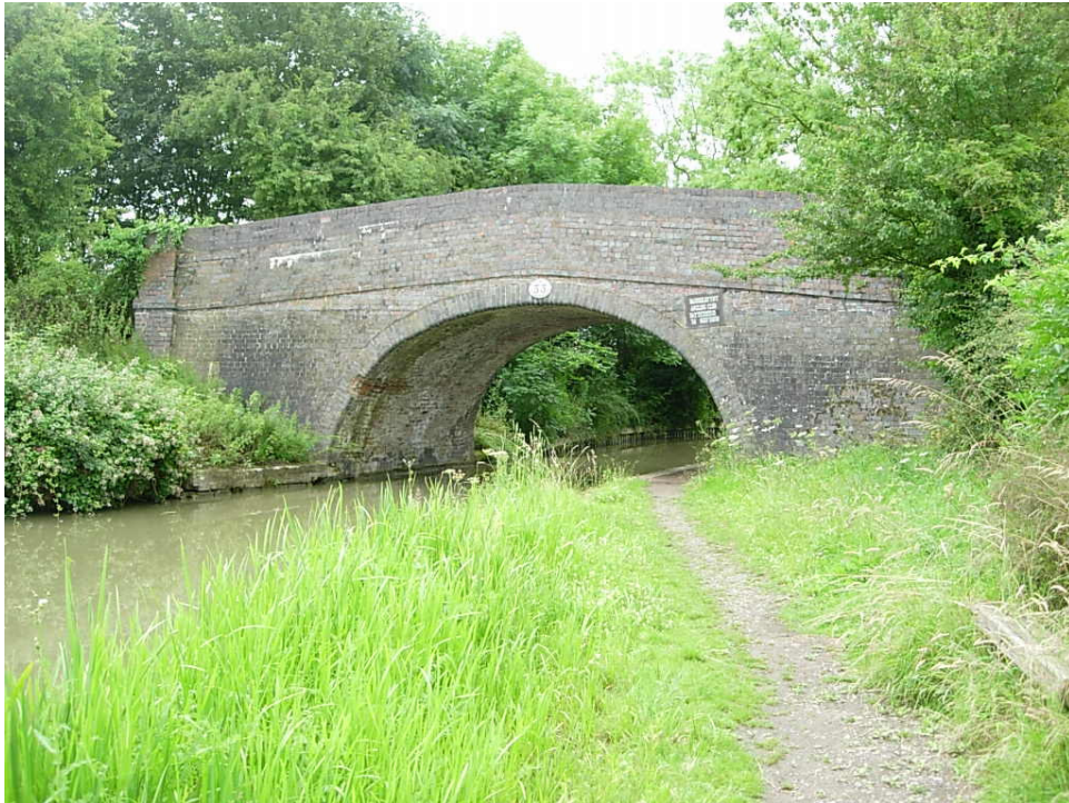
Bridge 33 (Geary's Bridge)North Elevation This brick structure has a modern brick soldier course to cap the parapets
