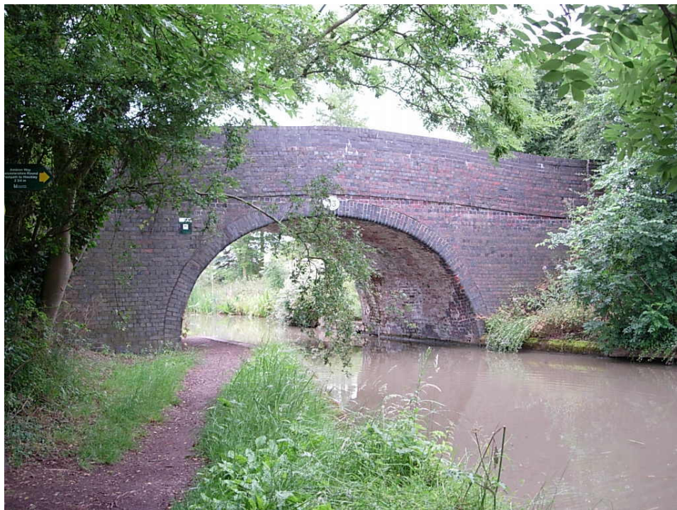
Bridge 33 South Elevation The brick arch is in need of repairs
