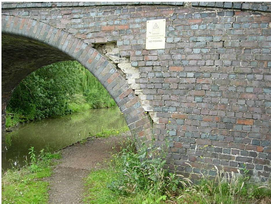
Bridge 29 North Elevation The abutments and parapets are in urgent need of repair
