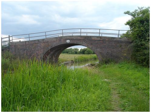
Bridge 39 North Elevation showing the detrimental impact of the railings
