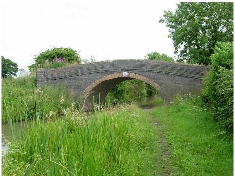
Bridge 36 North Elevation The north side of the bridge and arch needs re-pointing and half of the stone copings have been replaced with concrete copings.
