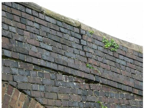
Bridge 36 South Elevation The crack in the brick parapet requires pointing and a section of concrete coping should be replaced with stone copings
