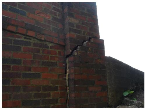
Bridge 40 There is a major crack in the abutments that has been re-pointed but movement is still recurring which has re-opened the fracture
