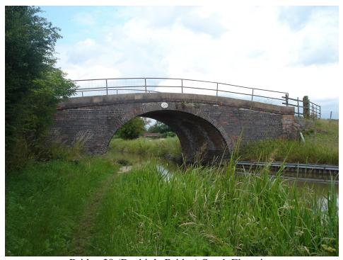
Bridge 39 (Deakin's Bridge) South Elevation This accommodation bridge has had its brick parapets removed and replaced with modern railings. These are unsightly and detract from its appearance. They should be replaced with brickwork to match existing brickwork.
