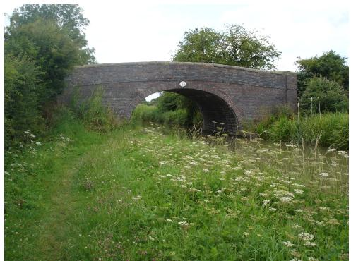
Bridge 38 (Fox Bridge) South Elevation A brick bridge in fair condition that has all its stone copings in place on brick parapets.
