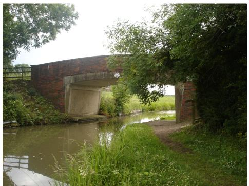
Bridge 40 North Elevation The bridge is built of red brickwork with concrete copings
