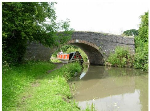
Bridge 36 (Hook's Bridge) South Elevation This Bridge is unusual in having a red brick arch with blue brick parapets and buttresses. The parapet needs repointing.
