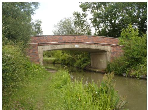
Bridge 40 (Coton Bridge) South Elevation The original brick bridge has been replaced with a concrete road bridge which out of character with the rural qualities of the canal.
