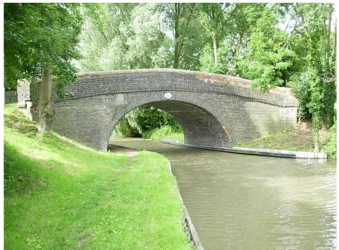
Bridge 37 (Welsboro Bridge) South Elevation This road bridge has been repaired with red brickwork that is out of character. The parapets are in need of re-pointing and concrete copings have mainly replaced the original copings. Part of the parapet has recently been badly damaged by a vehicle and needs re-building.
