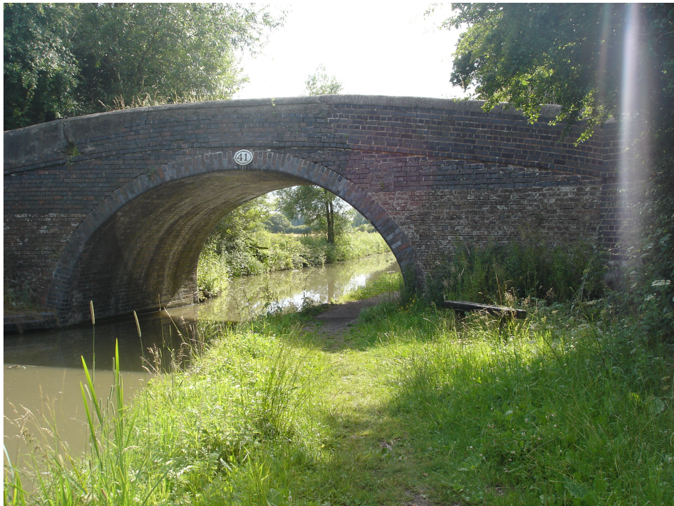
Bridge 41 North Elevation The poor repair work has had a detrimental impact on the appearance of the bridge All of the original stone copings have been replaced with concrete.
