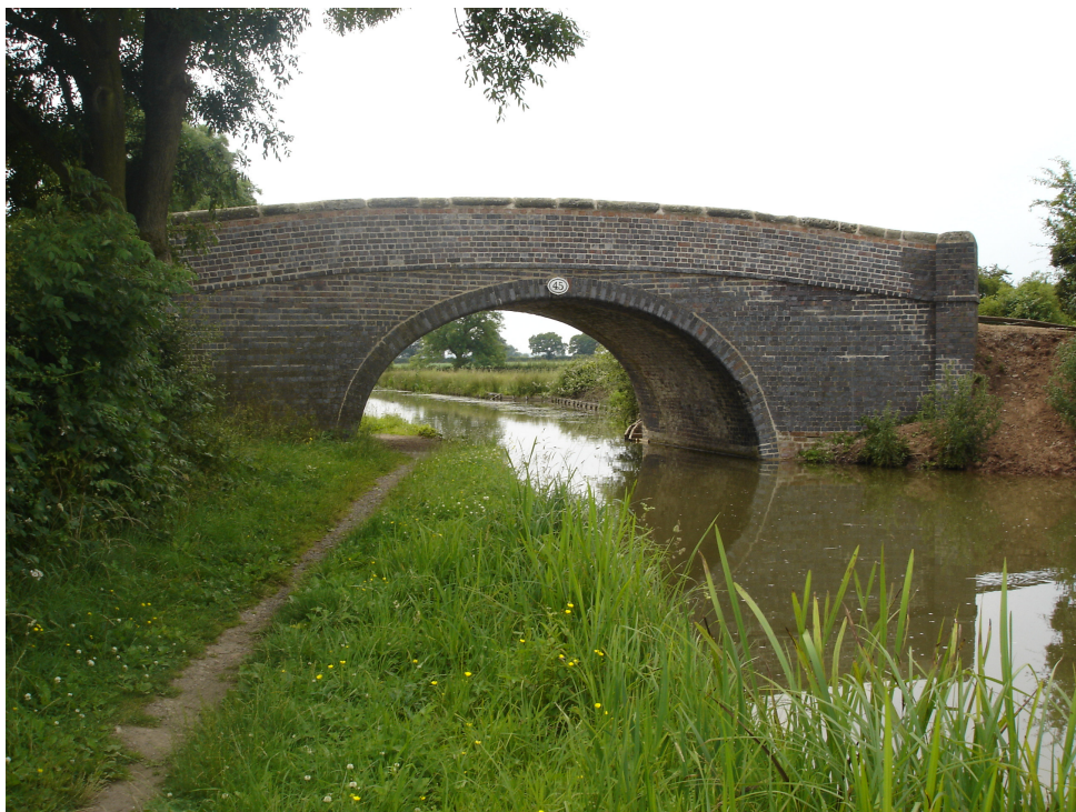
Bridge 45 South Elevation
