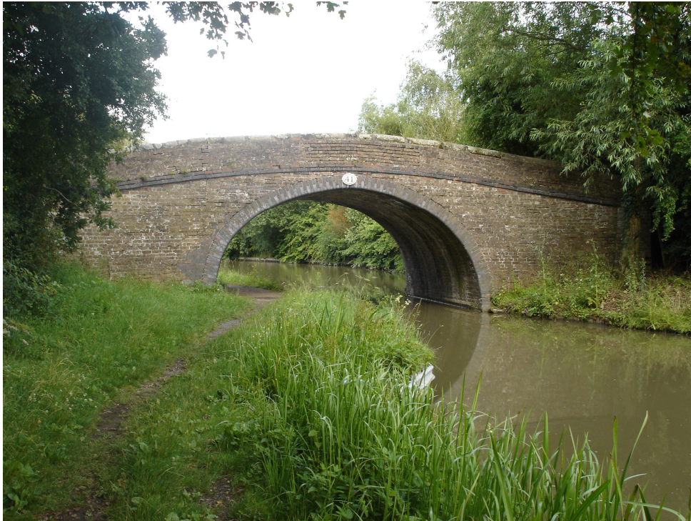
Bridge 41 (Jackson's Bridge) South Elevation
