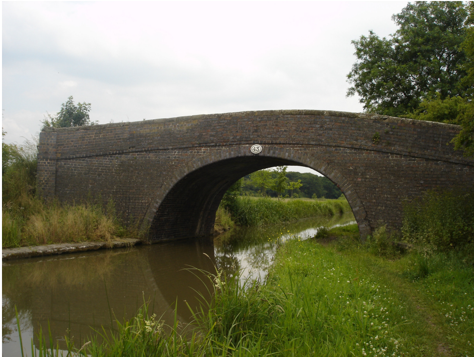
Bridge 43 (King's Bridge) North Elevation The Bridge is in good condition with all its original stone copings in place.
