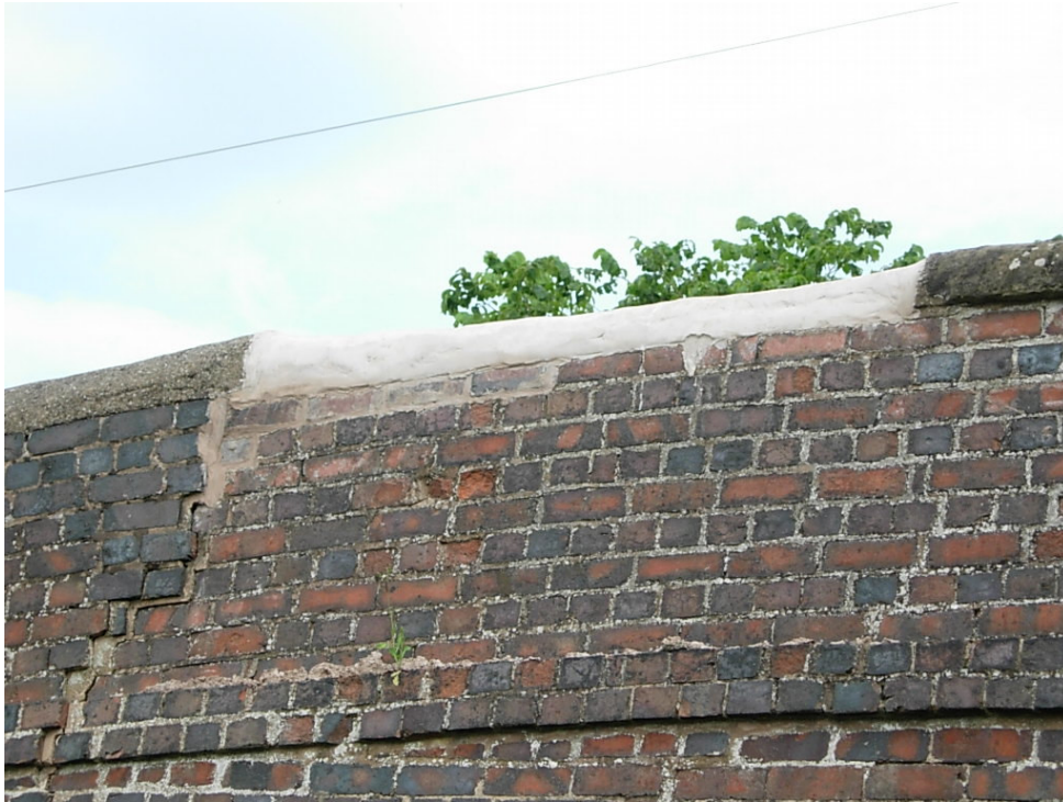
Bridge 46 showing the unsatisfactory repair to the copings. The stone copings have been replaced with sand/cement mortar which has a detrimental impact on its appearance. Work is also needed to repair the open joints on the parapet wall where the brick work has fractured
