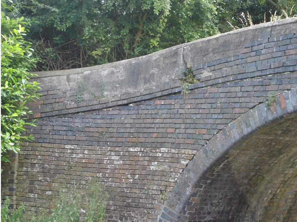
Bridge 41 North Elevation showing the settlement crack that needs attention
