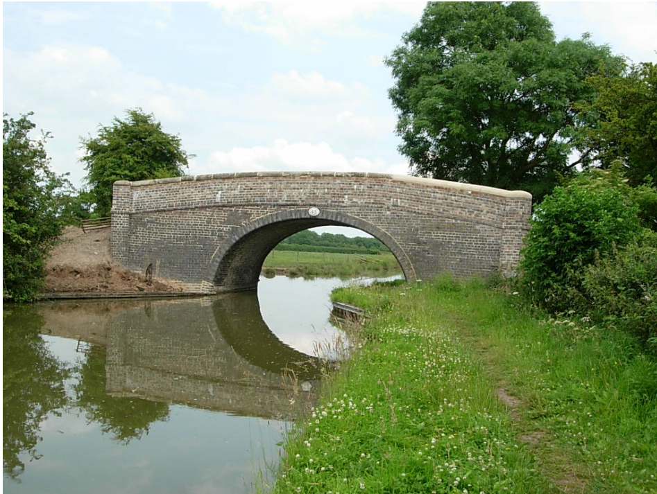
Bridge 45 (Iliffe Bridge) North Elevation
