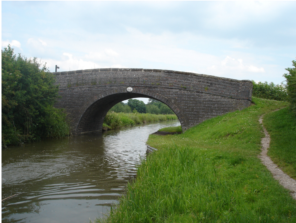
Bridge 44 (Carlton Bridge) North Elevation This road bridge marks the start of the canal's Site of Special Scientific Importance (SSSI) running northwards. The Bridge is in good condition with all its original stone copings in place.
