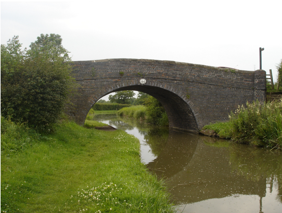
Bridge 44 South Elevation
