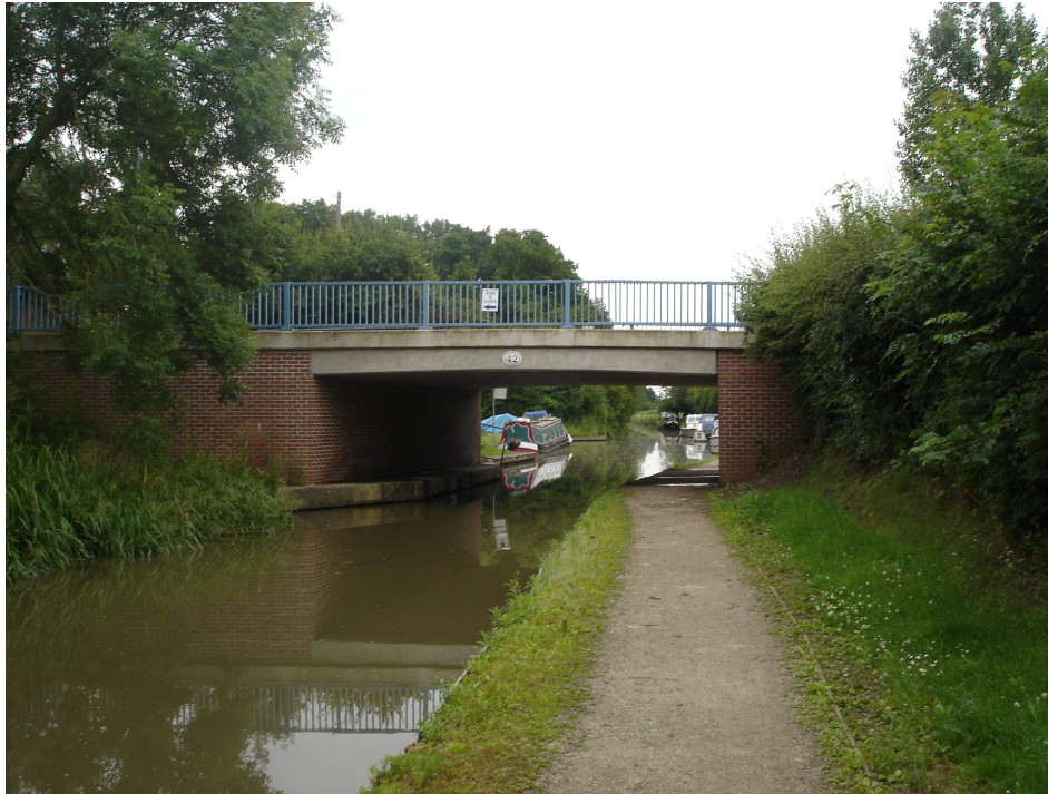
Bridge 42 (Bosworth Wharf Bridge) North Elevation
