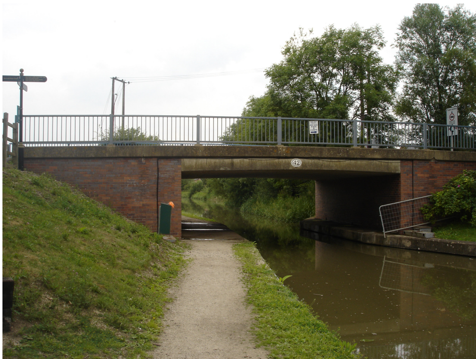
Bridge 42 South Elevation
