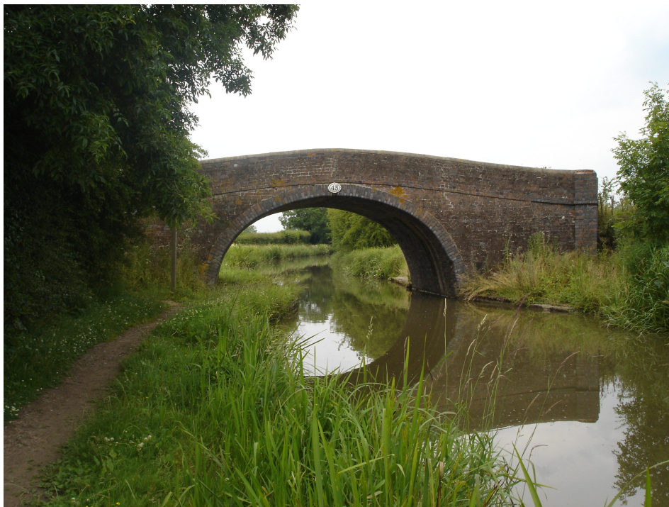
Bridge 43 South Elevation
