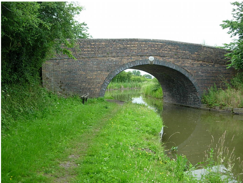
Bridge 46 South Elevation
