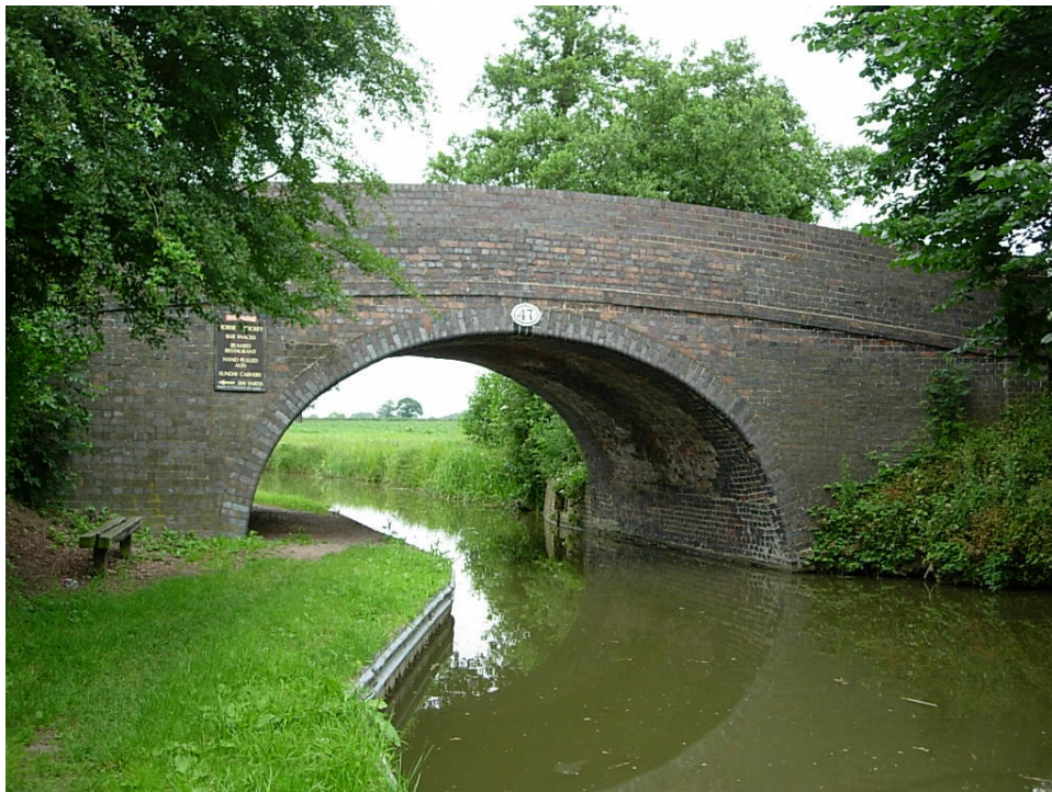
Bridge 47 South Elevation
