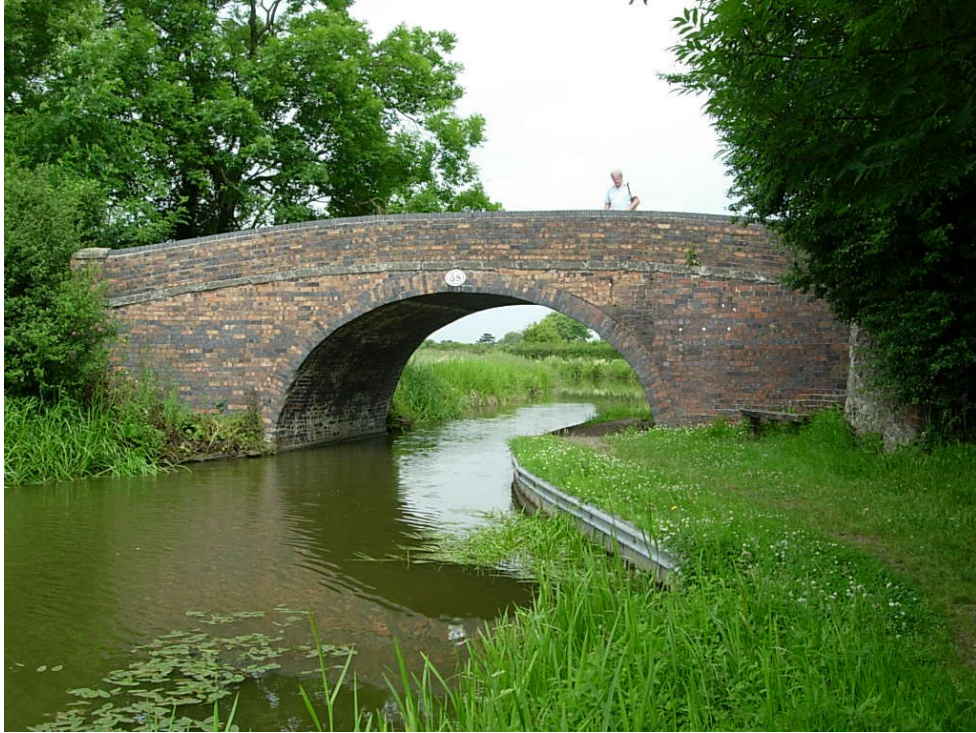
Bridge 58 South Elevation The bridge has previously been repaired and is generally in good condition
