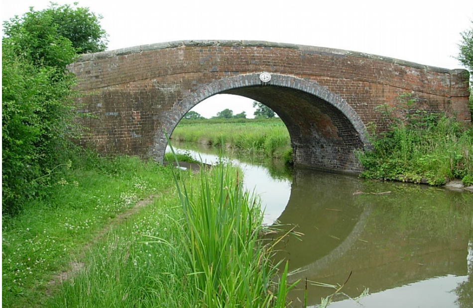
Bridge 48 South Elevation
