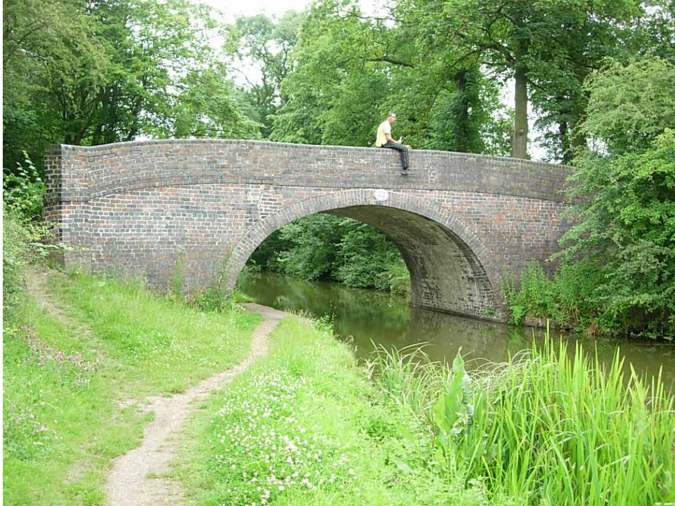
Bridge 57 North Elevation There is slight movement of the arch away from the parapet walls
