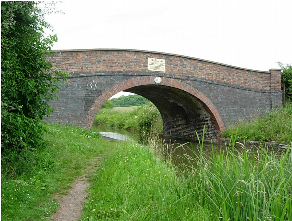
Bridge 51 South Elevation
