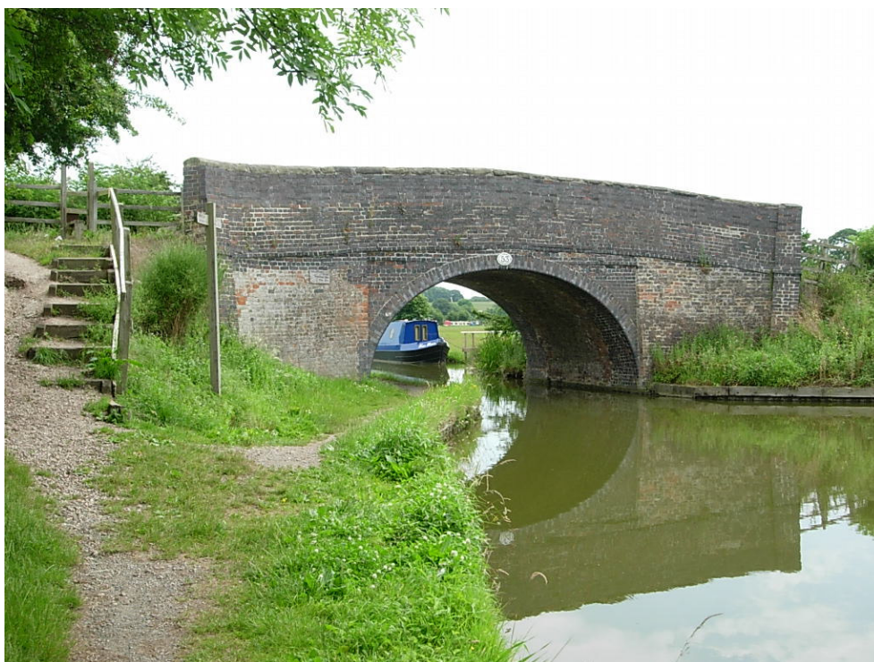
Bridge 53 (Town Bridge) North Elevation This road bridge has been repaired at various times in the past and is currently in good condition
