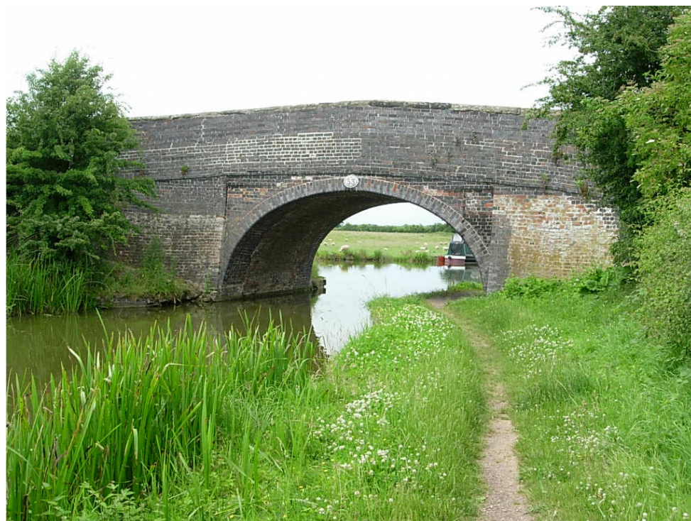
Bridge 53 South Elevation
