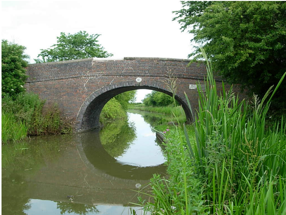
Bridge 46 (Fairfield Bridge) North elevation) A fine brick bridge which has retained the majority of its original stone copings. The bridge has been badly repaired in the past and work is now required to rectify this.
