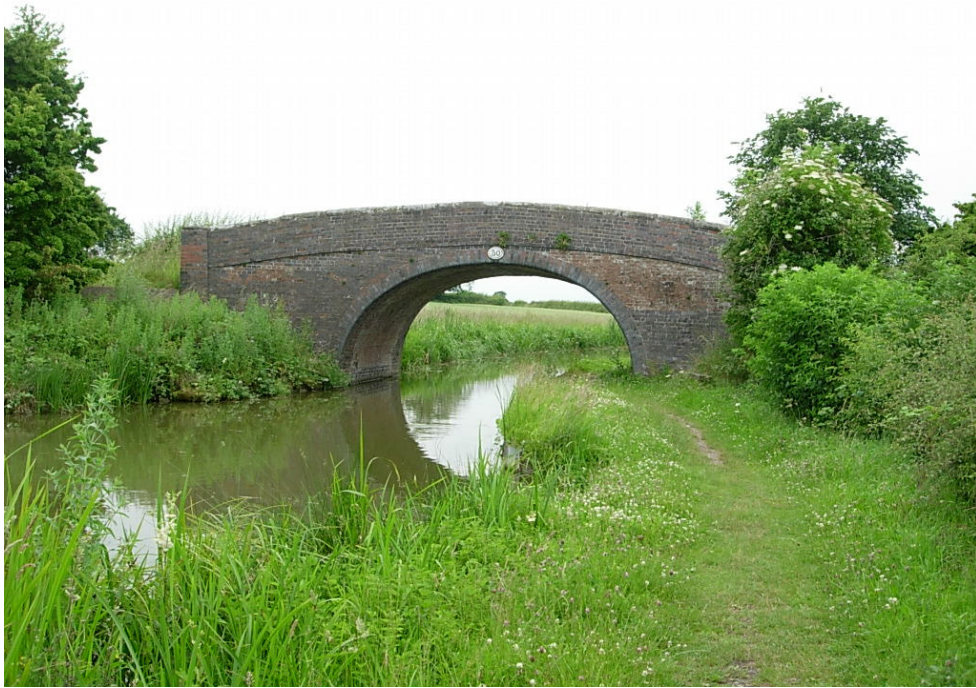
Bridge 50 (Bates Bridge) North Elevation This accommodation bridge is in good condition. Copings have been re-bedded.
