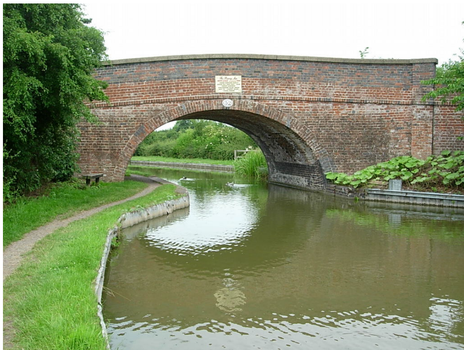
Bridge 52 South Elevation
