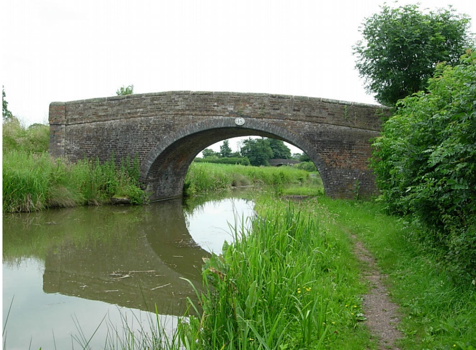
Bridge 48 (Dakins Bridge) North Elevation This road bridge is in fair condition, however, the springing points of arch are in need of repair
