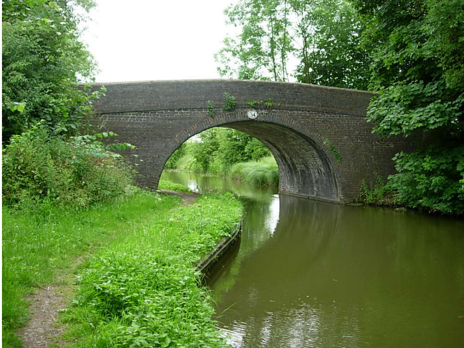
Bridge 54 (Hill's Bridge) North Elevation The Bridge is generally in good condition
