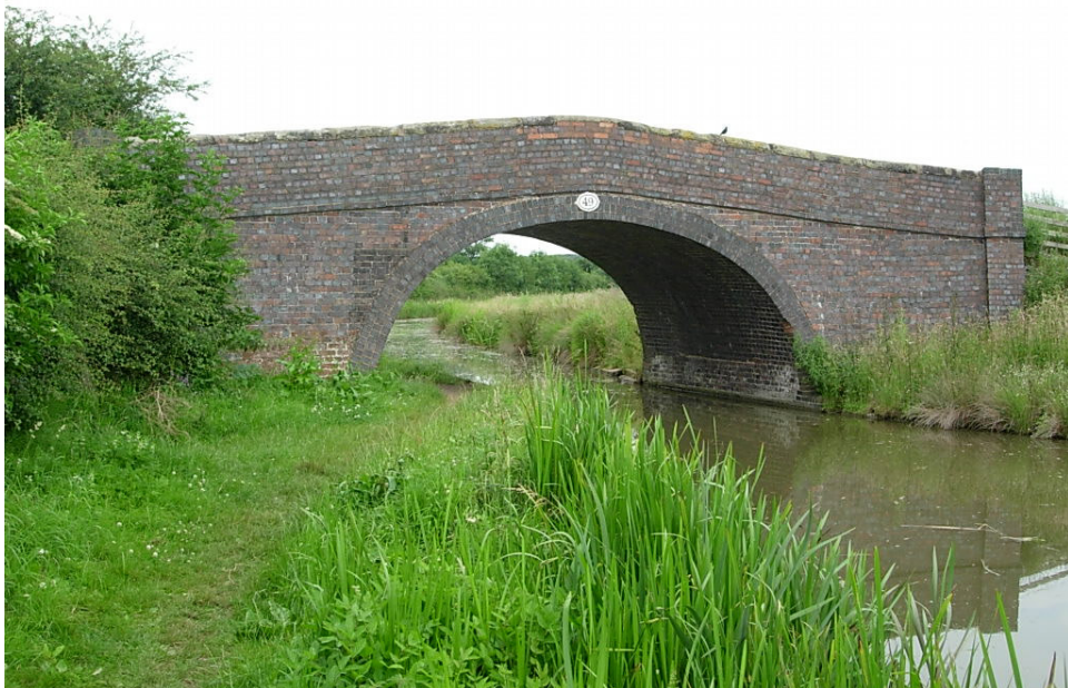
Bridge 49 South Elevation
