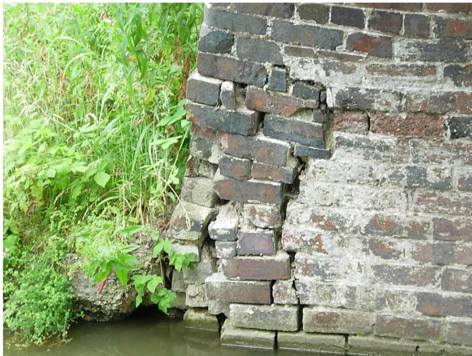
Bridge 48 showing the damaged brickwork requiring attention
