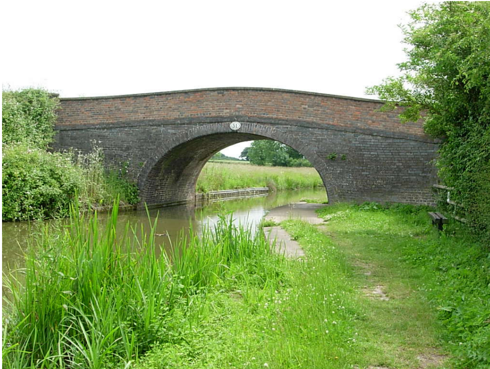
Bridge 51 (Bates Wharf Bridge) North Elevation The bridge which provides vehicular access along a public road to Shackerstone Station is generally in good condition. However, the parapet wall has been repaired in a non matching brick with concrete copings have been utilized.
