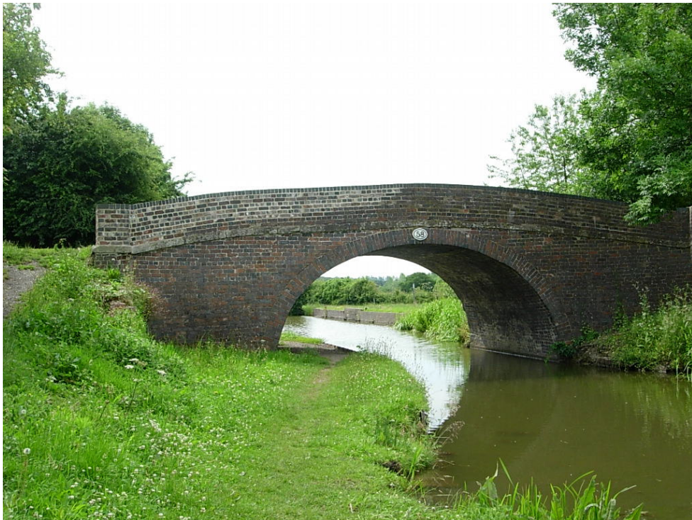
Bridge 58 North Elevation
