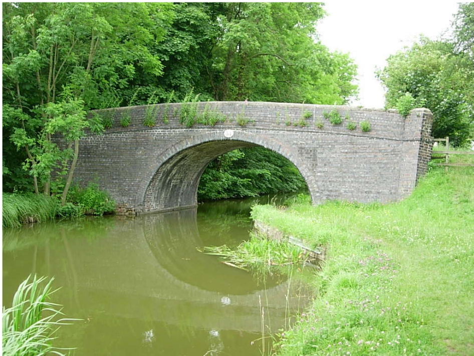
Bridge 54 South Elevation Vegetation should be removed and parapets repointed
