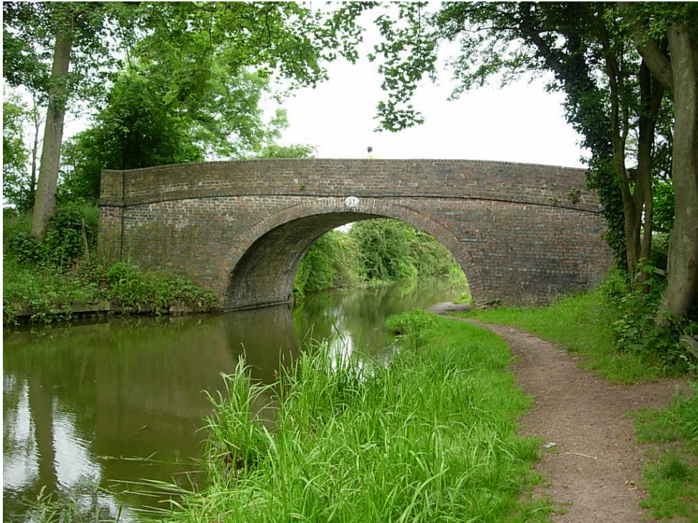
Bridge 57 South Elevation
