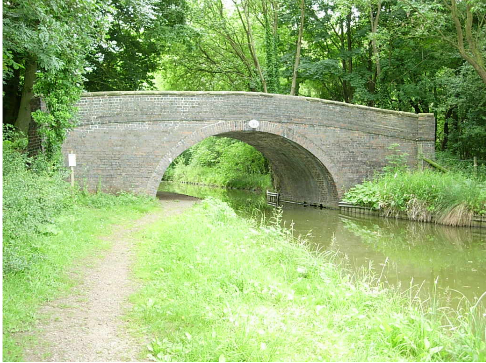
Bridge 56 : (Timms Bridge) North Elevation The bridge is generally in good condition
