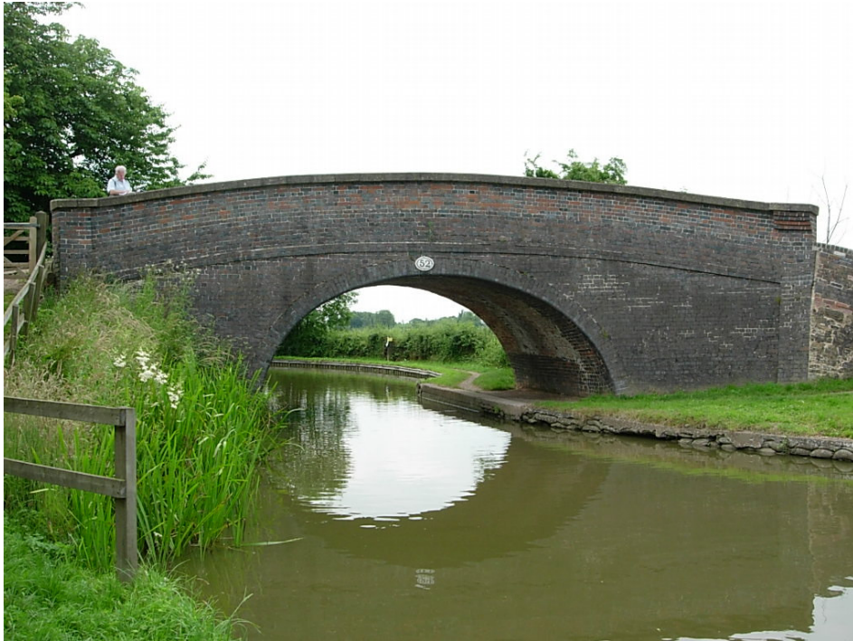
Bridge 52 (Turn Bridge) North Elevation
