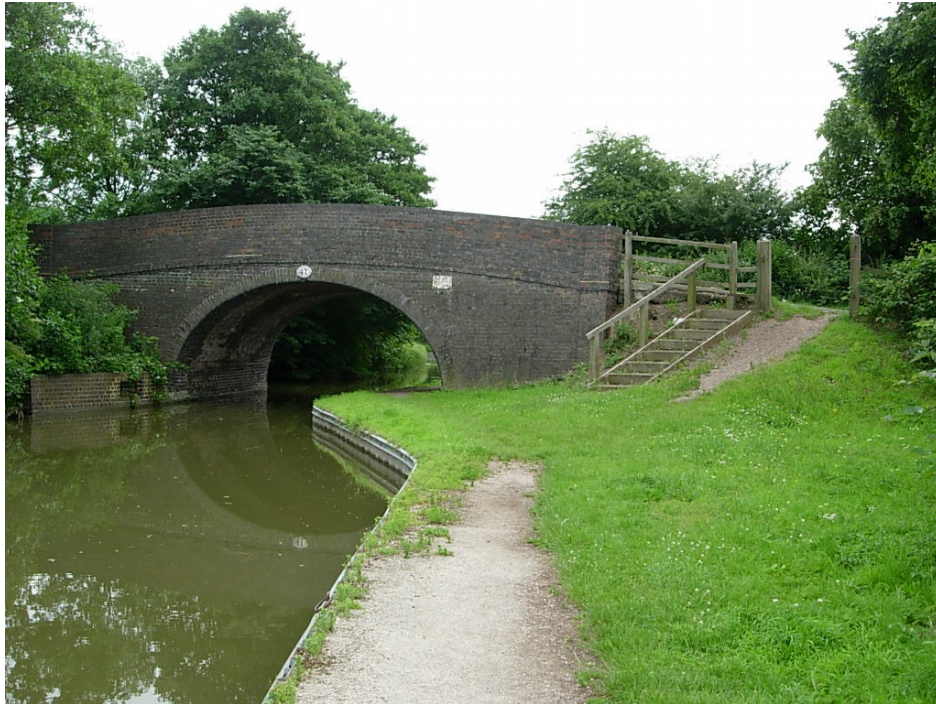
Bridge 47 (Congerstone Bridge) North Elevation This road bridge is in good condition
