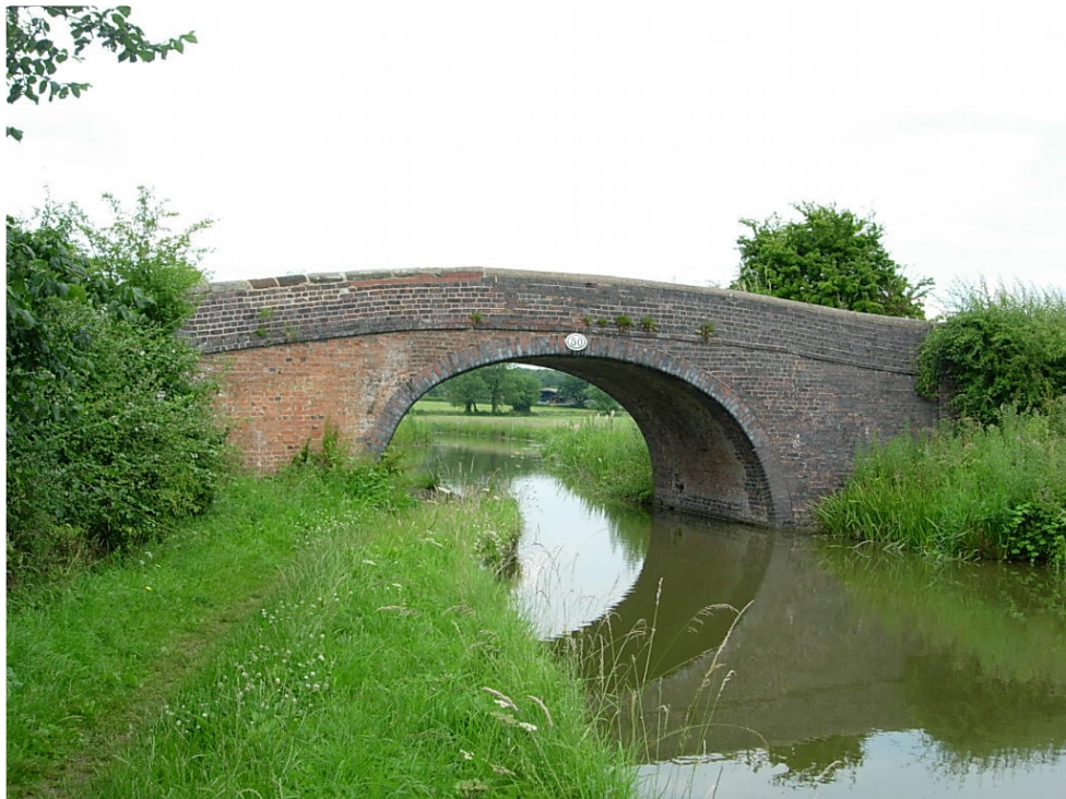
Bridge 50 South Elevation Repairs have been unsympathetically completed in none matching brickwork
