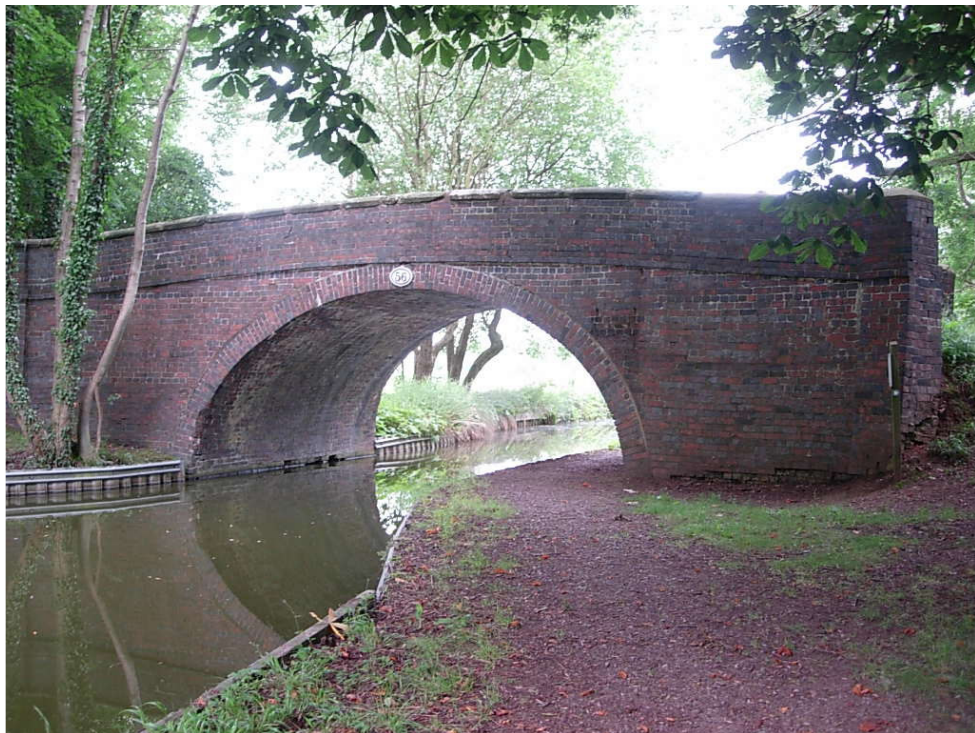
Bridge 56 South Elevation
