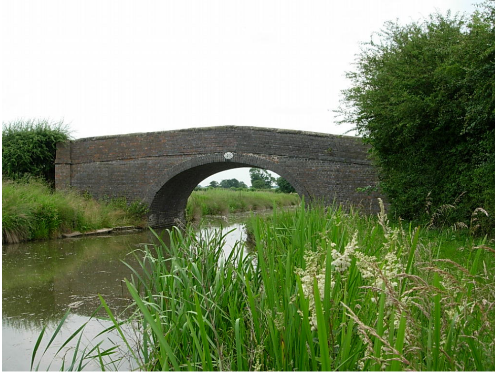
Bridge 49 (Terrace Bridge) North Elevation This road bridge is in fair condition, however, the springing points of arch are in need of repair
