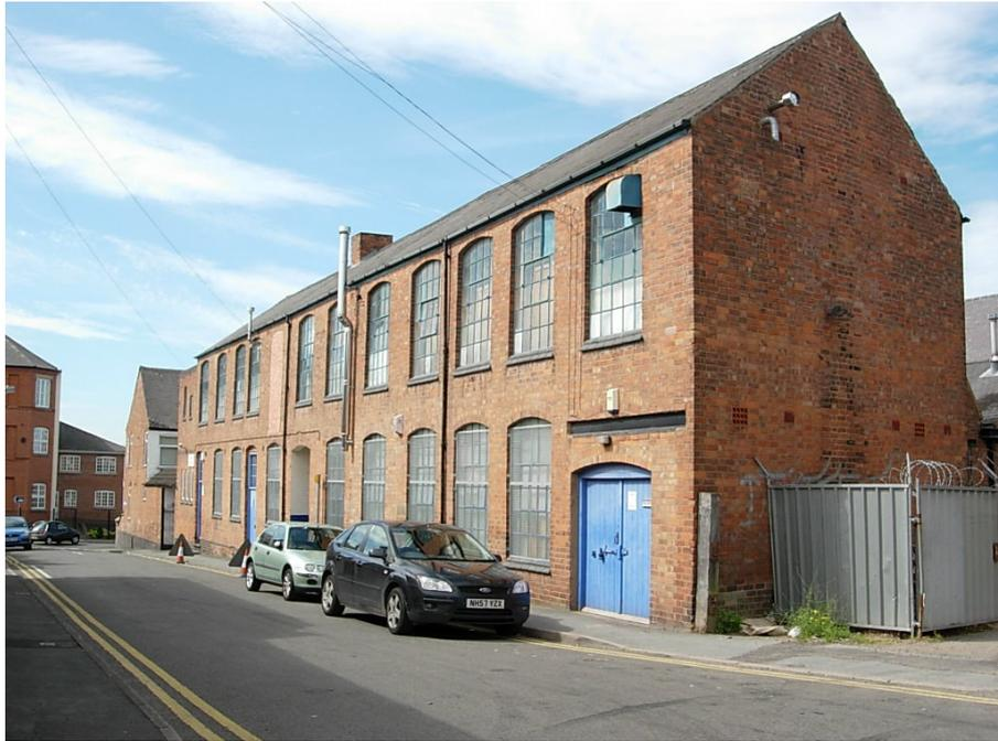
The former Amos Moore factory is one of the better examples of boot and shoe factories in the area. It has retained its original cast iron windows and slate roof covering. This company was one of the earliest shoe manufacturers in Barwell.
