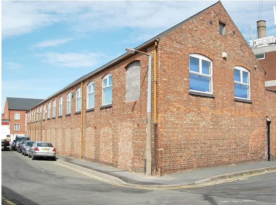
This part of the Harvey, Harvey & Company factory fronts George Street. Unfortunately its original cast iron windows have been replaced with plastic of inappropriate design. Those on the ground floor have been blocked up. This has a detrimental appearance on the conservation area.
