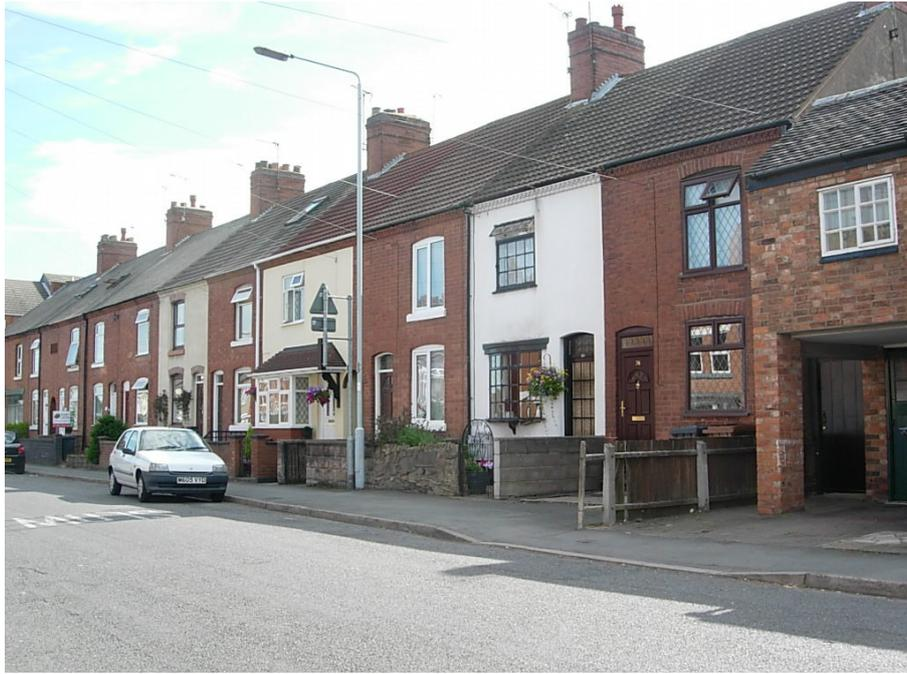
The southern end of the same terrace which has suffered from inappropriate features such as concrete roof tiles and bow windows.
