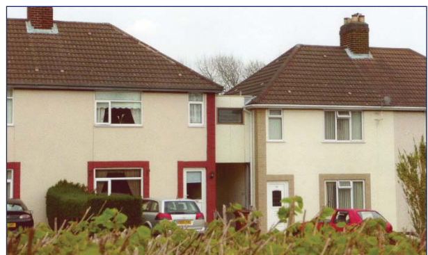
Semi-detached houses showing 'bridge' bathrooms matching adjacent rendered walls, Markfield Road
