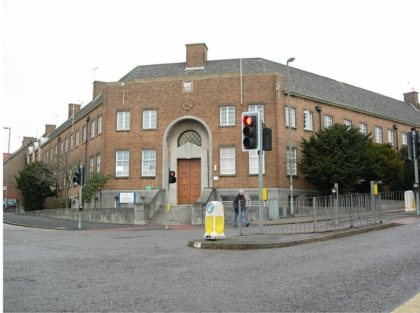
Hinckley Police Station in the Art Deco style. This important building dominates the road junction of Hollycroft with Bond Street.
