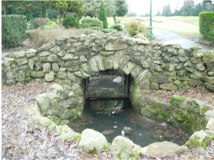
This pond collects water from an artificial stream which is then re-circulated by water pump. The stream is an original feature of the park.
