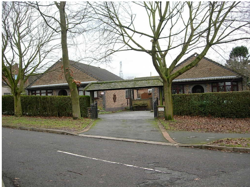
29 – 31 Westray Drive. These houses also have limited impact, being well set back behind the garden hedge.
