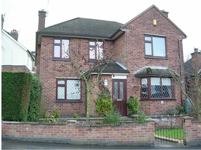
27 St. George's Avenue. The modern window sub-divisions on this property detract from its appearance.
