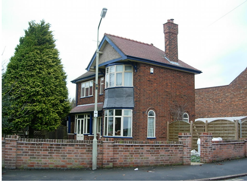
9 Shakespeare Drive. This property on the corner of Canning Street has recently had its garden wall rebuilt. The curved top fence panels are out of character.
