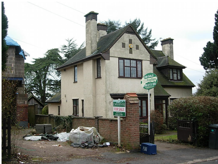
21 St. George's Avenue. The side garage is set well back to avoid impacting on the space between buildings. The vehicular street entrance has also been kept to a minimum.
