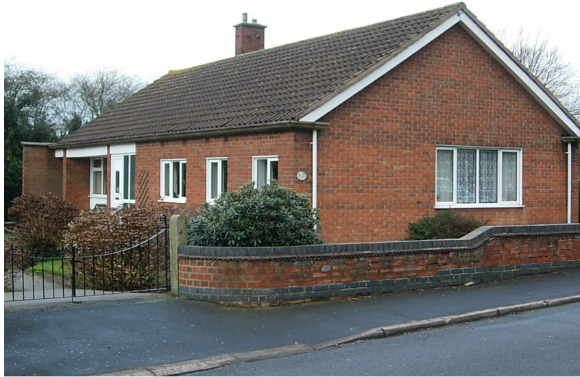
30 St. George's Avenue. This property has limited impact on the street scene because it is set back behind a low brick wall.
