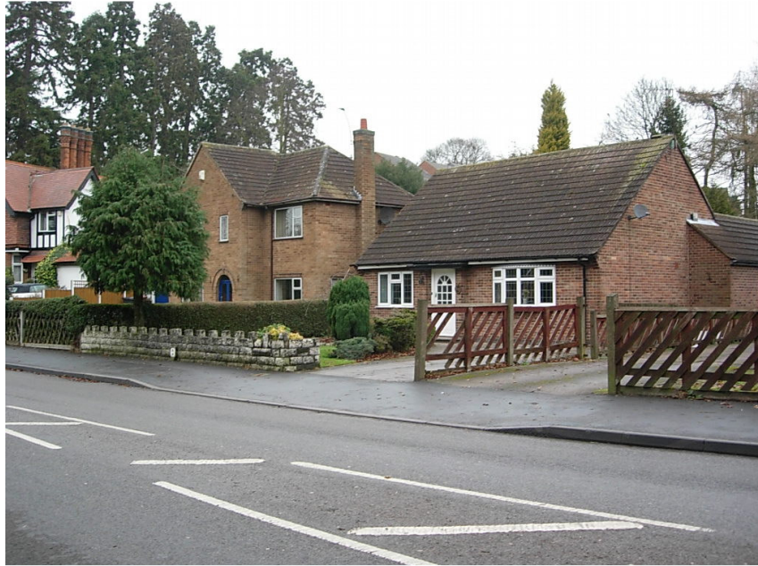
45 – 56 Hollycroft. The reconstituted stone wall is out of character with the other walls in the conservation area.
