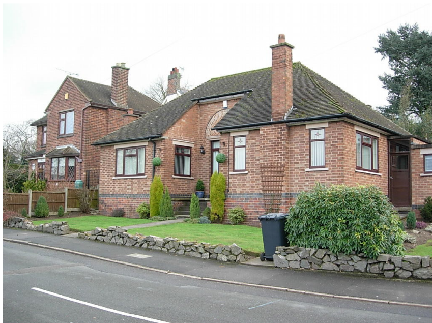
29 St. George's Avenue. The stone wall fronting this interesting property detracts from its appearance and character of the conservation area. It should be constructed of brickwork and is too low.
