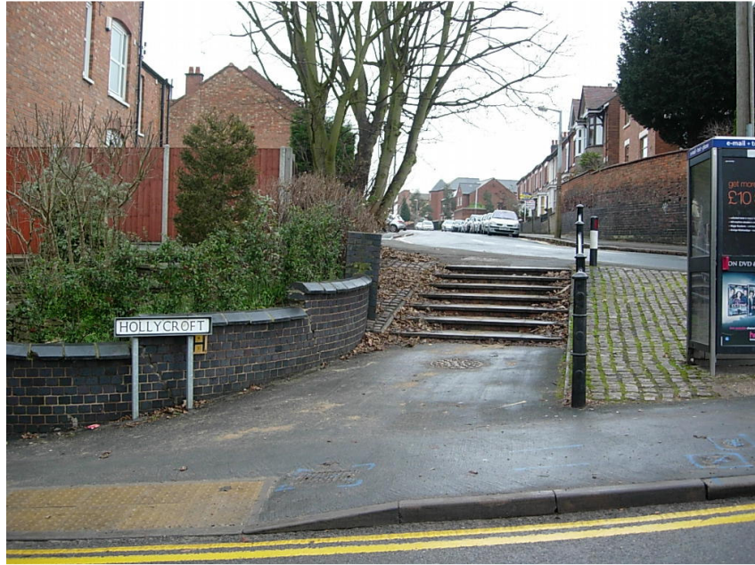
This area at the junction of Hollycroft and Factory Road has been improved and re-surfaced by the council.
