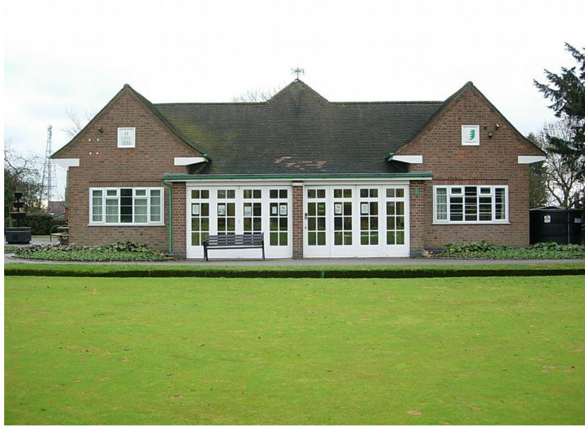
The modern French window double screens have had a detrimental impact on the appearance of the park's bowling green pavilion.
