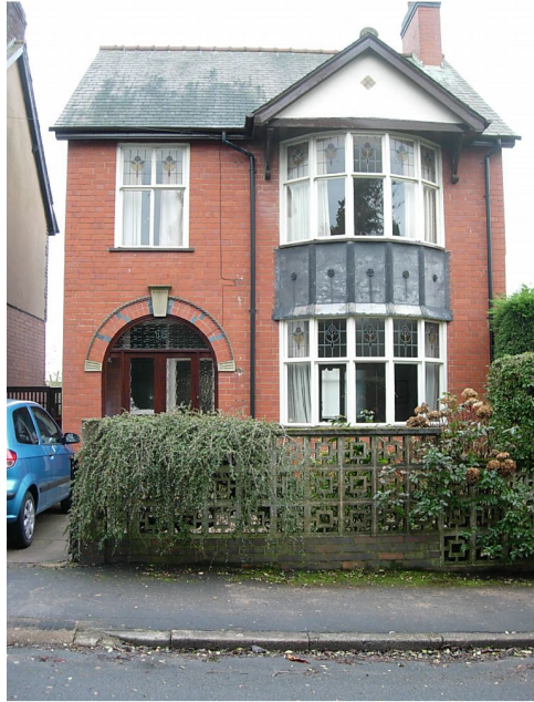
15 St. George's Avenue. The street frontage opening to this property has been kept to a minimum.
