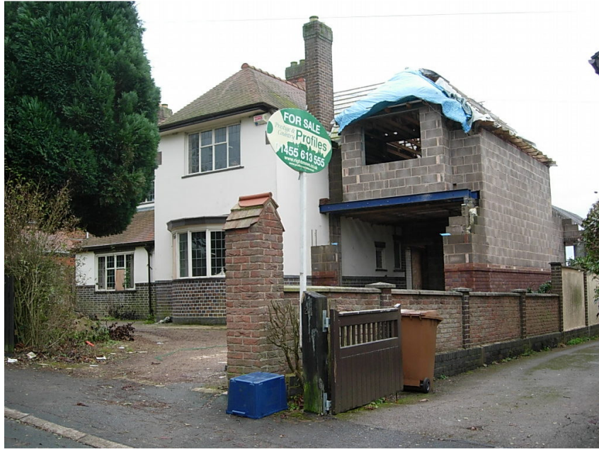
19 St. George's Avenue. The low level brick plinth has been carried around the new side extension which has also been set back to avoid dominating the principle façade.
