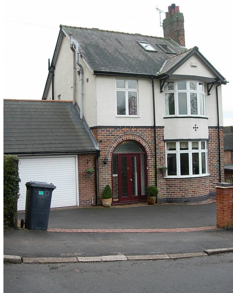
25 St. George's Avenue. The garage roof and door are out of scale with other features on this property.
