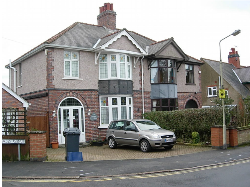
1 – 3 St .George's Avenue. This property, although well maintained, has lost most of its garden wall which impacts on the street scene. The gable bargeboard is also out of character.
