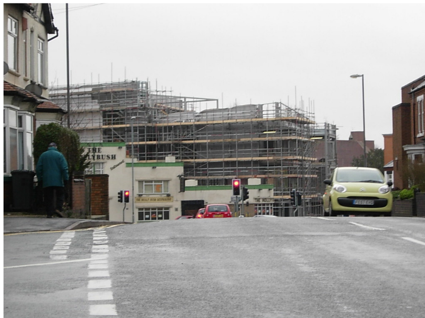
The recent demolition of the 1970's extension to the Atkins factory has enabled a new view of the Unitarian Chapel to be created.
