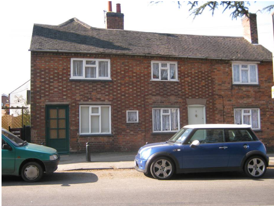
The decorative pattern on the front elevation of 15 & 17 Hinckley Road has been achieved utilizing brick headers. It is unfortunate that the traditional brick arches have been replaced by concrete lintols above the windows and doors.
