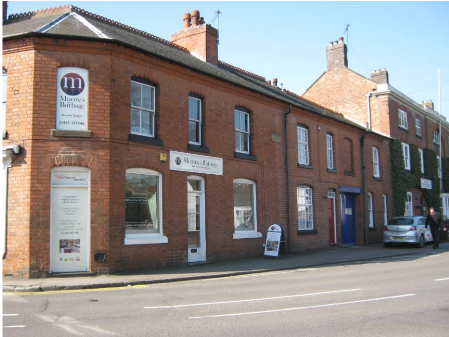
Looking north westwards along Church Street. The terrace has retained its historic features including the segmental lintols, sash windows, slate roof finish, decorative ridge tiles and facing brickwork. This has had a major impact on the street scene and the unity of the terrace.
