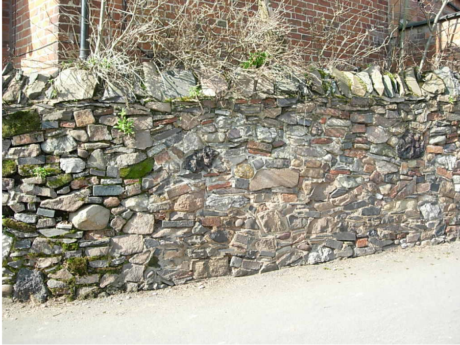
The textured face of this fine stone wall sited at the side of The Croft on Church Street adds character to this part of the conservation area.
