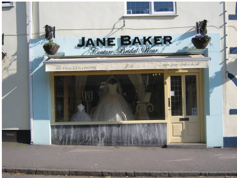
The shop front to these premises has been built in the art-deco style which is in conflict with the appearance of the traditional retractable canopy.
