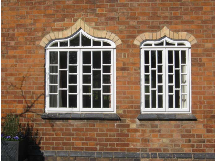
The different design of traditional windows adds interest in conservation areas. These timber windows with ogee heads are on the Grade II listed property 28 Church Street. The original windows were cast iron.
