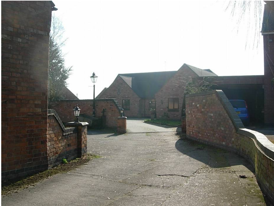
Although two modern dwellings are accessed from this private drive, being set well back from the carriageway, their visual impact on Aston Lane is negligible
