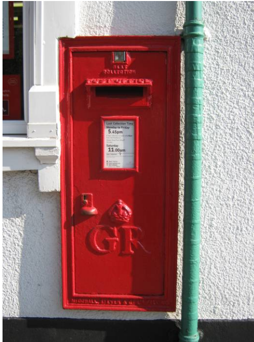
This cast iron George VI post box is an interesting feature sited in the wall of the post office which should be retained.
