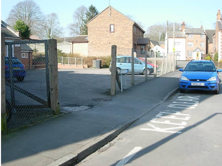
The concrete post & wire fence along the Burbage Congregational Church's frontage should be replaced with a wall or railings in keeping with the traditional character of the conservation area.
