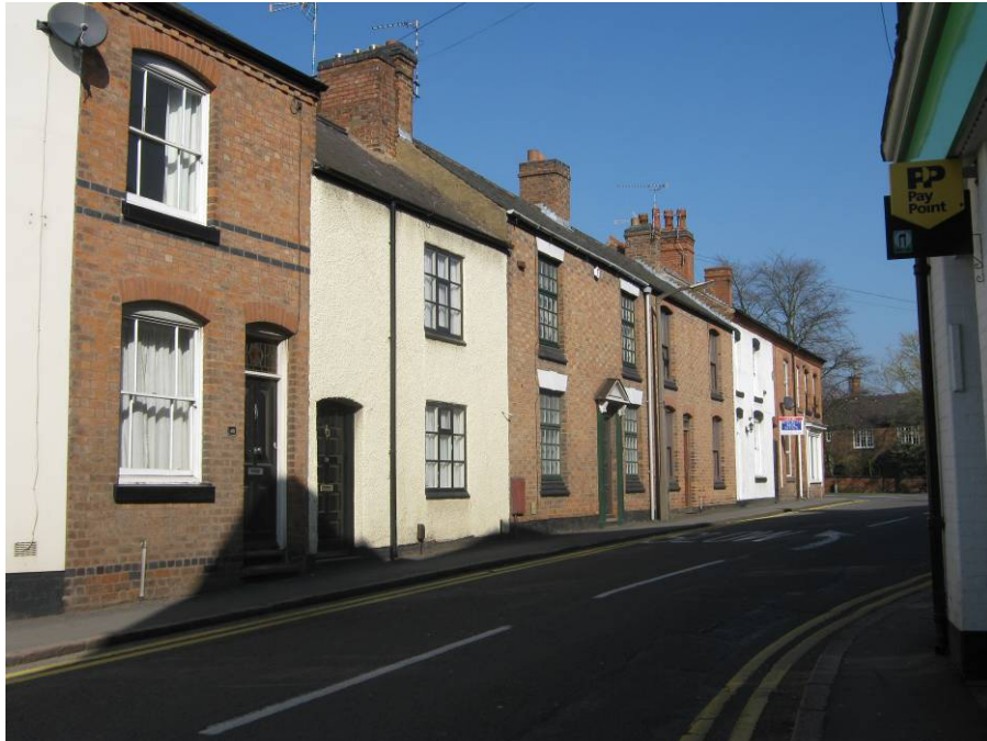
The unity of the terrace on the west side of Church Street has been lost due to the rendering and modernization of several properties. However, this length of the road still retains its granite kerbs.
