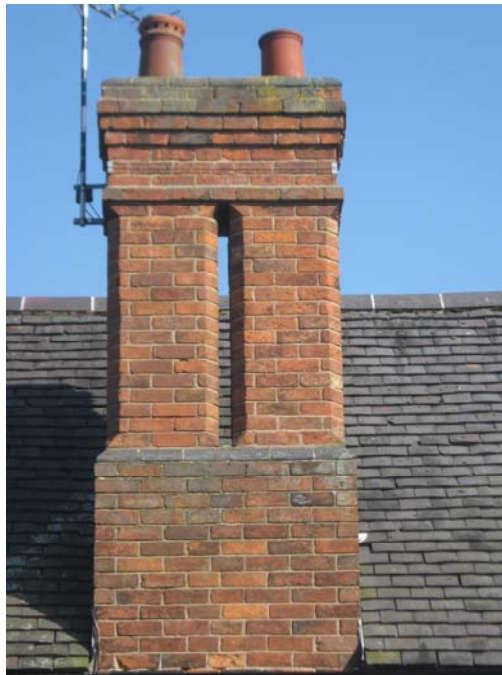
This eye catching chimney is on the Grade II listed dwelling, 28 Church Street.
