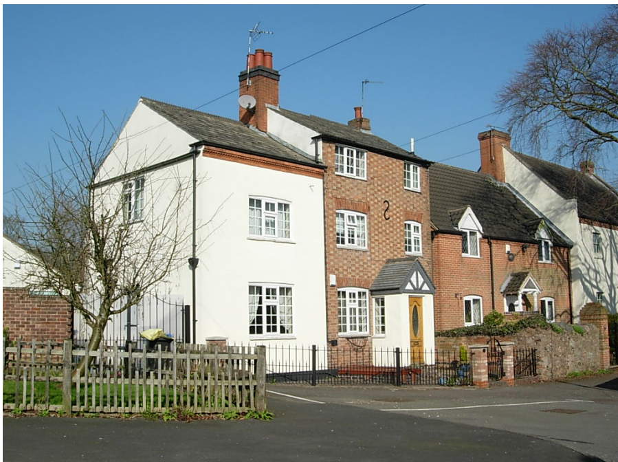
Interest in this group on the Horsepool is achieved by the variation in roof heights and choice of materials. It is not a terrace, but a collection of attached properties.
