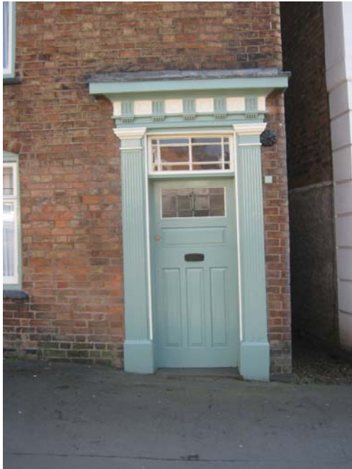
There are a number of attractive front doors scattered around the conservation area; this one is at 77 Church Street.
