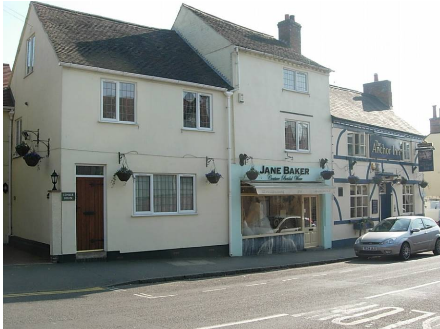
63-67 Church Street is a pleasant block of properties dominated by the 3-storey shop.
