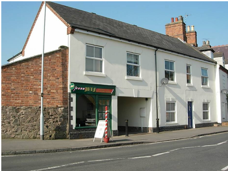
This modern property, 2 & 2a Church Street blends in with the rest of the block. The shop front is in scale. Unfortunately, the chimney stacks are missing. The impact of changes on the unity of the terrace should always be carefully considered particularly in conservation areas where the street scene is particularly important.
