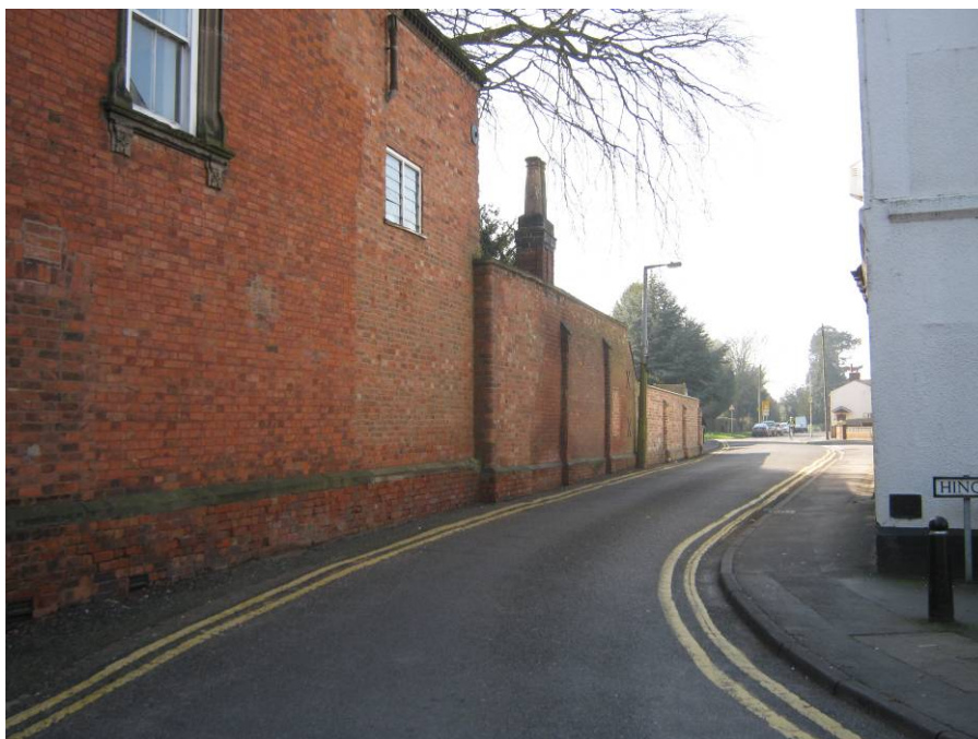
View looking westwards along Grove Road. The high brick wall is an important feature in the conservation area.
