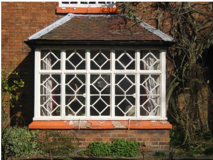
One of a pair of hipped-roof square bays on the front elevation of the Manor House showing the lozenge glazing.
