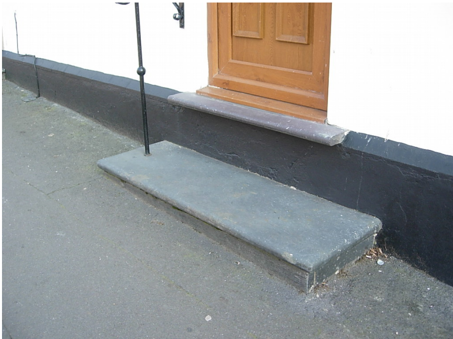
Slate steps fronting dwelling on Church Street are a traditional feature of the conservation area.
