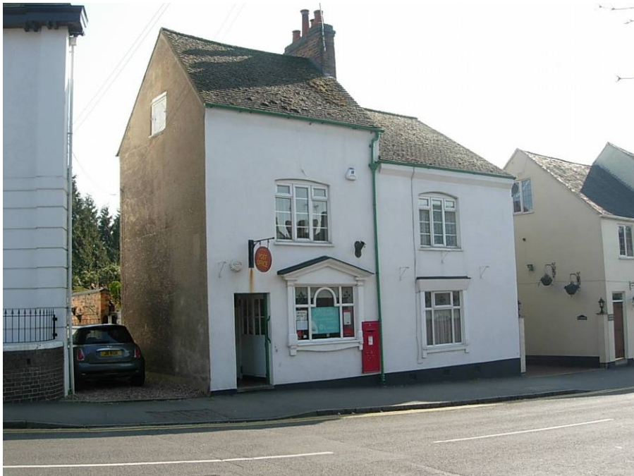
Although 71 Church Street has been converted to a post office and its shop front is overly decorated and it has lost its second floor window. However it is not over prominent in the street scene.
