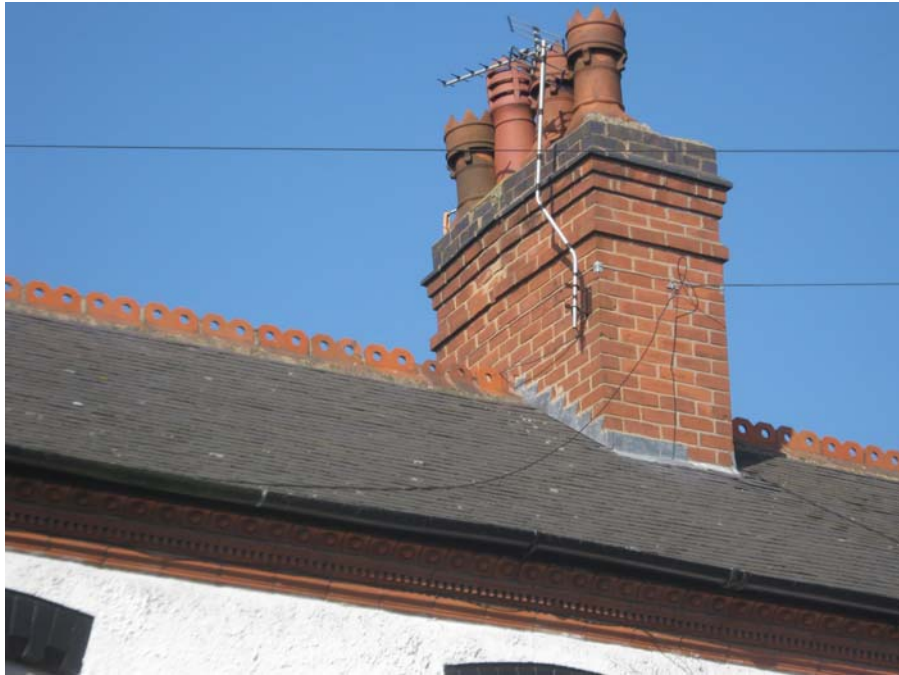
Chimney stacks and pots play an important role in the traditional character of conservation areas.
