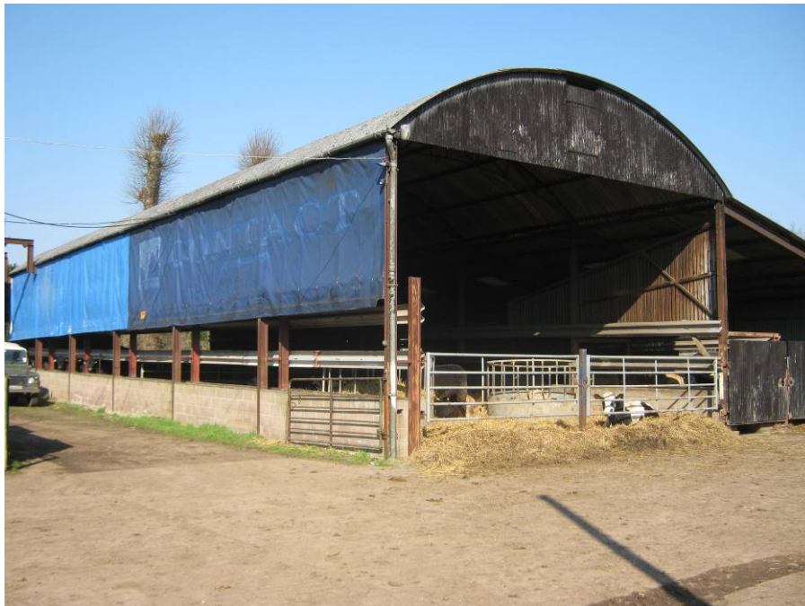
This large Dutch barn is an imposing structure at Manor Farm. These buildings, once very common, are increasingly being demolished and are becoming rare. Further losses should be avoided.
