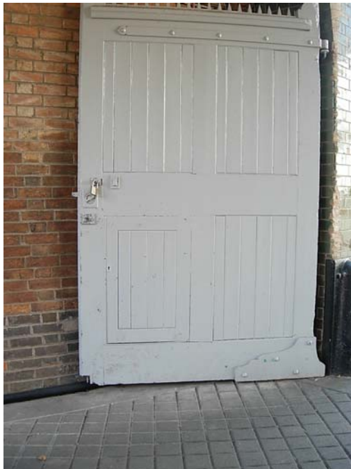
This hefty timber door is sited at the archway leading to the rear of the Co-operative store.
