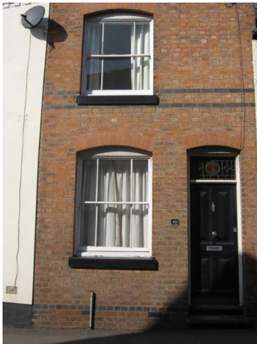
Sash windows are also important features in conservation areas that sadly are being replaced by modern plastic windows.
