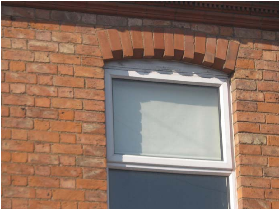
The saw tooth lintel on this property is a traditional detail which adds to the character of the property.
