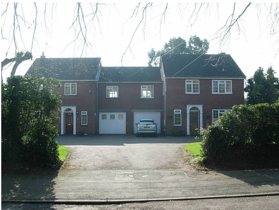
These large properties, 2 & 4 Aston Lane unfortunately do not respect the traditional character of Aston Lane by way of their design, use of modern materials and siting. By being sited well back from the carriageway, enclosure on the lane has also been lost.
