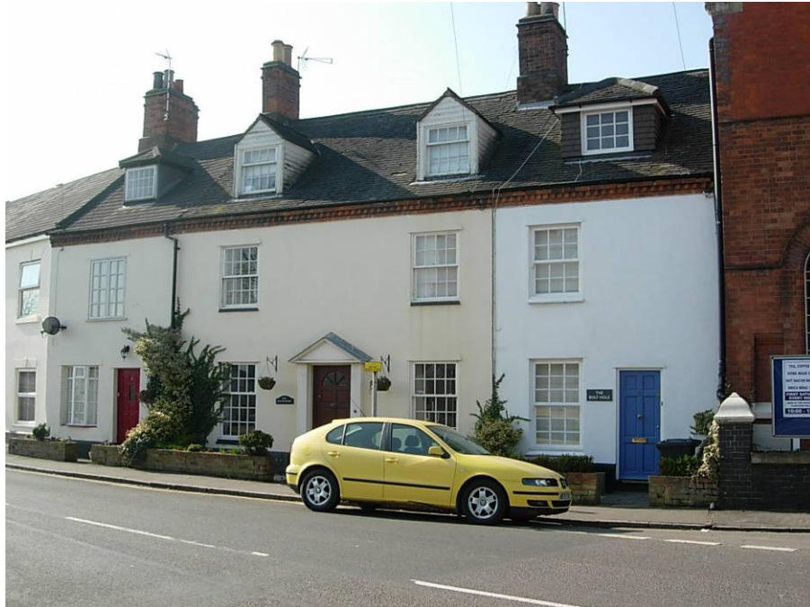
This attractive group of dwellings; 6-10 Church Street still retain their impressive chimney stacks and pots. Unfortunately the original cast iron railing which fronted the properties have been lost.
