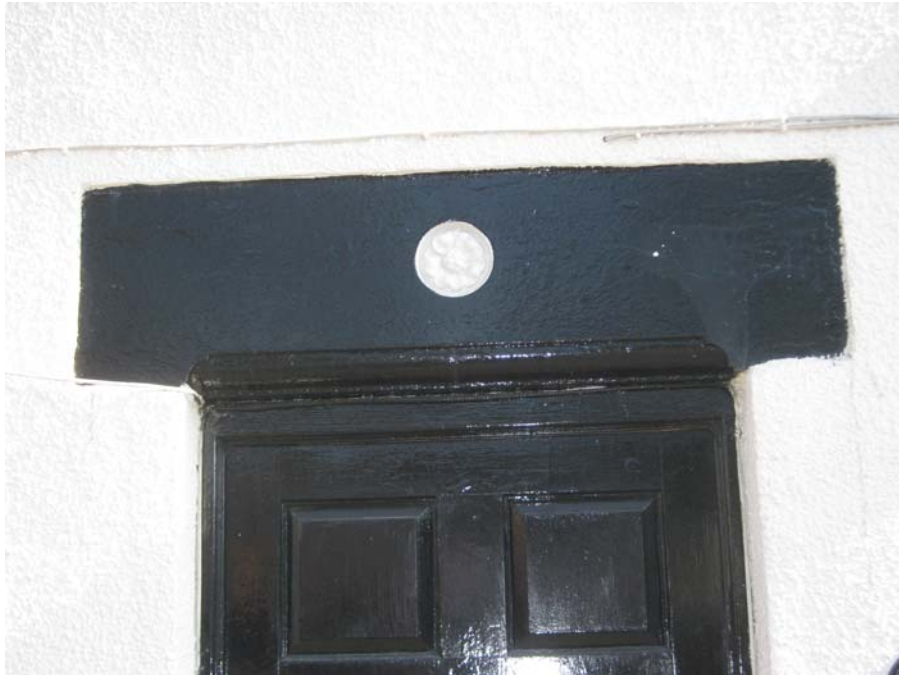
Lintols also contribute to the character of the Burbage Conservation Area.
