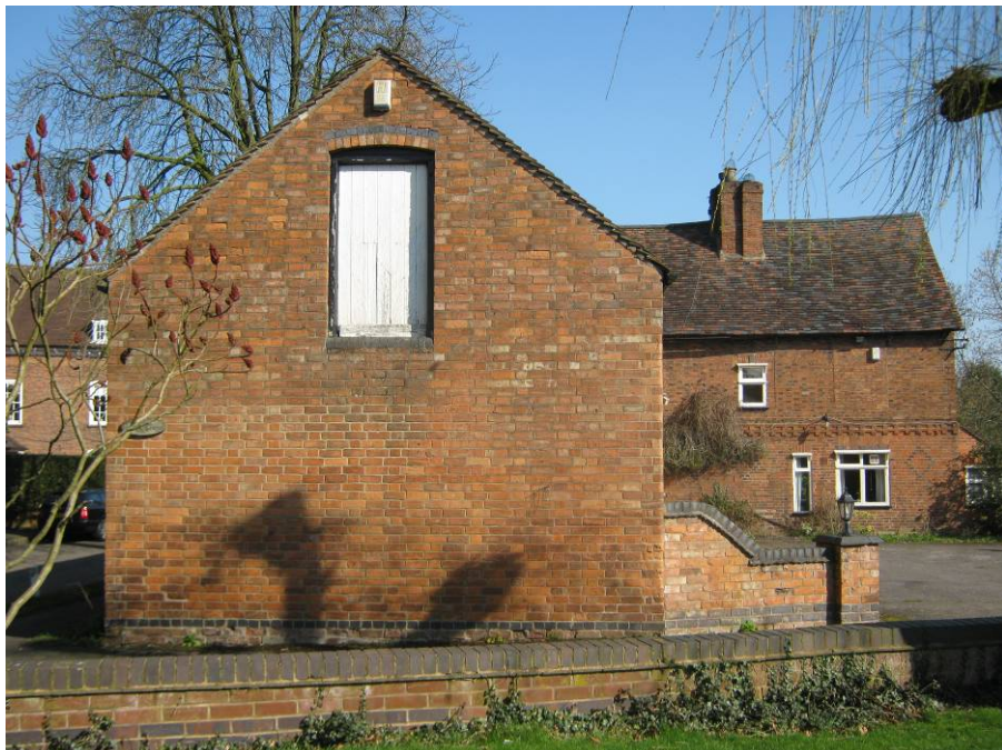
The gable end to the out building attached to the Old Grange. The high level opening, brick segmental arch and rubble plinth are important detail features which add interest to its low key rural appearance.
