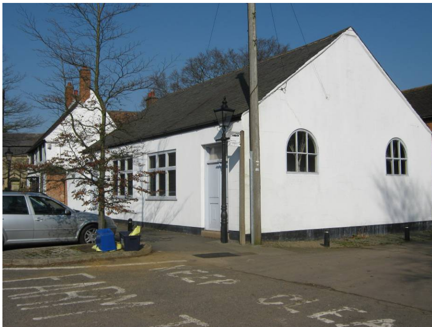
The former church rooms are now used as a shoe showroom. Although the window openings and door locations have been changed, it remains an important historic building in the conservation area. The high chimney adjacent is a key feature which should be retained.
