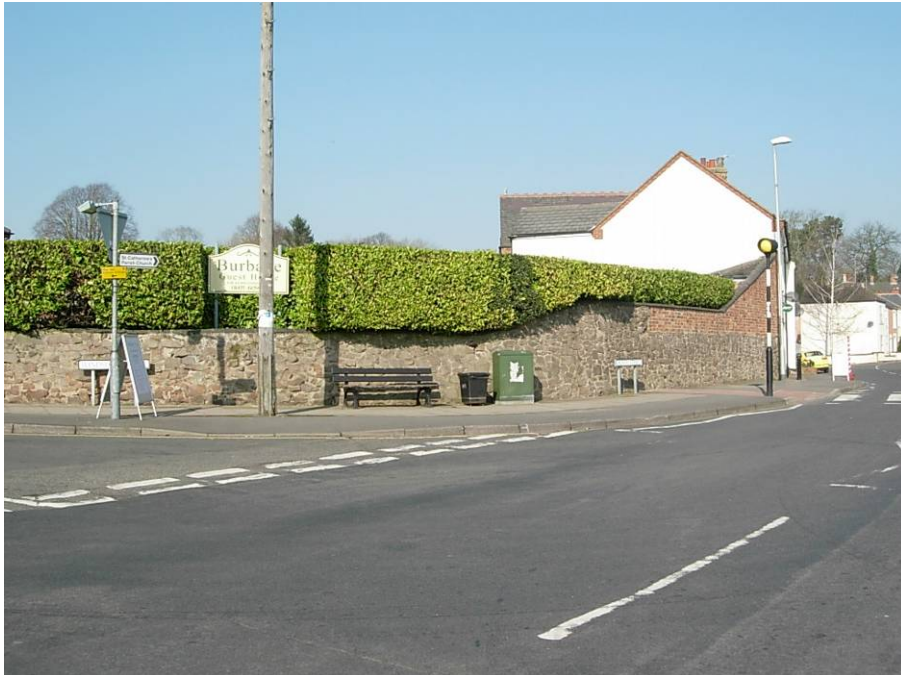
The granite wall and hedge at the junction of Windsor Street/Church Street are pleasant features at the entrance to the conservation area which should be retained.
