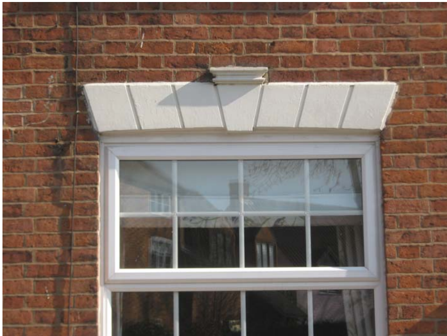
This feature is known as the Hinckley lintol where it is very common. The plastic windows unsuccessfully try to mimic sash windows
