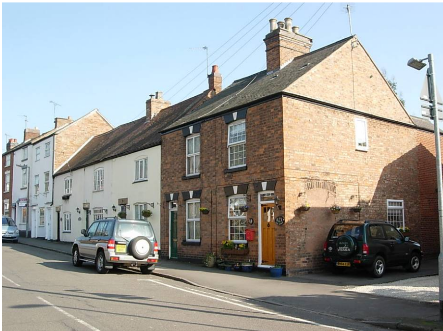
The dwellings at 35-37 Church Street have retained their traditional appearance. Their original brick construction, window openings, lintols and chimney add significantly to the character of the street scene. The side door, that appears to be an added feature, has unfortunately been bricked up. It is unfortunate that the adjoining properties have been rendered.
