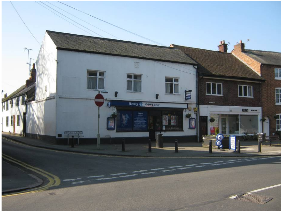
1 & 3 Hinckley Road forms part of a pleasant terrace of properties. This more recent building replaced a three storey property which previously occupied this site.
