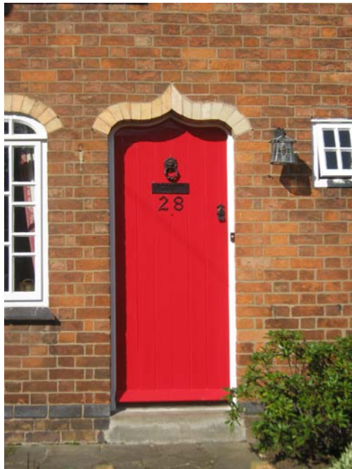
28 and 30 Church Street have painted boarded doors with ogee heads
