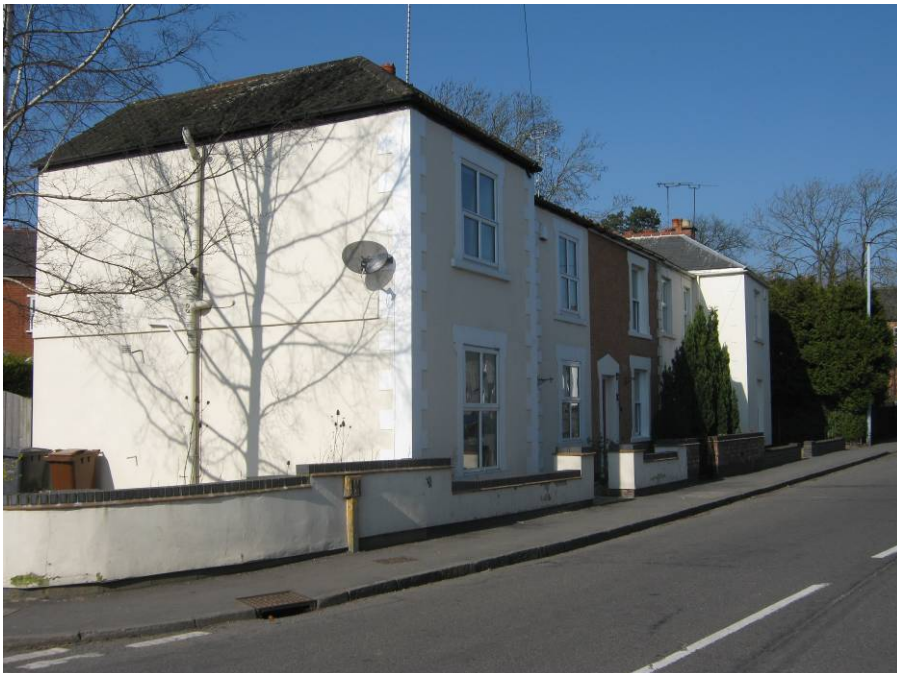
12-16 Church Street is a pleasant block of dwellings that have been rendered and modernised. They originally had railings and a low wall to mark the street boundary. The siting of the satellite dish is unfortunate.
