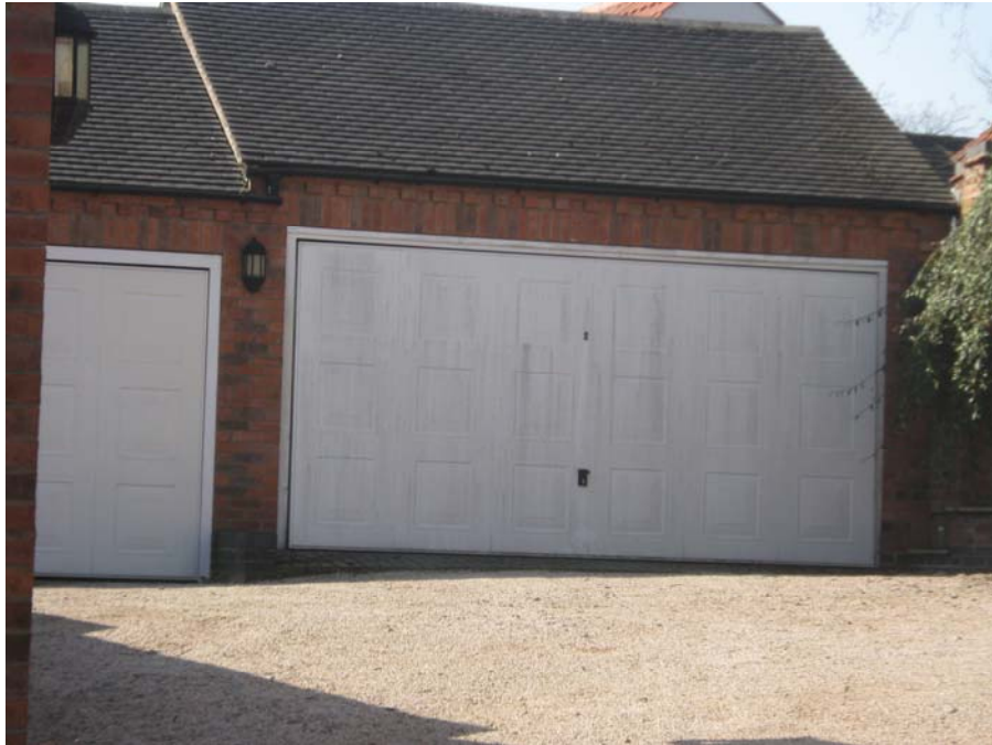
Double garage doors are not a traditional feature in conservation areas. Any future developments should consider using 2 timber doors and not as shown above.
