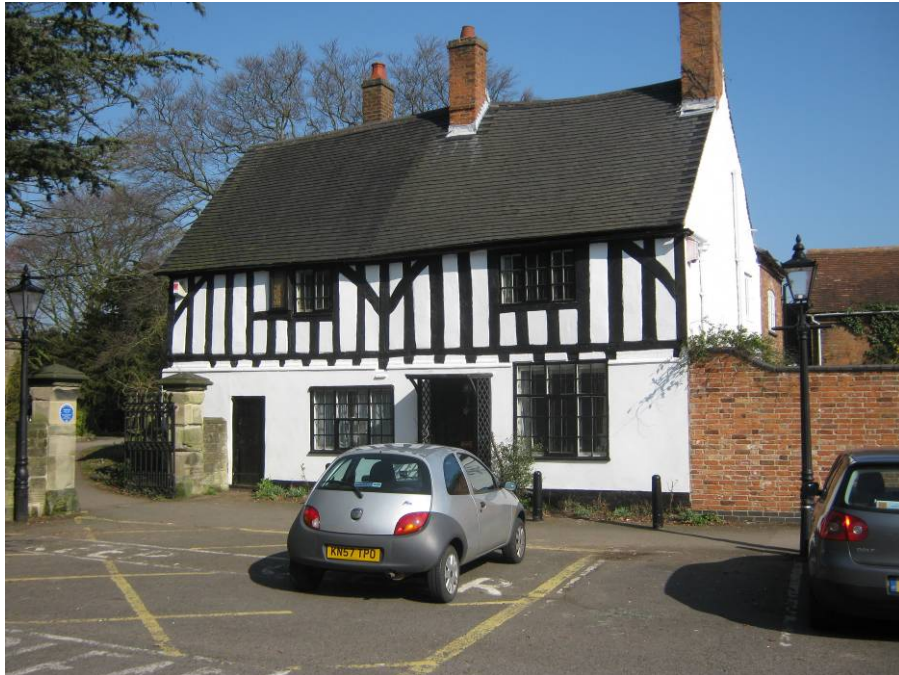
Archers Cottage on Church Street is a late C16 Grade II listed property that was under built in C19 and restored in C20. The dwelling has close studded timber framing on the first floor with curved braces and rendered infill panels. Its roof is plain tiled with brick chimney stacks.
