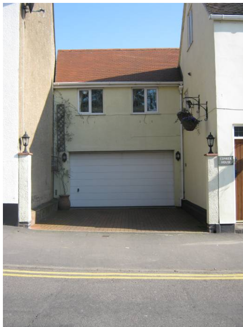
The visual quality of the conservation area would be improved if the double plastic garage door was to be replaced by two timber doors. It is unfortunate that generally modern plastic windows and doors are replacing traditional timber features in the conservation area.
