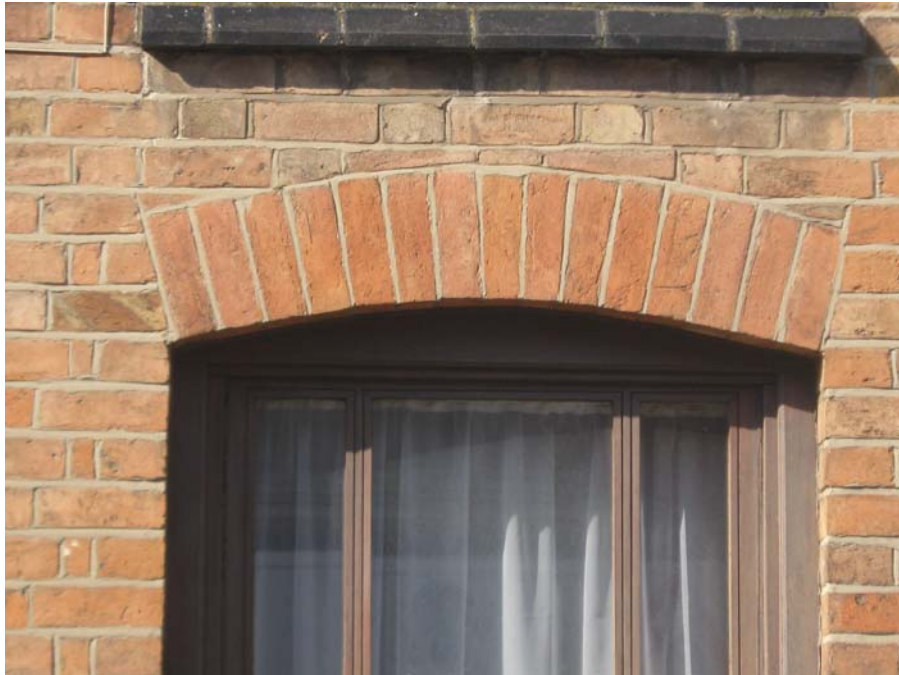
A traditional segmental arch lintol which has been re-pointed.
