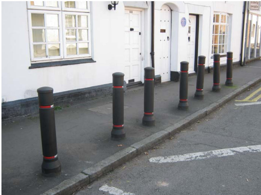
This row of unattractive plastic bollards should be replaced with the 'gunner' type bollards utilized in other areas of the centre.
