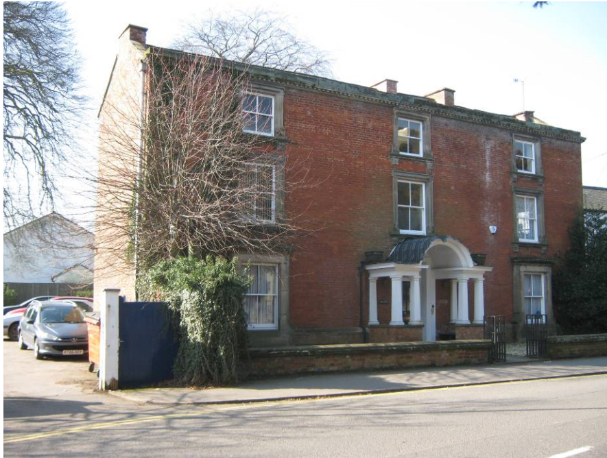
Cedar Lawns is a 3-storey Grade II listed building built in red brick with a Swithland slate roof. The property has a central paneled door with fanlight under a large round-headed hood that was added in the early C20. The building that is now used as offices is fronted by a low brick wall that was once topped with iron railings. The four chimney stacks have lost their pots.
