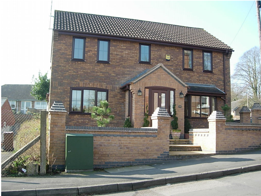
2 Horsepool is a modern dwelling with a subdued design which is set behind a low brick wall. Although its design features are none traditional and the materials used are out of character, its impact on the street scene is neutral.
