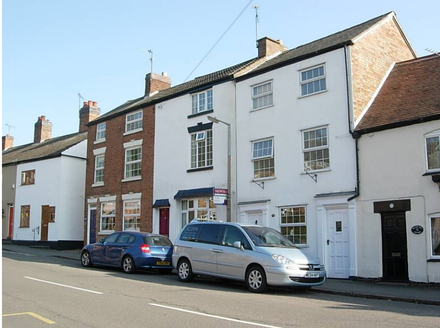
This impressive block of 3 storey properties, 45-49 Church Street, has been spoilt by the introduction of concrete roof tiles, bow window and the loss of lintols. The ground floor of number 45 was originally a shop.
