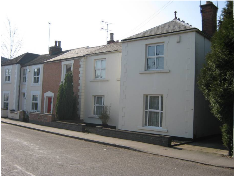
12-16 Church Street looking north westwards. A boundary treatment which was consistent across the whole frontage, would improve their appearance.
