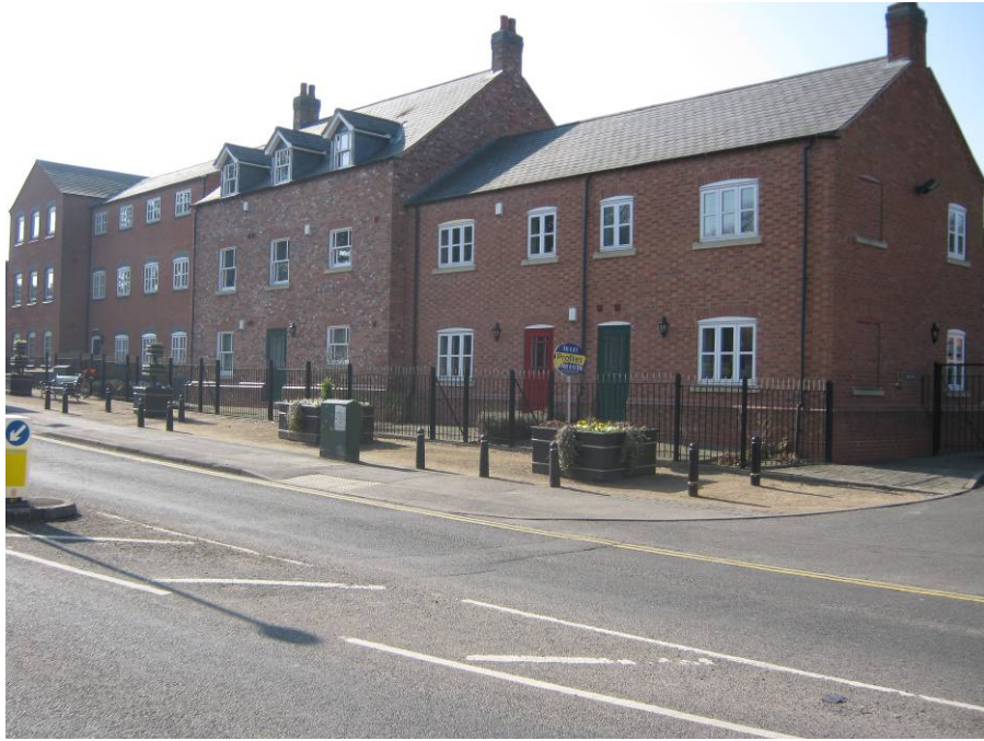
The modern terrace of flats on the west side of Hinckley Road incorporates traditional features, materials and enclose the space which helps to direct views southwards down Church Street. The joinery workshop and offices of Paul & Company formerly occupied this site.
