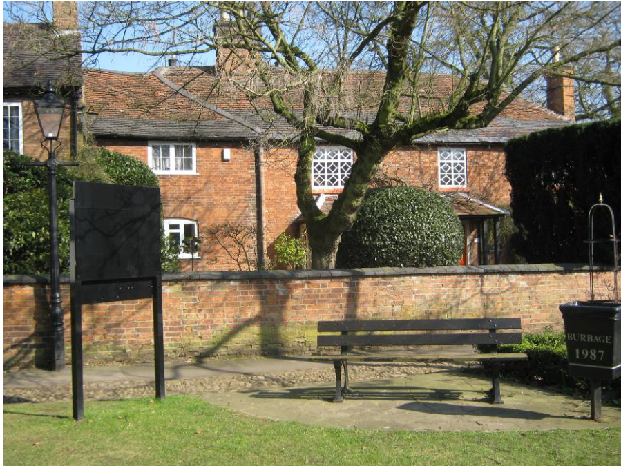
The Grade II listed C17 Manor House. The property was dressed in the C19 with red brick and has a plain tiled roof with some Swithland slates at the eaves. Some of its casements are iron framed with lozenge glazing. The brick wall is an important feature in the conservation area forming a strong edge to the space
