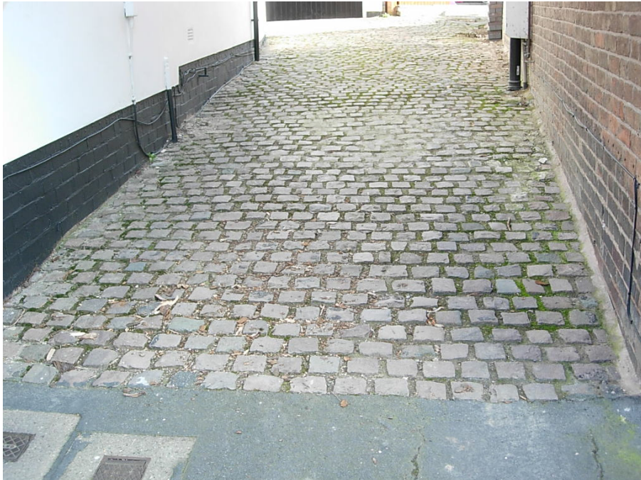
Access on Church Street surfaced with granite setts.
