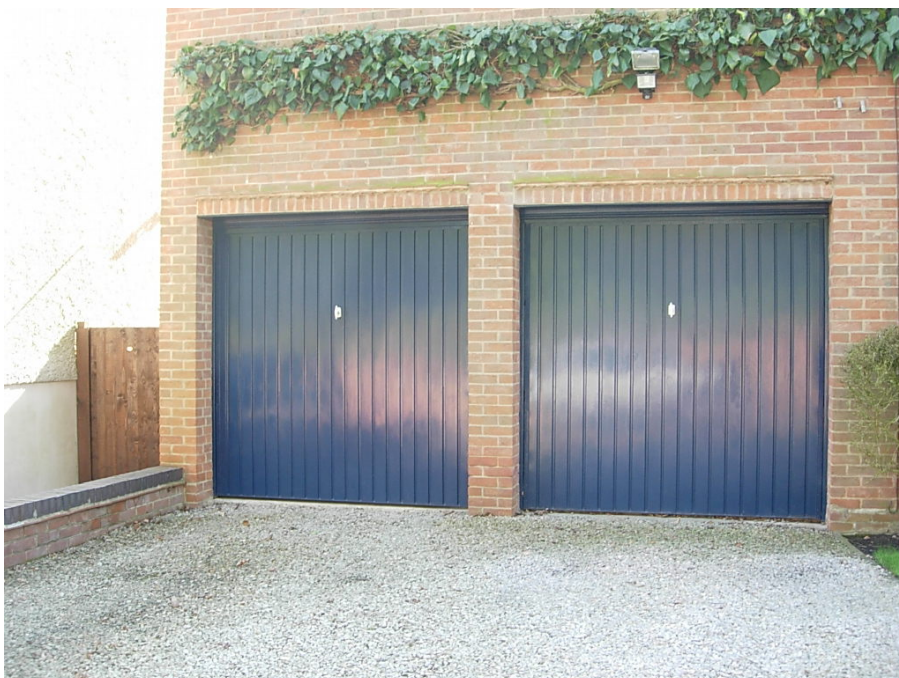
The use of 2 doors in a double garage painted in a dark colour is preferable to the installation of one double door painted in white.
