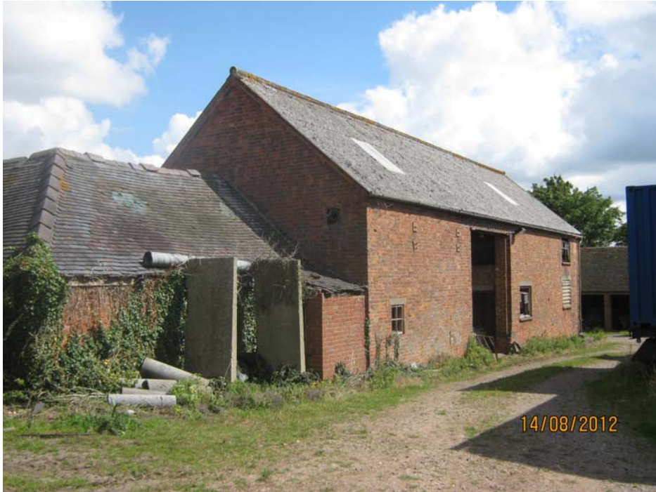
One of the large imposing buildings sited at the former Bilstone Hill Farm complex. The Farmstead has a number of fine traditional buildings, however, several are in need of urgent restoration.
