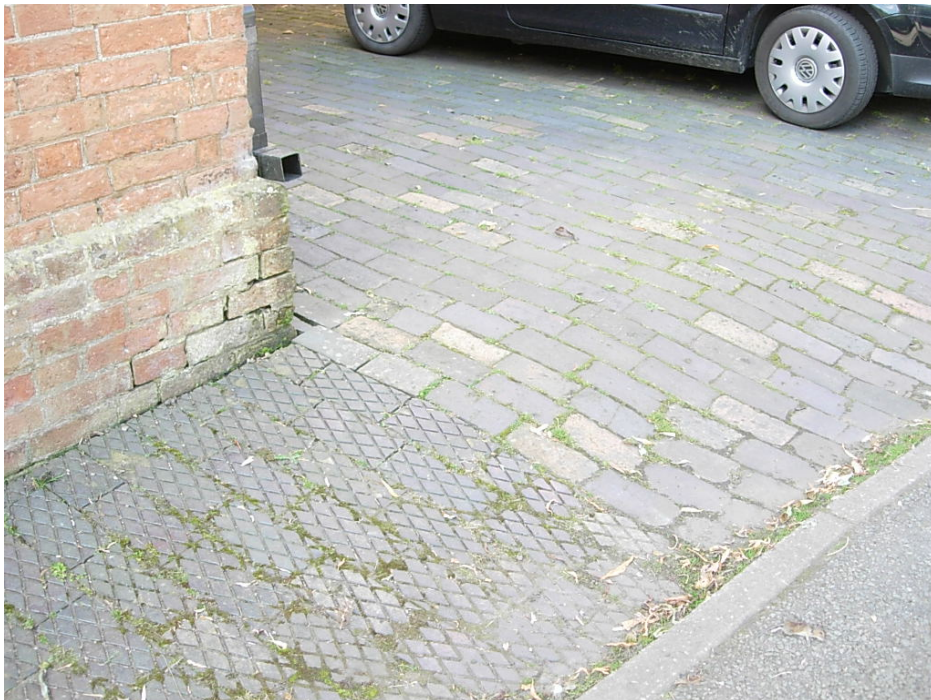
The diamond pattern and plain brick pavers which form two different ground treatments used at 25 Main Road enhance the rural character of Bilstone.
