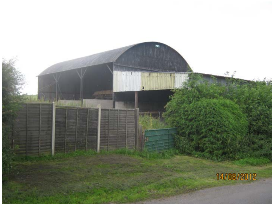
The large Dutch Barn at Deans Farm is a prominent feature that adds to the rural charm of Bilstone. Unfortunately, the fencing is out of character and consideration should be given to replacing it with traditional fencing such as a post and rail agricultural fence and hedging.
