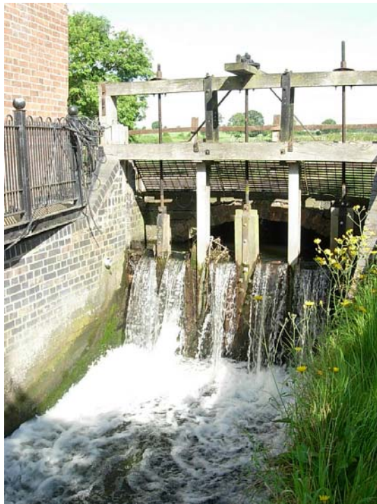
The sluice-gate on the River Sence adjacent Bilstone Watermill is of considerable interest to ramblers using the field footpath to Congestone.
