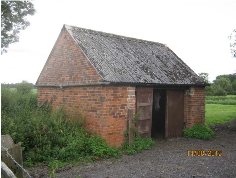
This quaint outbuilding to the rear of Drove House is spoilt with the use of a non-traditional roofing material.
