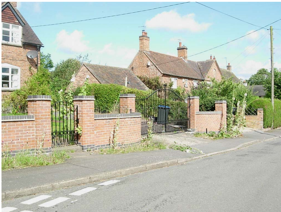
The modern brick wall and gates at 28 Main Road are suburban in character and do little to enhance the rural character of Bilstone.
