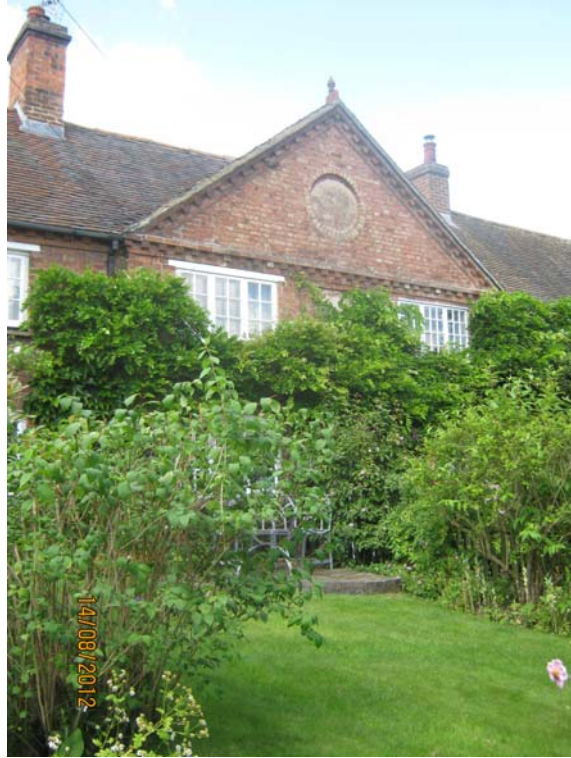
25 Main Road has a delightful brick pediment feature on its front elevation. The property was once used as a chapel until 1805.
