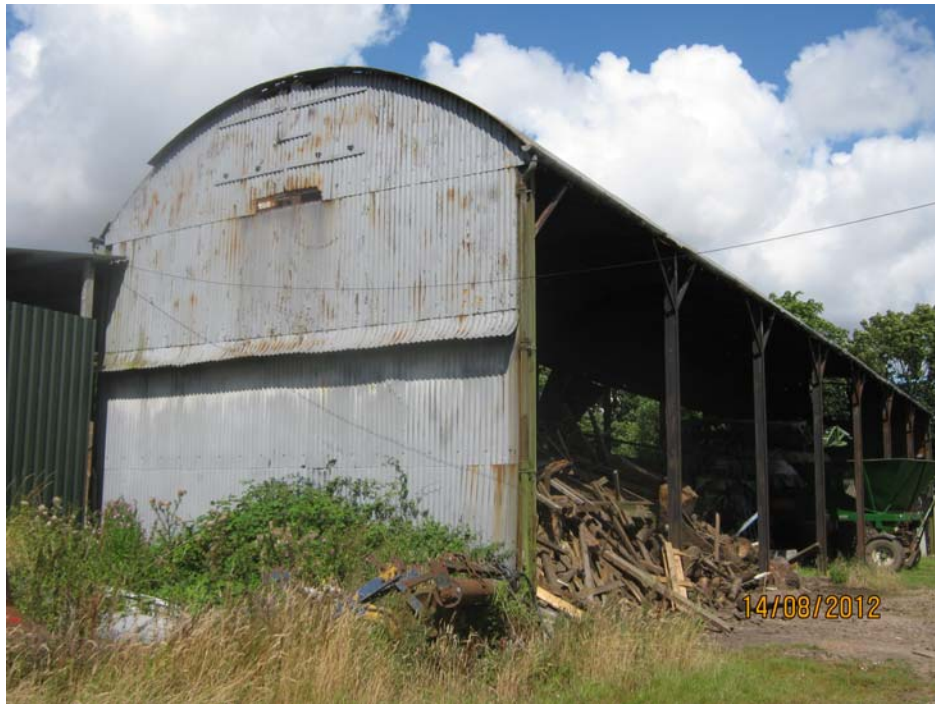
This large imposing Dutch Barn is an excellent prominent feature sited on the Bilstone Hill Farm complex, unfortunately, it is in need of some repairs.
