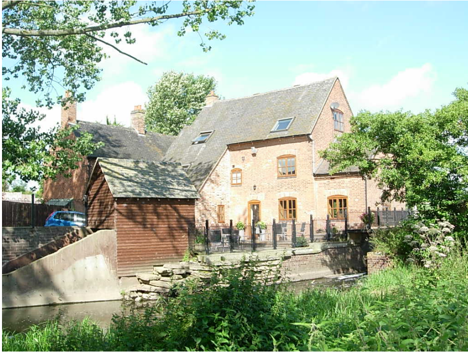
The rear elevation of Bilstone Watermill with the River Sence in the foreground. It is unfortunate that loose irregular slabs have been used to form the edge of the mill race.
