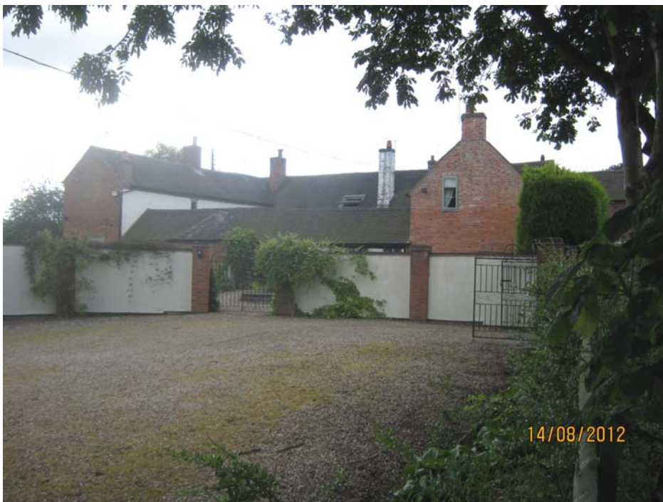
Rear of Drove House showing rear service buildings that once contained pigsties; coal houses and earth closets.
