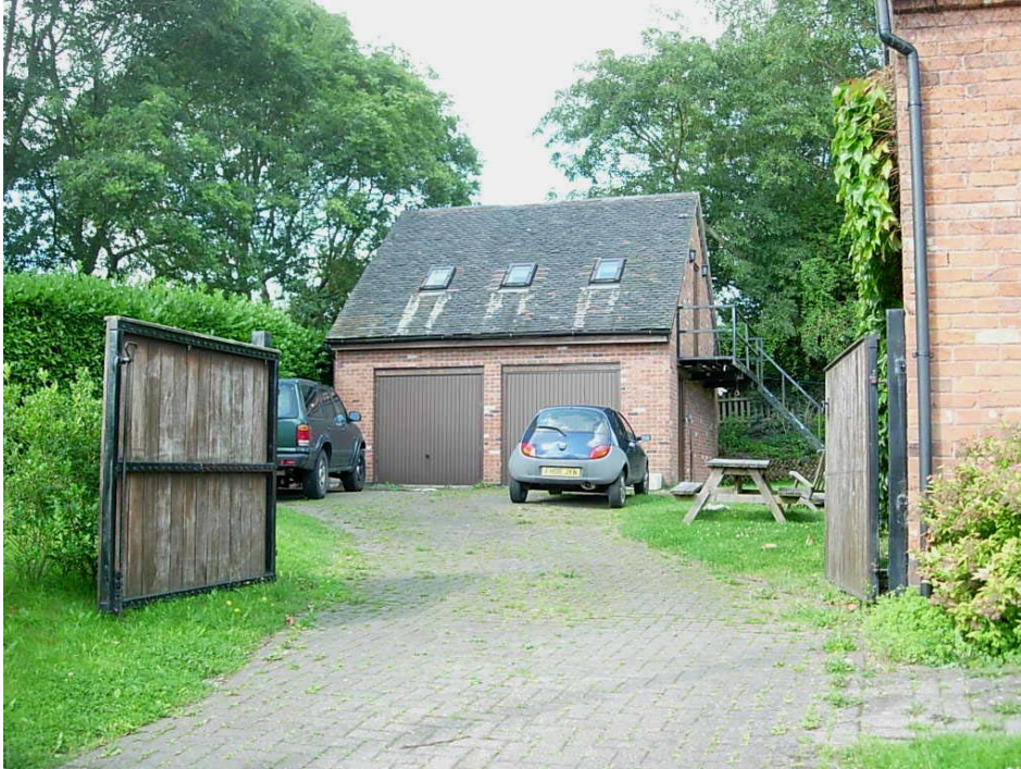
This double garage at 29 Main Road is acceptable with 2 timber doors although it would have been preferable if the roof lights were confined to the rear elevation only.
