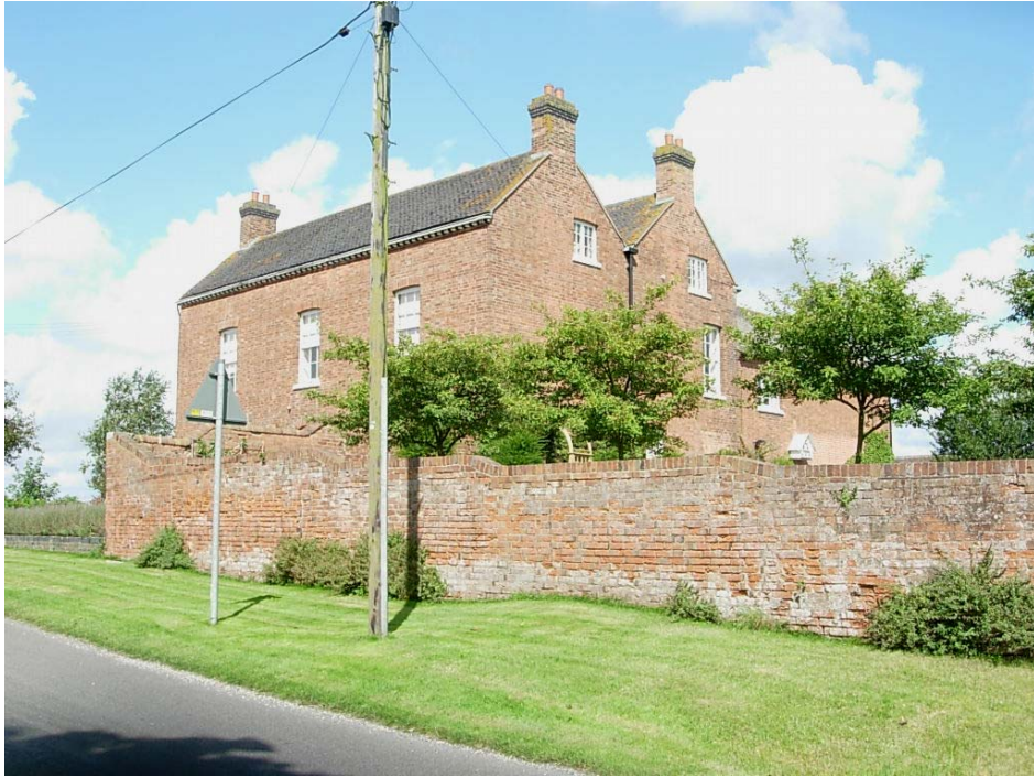
Bilstone Hill Farmhouse is a large imposing early C19 Grade 2 Listed Building built in red brick with a plain tiled roof and end chimney stacks. The 2 storey property has twin end gables and gable-lit attic. The side garden is enclosed by a high traditional brick wall.
