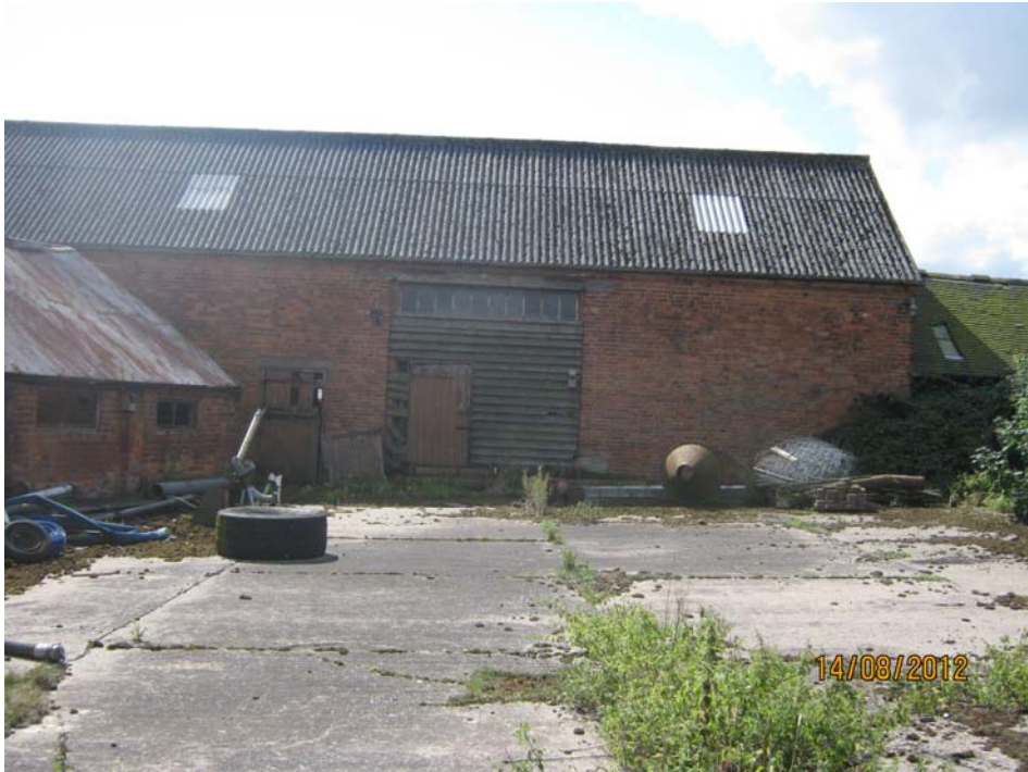
The northern elevation of the large barn sited at the former Bilstone Hill Farm.
