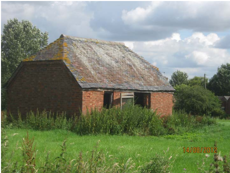
This quaint derelict half hipped building is sited in a large paddock to the west of Main Road. Such buildings add significantly to the village's rural character and their loss should be avoided.
