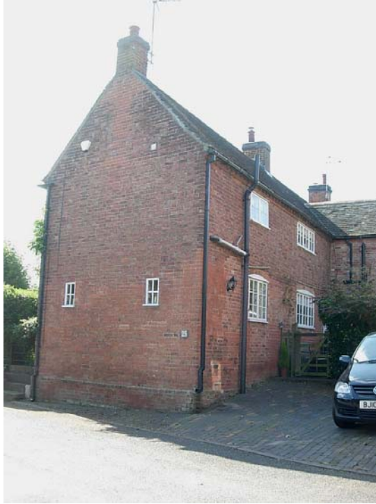
The gable end of 25 Main Road sited at a bend in the carriageway is an imposing feature.
