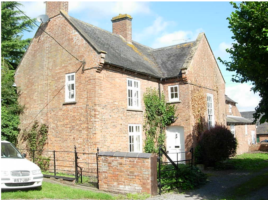
Dean's Farm looking south westwards showing its prominent corbelled gable ends and Georgian style windows
