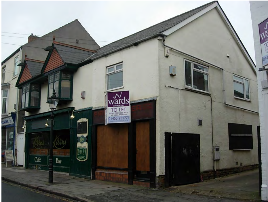
15-19 New Buildings are mid C19 buildings that have been heavily modified by the addition of bay windows and projecting gables. These add to the group's significance as do the traditionally designed shop fronts.
