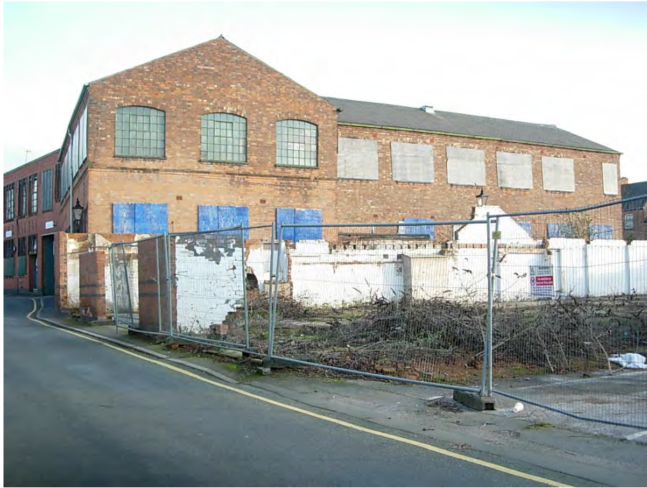
The recent demolition of 21 Wood Street detracts from the appearance of important heritage assets.
