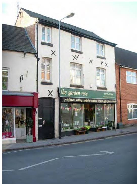
4 New Buildings is a late C19 building with a Welsh slate roof which has been rendered. It has a separate yard entrance on the frontage.
