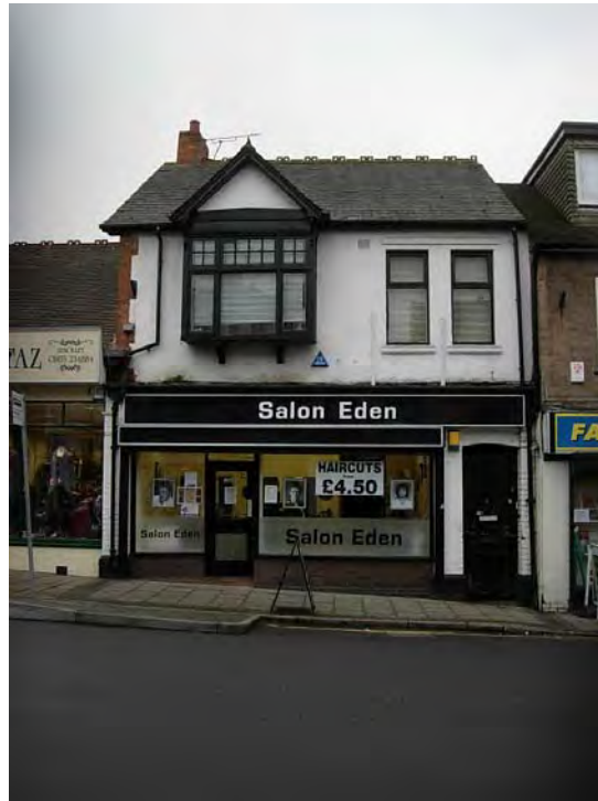
73 Castle Street is probably an early C20 building with a pendent bay at first floor.
