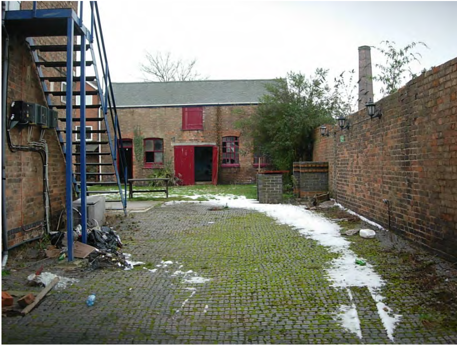
This yard at 113 Castle Street has retained its original setts and two interesting outbuildings.
