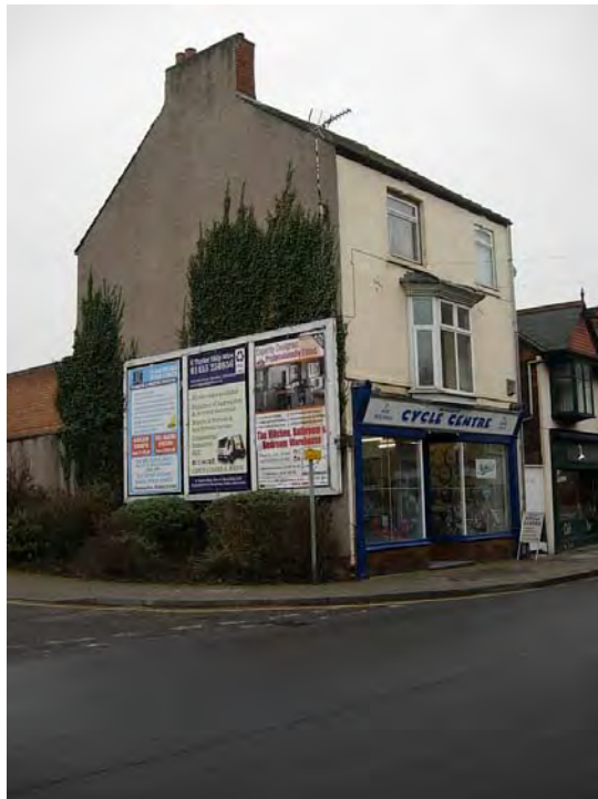
21 New Buildings is a late C19 building that has retained its early C20 shop front and bay window at first floor. The large posters on its gable end detract from the street scene.
