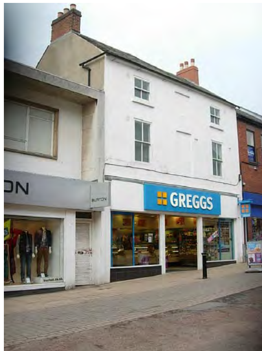
22 Castle Street is probably an early C19 building with a late C20 shop front. It has unfortunately, had its street façade painted although it has retained its chimneys and traditional style windows on the upper floors.
