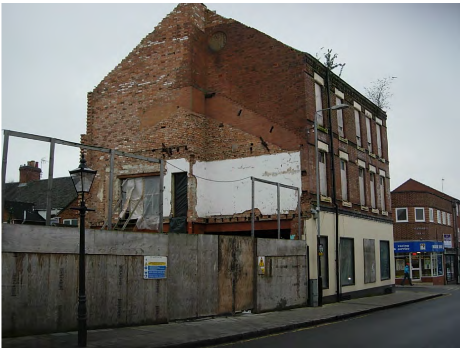
The property 109 Castle Street has recently been demolished. The vacant site is an eyesore and in urgent need of re-development
