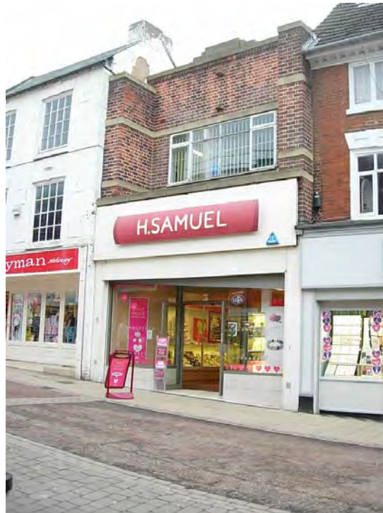
21 Castle Street is a mid C20 building and although not of a traditional appearance, is not obtrusive in the street scene.
