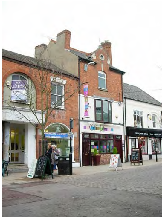
The quality of 80 Castle Street can still be seen despite the modern bay and shop front which have been added.
