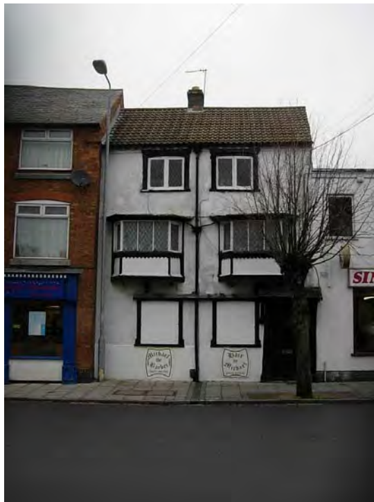
130 Castle Street is probably C19 with C20 glazing and canted bays at first floor.
