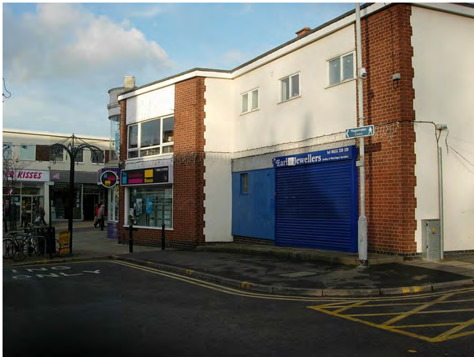
1-3 Church Walk is a Council owned building that has no historic and very limited architectural interest.
