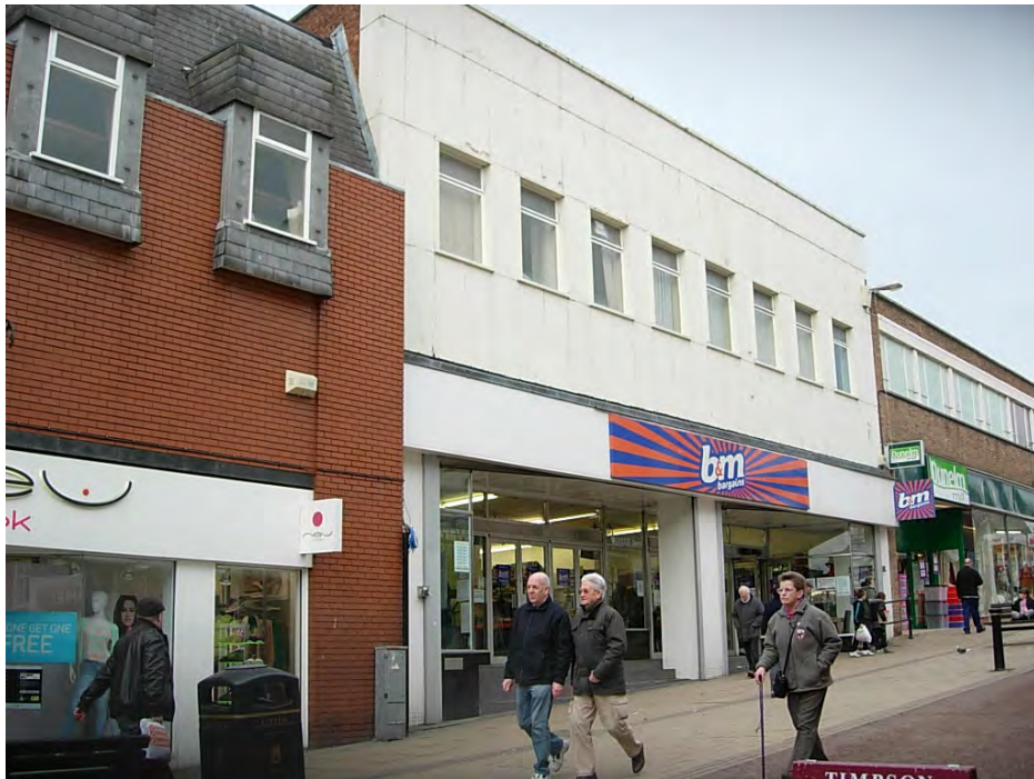
36 & 38 Castle Street lacks interest and has limited impact on the street scene.
