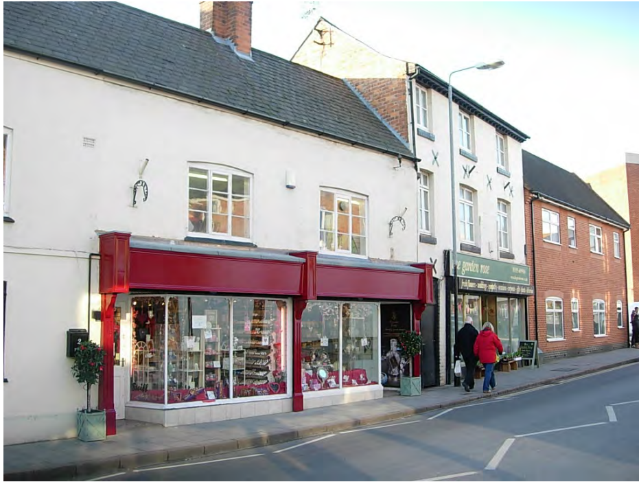
These new shop fronts in a traditional form at 2 New Buildings enhance the street scene.
