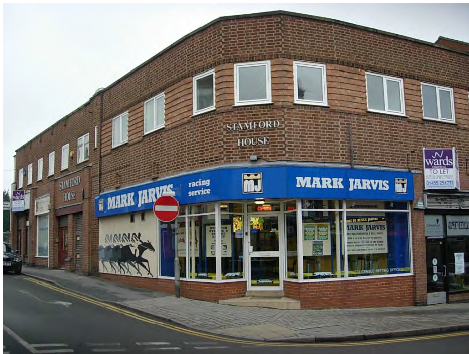
On the opposite corner of Hill Street is 97 & 97a Castle Street which is an unmemorable mid C20 building.
