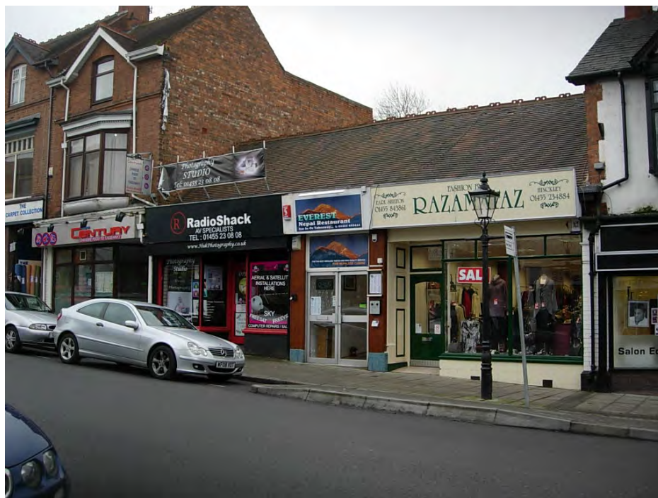
75-81 Castle Street is an early C20 building with C20 shop fronts, both of which have recessed entrances.
