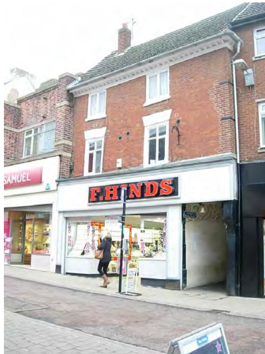
19 Castle Street is a C18 building that incorporates the entrance to Bell Entry, an important jitty which links this street to the church. The C20 shop front incorporates an overly large fascia which detracts from the appearance of this fine building.
