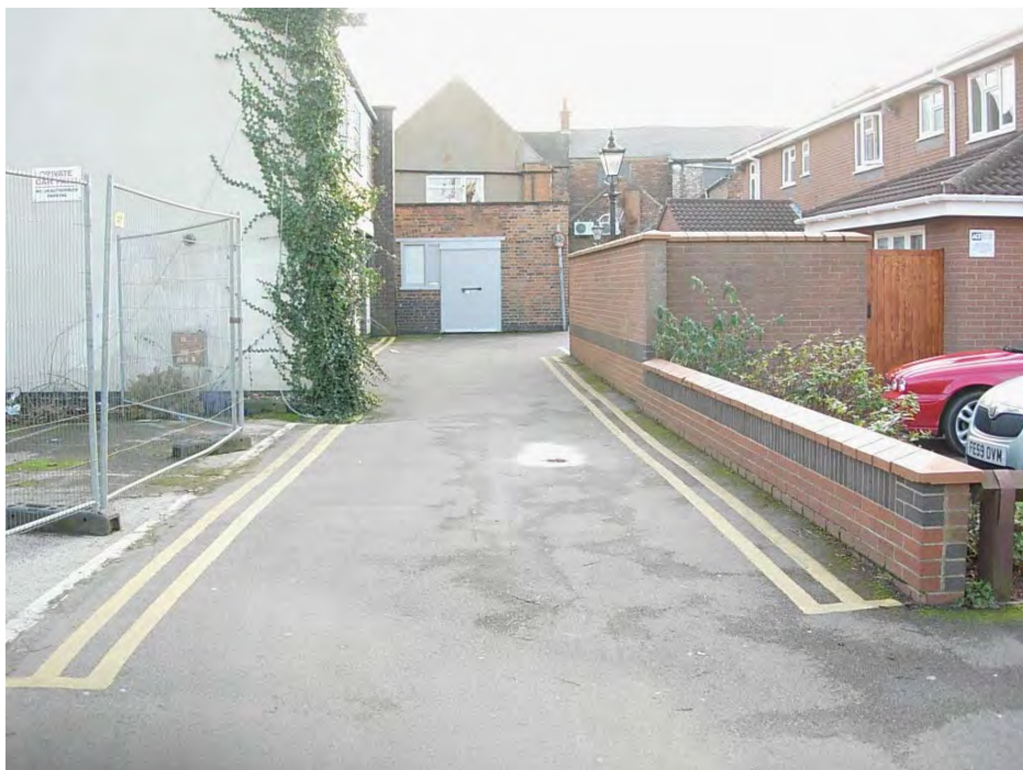
The demolition site flanking the Crown & Anchor Yard has unfortunately created a large gap in the yard frontage.
