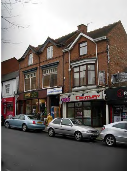
83-87 Castle Street is a late C19 building with a canted bay at first floor. Eastern large first floor windows may have replaced original bays.
