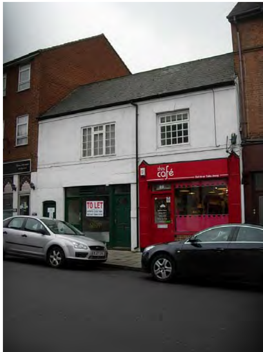
89-91 Castle Street is probably a C18 building with splayed and grooved lintels, C20 shop fronts and segmental arched opening to form a yard entrance.
