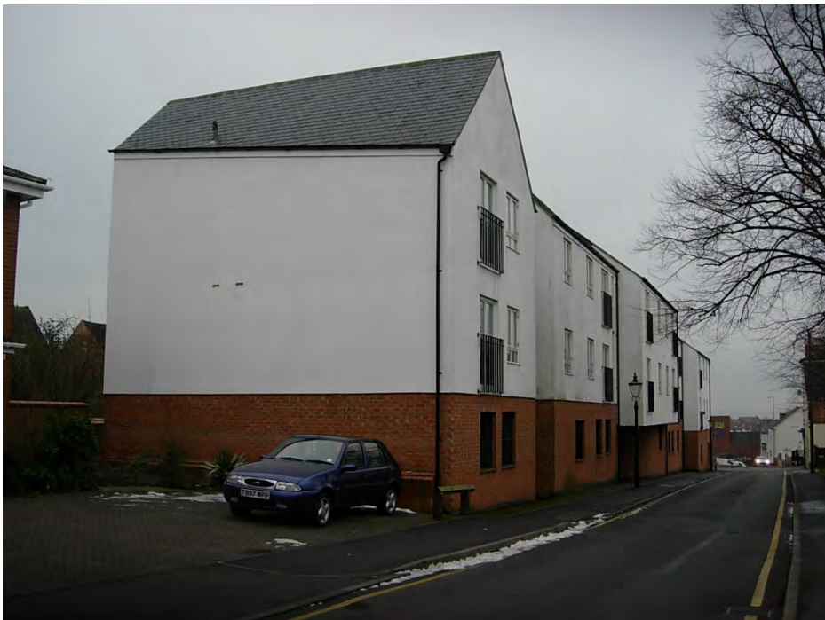
Castle Point sited at the western end of Wood Street that is set at the back of the pavement, extends the same factory style as those factories at the head of Wood Street.
