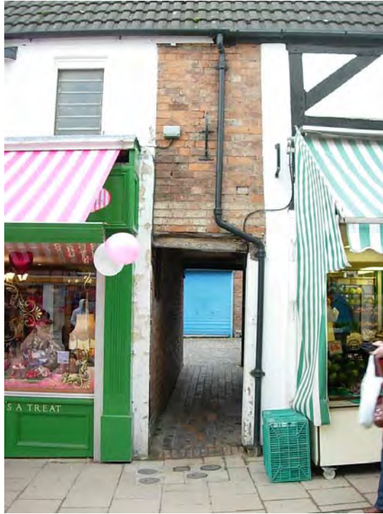
The entrance into Lilley's Yard is very low and incorporates an old timber lintel. The old brick pavers covering the floor add character to this entrance.
