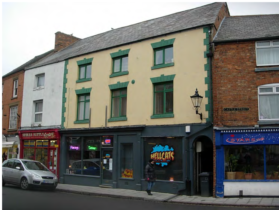
126 Castle Street was constructed in the early C18 and includes an arched yard entry and a C20 shop front. The colour scheme adopted for the building is unfortunate.
