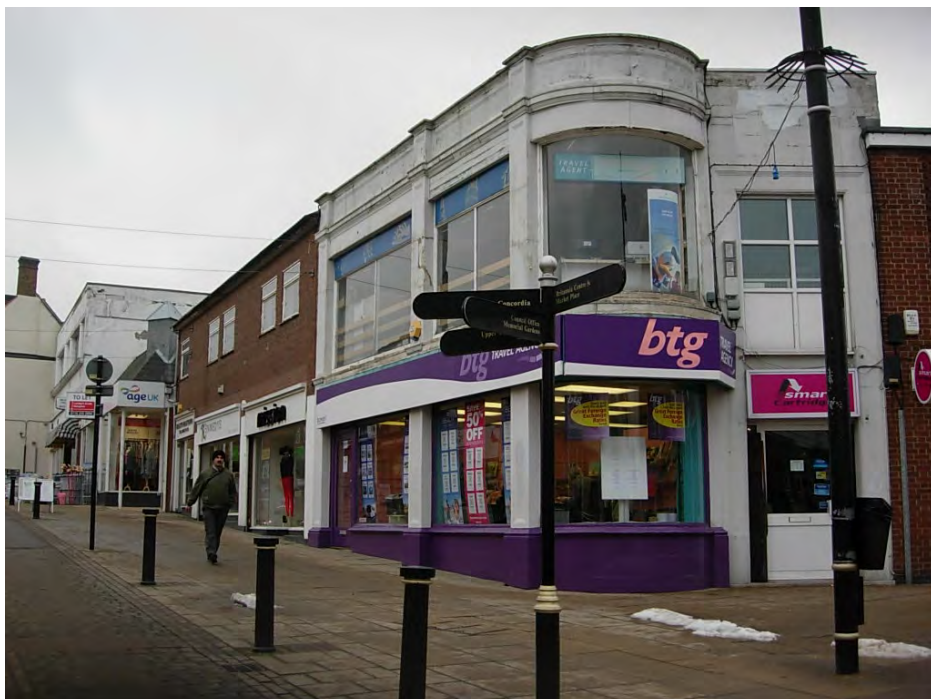
39-43 Castle Street. The corner building was originally the gas showrooms and extended a further 2 bays to the south. Its 2 storey curved corner bay is a landmark on this part of Castle Street. The attached building to the north is late C20 and of no historical interest.
