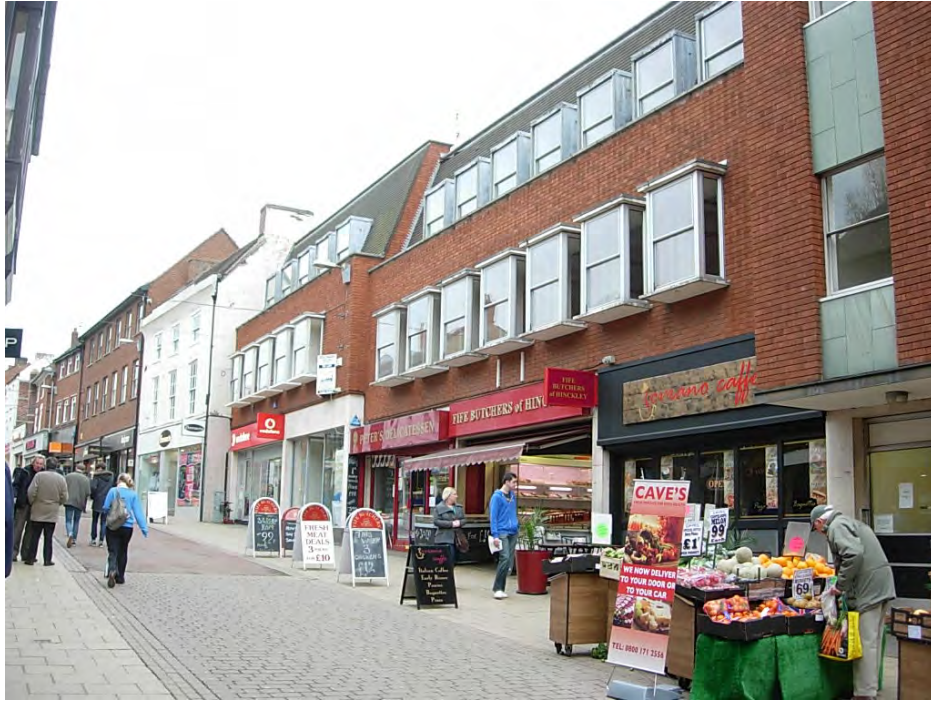
3-9 Castle Street are late C20 buildings that extend down to the Market Place and along its frontage. Although generally out of character, they are of interest in places.
