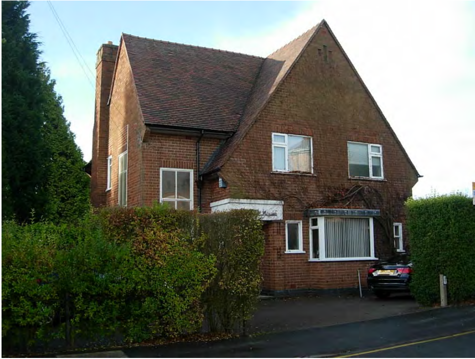
The western side of Hill Street was developed in the 1930's and has several interesting properties similar to The Mead on Hill Street
