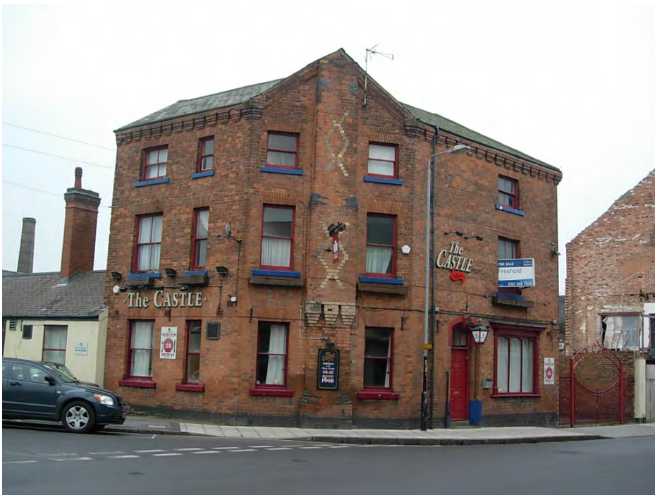
113 Castle Street is a landmark building constructed in the late C19 that has an interesting projecting stack on the centre bay and polychromatic brickwork.
