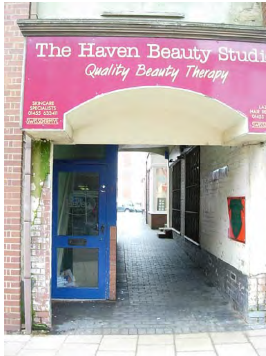
Entrance into Crown Court. Regular maintenance would considerably improve the appearance of this jitty.
