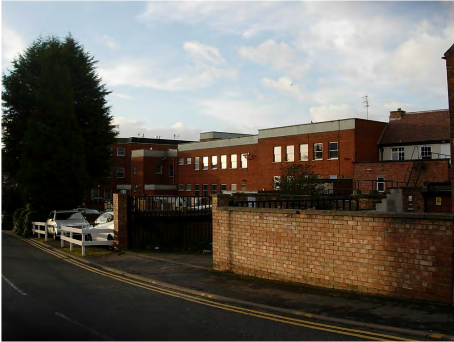
Rear of 3-9 Castle Street viewed from Church Walk with car parks and service yards in the foreground.
