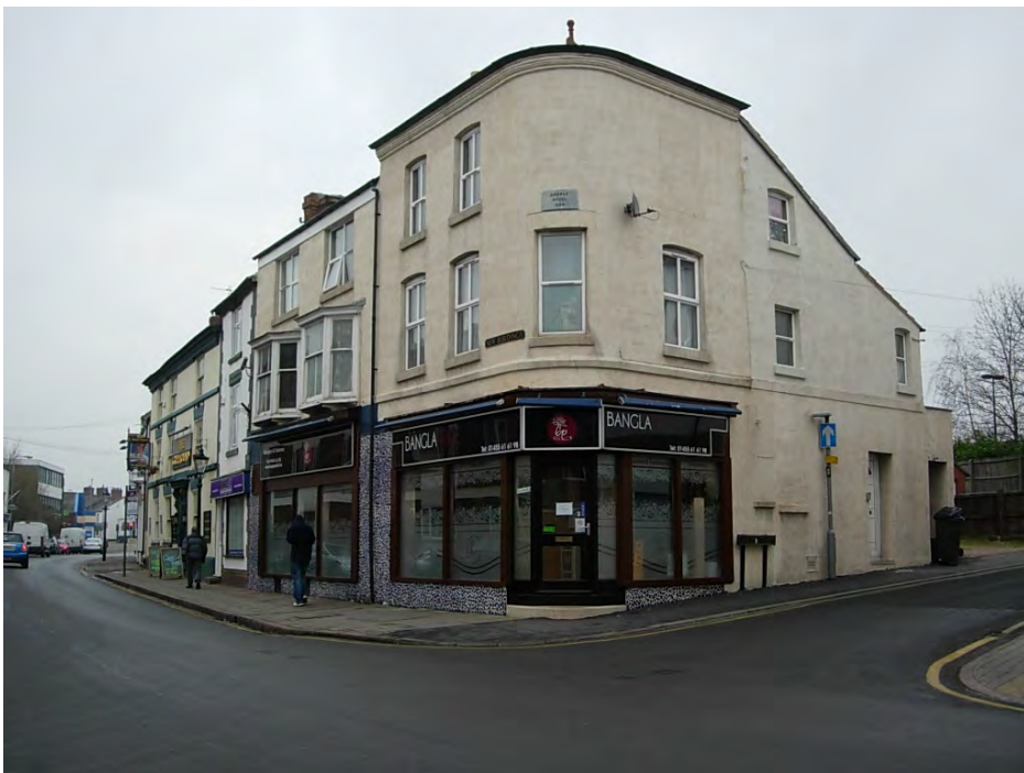
The tablet above the entrance door to 3-5 New Buildings indicates this building was constructed in 1884 as Argyle House. It has a feature curved corner and sash windows to the upper floors. The mosaic tiles detract from its appearance.
