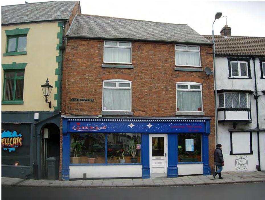
128 Castle St is an early C19 building with brick segmental arch lintels and C20 shop front and windows.
