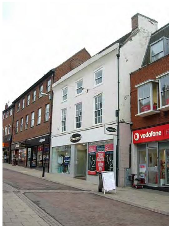
11 Castle Street is a grade II listed building that suffers badly from a lack of maintenance.
