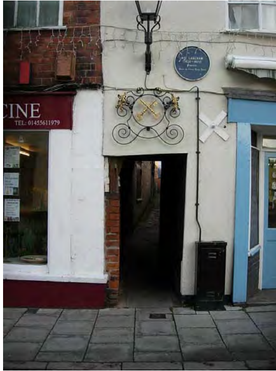
Cross Keys Yard includes some timber framing exposed on the left side of the jitty.
