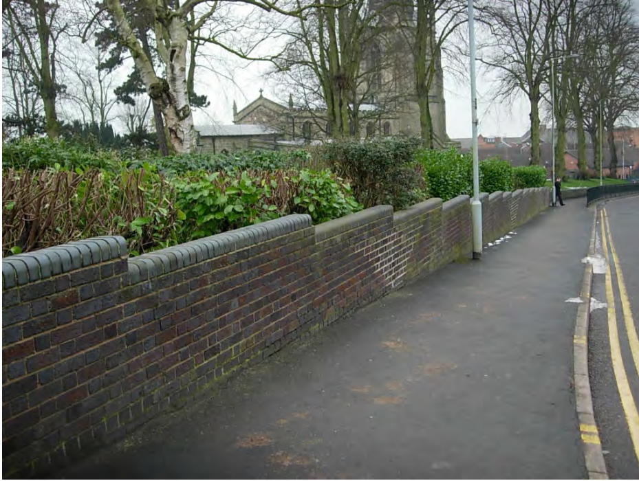
The blue brick boundary wall on the south side of Church Walk with its saddleback copings defines the extent of the churchyard and is a very important historic feature and an asset in the Conservation Area.
