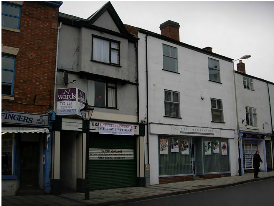
106/108 Castle Street is a C18 building that during the late C19, was the Crown and Anchor public house. The frontage includes the yard entry and is unusual in including a small roof gable and projecting bay at second floor. The rear range is probably C19.
