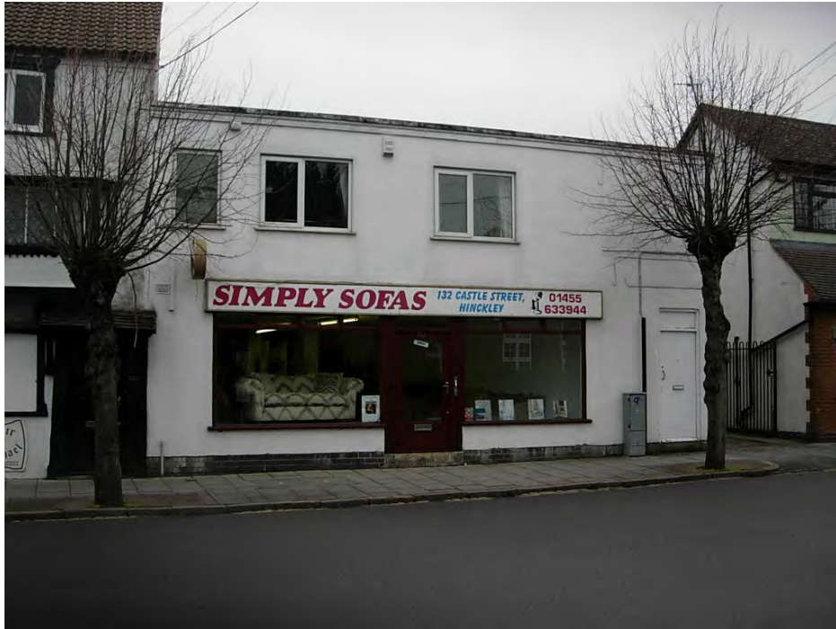
132 Castle Street is a late C20 building of limited interest.
