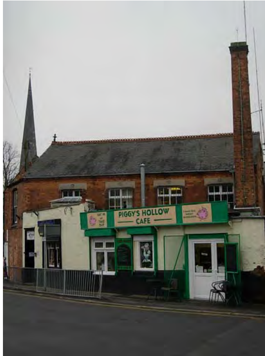
This view of 5-7 Church Walk shows one of the few brick factory chimneys remaining in the town centre. These are important relics of the hosiery industry which must be retained.
