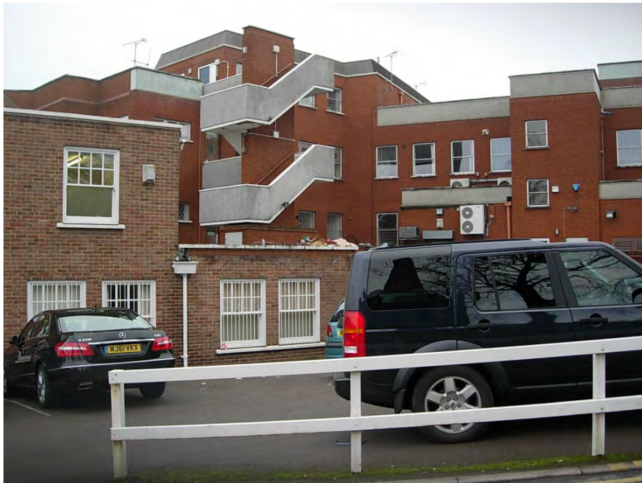
Rear of 1 & 3 Castle Street viewed from Church Walk. This street is blighted by car parks and rear service areas.
