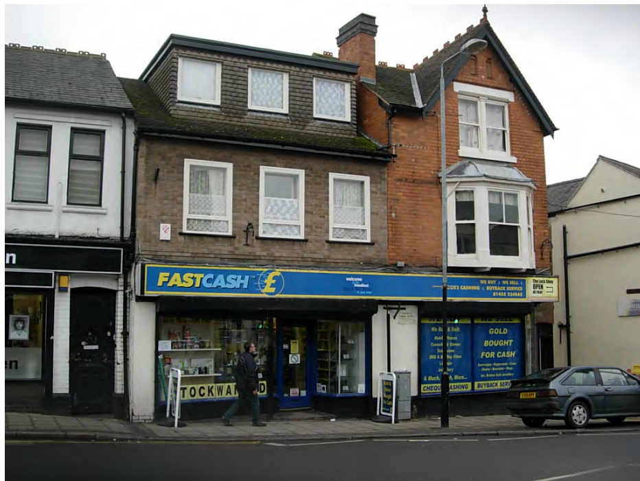
69-71 Castle Street is a combination of two buildings. The right hand side is late C19 with a canted bay at first floor. The left hand building is mid C20 with a recessed entrance and an overly dominant flat roofed dormer.
