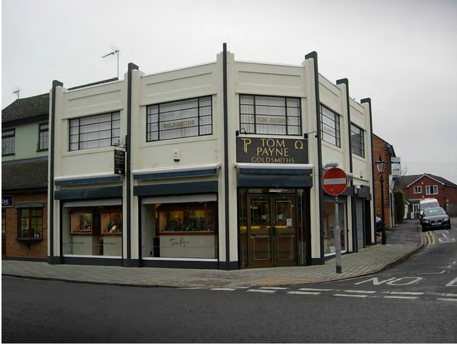
140-144 Castle Street was constructed in the 1930's in the Art Decoratif style and is a very interesting heritage asset that completes the commercial centre.
