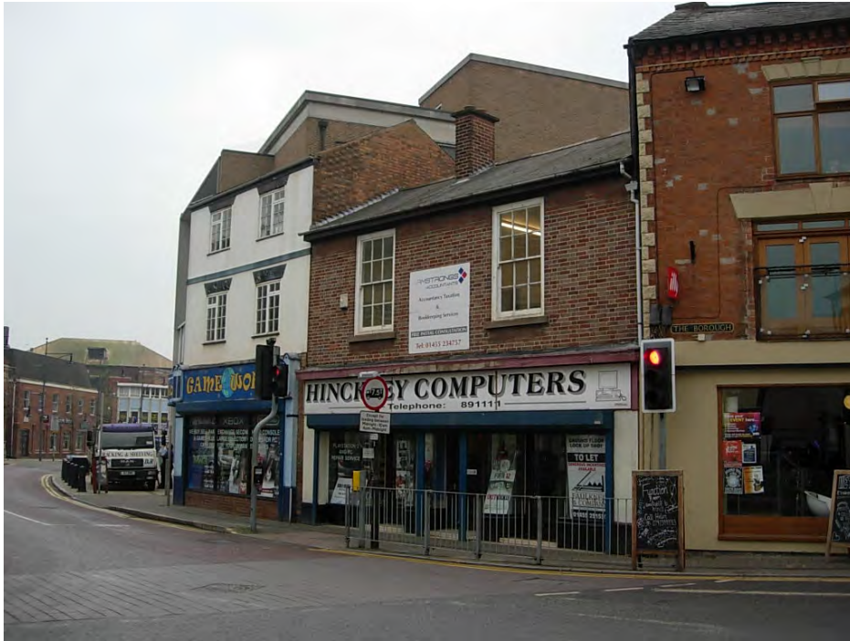
20 The Borough has been reconstructed in the mid C20 but does retain vertically proportioned windows, a slate roof and a central brick chimney. Its appearance, however, is spoiled by the projecting roller shutter and its housing.
