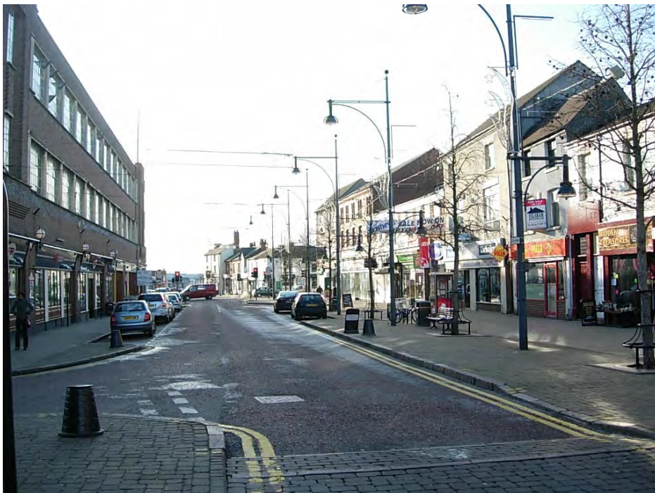
. This view looking south along Regent Street highlights the difference in scales of the C20 former hosiery factory and the C18/19 frontages on the western side. All of the buildings on the western side and the former hosiery building on the eastern side of the photograph are important heritage assets which must be protected.
