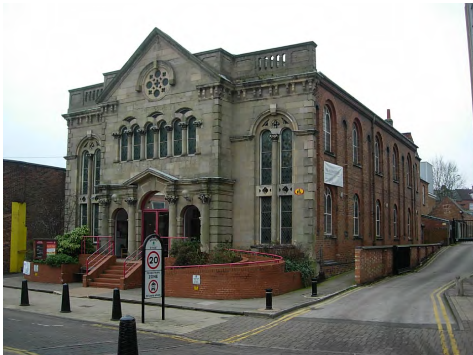
The United Reform Church is a very distinctive Grade II listed Non-conformist Church designed by F. Drake that has a street frontage of ashlar stone in the Italianate style. The remainder of the structure and the attached school rooms are of brickwork with slate roofs.
