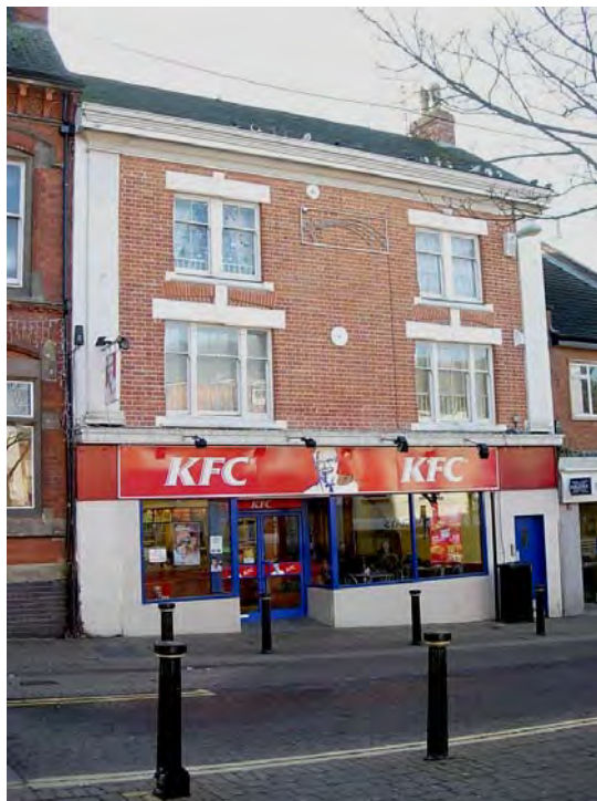
12 Market Place. The upper floors of this building have been carefully restored and add interest to the Market Place. It is unfortunate that the shop fascia is overly large and the colours of this and the shop front are not in keeping with the Conservation Area.
