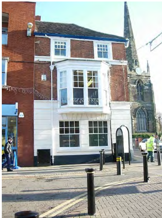
2 Market Place. The view of this building from the Market Place is interesting in that the bay window was a later addition to the property which considerably improved the appearance of the building.
