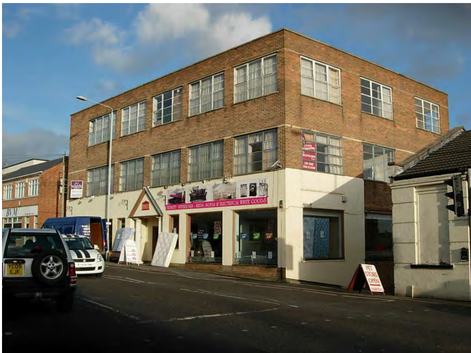
Abbott House, Trinity Lane. This former factory has been converted into retail space. It stands at the entrance to Blockleys Yard. The signage and the timber pediment sit uncomfortably on the face of the building. These features are out of character with the simple rectangular form of the building.
