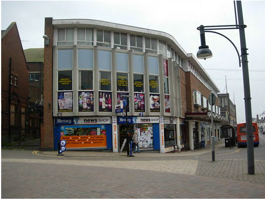
Northern end of the Edwards Centre reflects a style of design common during the 1960s and the 1970s. It is unfortunate that the small development blocks of earlier periods, has been lost.
