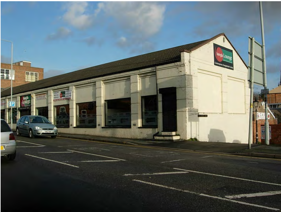
91 Trinity Lane and the entrance into Blue Boar Yard. This was a factory until recently when it was converted into a restaurant.
