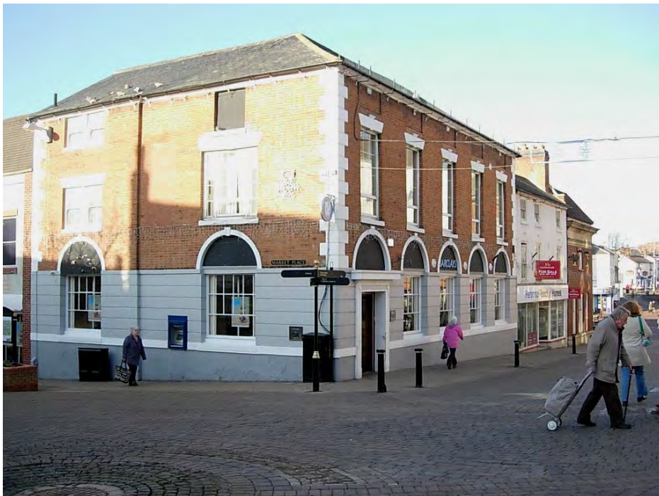
This elegant listed building suffers from the installation of plastic double glazed windows at first floor which detract from its appearance. These were unfortunately granted consent by the local authority in the late 1980's. However it remains an important heritage asset in the Conservation Area.
