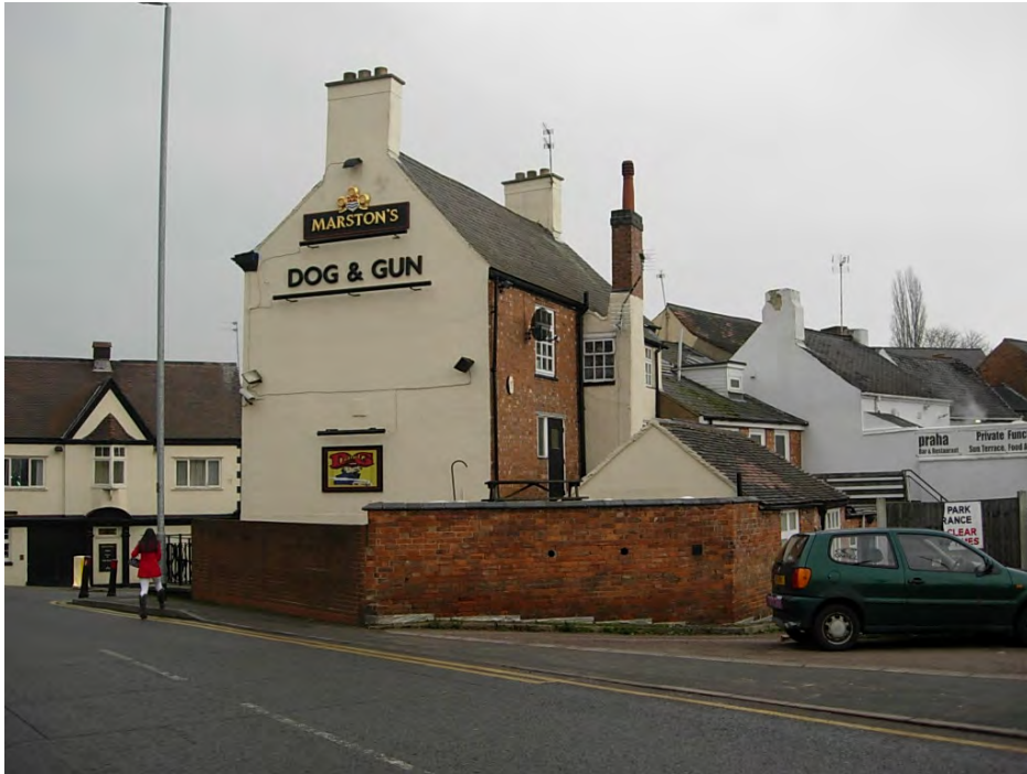
The Dog & Gun Pub from Mansion Street. This view shows the tall brick chimney stacks and high brick boundary walls which are a feature of this public house.
