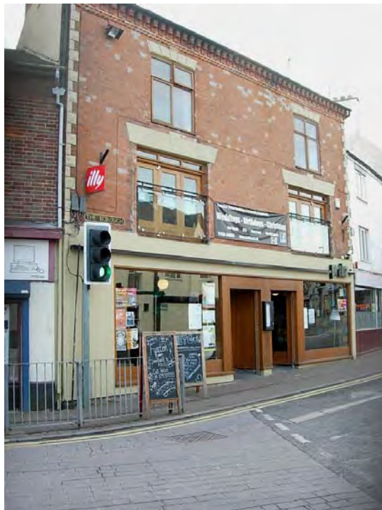
22/24 The Borough is predominantly a mid C19 building that has overly large openings at first floor which may have been originally intended for bay windows. Should these features be added in the future, they will significantly improve the buildings appearance.
