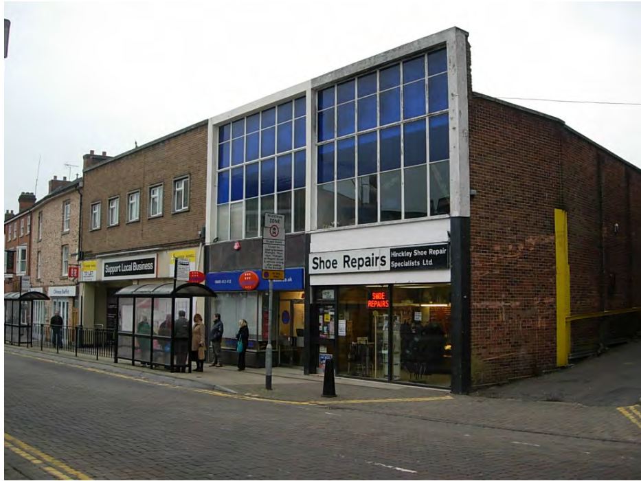
2-6 The Borough is a development from the 1970's which although quite different in appearance to other buildings on the western side of the street, uses similar plot sizes and parapet heights to the other traditional buildings.
