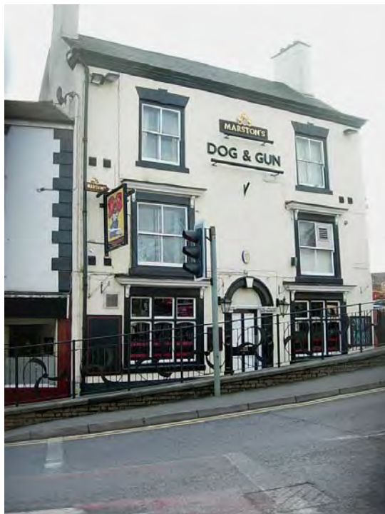
28 The Borough is largely a mid C19 property with a rendered frontage and a rear courtyard. Its street elevation sparkles and considerably adds to the character of this part of the street. It is an important heritage asset to the Conservation Area.
