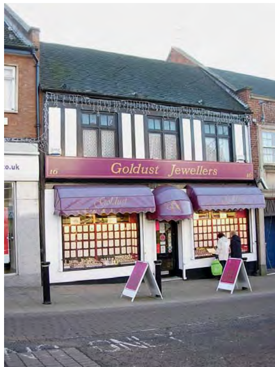
16 Market Place. Although this building suggests a traditional appearance, it is mid C20. The signage is overly large and the plastic canopies detract from its appearance.
