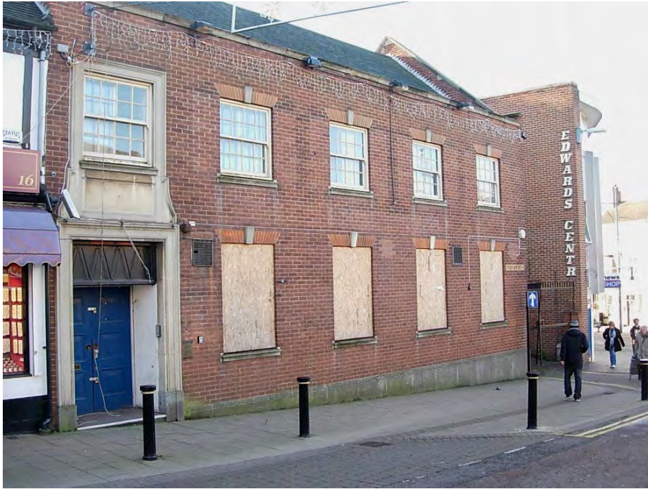
18 Market Place. This building which replaced the George Inn, forms part of a very large club building which has been vacant and boarded up for a long period. The proportions and stone details around the windows and doorway have given the mid C20 building, a semi traditional appearance.
