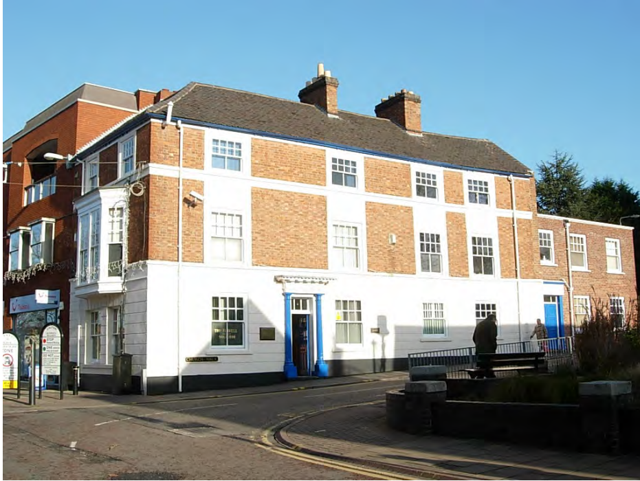
2 Market Place. This listed building is a very elegant structure and an important heritage asset. The first floor bay window adds significant character to both the Market Place and Station Road.
