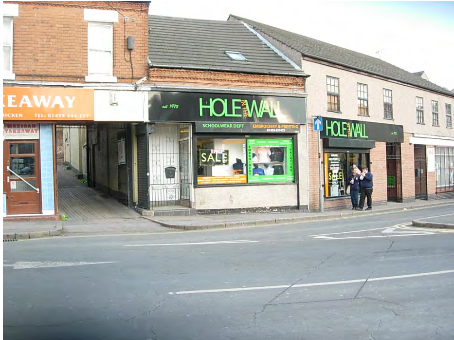
Although the original recessed entrance in this shop front has been retained, the oversized shop fascia and the concrete roof tiles detract from the appearance of this building.
