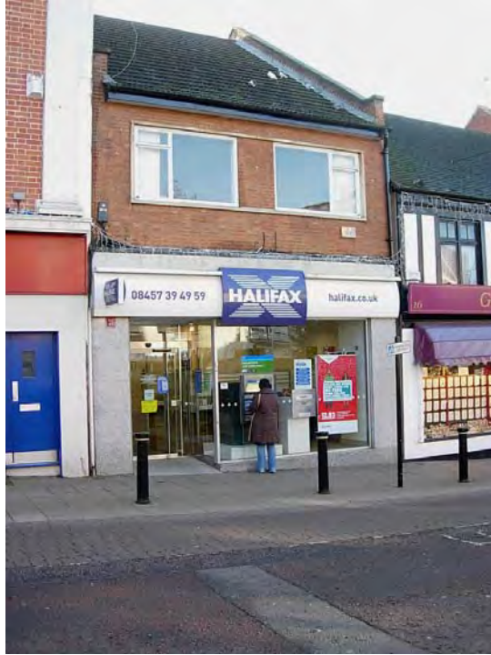
14 Market Place. This unremarkable mid C20 building occupies a significant location in the Market Place. The design has retained a traditional recessed entrance although the window proportions do not reflect the vertical proportions of most other traditional buildings facing into the Market Place.
