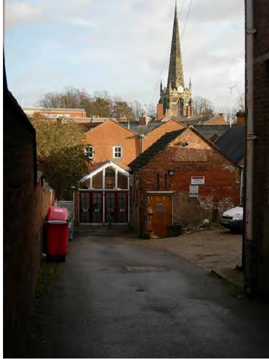
Trinity Yard. This jitty has a fine view of St Mary's Church. The buildings in the foreground require improved maintenance.
