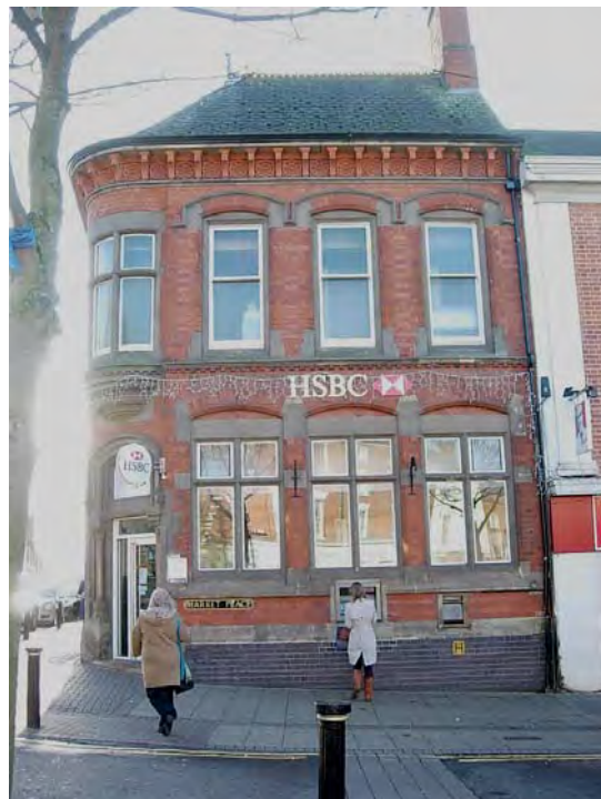
10 Market Place presents a very interesting frontage to the Market Place and successfully turns the corner with Station Road with a notable entrance and a hanging bay at first floor.
