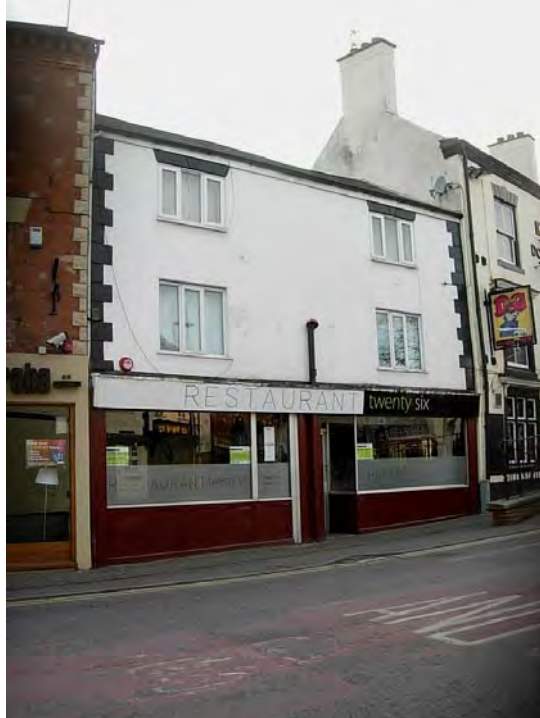
26 The Borough is a late C18 building that has a simple façade with a C20 shop front and windows which unfortunately detract from its appearance.
