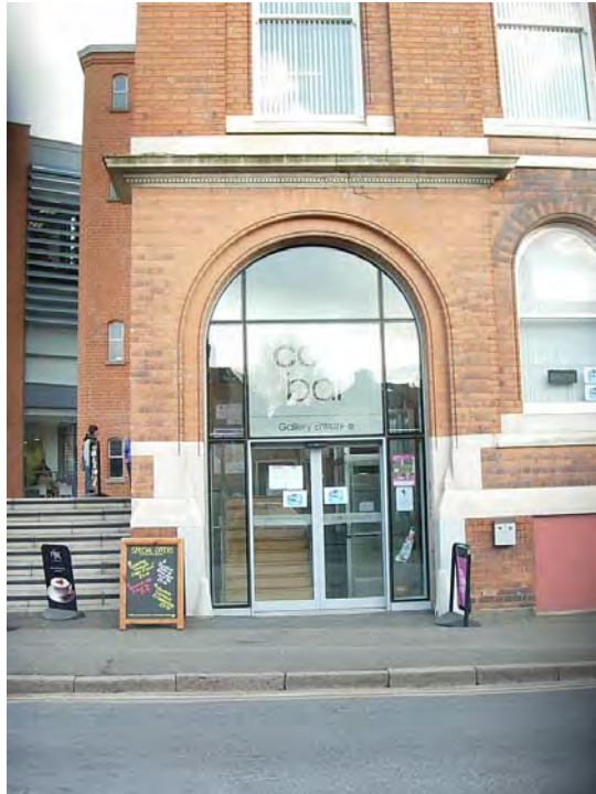
This secondary entrance into the ground floor of the Atkins building has a fine brick arch and stone jambs.
