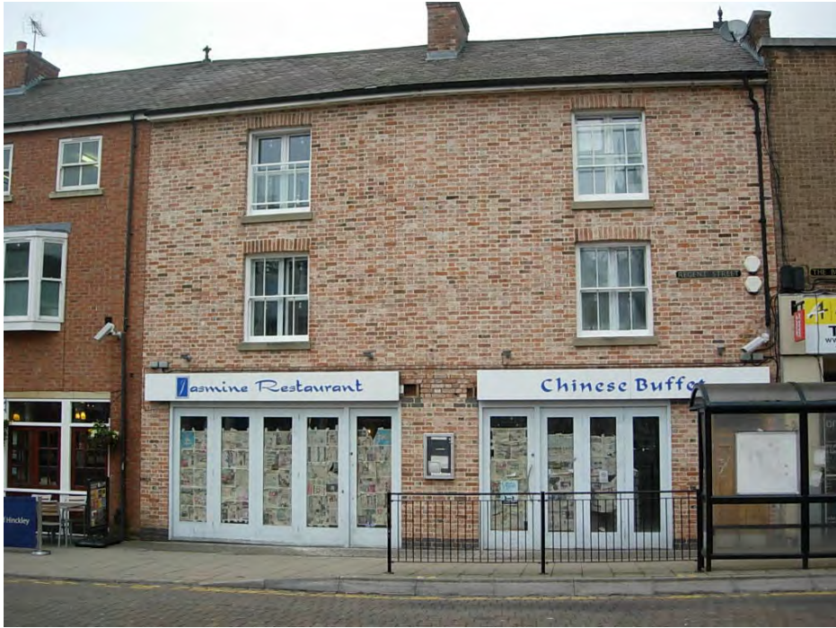
1 Regent Street, although recently rebuilt, includes a slate roof covering, central chimney stack, and sash windows at first and second floors with brick soldier course lintols.
