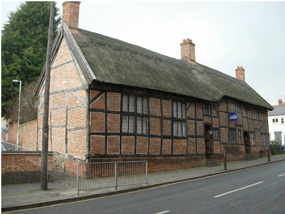
The Hinckley and District Museum occupies a range of 3 or 4 timber framed cottages, probably C17, which were restored in 1927-28 by the Atkins brothers and used as the company's board room. It is an important heritage asset.
