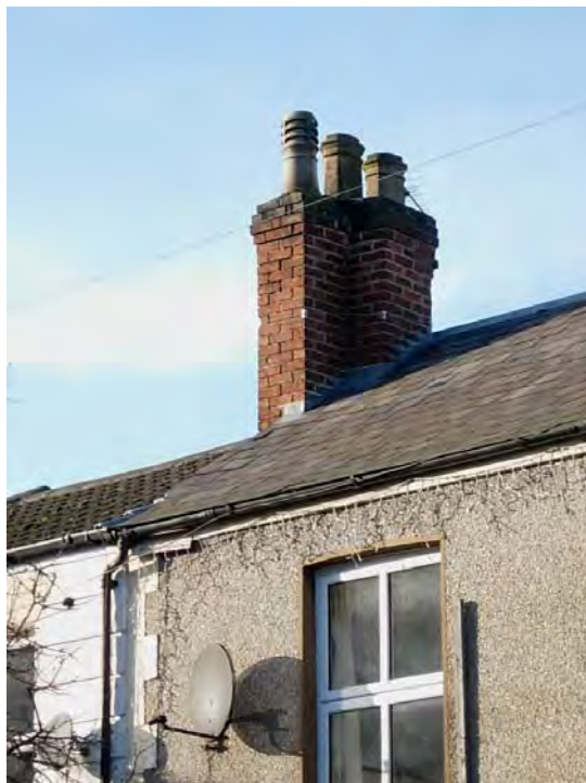
One of the few remaining properties on Regent Street that has retained its traditional chimney stack and pots. However this must be set against the detrimental impact of the street facing satellite dish and the plastic window.
