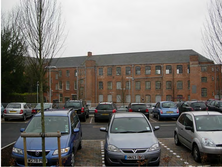
A distant view of the former Atkins factory, seen from the new College car park.
