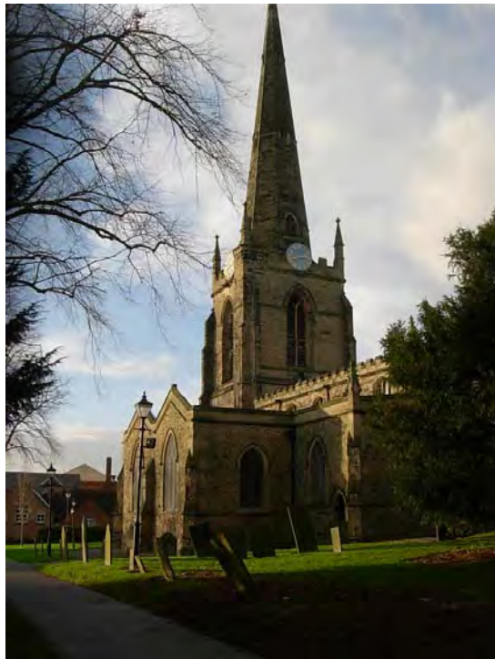
Views of the fine west tower of St Mary's Church add significantly to the character of the Conservation Area from wherever it is visible.
