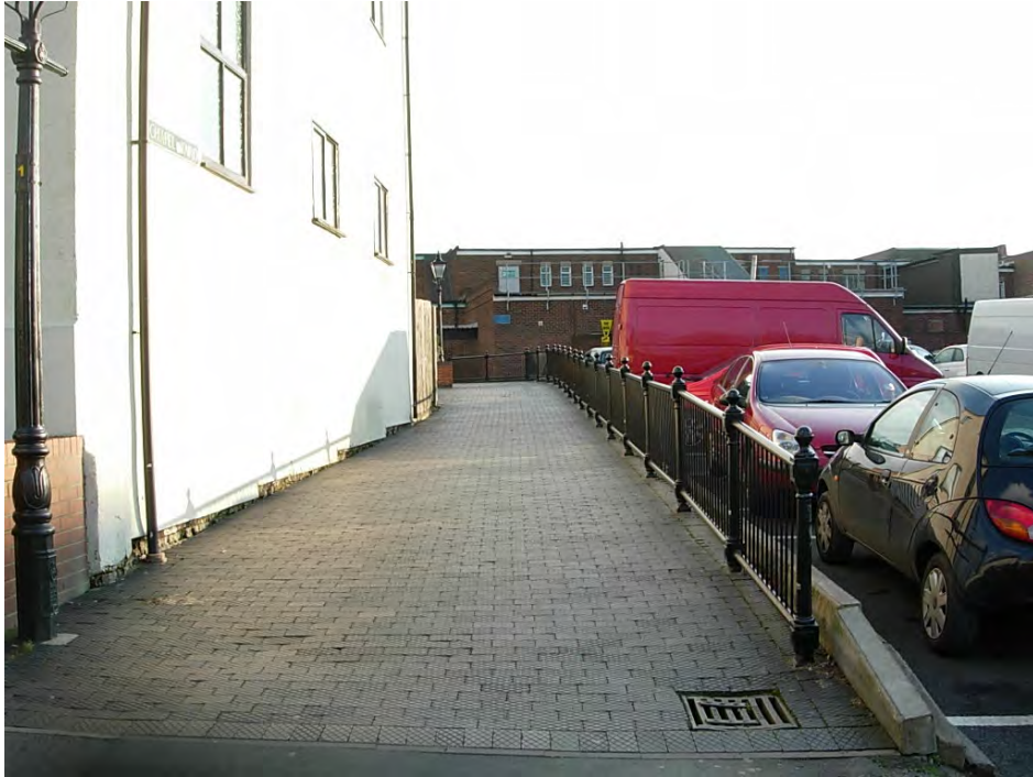
Chapel Yard jitty was recently surfaced with diamond pattern pavers and heritage lighting and the balustrade added.
