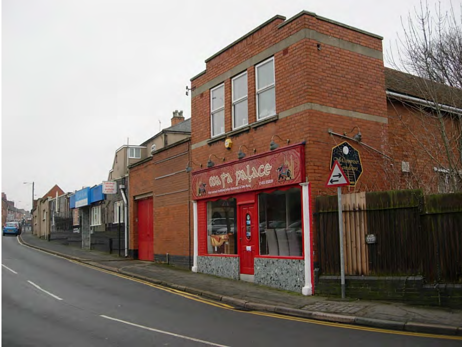
8 Holliers Walk is one of several poor quality buildings on this part of Holliers Walk.
