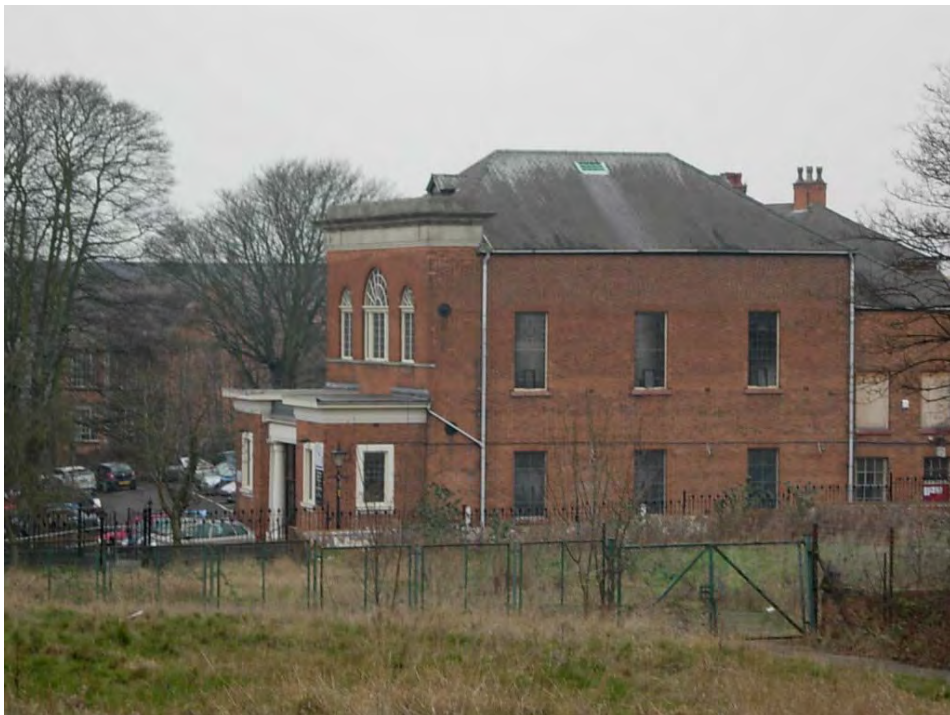
The flat roofed south porch built 1920-21 was constructed as a First World War Memorial at the Hinckley Baptist Chapel (built 1806-7)
