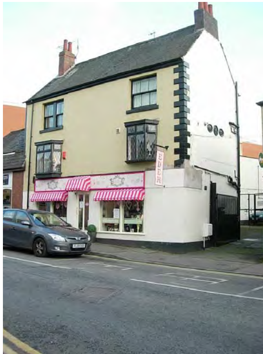
7 Stockwell Head was rebuilt in 1887. This building originally had a corner shop front which regrettably has been lost.
