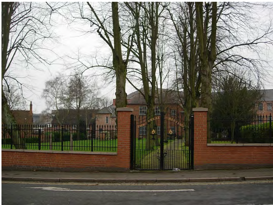
The rear access to the Great Meeting Unitarian Chapel yard. Although the yard has been cleared of grave stones, the space with its fine avenue of trees, is a key green area in the town centre and is very important for the setting of the Church.
