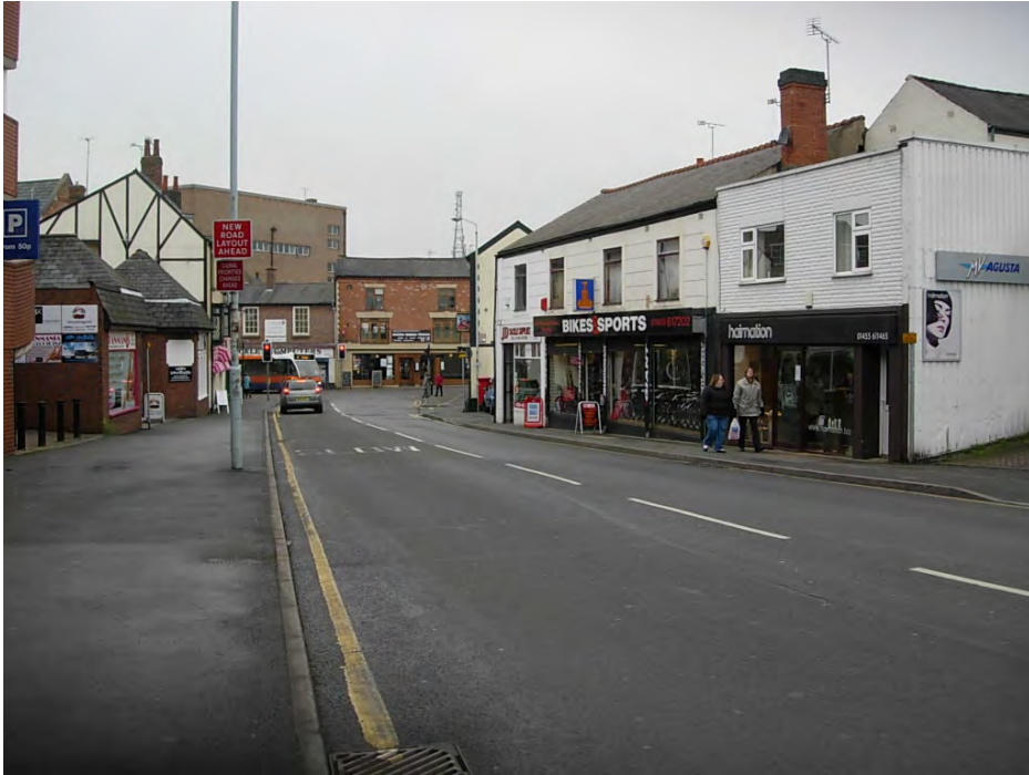
This view highlights the poor appearance of the Nationwide Building Society building which could be an important landmark building in the town centre.
