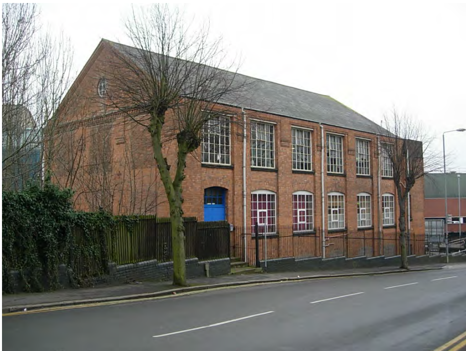
The north west elevation of the Concordia Theatre which unfortunately has had plastic windows inserted at ground floor. It was formerly part of the hosiery factory.
