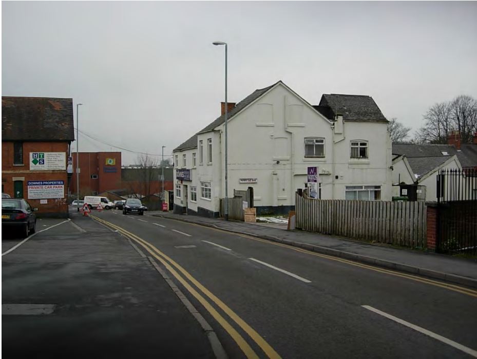
This view of Stockwell Head looking westwards, highlights the many open frontages which have a major detrimental impact on the street and the visitor experience.
