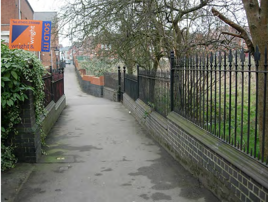
Baptist Walk showing the new low brick boundary wall with cast iron coping and decorative railings which formed the boundary to the former Bodycote factory. This is a most important jitty and heritage asset.
