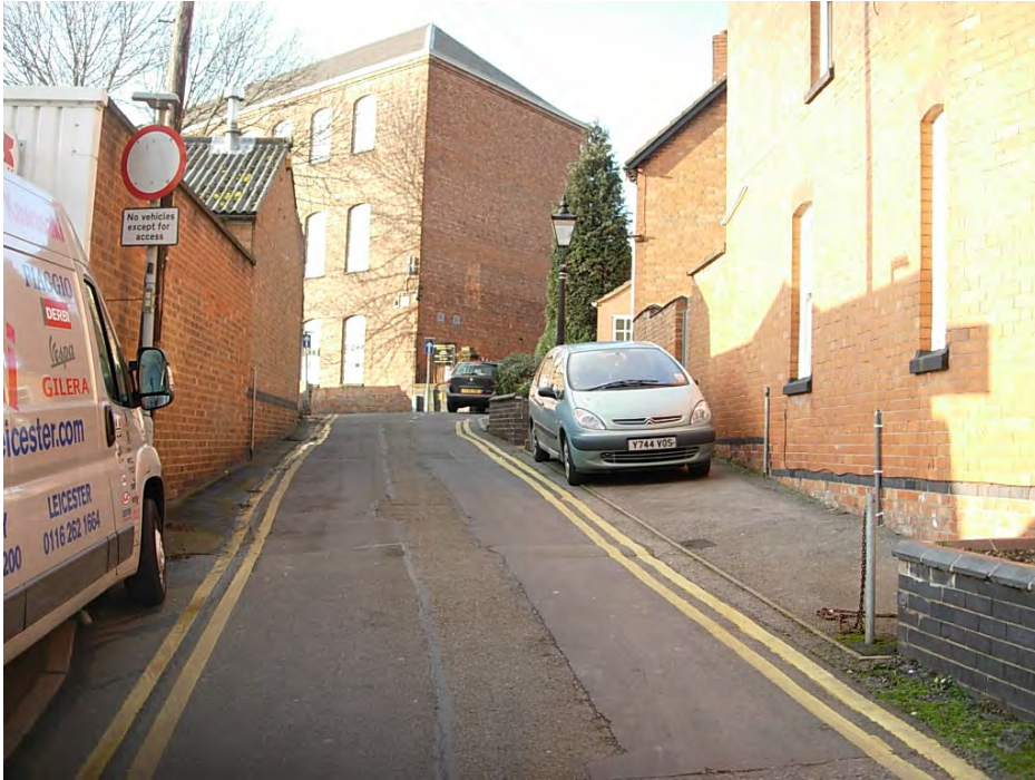
Baines Lane provides an important view of the listed former Atkins factory.
