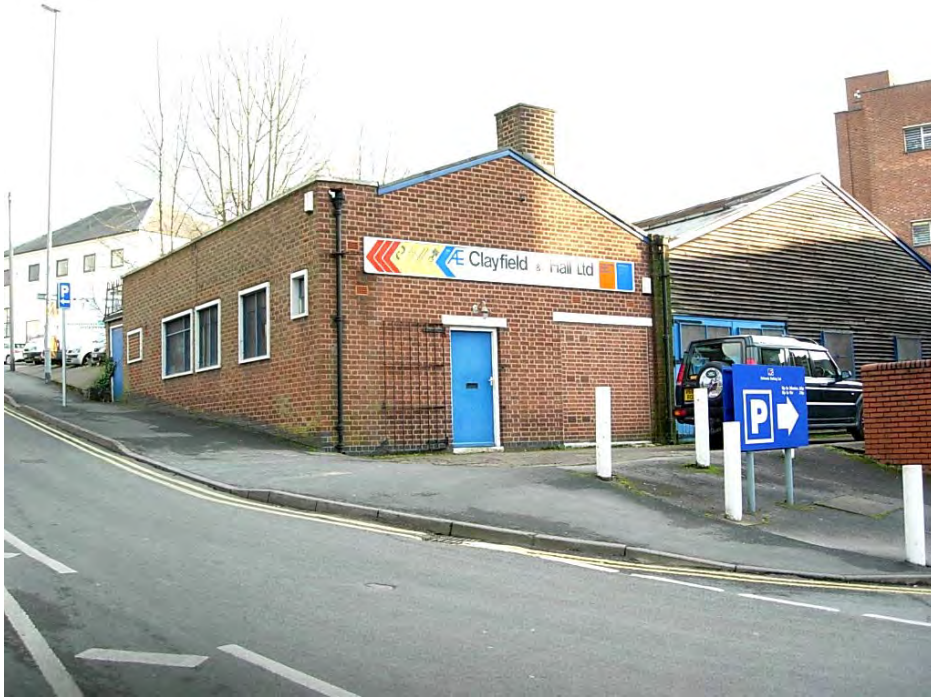
51 Stockwell Head is a former factory building with a timber clad extension dating from the 1950's.
