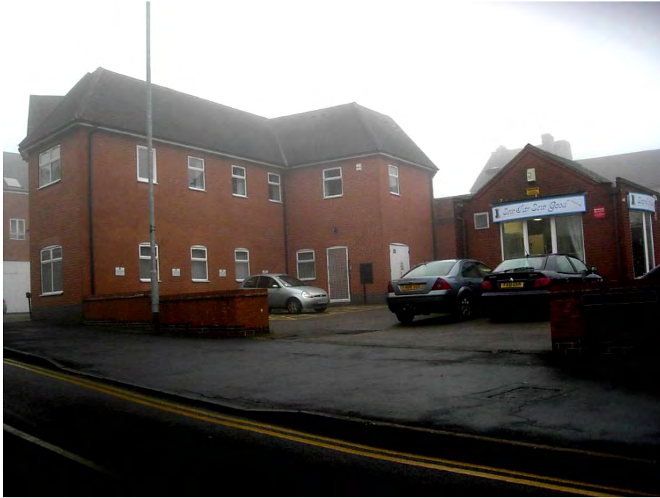
The rear of 6 New Buildings is a plain structure highly visible from Stockwell Head that adds almost nothing to the street scene.
