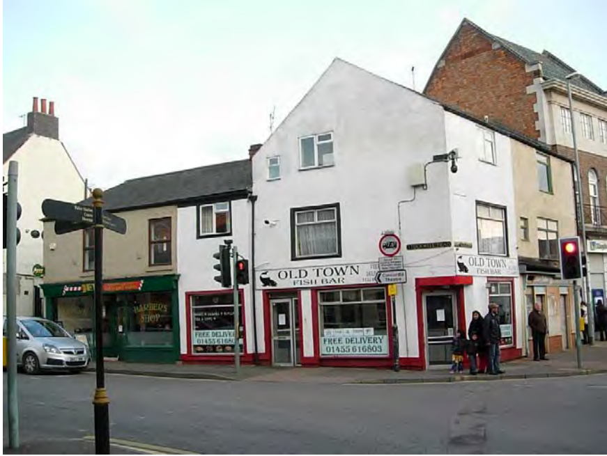
27 The Borough & 5 Stockwell Head have retained their slate roofs and some of their former sash window openings.
