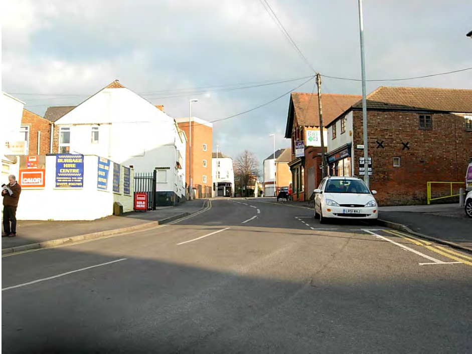
Stockwell Head looking east. This street has suffered in the recent past through inappropriate demolition and the construction of poor quality frontages.
