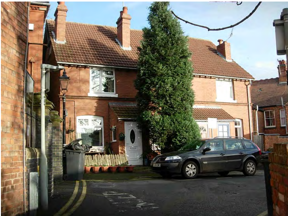
The terrace, 2-6 Baines Lane, was originally constructed by the trustees of the Unitarian Chapel. The partial loss of the end chimney stack is unfortunate.
