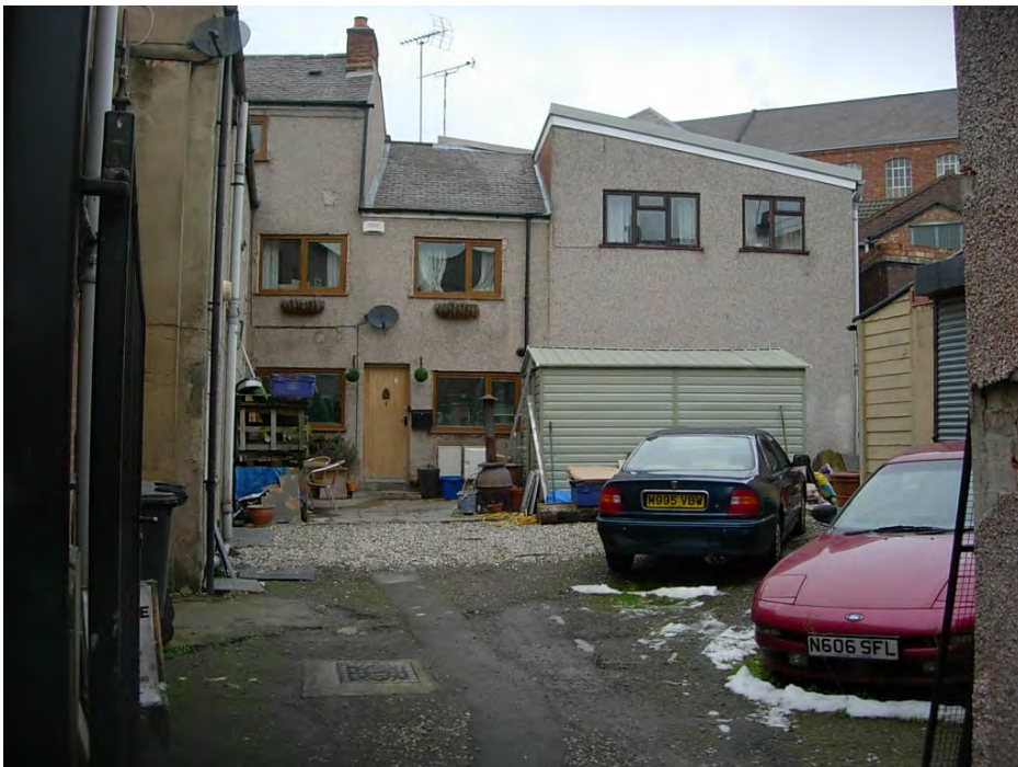
Brooke's Yard was the original location of the manufacturer of Brooks bicycle saddles. Unfortunately the poor ground surfacing, the clutter and the incongruous built form detracts from the appearance of this important historic yard.
