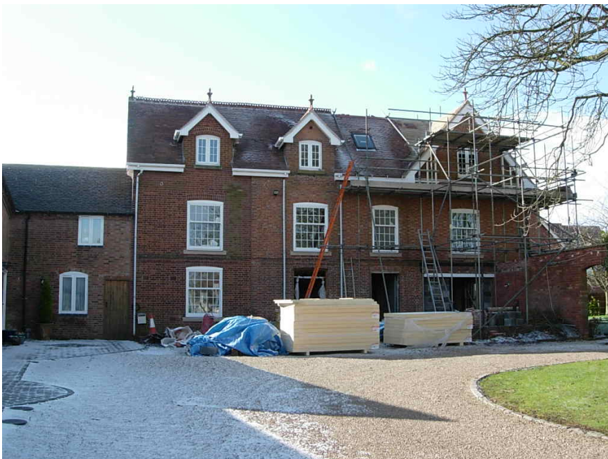
Park House is a large detached property. This former farmhouse is set in large grounds and is currently undergoing major refurbishment.
