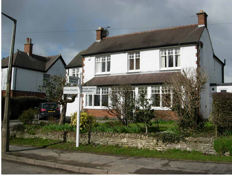
48 Station Road has retained its slate roof, roof ridge tiles and gable end chimneys
