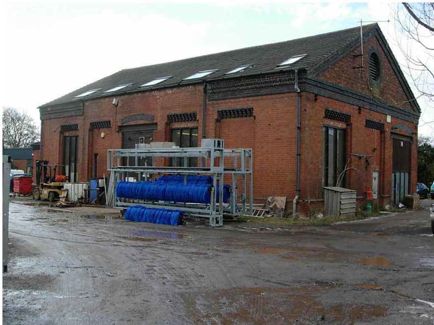
The roof lights inserted in the former engine shed are modern additions which tend to devalue the character of this fine building. It is important that buildings at this former railway complex are retained in their original form where possible.
