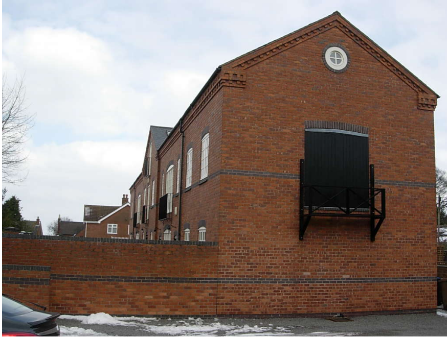
The Barracks, sited to the rear of the George & Dragon Public House off Station Road, is a modern block of flats built in 1995. The property was built to reflect a stable block with dental course detailing along the eaves and on the gable end.
