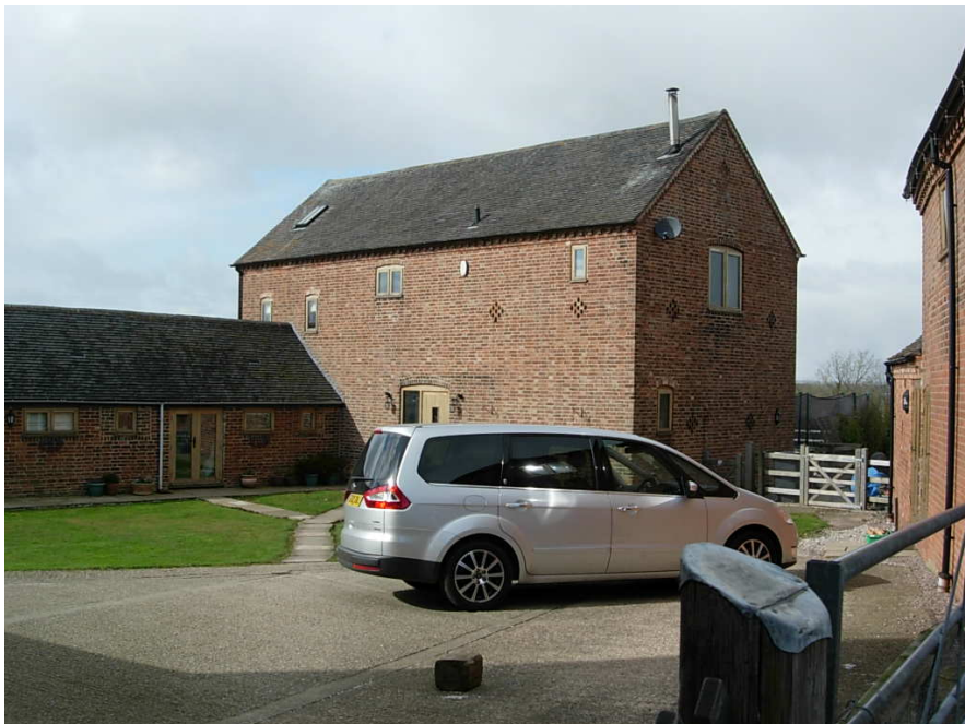
One of the out buildings to the rear of Crown Hill Farmhouse successfully converted into a dwelling.
