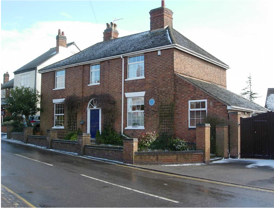
31 Station Road is an excellent large imposing property that was once the former grammar school. Unfortunately, the side extension with its mono pitched roof tends to spoil the symmetry of the property.
