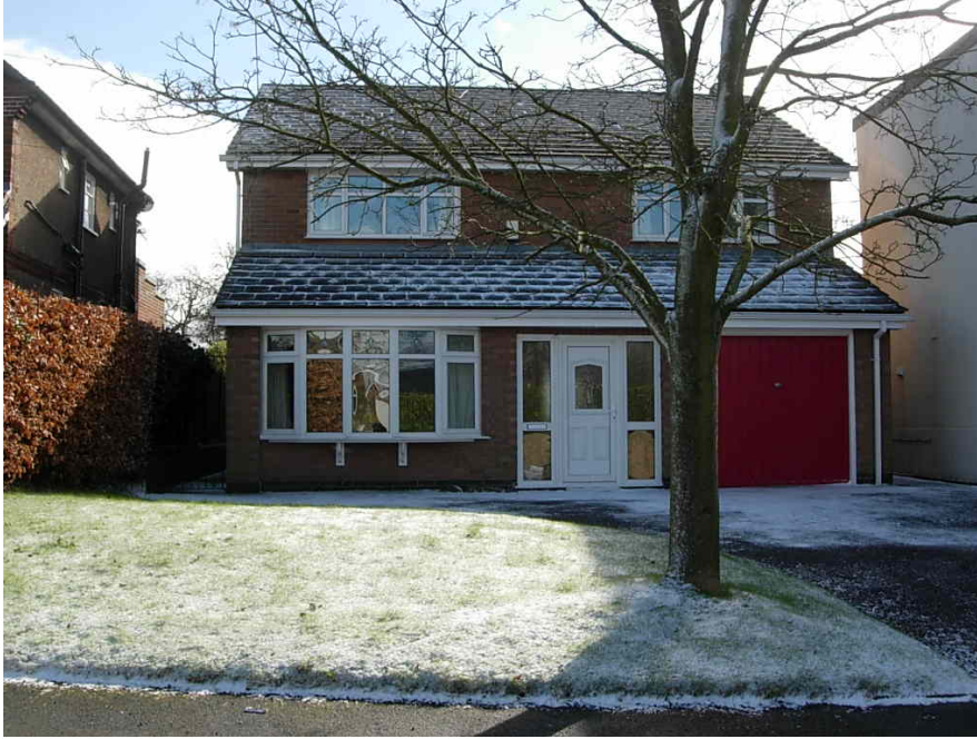
27 Station Road is a modern detached dwelling that does not reflect the character of the Conservation Area.
