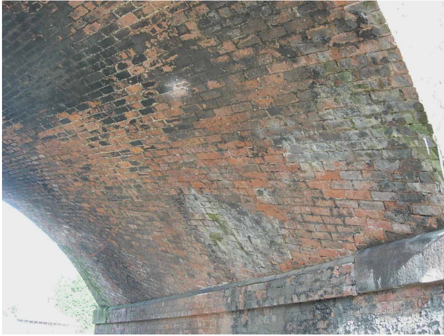
View of the underneath of the railway arch at the Upton Lane road bridge. The bricks in the arch have been laid at an angle to the bridge abutments.
