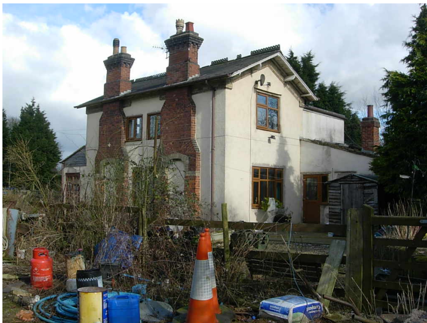
Although the property 'The Willows' on Upton Lane has been considerably modernised it still retains some interesting features including its imposing chimney stacks. The property was originally the Station Master's house.
