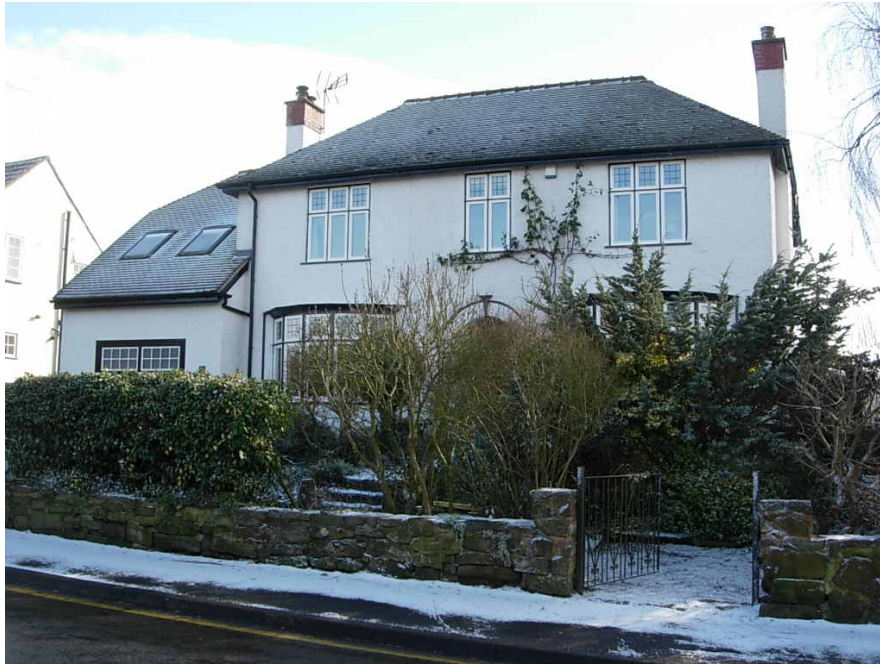
23 Station Road is a pleasant dwelling fronted by mature planting that helps soften the street scene. If possible, the roof lights in the garage should have been inserted on the rear elevation away from public view.
