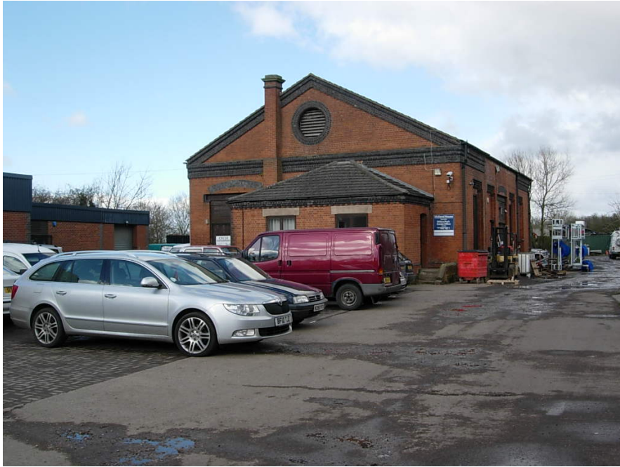
The old railway engine shed is now used for industrial purposes.
