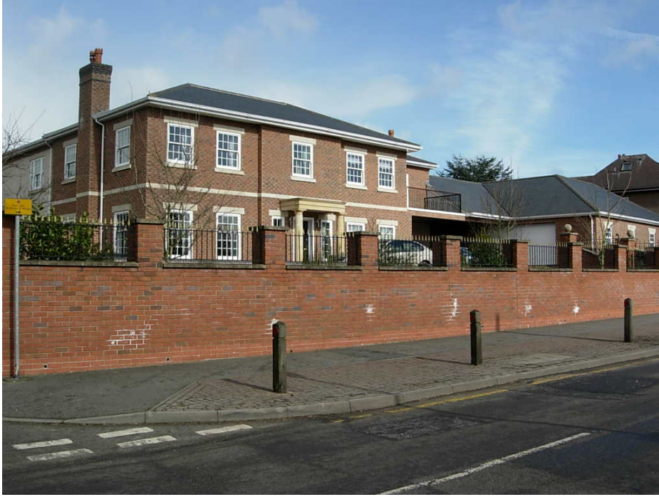
26-28 Station Road was originally a factory that has been substantially re-built on its front elevation using modern bricks.
