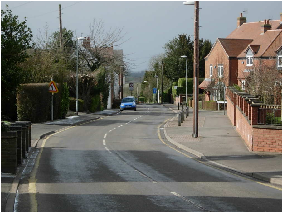
View looking westwards down Station Road. The chicane and highway signage detract from the attractive views to open countryside and should be reconsidered by the Highway Authority.
