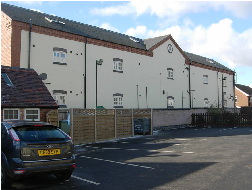
It is unfortunate that the rear of the Barracks has been rendered and not built entirely in brick. The roof lights would have been less prominent if they were recessed into the roof
