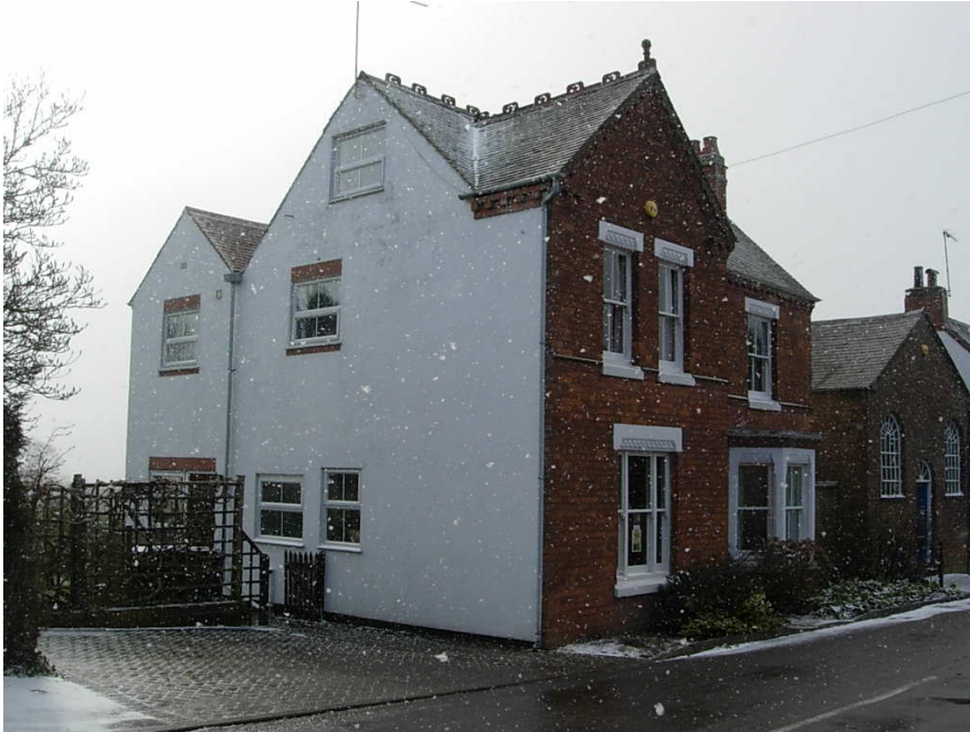
45 Station Road is a large detached residence that has lost some of its elegance with the modified window openings and rendering on its eastern elevation.
