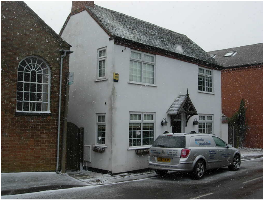
49 Station Road is a character property that has retained its gable end chimney stack.
