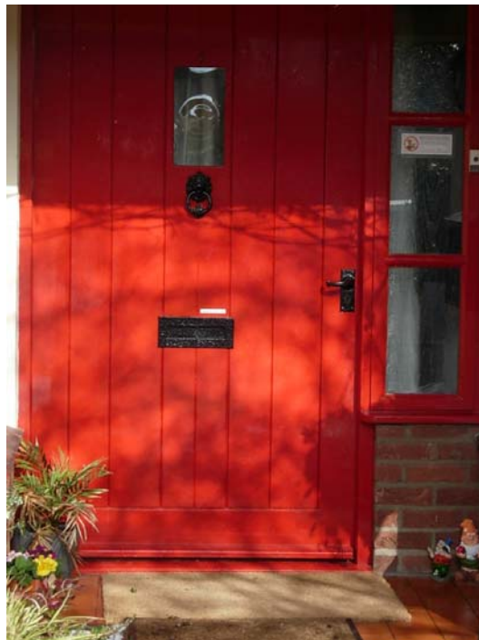
The wide paneled door on The Old Forge.
