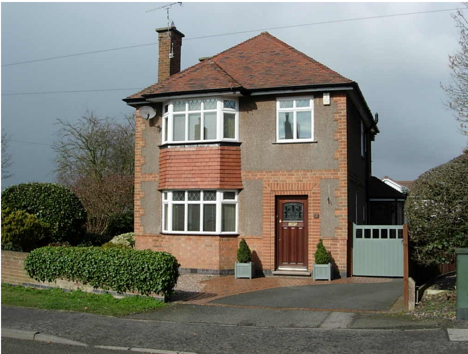
16 Station Road is a typical inter-war dwelling with clay roof tiles and a two storey bay window.
