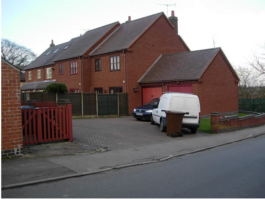
This parking area servicing the properties 7 – 11 High Street has destroyed the traditional enclosure of the street to the detriment of the Conservation Area
