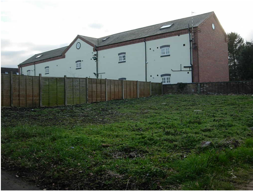
The rear of the Barracks viewed from Church Walks.
