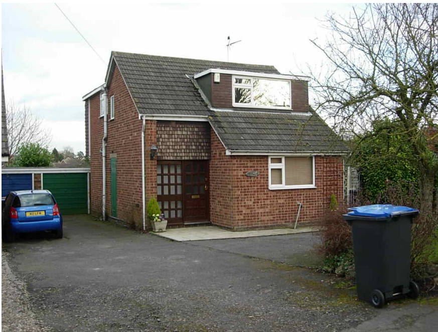
The property, Springbank, is a modern dwelling that does little to enhance the quality of the Conservation Area by way of its large dormer window and flat roof rear extension.
