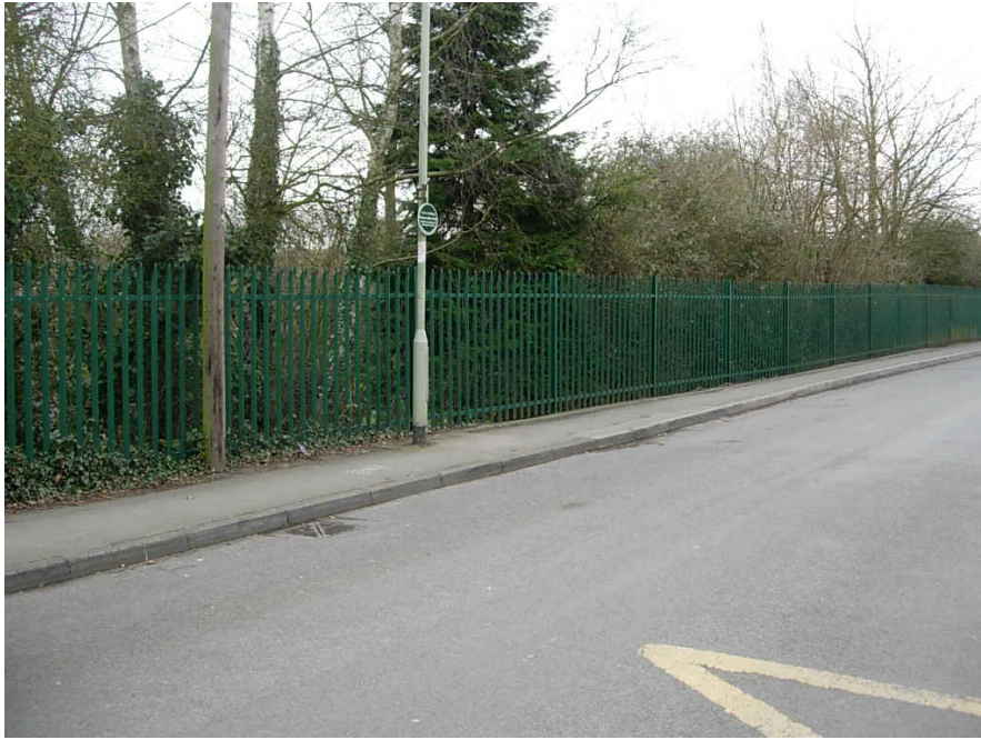
The palisade fencing running along High Street needs to be replaced with traditional railings.
