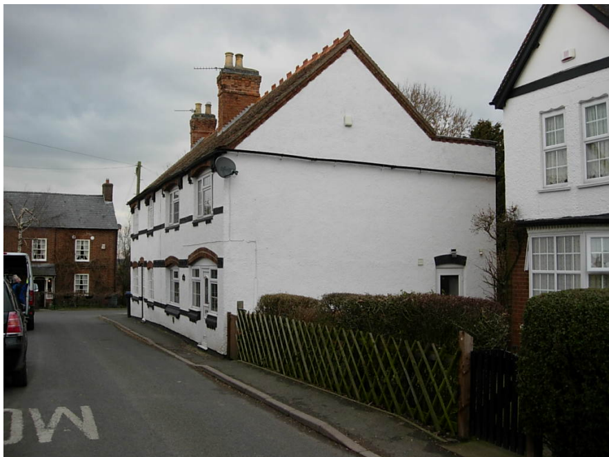
The gable end of The Cottage showing the property appears to have had a small rear extension built at sometime in the past.
