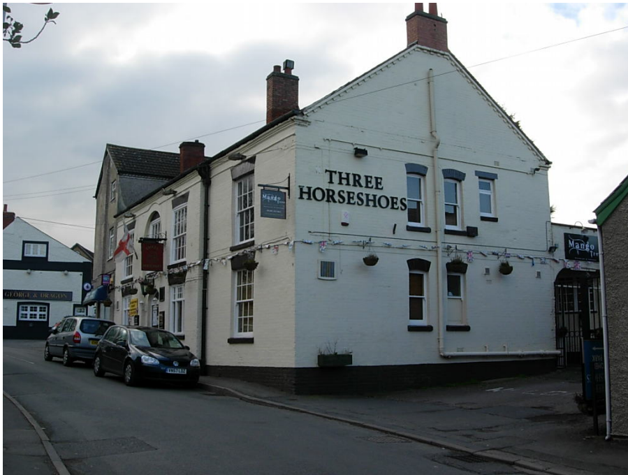
The imposing gable end of the Three Horseshoes pub adds to the character of the Conservation Area.
