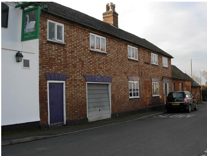
The integral garage inserted in this dwelling is an incongruent feature that detracts from the visual quality of the property.
