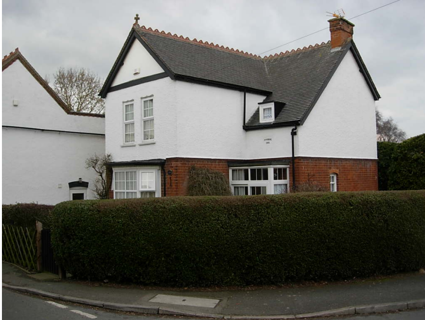
Ivydene is an attractive detached property on the corner of High Street and Roseway built in red brick up to the first floor. The property has a slate roof with ornate ridge tiles and is enclosed with a high privet hedge.
