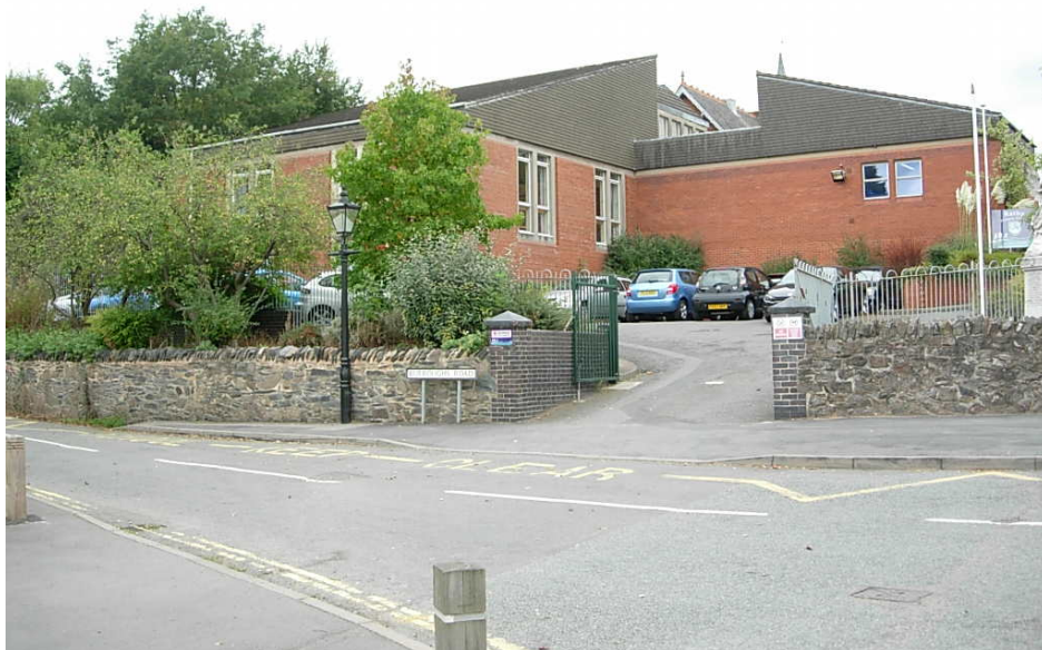
The modern extension to Ratby Primary School is built in red brick with mono-pitched roofs. It is unfortunate that the modern extension has now obscured the excellent side elevation of the Victorian school.
