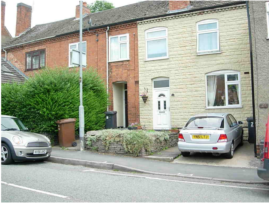
The concrete cladding and roof tiles used at 22 Main Street are a poor substitute to the original materials and breakup the uniformity of the terrace.
