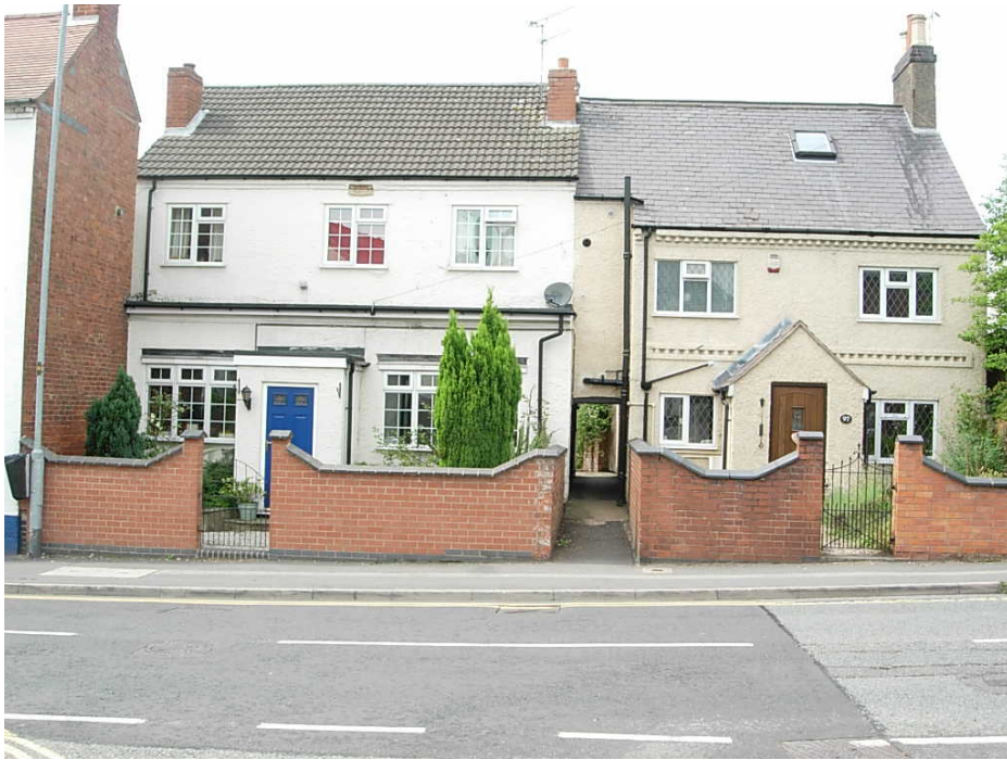
The property 95 Main Street was once the Earl of Stamford Arms Public House. The property has been considerably modernised with bow windows, concrete roof tiles and the chimney stacks reduced in height. The front of 97 Main Street has been painted and a roof light installed. The central passageway between the two properties once accessed Stamford Arms Yard.
