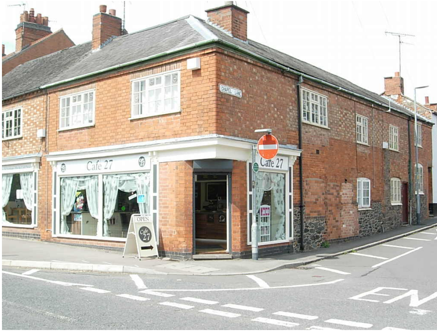
The property sited on the corner of Station Road and Chapel Lane has been a shop for a considerable period of time.
