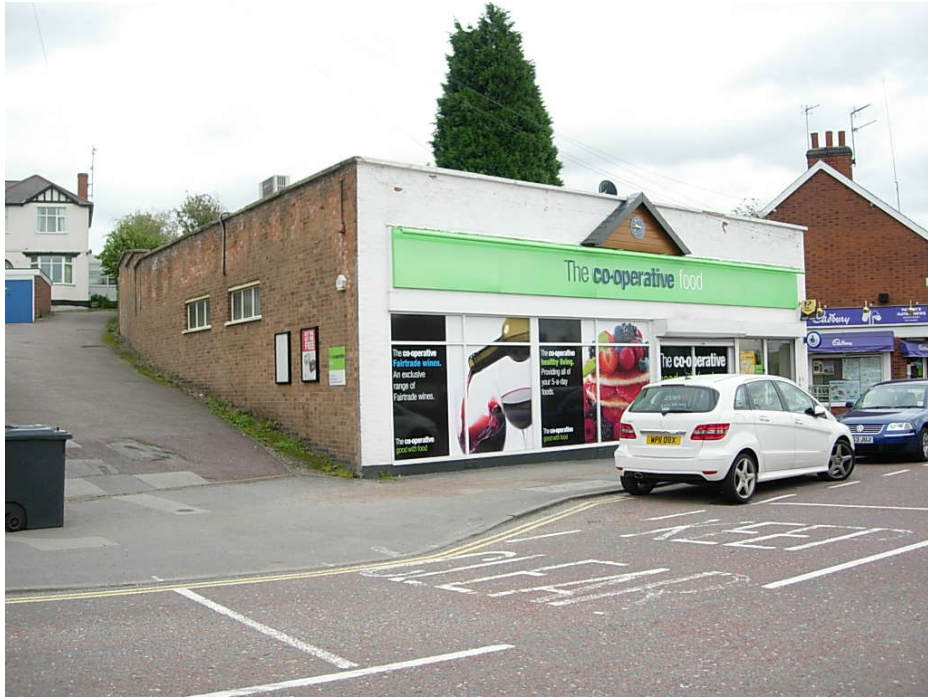
The Co-Operative store is an important village facility, however its design and dominant shop front treatment is a poor closing feature standing at the junction of Main Street/Station Road/Desford Lane.
