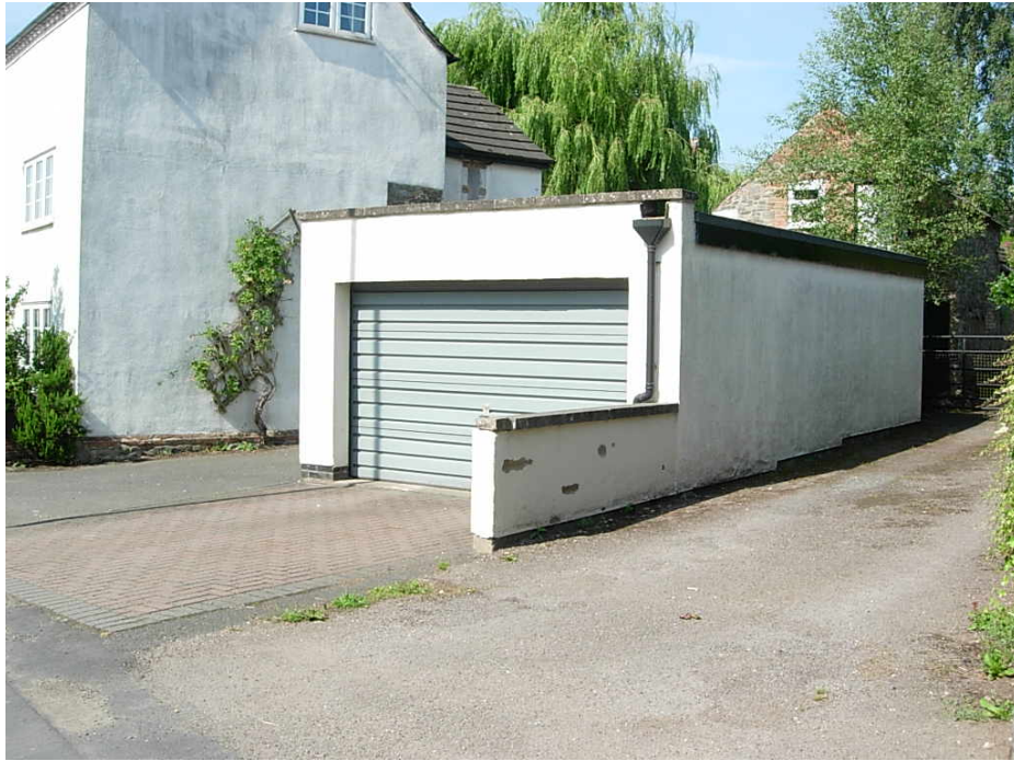
This flat roof garage with its double door, adjacent 107 Main Street is a poor visual feature at the entrance to the Conservation Area.
