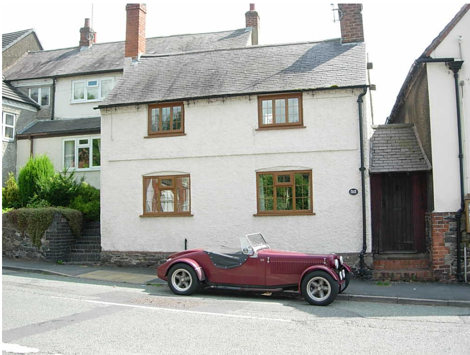
52 Main Street is a detached property that is sited on the back edge of the pavement. The dwelling that has been rendered still retains its stone plinth and gable chimney stacks.
