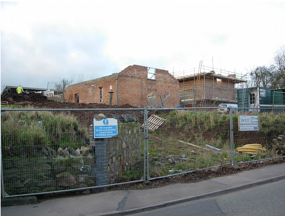
9 and 11 Main Street during their conversion work into residential properties.
