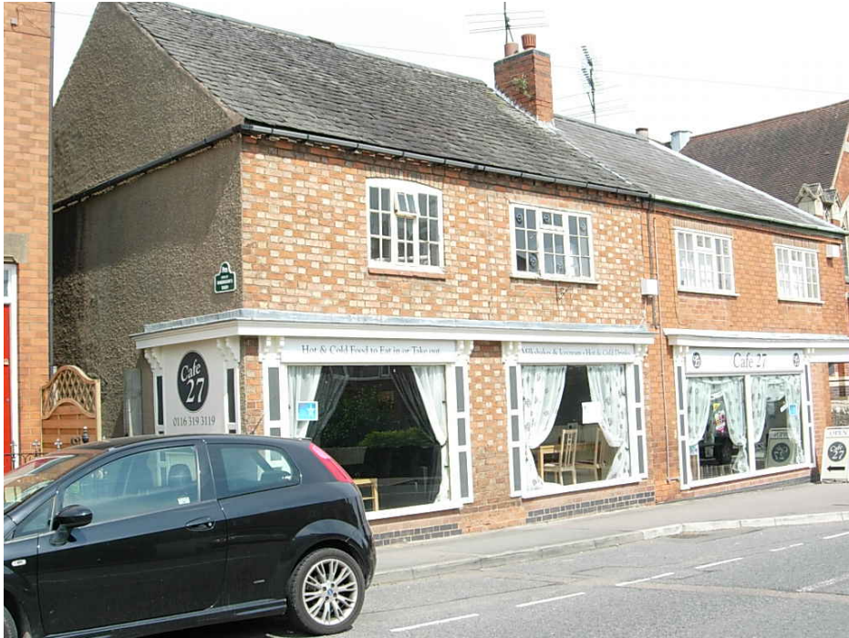
This property, 21 Station Road, has recently been converted into a café.
