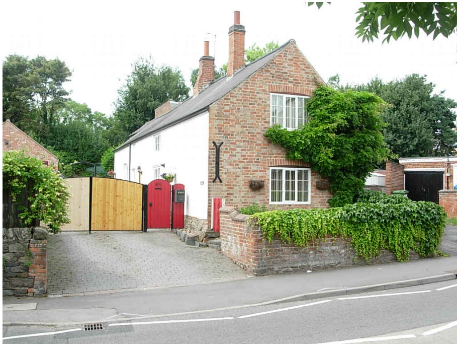
The Grade II listed building, 85 Main Street, is a large cruck-framed dwelling probably built early in the C17. The property is built in red brick, although its southern elevation has since been rendered, and has a plain tiled roof which replaced the original thatch roof covering. It has retained its brick ridge chimney stacks.
