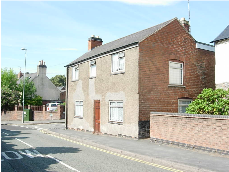
103 Main Street is a simple detached property sited on the corner of Main Street/ Stamford Street. The dwelling, built in red brick, has been rendered on its front elevation and has aluminum windows. It was originally a timber framed cottage of great character.
