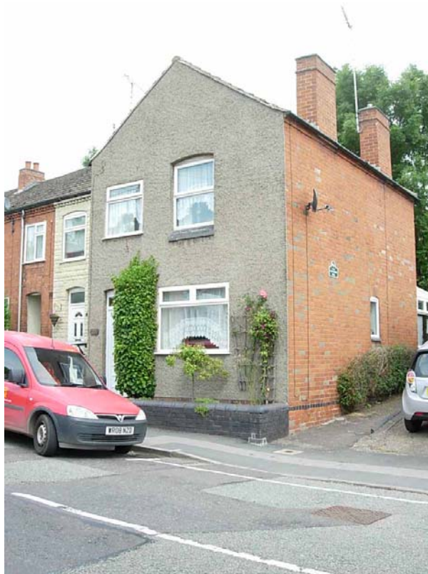
The front room to the large dwelling 20 Main Street was once the village post office. No doubt when the property was fully converted to residential, its frontage was rendered to conceal the conversion work.
