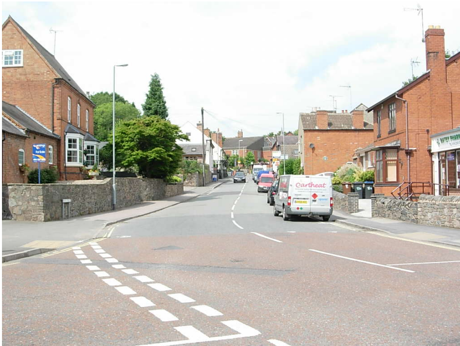
Ratby Primary School terminates views looking northwards up Main Street. Red/orange brick is a prominent building material in Ratby.
