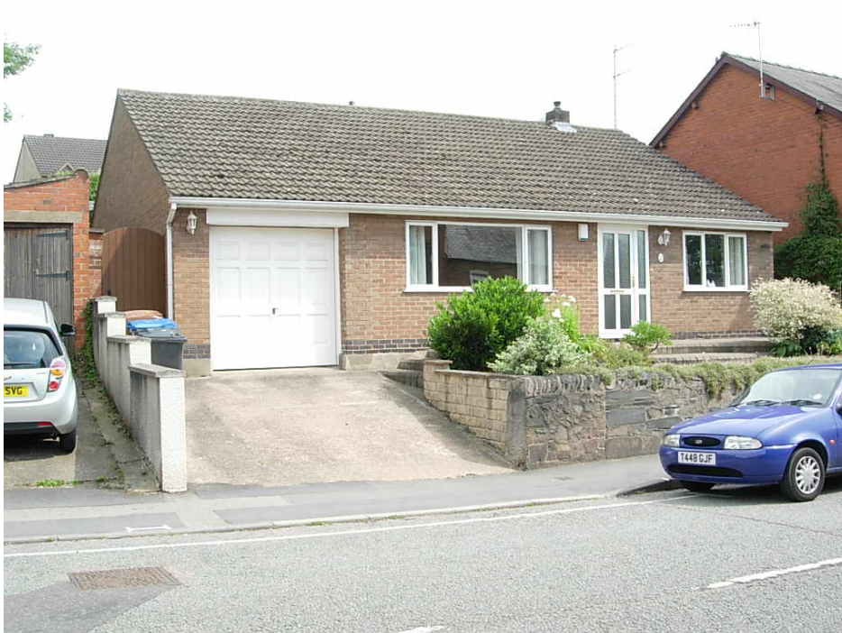
12 Main Street being of modern design and materials with an integral garage doesn't sit comfortably in the Conservation Area.
