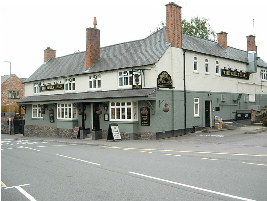
Bulls Head Public House, originally a farmhouse, is a large prominent building on Main Street that has been considerably extended and modernised. The extension on its northern elevation is built at a greater height to the original property due to the topography of the ground and this is reflected in different roof heights. The property still retains its stone plinth and prominent chimney stacks.
