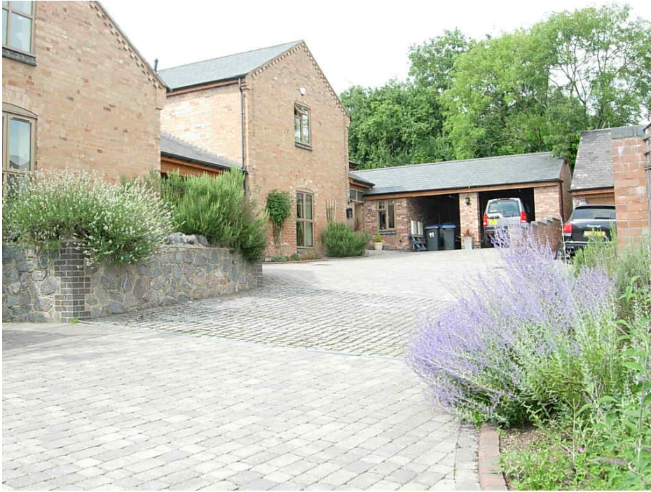
9 and 11 Main Street have been converted from barns into two large dwellings.
