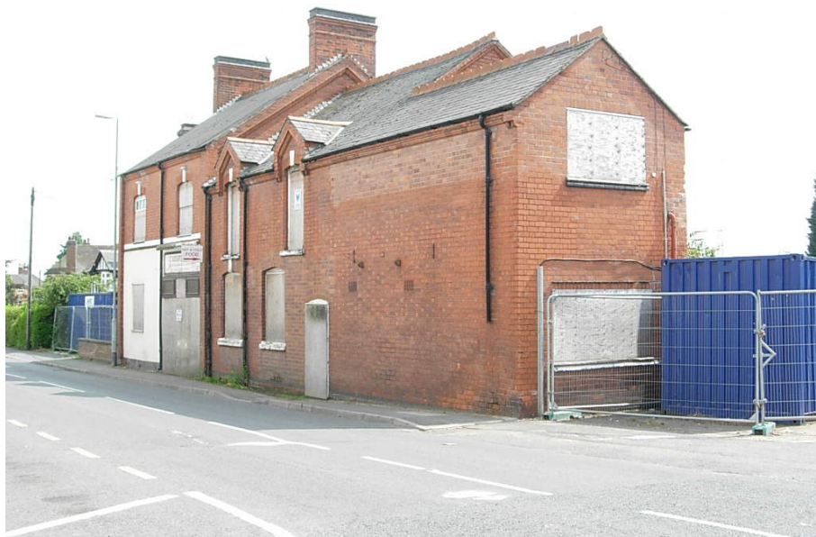
The former Geary's bakery shop, although not situated in the Conservation Area, is an important building as it provides enclosure at the entrance into the Conservation Area. Every effort should be made to retain this property.
