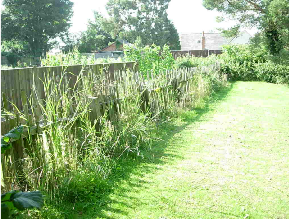
The timber fence running along the rear boundary to the Ratby Library is a poor feature that would benefit by being replaced with a traditional granite wall.
