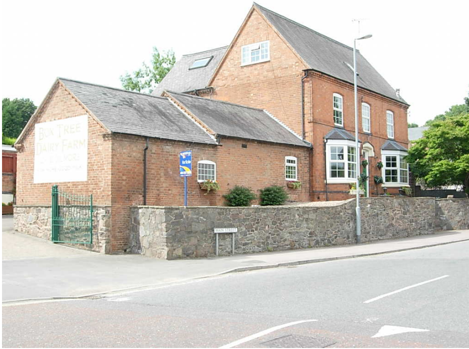
Box Tree Farm and its outbuildings are important features sited at the junction of Main Street and Desford Lane. The property has ceased to be a farm and unfortunately, it has lost its previously dominant chimneys and been restored using plastic windows and prominent roof lights.
