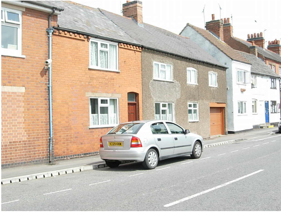
5 Station Road is built in red brick with a slate roof and has a fine dental course. The dwelling, 7 Station Road, has had its window openings altered and an integral garage constructed which is the reason why the front of the property has been rendered.
