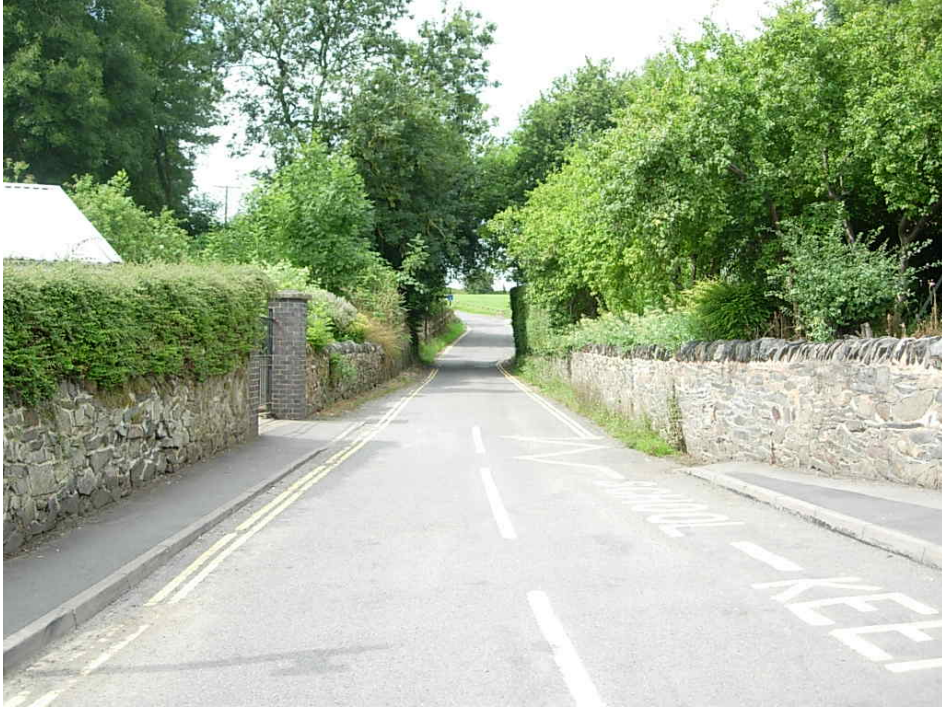
Excellent view looking westwards along Burroughs Road. This narrow lane that was originally an old coaching road is flanked by granite walls softened by foliage
