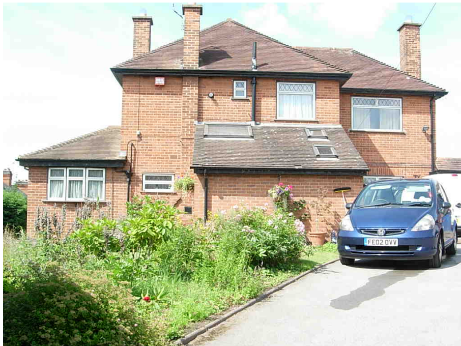
19 Berry's Lane is a large detached dwelling approached from a long drive.
