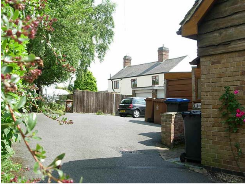
A view of the entrance to No. 24 and 26 Chapel Lane. No. 24 is a two storey dwelling that has retained its chimney stacks.
