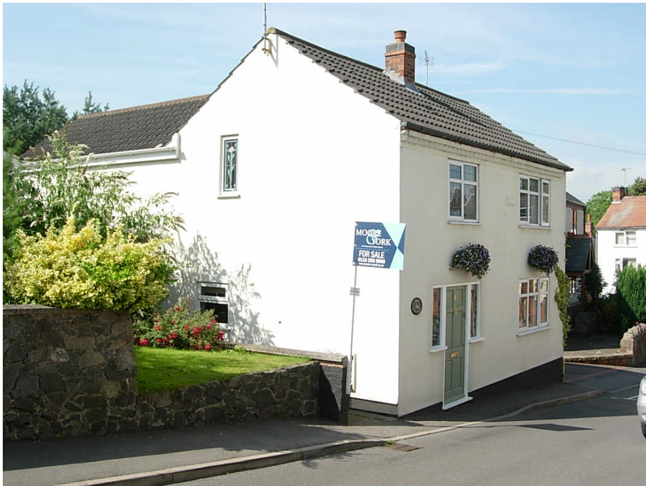
8 Church Lane is a detached cottage that has been considerably modernised with a large rear extension, plastic windows, rendered walls and concrete roof tiles.
