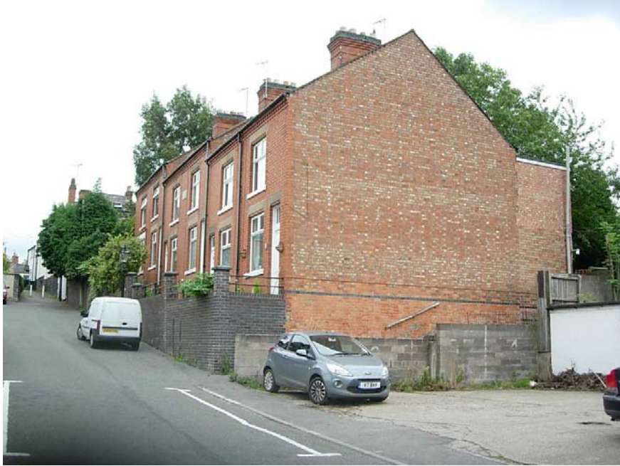
The gable to the block of the Victorian dwellings 8–18 Berry's Lane, built in 1898, is a prominent feature. The concrete block wall running down the side boundary of the Chinese take-away car park is an incongruent feature in the Conservation Area.
