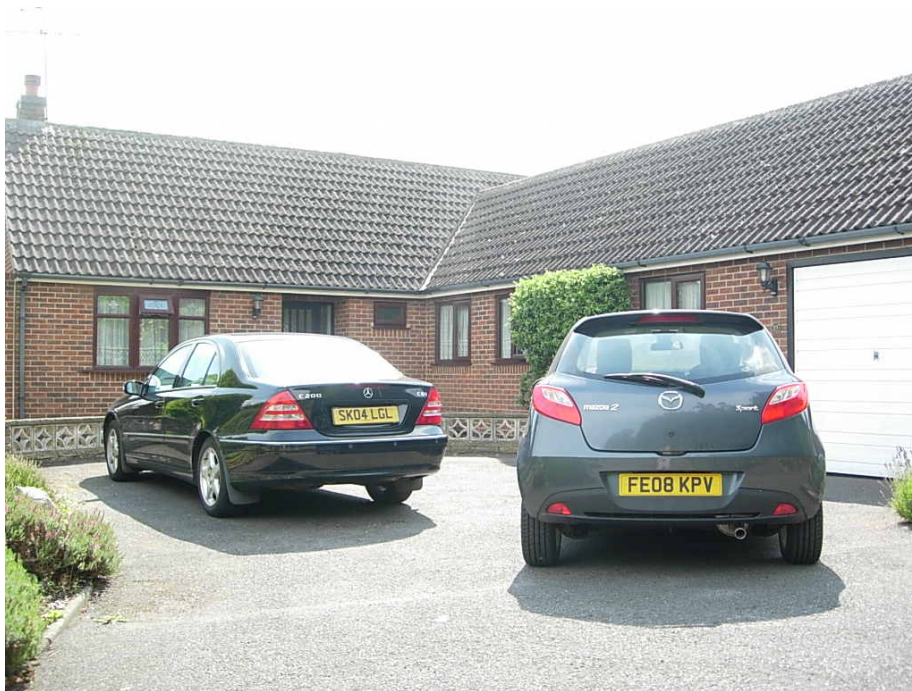
Concrete roof tiles, plastic windows and metal garage doors do not compliment the traditional character of the village Conservation Area.
