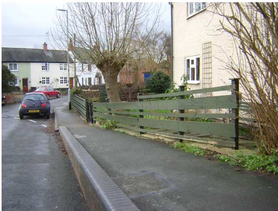
The timber fence fronting 68 Church Lane is visually poor. Consideration should be given to replacing it with a traditional stone or brick wall.
