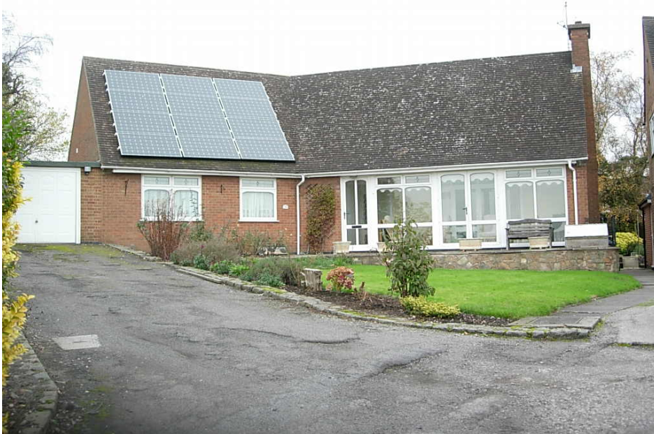
The solar panels on the roof of 34 Chapel Lane dominate the front elevation of the bungalow. Where possible solar panels should be located on rear elevations away from public view.
