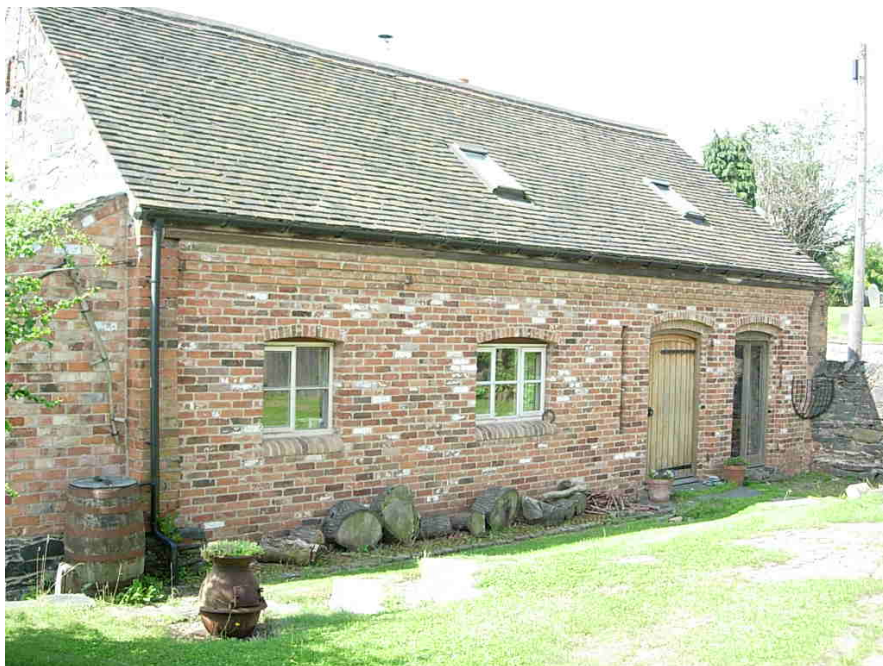
This property, once linked to Woodley Farm, has been converted to residential use. The roof lights would be less prominent had they been recessed.
