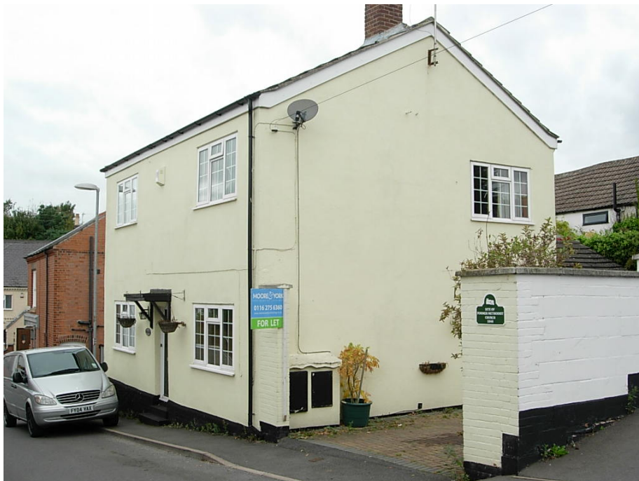
1 Church Lane is one of Ratby's core semi-detached dwellings that have also been considerably modernised and now converted into one dwelling. Its window openings have been enlarged, the front door centralised, walls rendered and re-roofed with concrete tiles.
