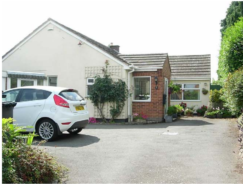
The form, materials used and detail design of these two bungalows are contrary to the traditional qualities of the Conservation Area.
