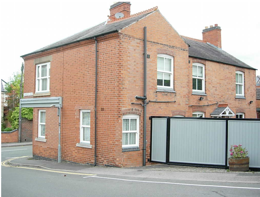
The high timber fence to the rear of 88 Main Street is not in keeping with the traditional character of the property.
