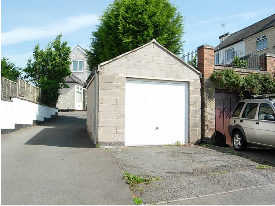
The materials of this garage are unsympathetic to the Conservation Area.
