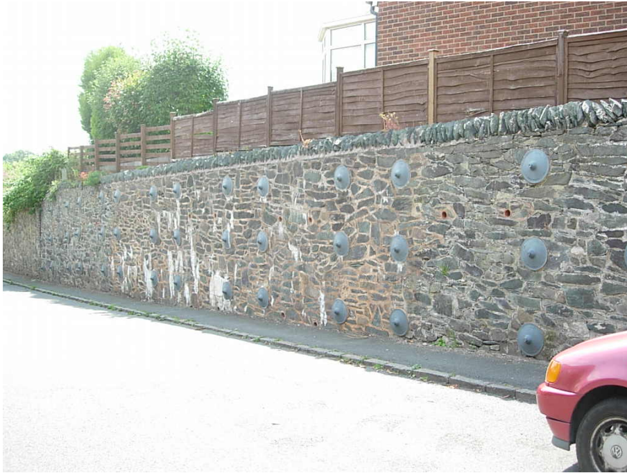
This stone and slate wall has been carefully stabilized with steel plates which, in their own way, add character to the Conservation Area.
