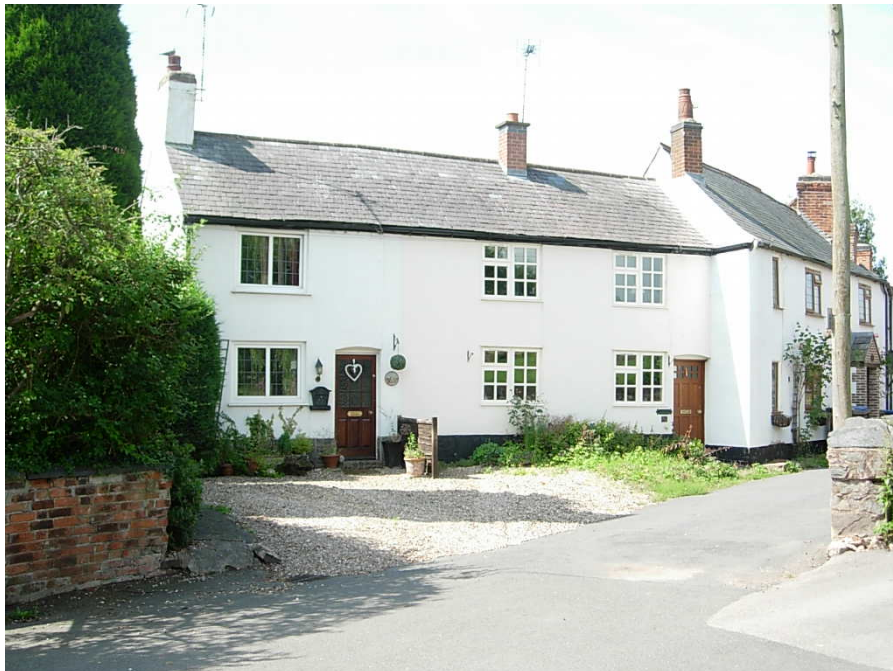
This view highlights the detrimental impact that different styles of window can have on terraced properties.
