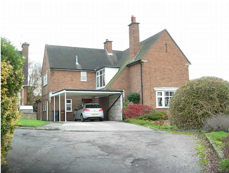
The scale of the dormer structure and flat roof car port at 32 Chapel Lane tend to dominate the appearance of the traditional period property.
