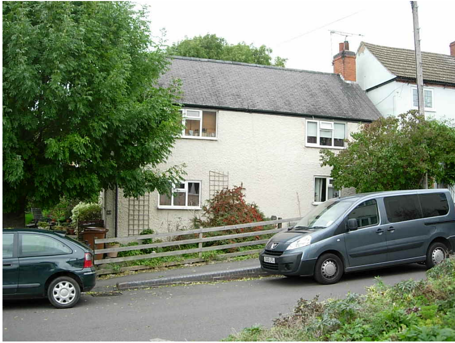
68 Church Walk is a rendered property that has had its window openings enlarged. However, the dwelling still retains its slate roof and gable chimney stacks.
