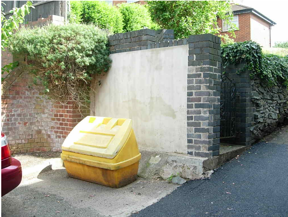
This brick wall on Berry's Lane was recently improved by the Borough Council as a project identified in the previous Conservation Management Plan.
