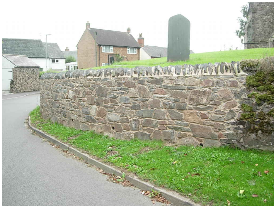
This section of churchyard wall on Church Lane has recently been rebuilt as a project put forward in the previous management plan review. The granite churchyard wall is an important feature in the Conservation Area and every effort should be given to ensure its retention.
