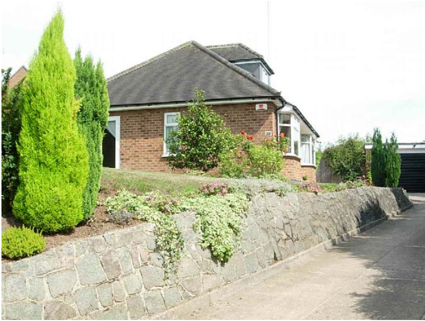
28 Chapel Lane is a modern dormer bungalow set back from the highway.
