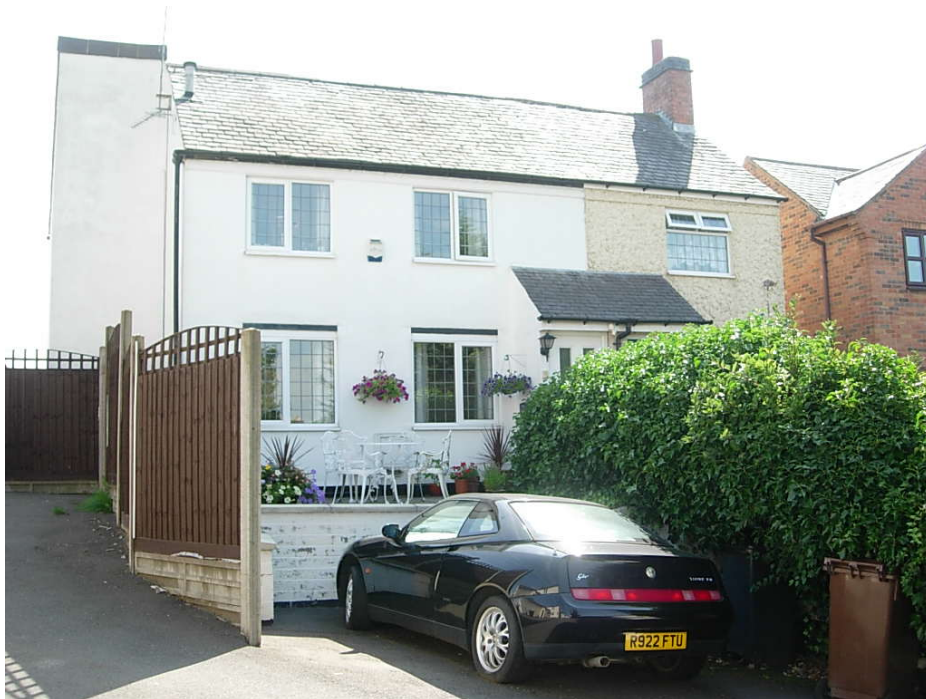
The unity of 9 and 11 Church Lane has been lost due to each dwelling being modernised separately. The two dwellings stand well back from the highway.
