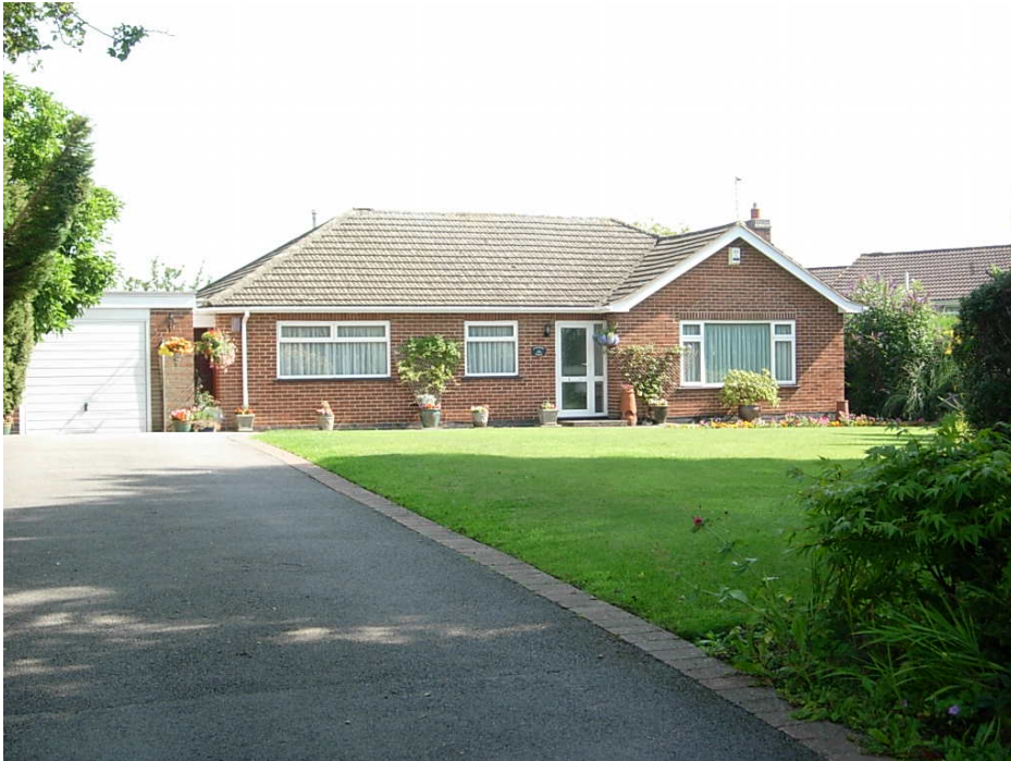
27 Church Lane is a modern bungalow set back from the highway.
