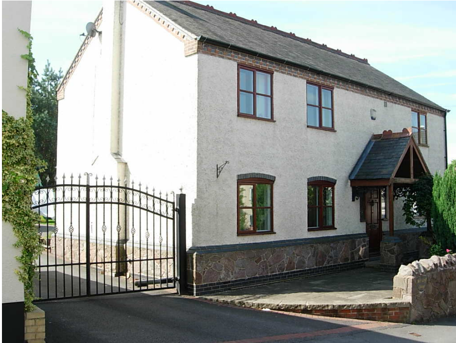
The property 6 Church Lane is a modern detached dwelling with an artificial stone plinth, rendered walls fronted with a granite wall.
