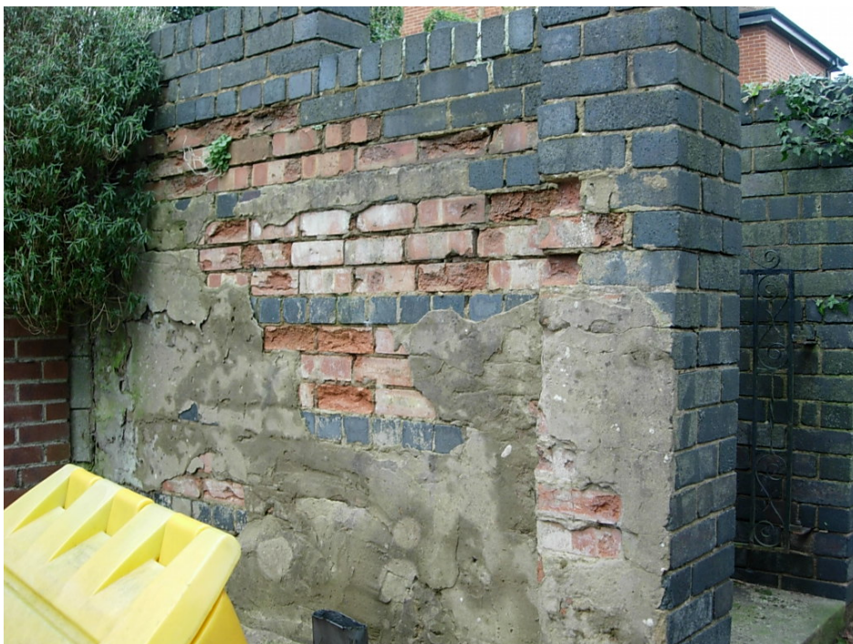
A picture of the brick wall on Berry's Lane before its improvement.
