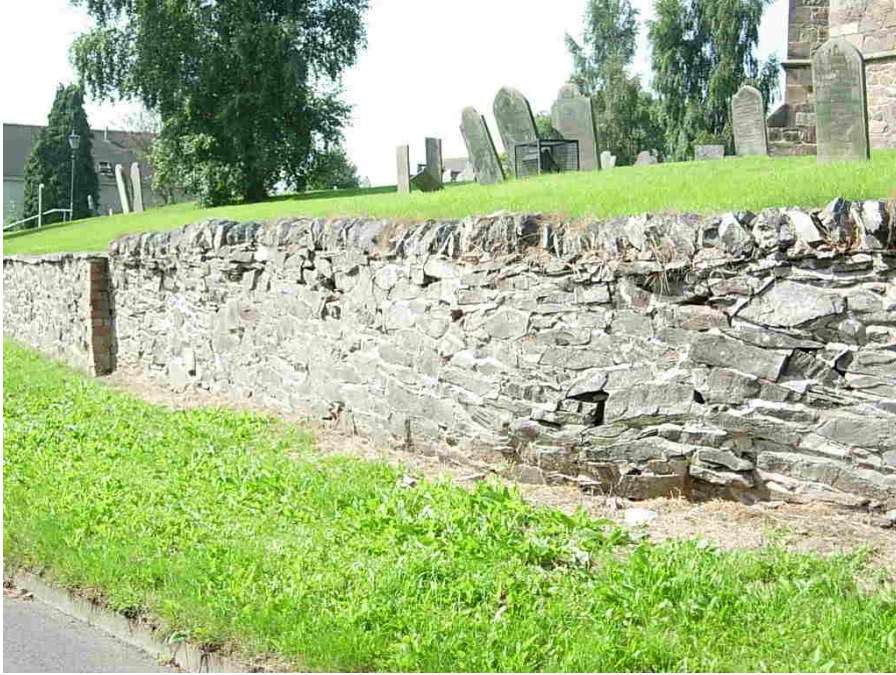
This section of churchyard retaining wall is starting to bulge due to the wet weather but is due to be re-built shortly.
