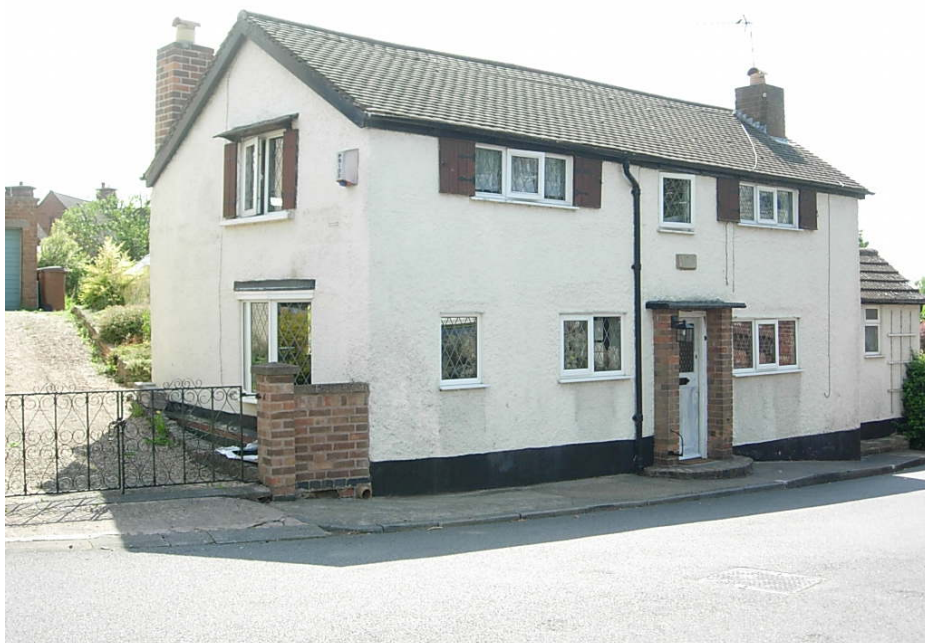
36 Chapel Lane is reputedly believed to be one of the oldest properties in the Conservation Area (thought to be 1675). However, the dwelling has been considerably modernised with plastic windows and concrete roof tiles.
