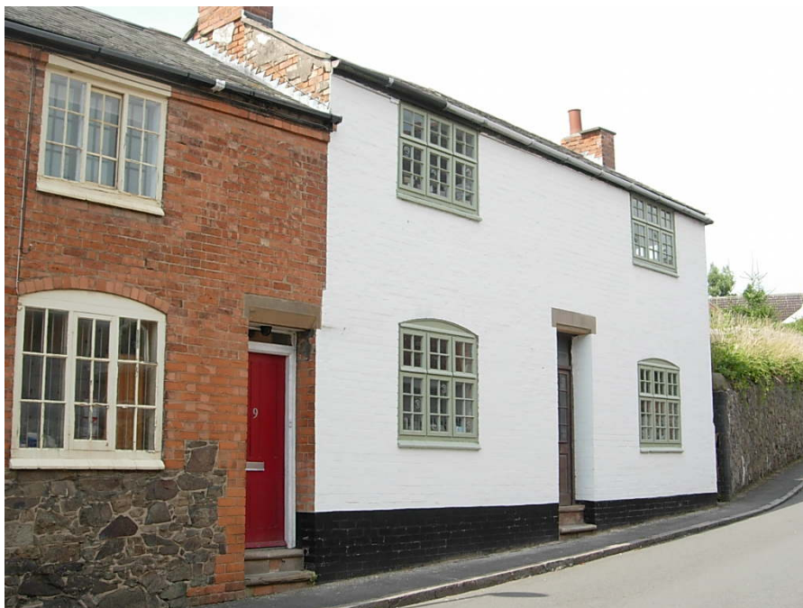
The design of the modern timber windows in the right hand building is overly fussy when compared to the traditional appearance of the windows in the left hand building.
