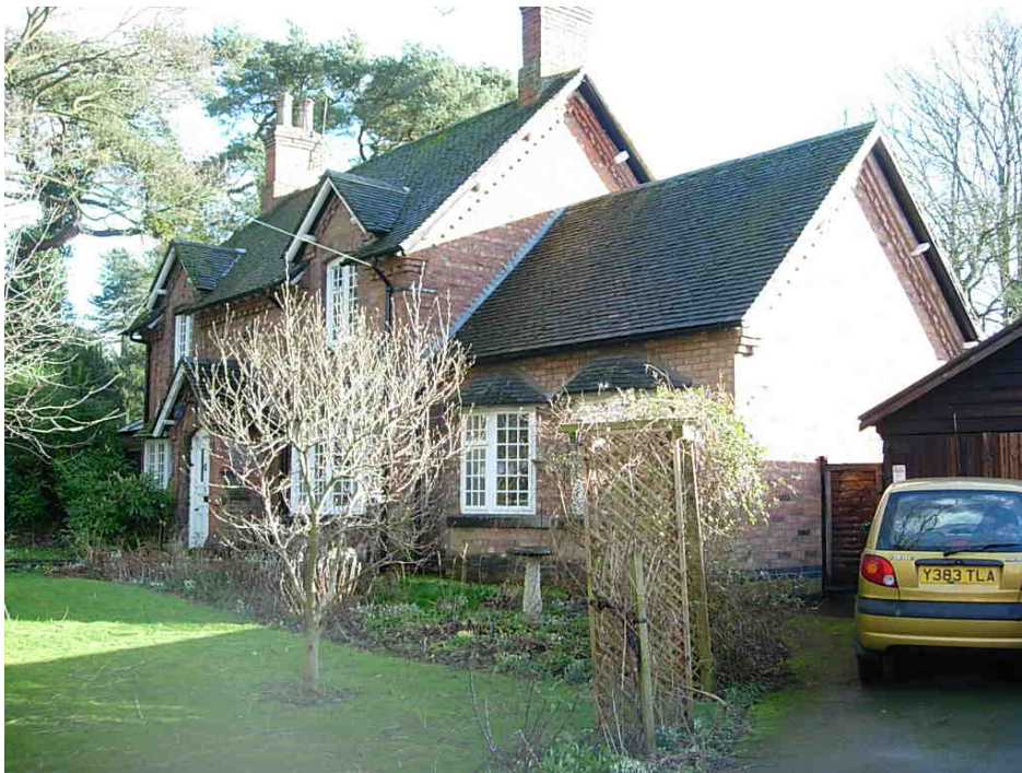
This property on Church Street is a fine example of a period from the late Victorian/Edwardian era.
