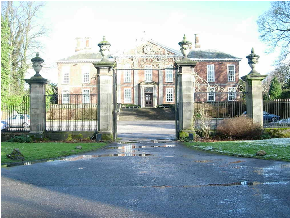
One of the impressive entrance gates to Bosworth Hall Hotel with all the urns intact. The gates would benefit from repainting.
