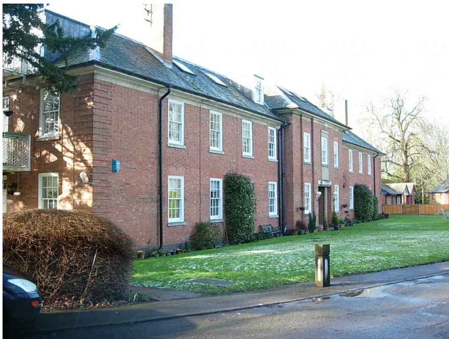
The front elevation of the former nurses flats in the grounds of the Bosworth Hall Hotel.
