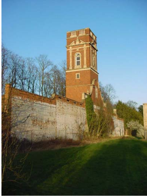
This Watertower is a major landmark visible on entering the Conservation Area. It unfortunately is in desperate need of repair.
