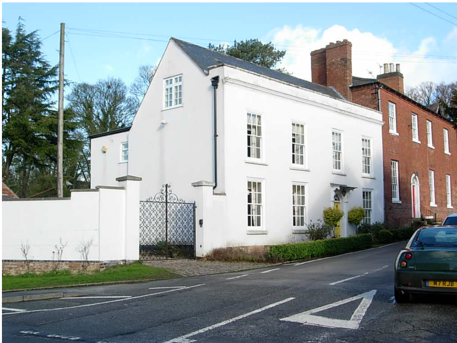
The Grey House is a Grade II listed building. The facade constructed in 1830 covers a timber framed farmhouse.
