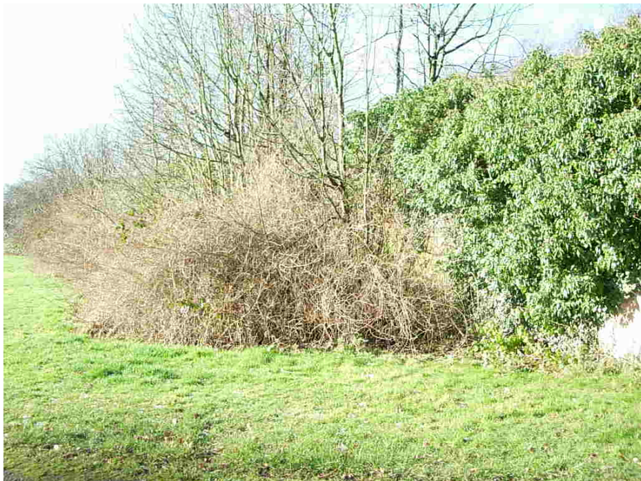
Ivy and self set trees are undermining the stability of the walls around the walled garden. They need to be removed urgently.
