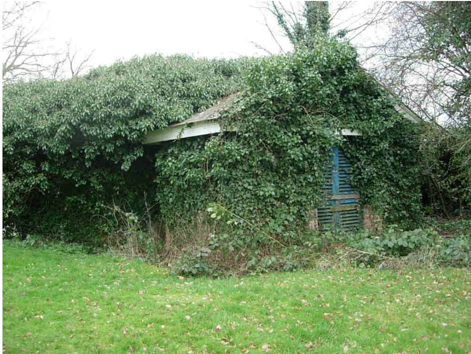
This feature building in front of Bosworth Hall is in need of urgent maintenance.
