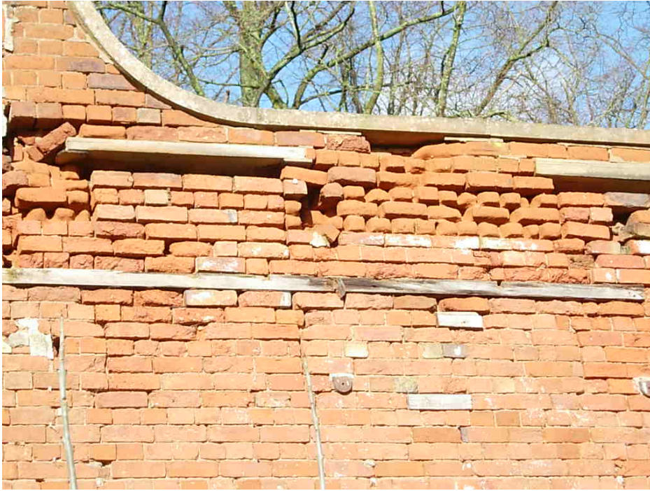
This is an example of the brickwork to the walled garden which is also in need of urgent conservation.
