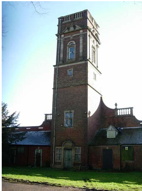
The Watertower, seen from the north, highlights the urgent need for repairs.
