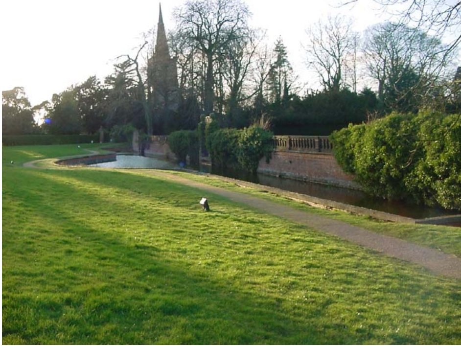
The walls around the garden are becoming over-run with ivy which is damaging the pointing.
