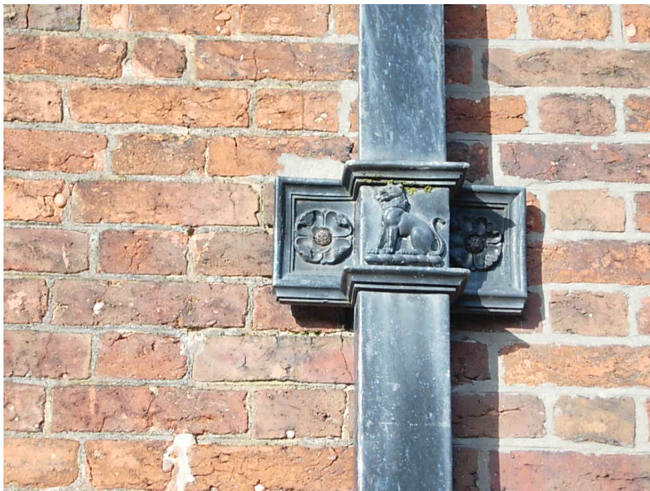
One of the excellent embellished surface water down pipes on Bosworth Hall.
