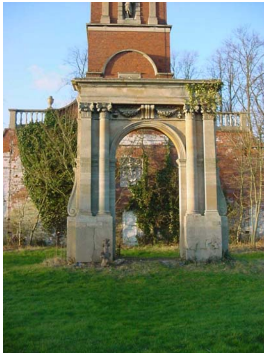
This arch originally formed part of the greenhouses in the walled garden to Bosworth Hall.
