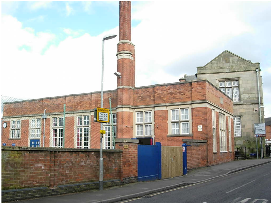
The games hall of the Dixie Grammar School on Station Road which was constructed in the 1930's and was originally intended to have a second storey.
