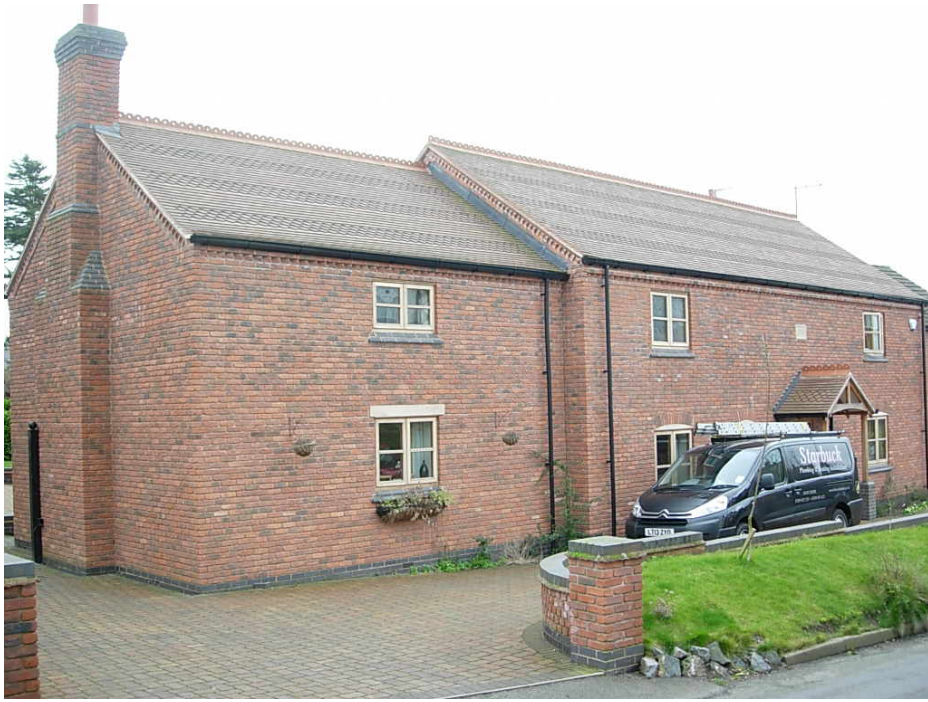
11 Sutton Lane is a very large modern property with an interesting tiled roof.
