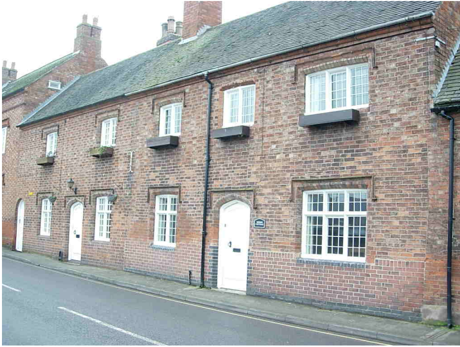
These properties on Station Road are of a higher status having pointed arch entrance doors and hood moldings to both windows and doors. Both properties are Grade II listed.
