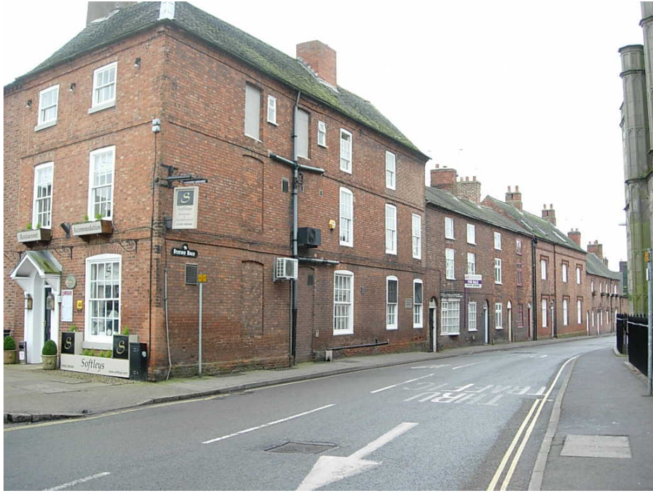
This view along Station Road highlights the differing status of buildings in the terrace.
