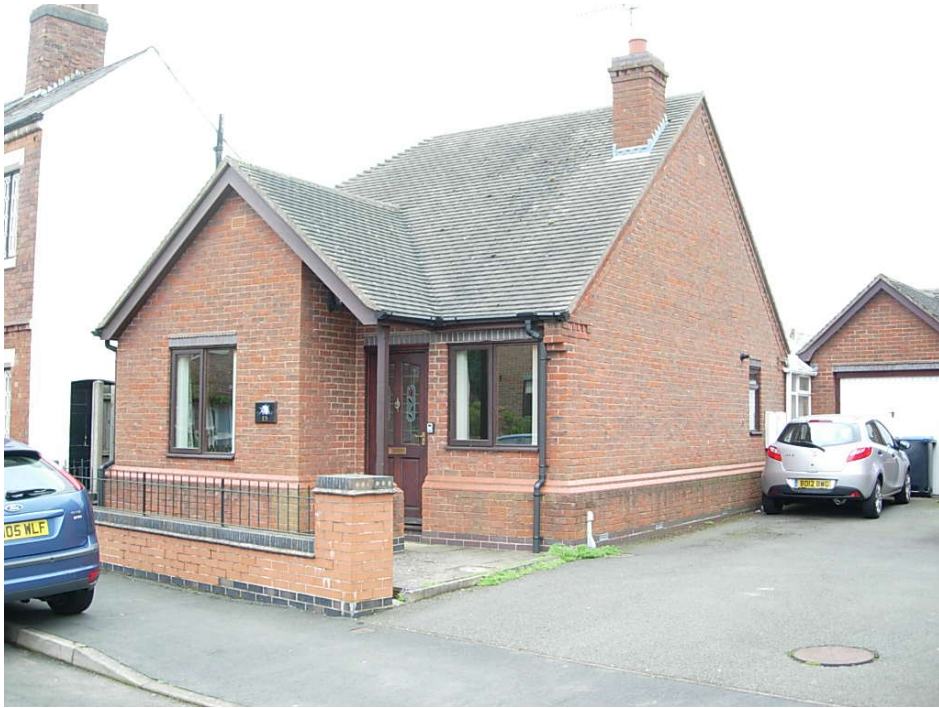
A further late C20 Property on Warwick Lane.
