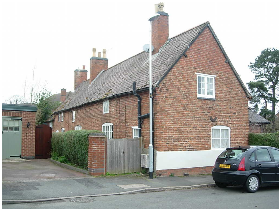
This is the rear of 4 Southfield Way and emphasises its simple form.
