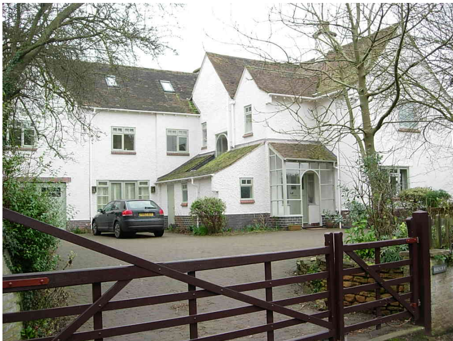
23 Sutton Lane has had a massive extension which detracts from its original form.
