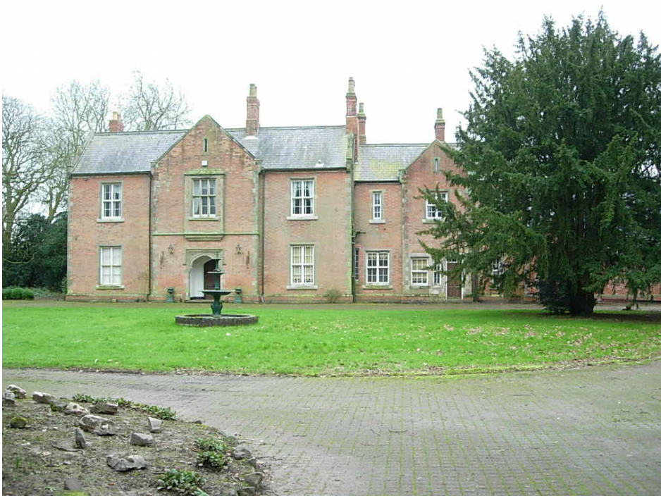
The Old Rectory is a fine substantial Grade II building set in very impressive grounds.
