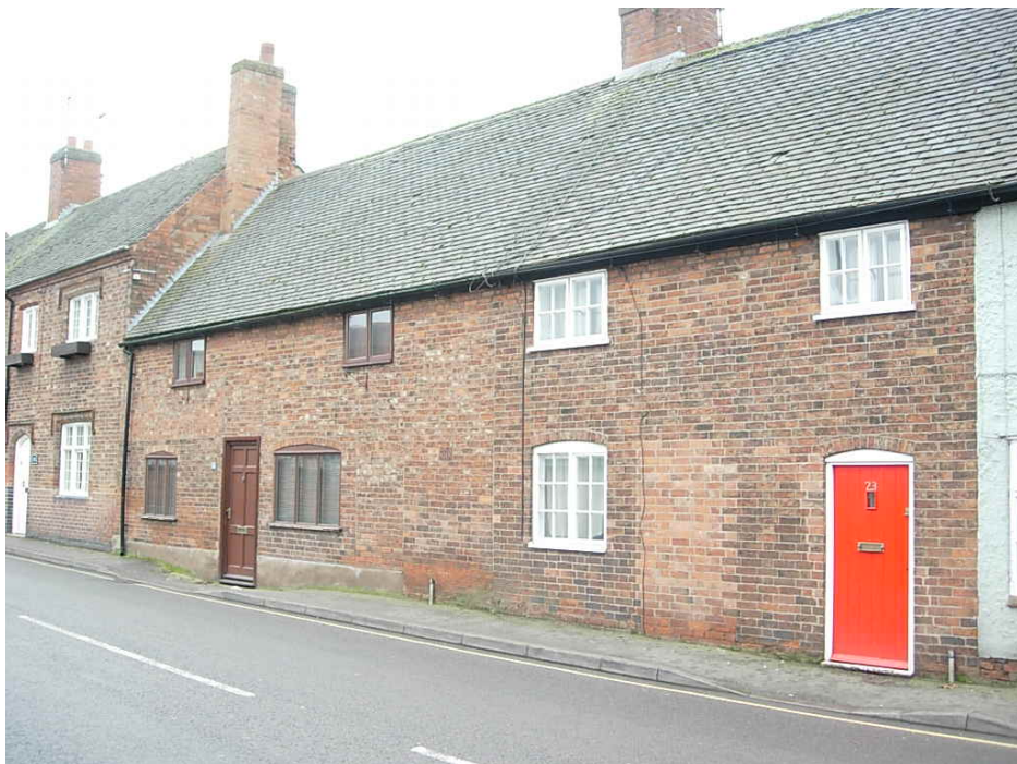
This is an extension of the same terrace on Station Road. It is possible to see where the doors have been bricked up to allow properties to be linked. They are Grade II listed.
