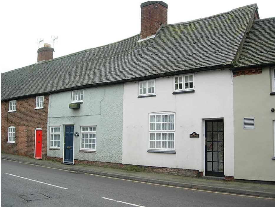
These vernacular properties form part of a long terrace on Station Road that are believed to have been occupied by framework knitters in the C18 and C19.
