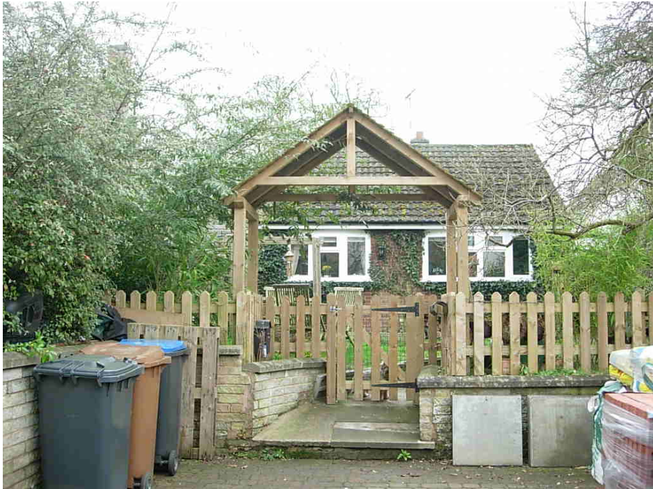
21 Sutton Lane is a small bungalow that has little traditional character.
