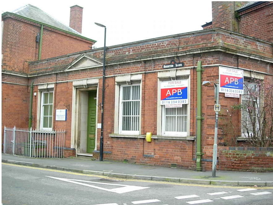
The former police station, although single storey, is an architecturally attractive building at the entrance to Shenton Lane.
