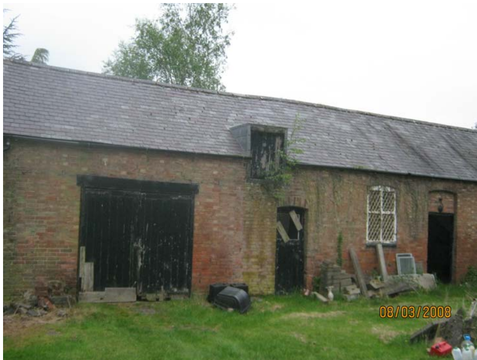
The Coach House is in a very poor state of repair and needs urgent repairs.
