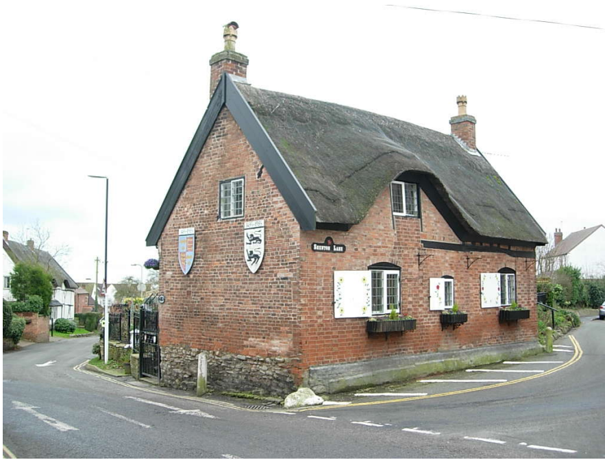
Rainbow cottage on Shenton Lane marks the end of the Market Place and is a C17 timber framed building.
