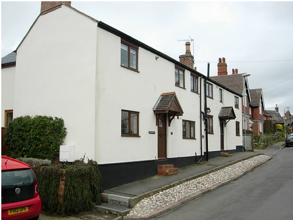
12 & 14 Sutton Lane are a pair of vernacular houses that stand up on a plinth above the road. The Borough Council carried out an enhancement scheme fronting the two properties constructing granite kerbing along the carriageway and laying cobbles as a decorative feature.
