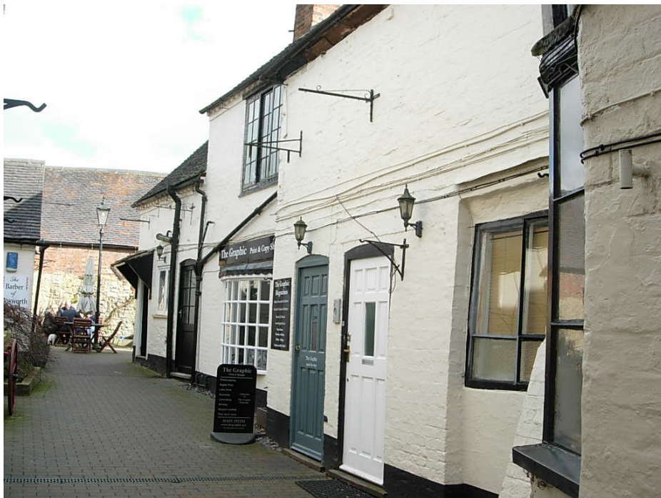
Wheatsheaf Courtyard. There is C16 timber framing of post and truss construction in the rear wing.
