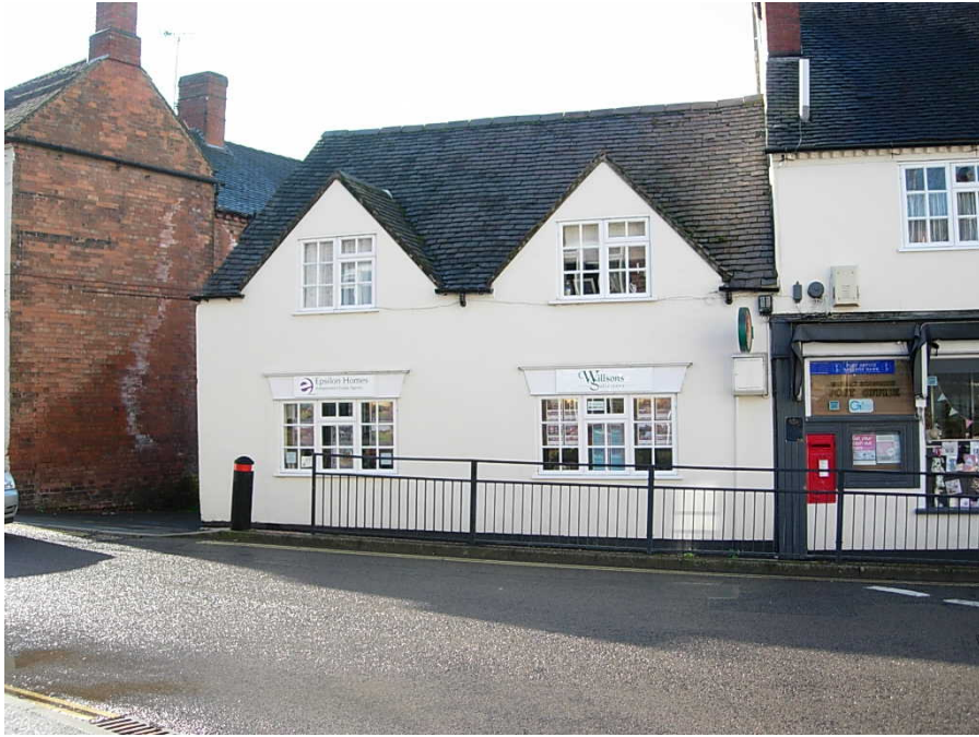
15a Main Street is an example of a simple vernacular building which adds to the street scene.
