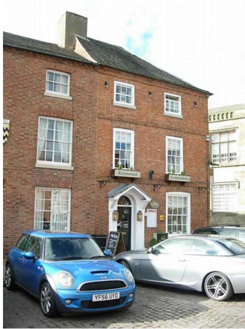
2 Market Place is Grade II listed and dates from the late C18. It is a fine historic building at the entrance to the Market Place.
