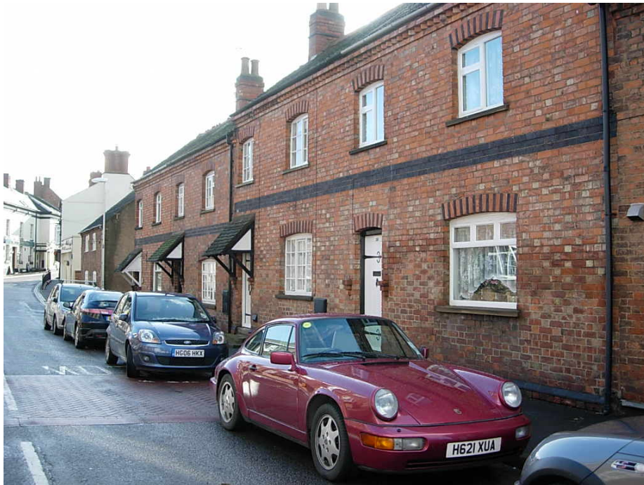
29-35 Main Street has polychromatic brick segmental arches which compliment the blue brick string course.
