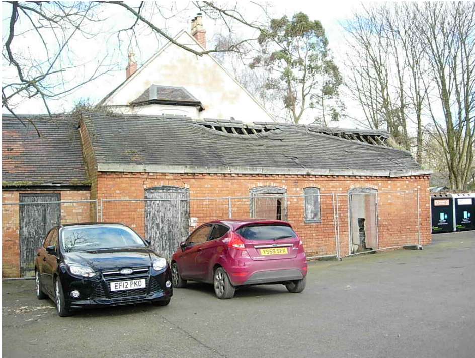
The out buildings to the Old Black Horse are important cartilage buildings but are urgently in need of repairs.
