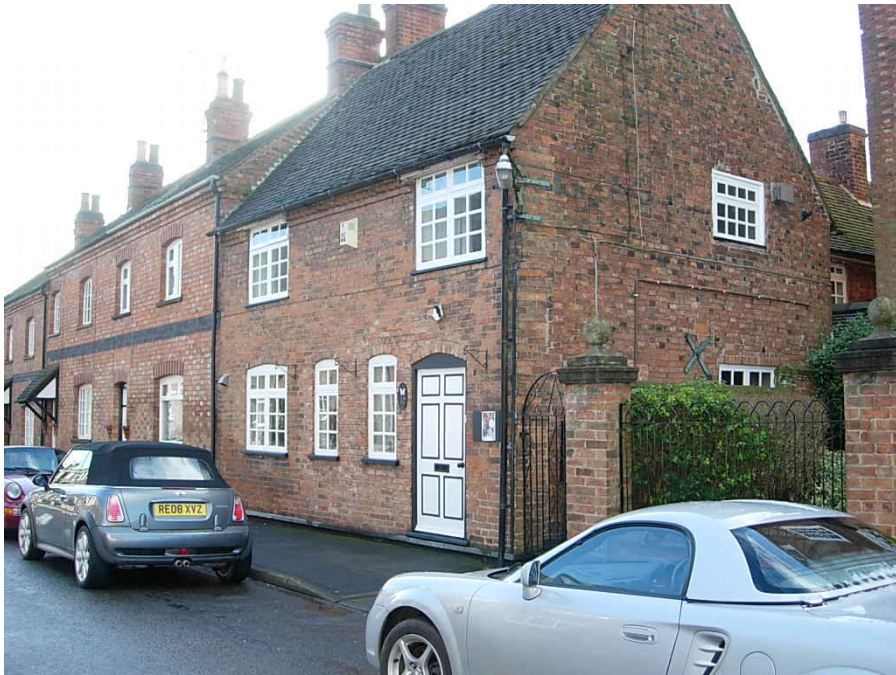
37 Main Street is likely to have had an original window replaced by a door on its street elevation.
