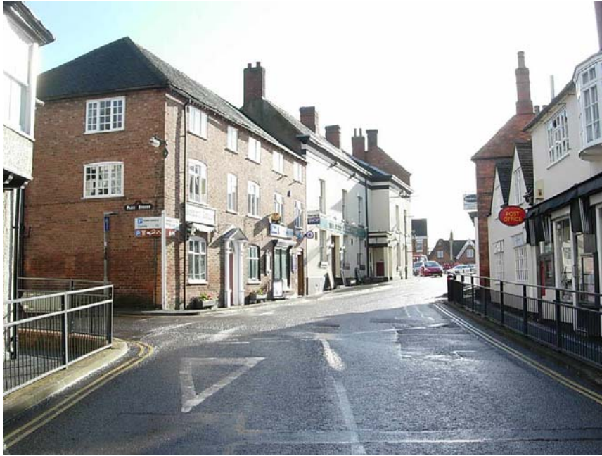
This view along Main Street highlights the importance of chimneys in the street scene.
