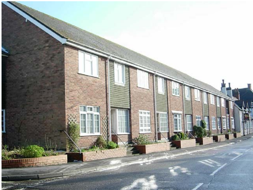
18-28 Main Street. This modern terrace replaced a historic terrace of framework knitter's cottages which were demolished in the 1960's.
