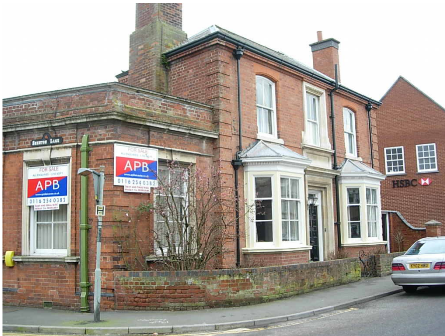
28 Market Place. This building is not listed but is a fine example of a late C19 property.
