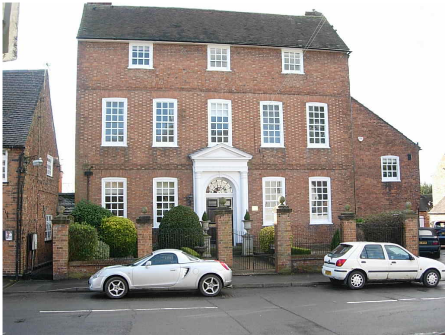
39 Main Street is a Grade II* listed building dating from the early C18. It had an additional floor added in the late C18.
