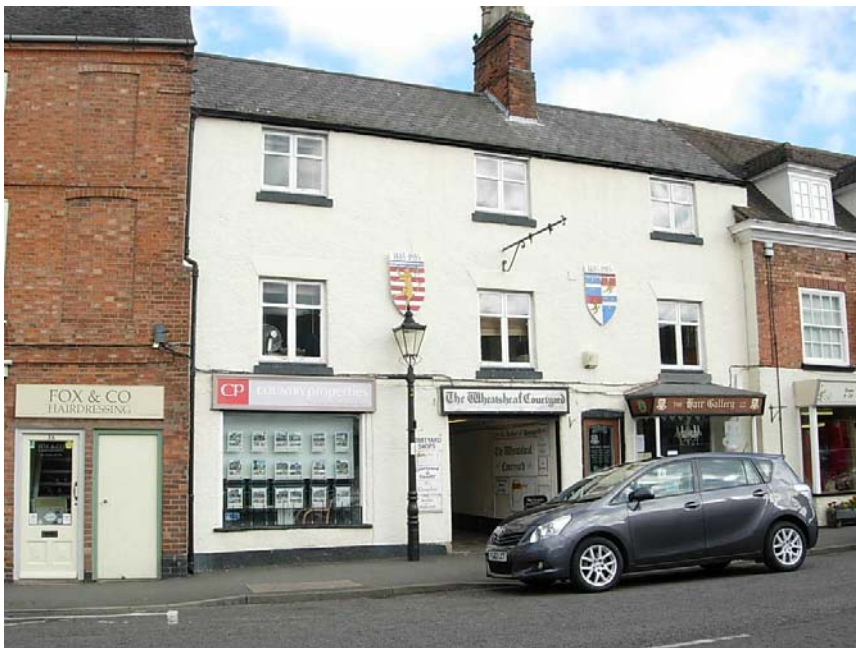
5 and 7 Market Place. These are also Grade II listed. The building was formerly an inn and has a central entry to a rear courtyard.
