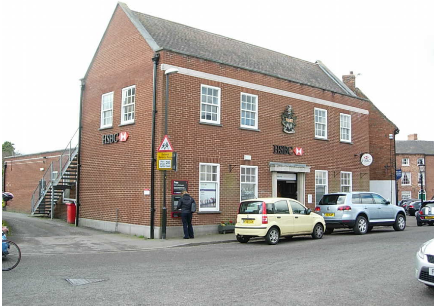
22 Market Place. This is a very simple modern building which although it has rectangular windows with a vertical emphasis, it lacks character.
