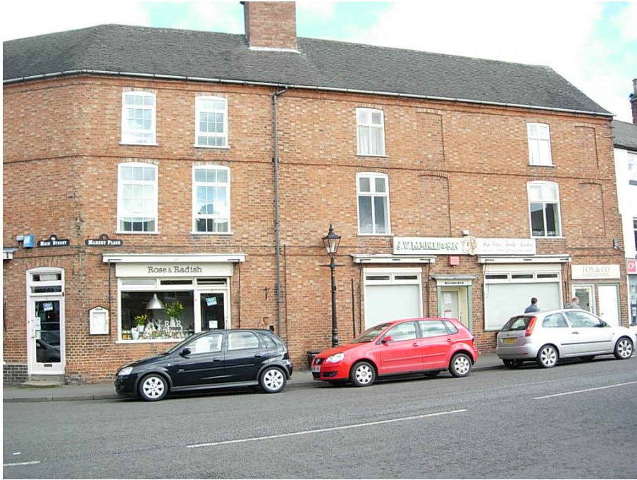
1, 3 and 3a Market Place are all Grade II listed. Unfortunately No. 3 has had non-traditional windows installed.
