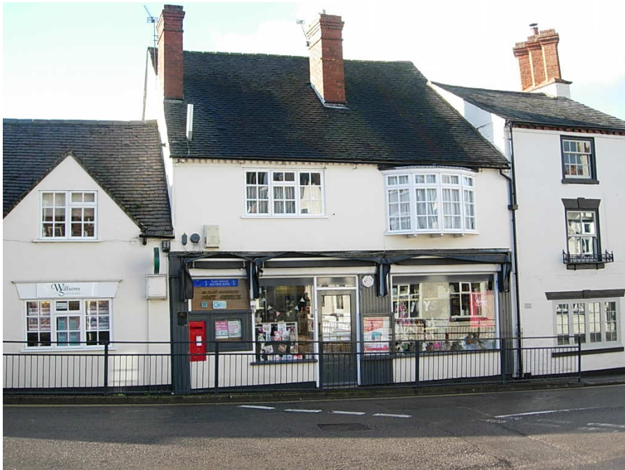
The appearance of 19 Main Street is spoiled by the plastic bow window at first floor.
