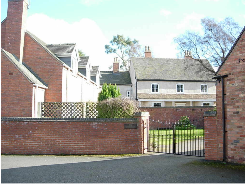
The modern property 10 Park Street is set back from the carriageway off a private drive.
