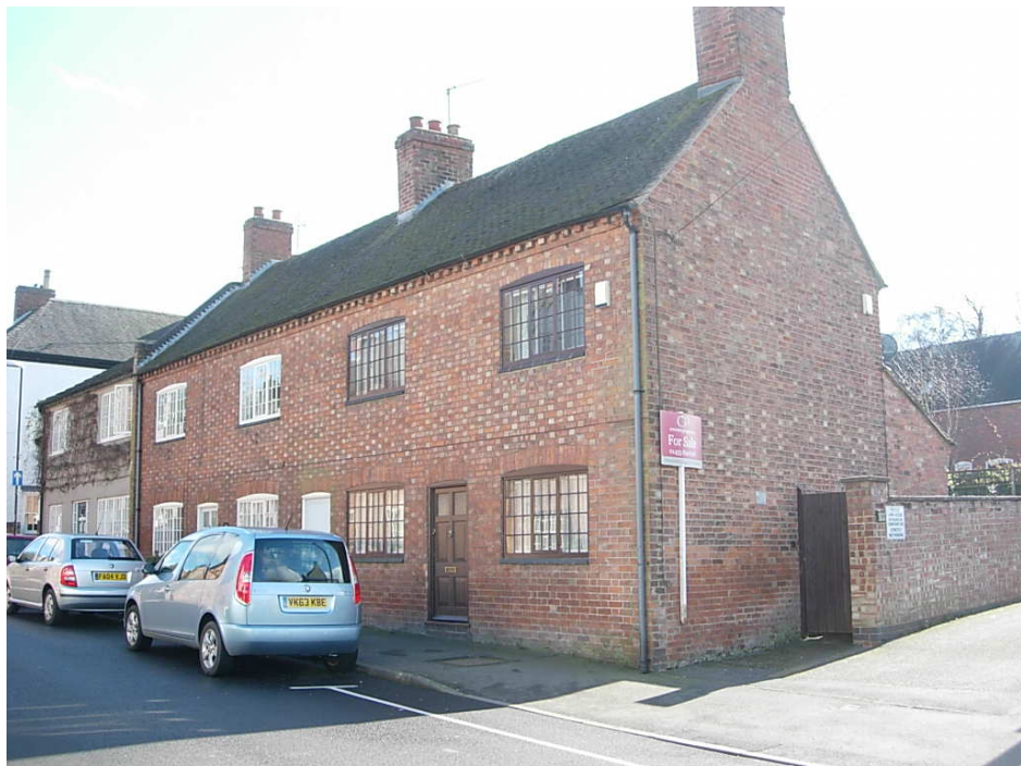
12 – 16 Park Street is a fine structure which has retained its chimneys and segmental arched lintels.
