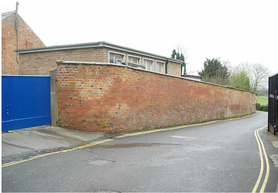
The traditional brick wall running down Back Lane directs views into open countryside
