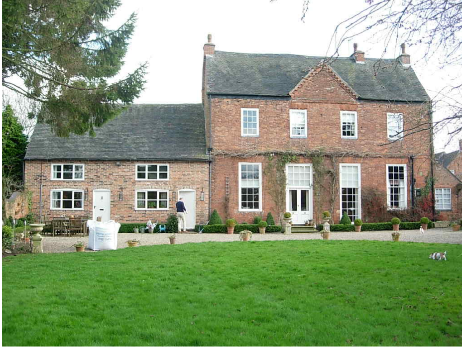
The excellent Grade II Listed 'Old Club House' is a late C18 two storey property built in brick with a plain tiled roof.
