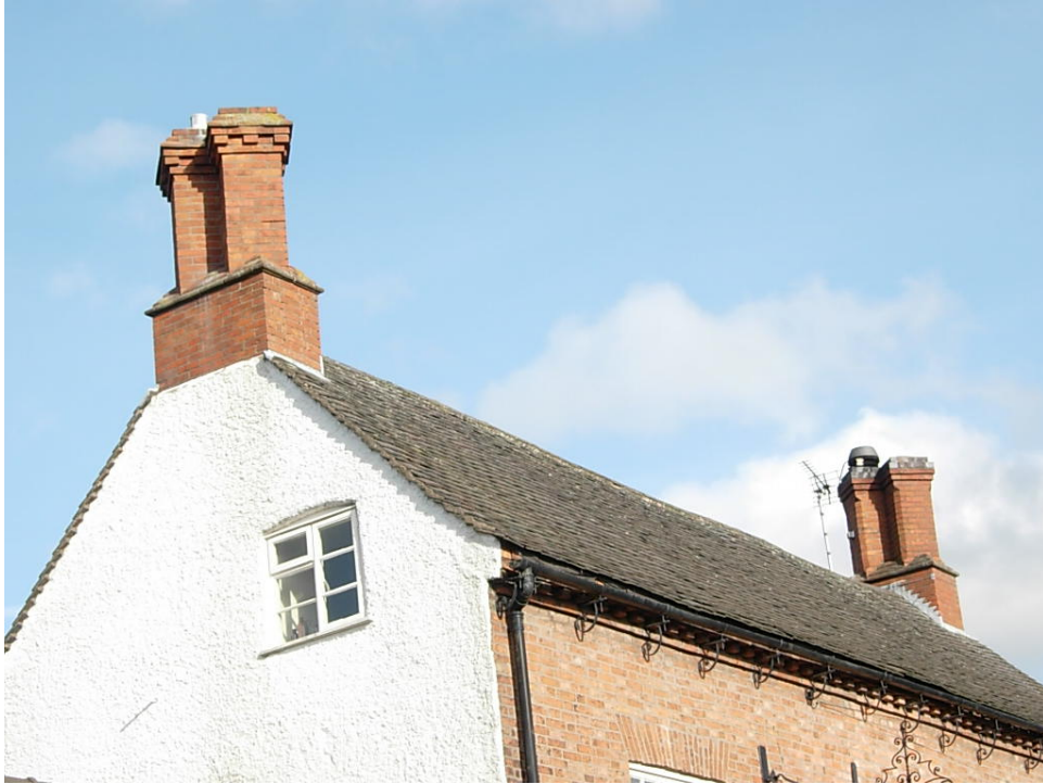
The decorative chimney stacks are an attractive feature on the property at 15 Park Street.
