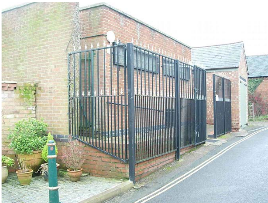
The iron railings fronting the public toilets on Back Lane are a poor visual feature that does little to enhance the Conservation Area.
