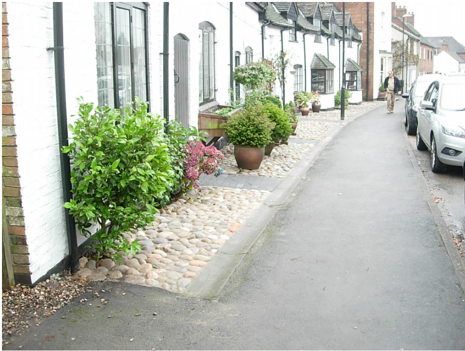
The frontage to the properties 24 – 30 Park Street was improved by the Borough Council as part of a joint scheme with residents and money from the Market Bosworth Millennium Fund.
