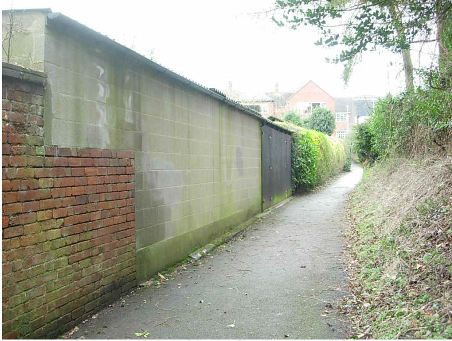
The materials to construct these out buildings spoil the setting of this pleasant footpath.
