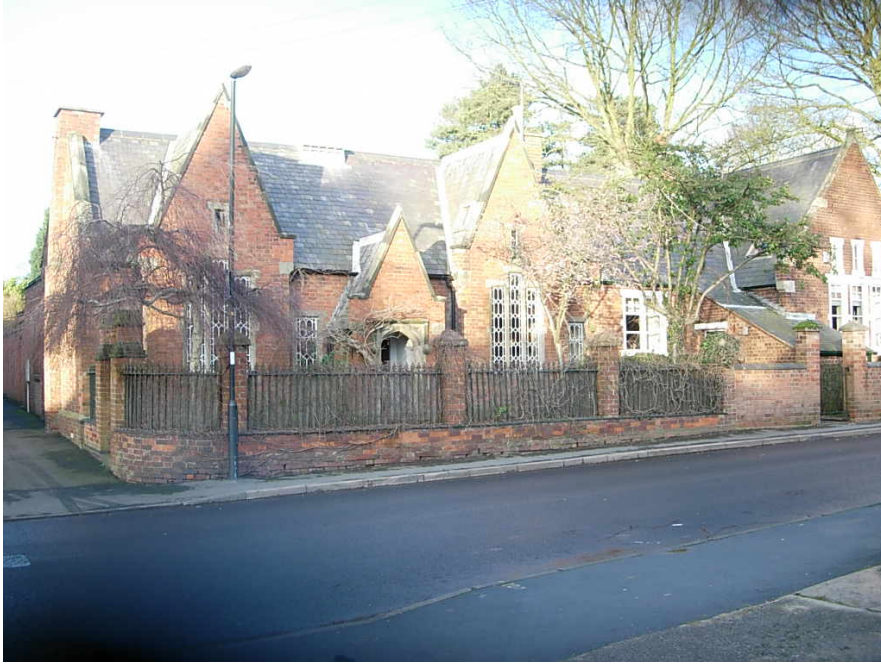
37-39 Park Street was formerly the Church of England School constructed in 1848 with a later C19 addition to the east and is Grade II listed.
