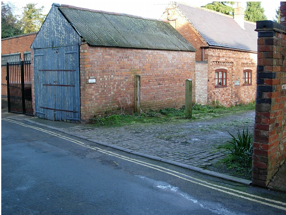
Consideration should be given to replacing the corrugated iron roof with a slate roof on the Coach House and out buildings on Back Lane..
