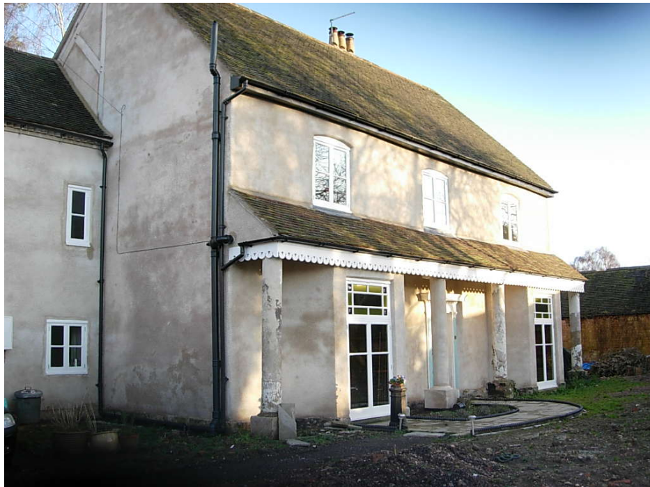
22 Park Street has been derelict for several years but is currently undergoing renovation.
