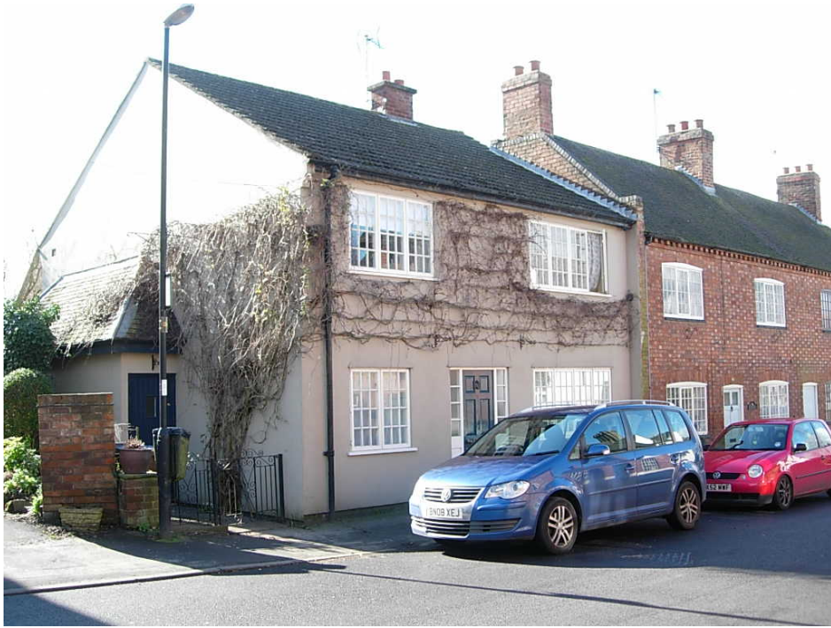
The insertion of overly large first floor windows at 20 Park Street are out of character and scale with the property.
