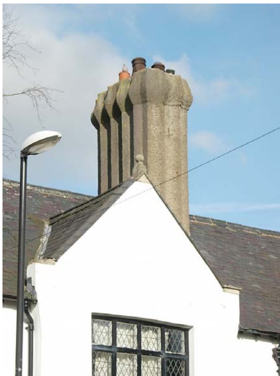
The impressive chimney at 9 and 11 Park Street.
