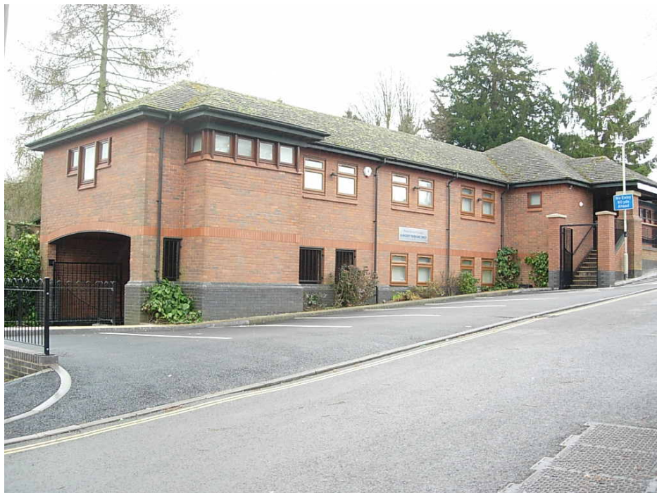
The large modern surgery sited at the western end of Back Lane is a visually dominant building.
