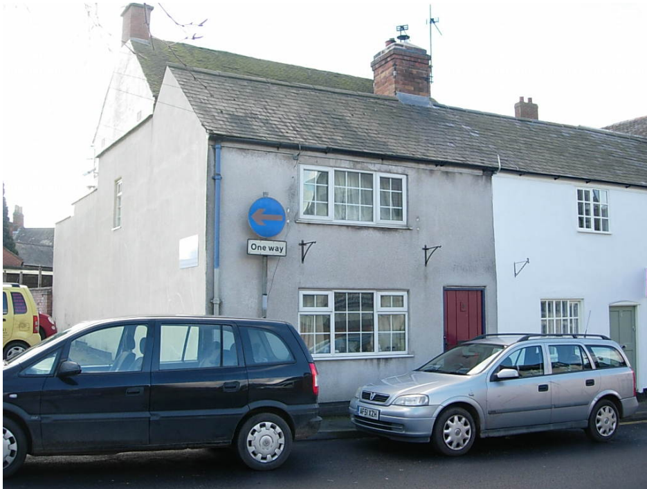
The design and size of these large windows inserted at 6 & 8 Park Street are out of character with the building.
