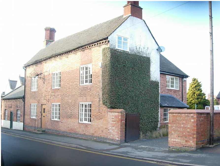
15 Park Street is a fine vernacular building with a simple elevation which includes Yorkshire light windows.
