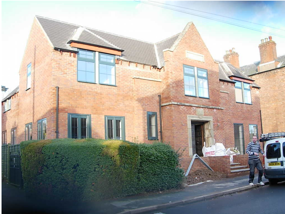
This new frontage building on St Peter's Church Hall has heavy unattractive windows but the general design is acceptable.
