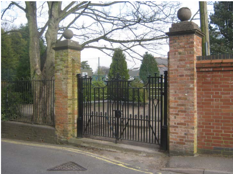
Repairs have been carried out to the rear entrance gate and piers to the Dixie Grammar School on Back Lane.
