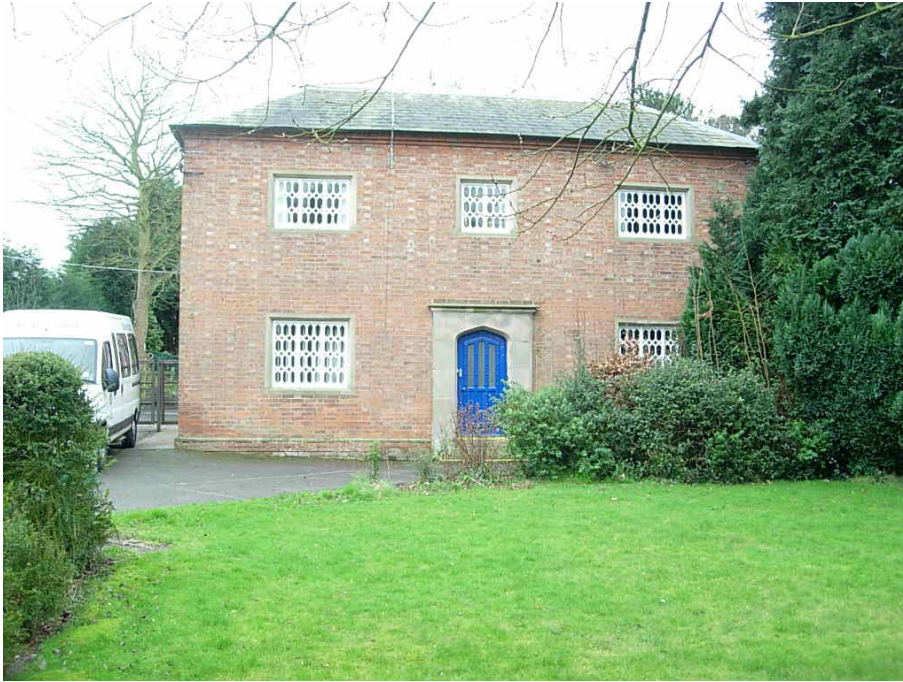
This fine building, constructed in 1828 as the Dixie Grammar School's Under Master's residence, is curtilage listed being sited in the grounds of the Dixie Grammar School.
