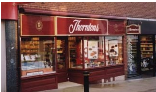
Recessed doorway with ramped non slip entrance
