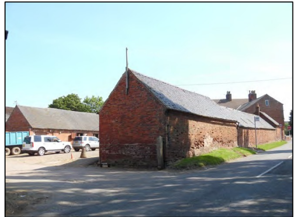
Figure 35 Barns at Elmside Farm
