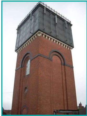
Hinckley Water Tower, constructed 1889. A likely inclusion within a local heritage list
